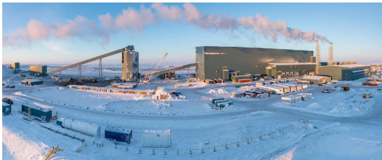
Photo 02: Meliadine Process Facility Complex (February 2019)
