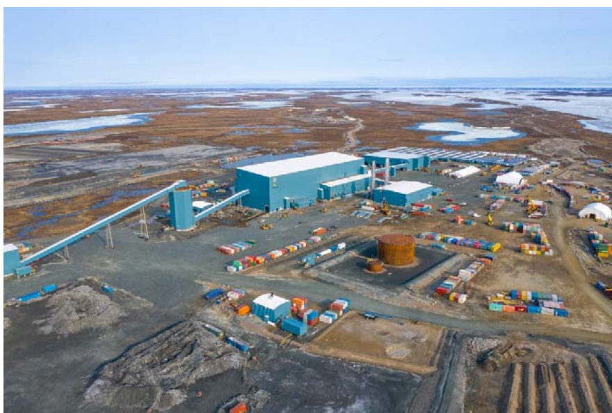
Photo 04: Meliadine site complex, looking northwest (June 2019)
