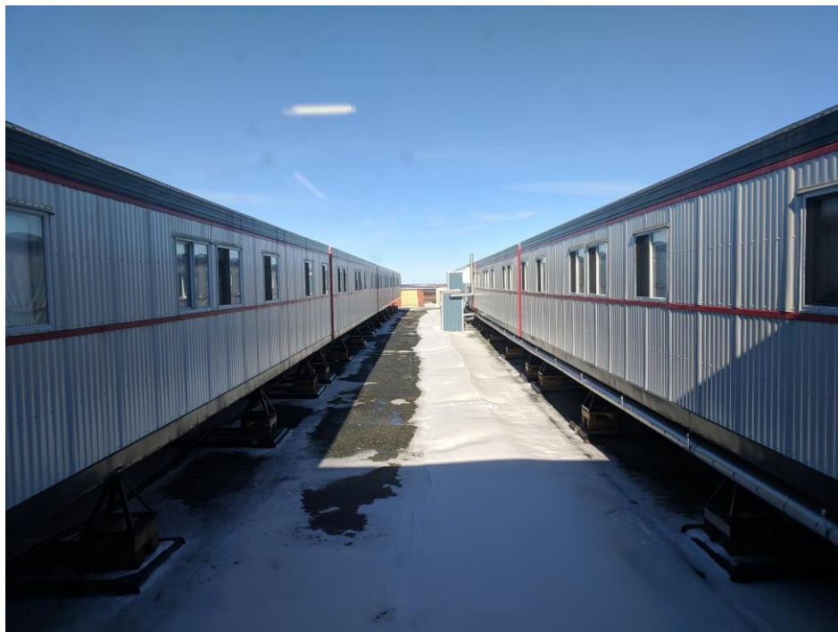
Figure 3: Snow removal from between camp accommodation trailers
