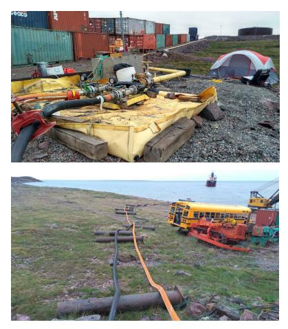
Photo 1: Diesel Transfer - Connection between shipper transfer hoses and Agnico permanent pipeline
