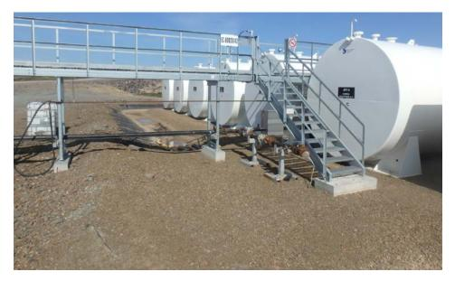
Photo 2: Jet-A Transfer - Connection between shipper transfer hoses and Agnico permanent pipeline
