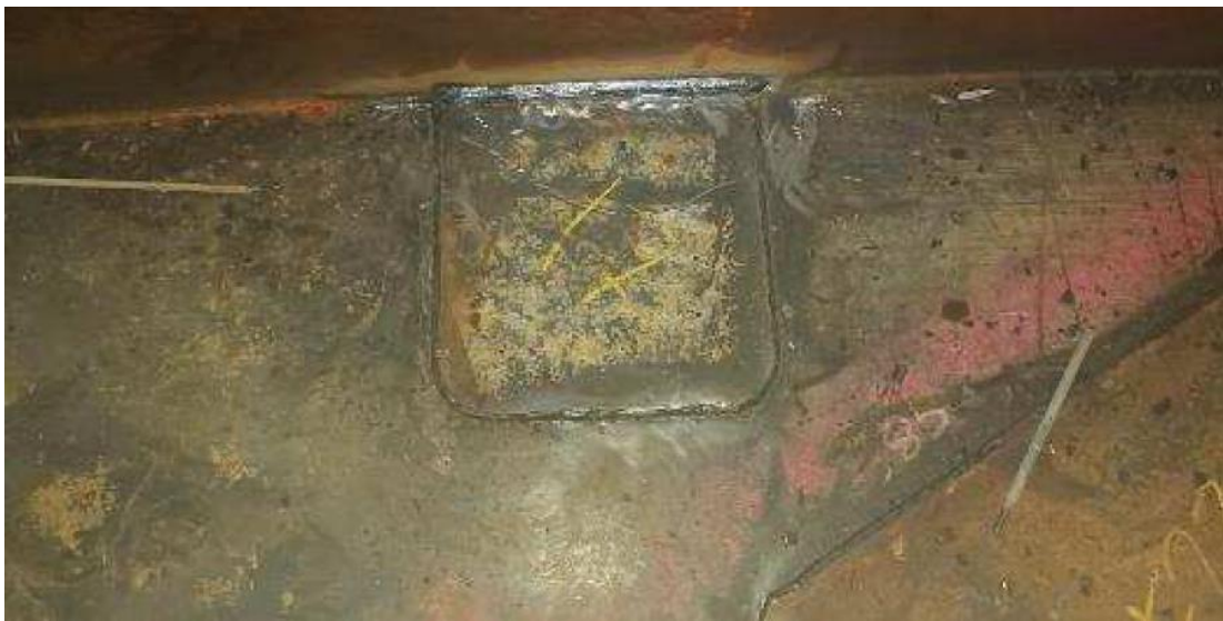
Patch plate over hole inside Fuel Tank #5
