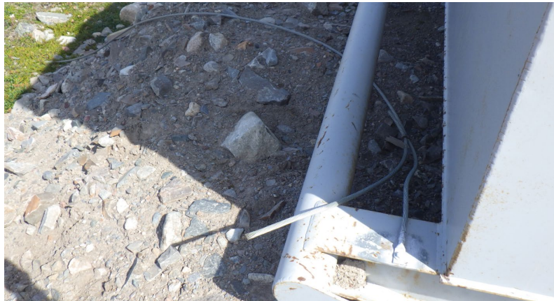
Figure 3-5 Surface Explosive Magazines – Grounding
