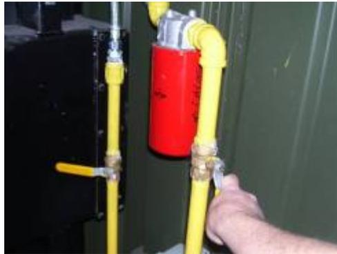
2. Unscrew the used filter. Use a bucket to catch the surplus fuel when you unscrew the filter.
