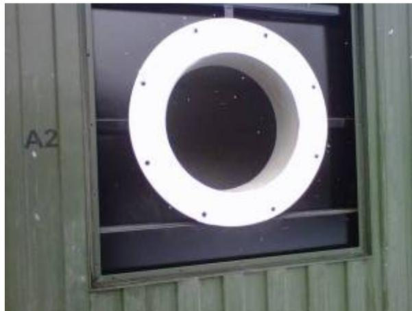
**Correctly Installed Gasket**
