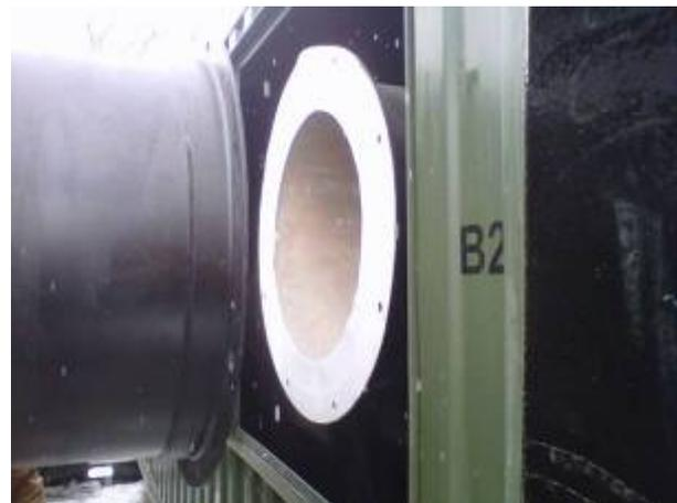
**Correctly Installed Gasket**
