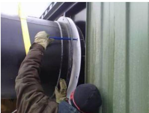
3. Once breech flanges are aligned and together bolt flanges together using the numerical order described in the pattern below using hardware provided.
