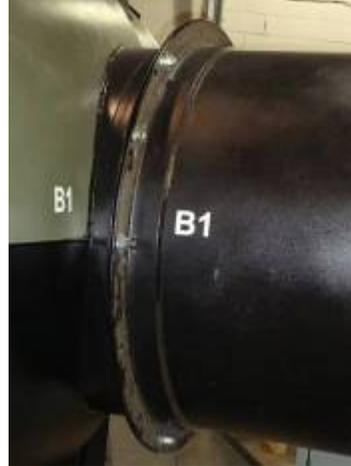
**Correctly installed Breech on Secondary Chamber**
