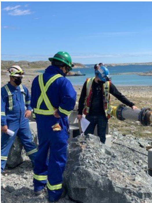
Photo 4: Reviewing the ship to shore procedure ensuring secondary containments are placed under each connection joint.
