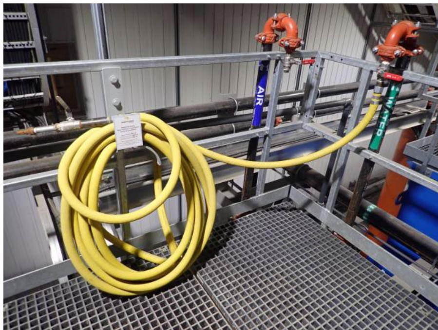
Figure 2: Zoom in image of the EWTP and photos of the MEL-14 sampling port inside the building (end of the yellow hose).
