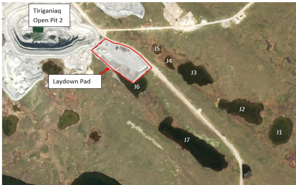
Figure 19: Laydown pad satellite image
