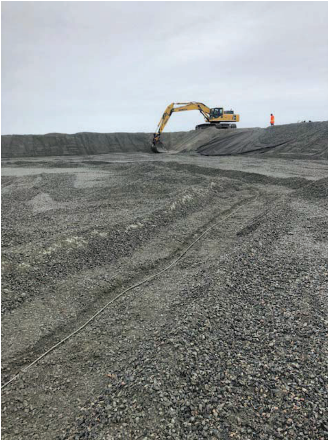
Pad and Berm construction
