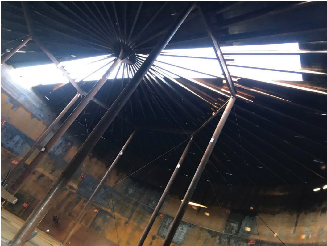
Tank roof structure
