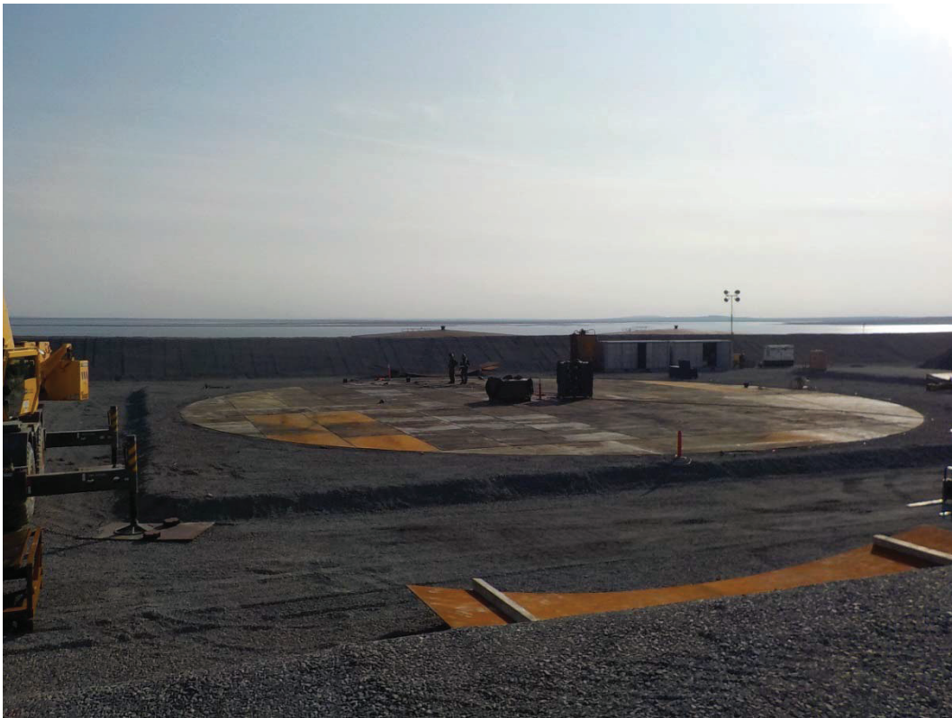
Tank floor construction
