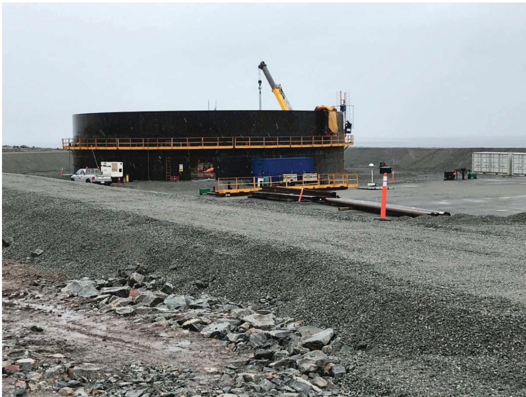
Tank wall welding
