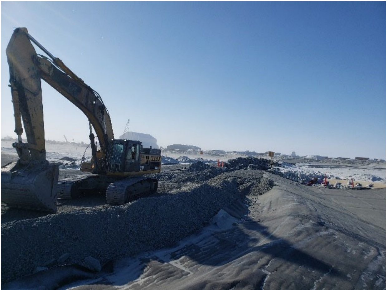
Figure 6. IVR Dike Construction, April 25, 2021. Looking south from Sta. 0+080. CAT excavator placing Zone 2A(FF) over installed geotextile.
