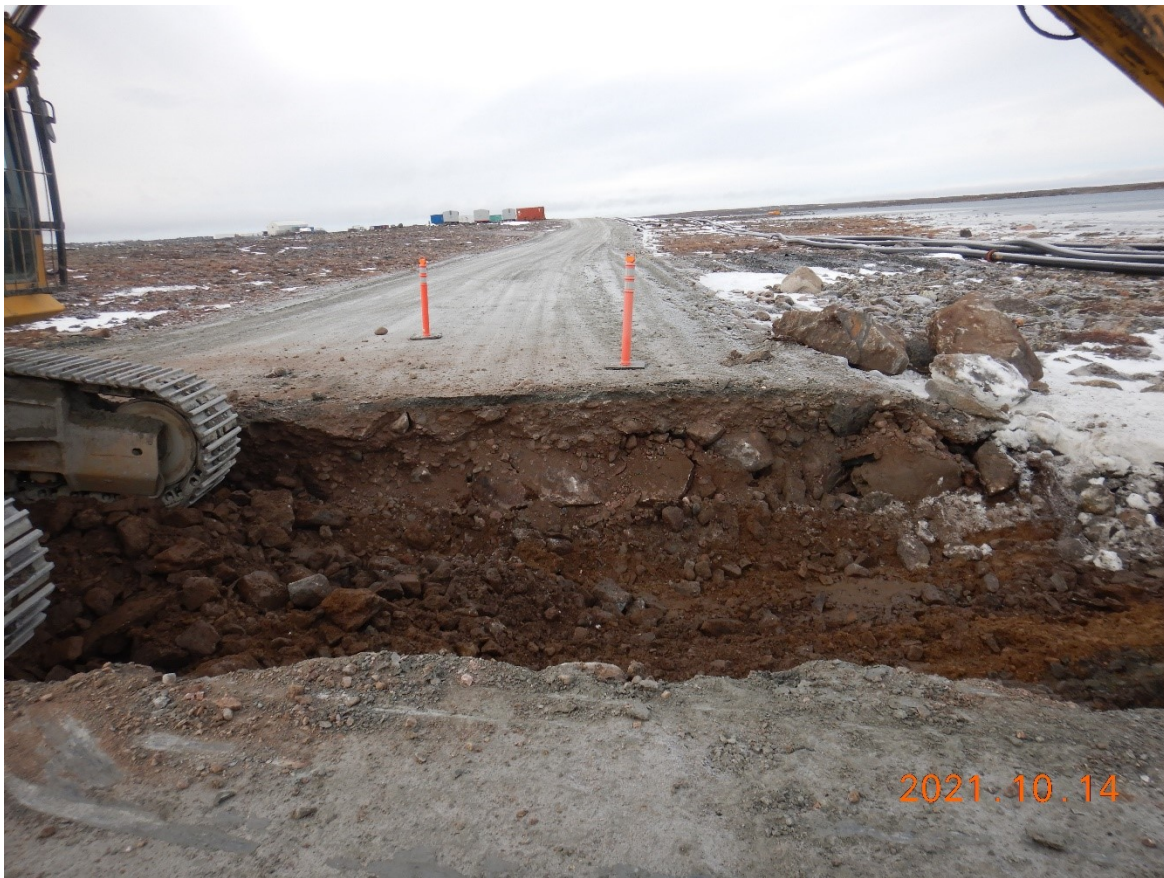
Figure 9. Culvert 22-2 construction - excavation phase. Looking west (Mammoth Lake on the right).
