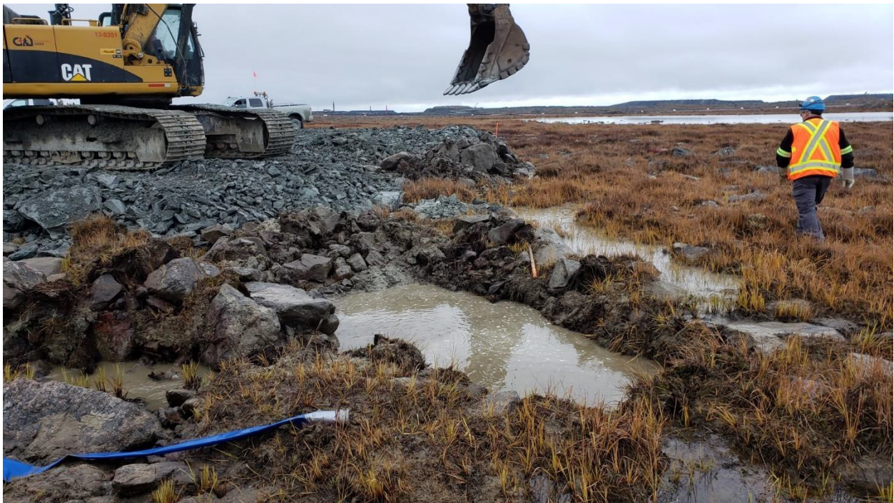
Figure 23. Excavation of a temporary sump, which was directed to mine site water management infrastructure.
