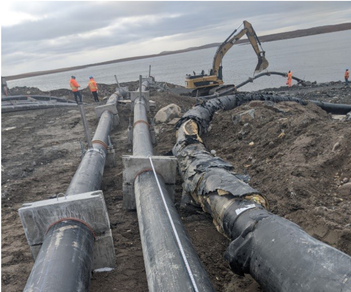
Figure 12. Onshore diffuser assembly work in progress (pipe on the right is unrelated to the diffuser installation project).
