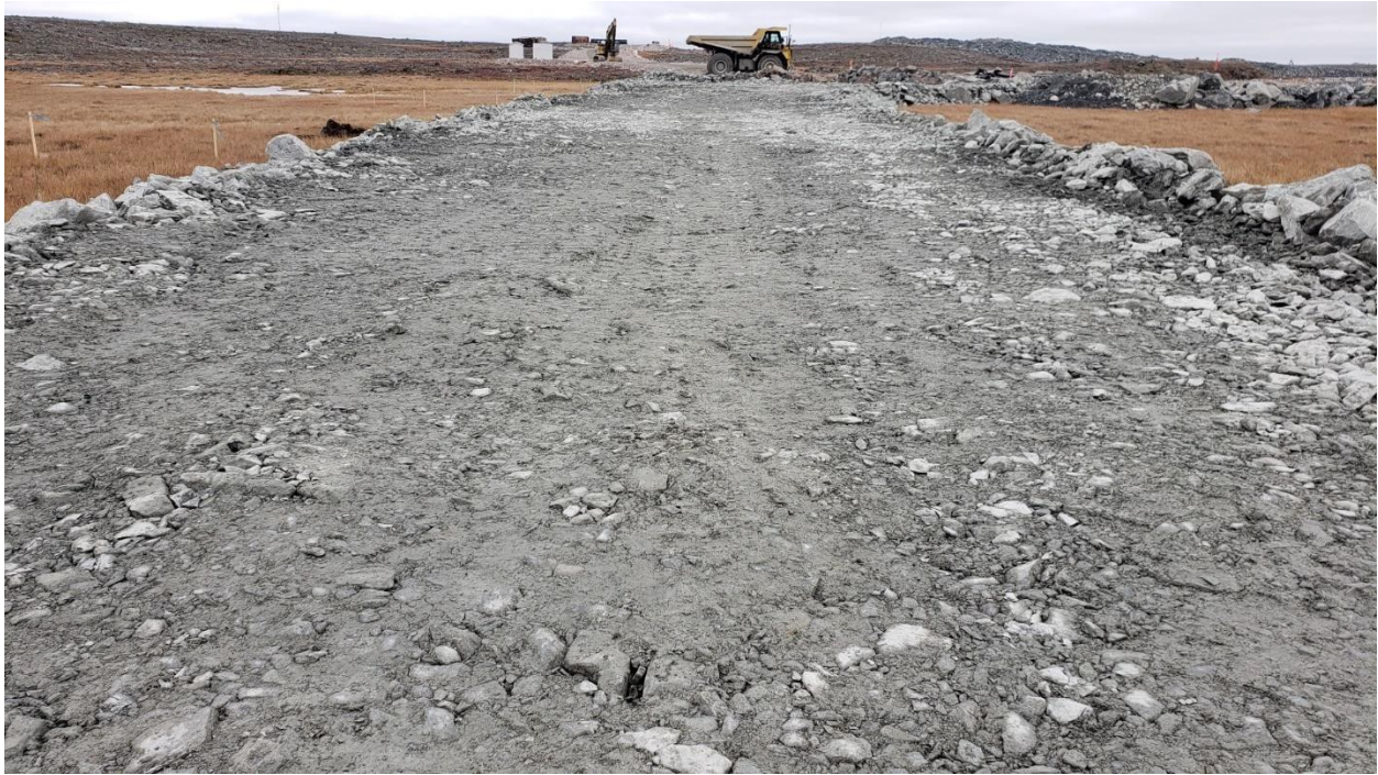
Figure 22. First lift of the IVR Diversion Channel berm construction, looking south.
