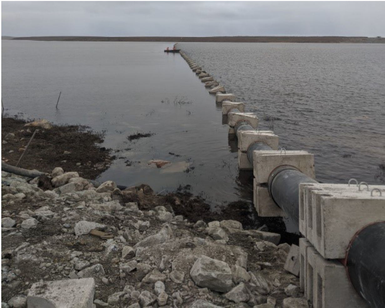
Figure 13. Final alignment of the diffuser in WTS prior to sinking.
