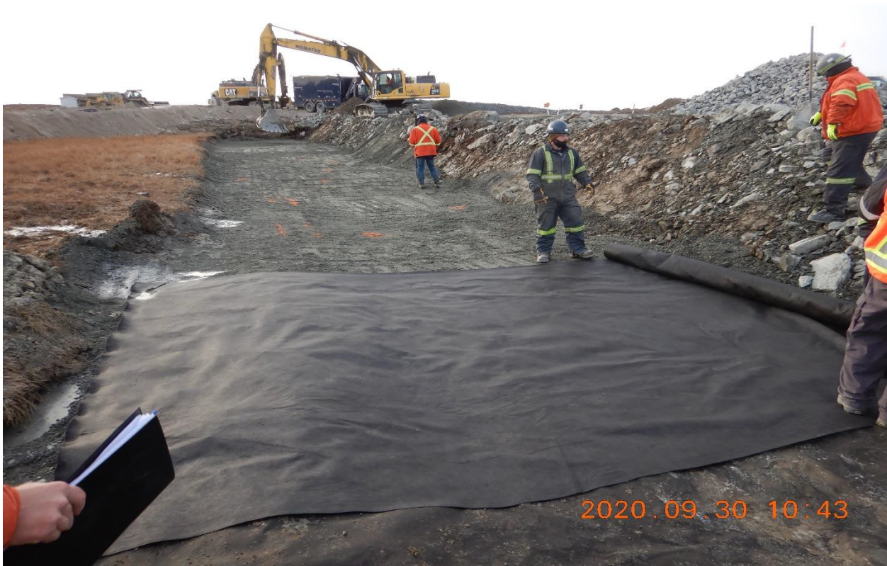
Figure 25. IVR Diversion Channel geotextile installation.
