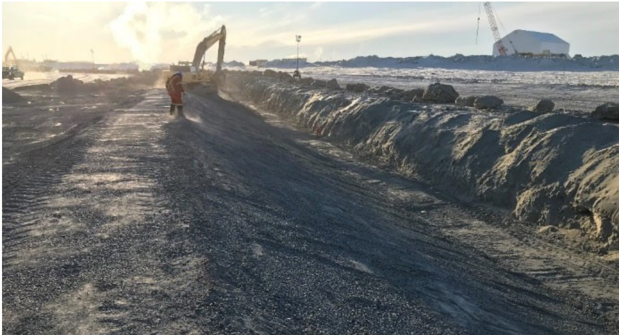
Figure 5. IVR Dike Construction, March 15, 2021. Looking east from Sta. 0+170. Approved surface for liner placement.
