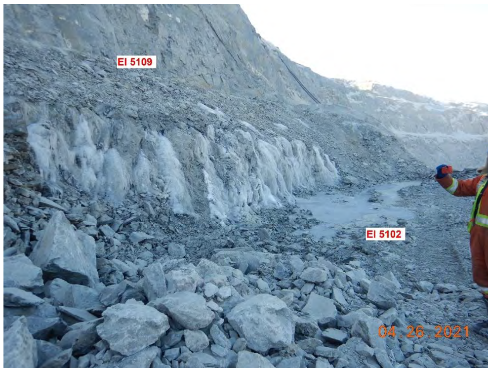
Photo 5: Pit seepage along south wall, looking southeast (April 26, 2021).
