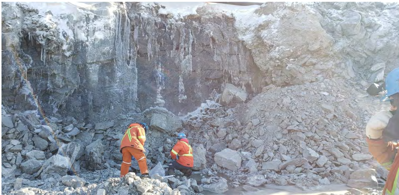
Photo 3: Pit seepage along south wall, looking south during ST-GW-WT-1 seepage sampling (April 4, 2021).
