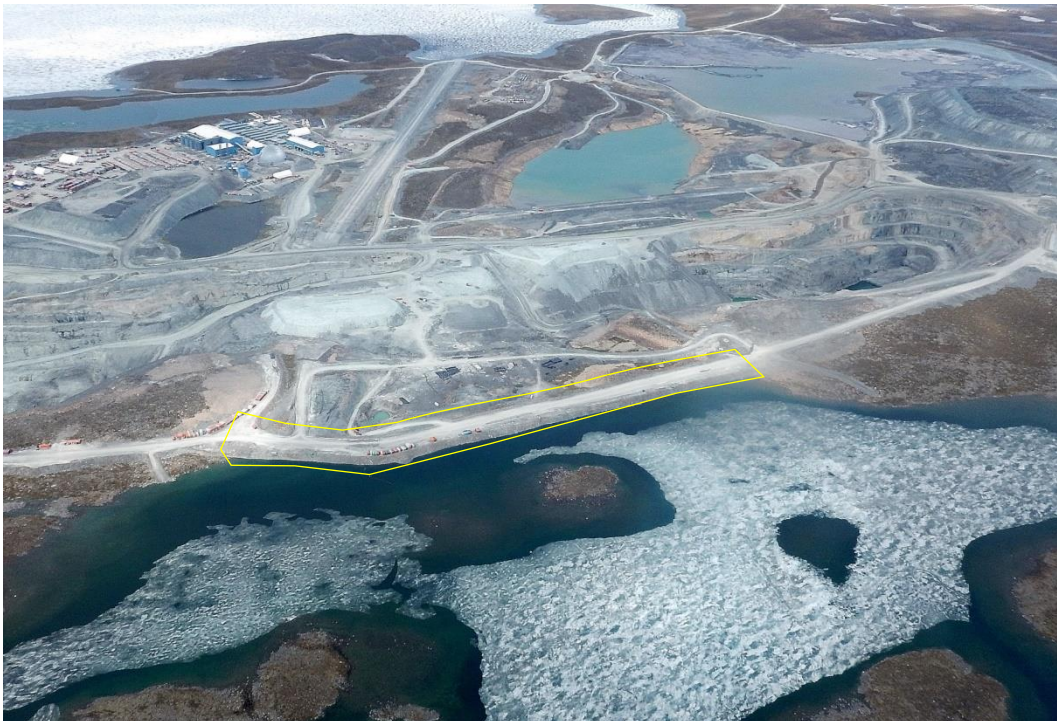
Figure 3-1 : Aerial View of East Dike
