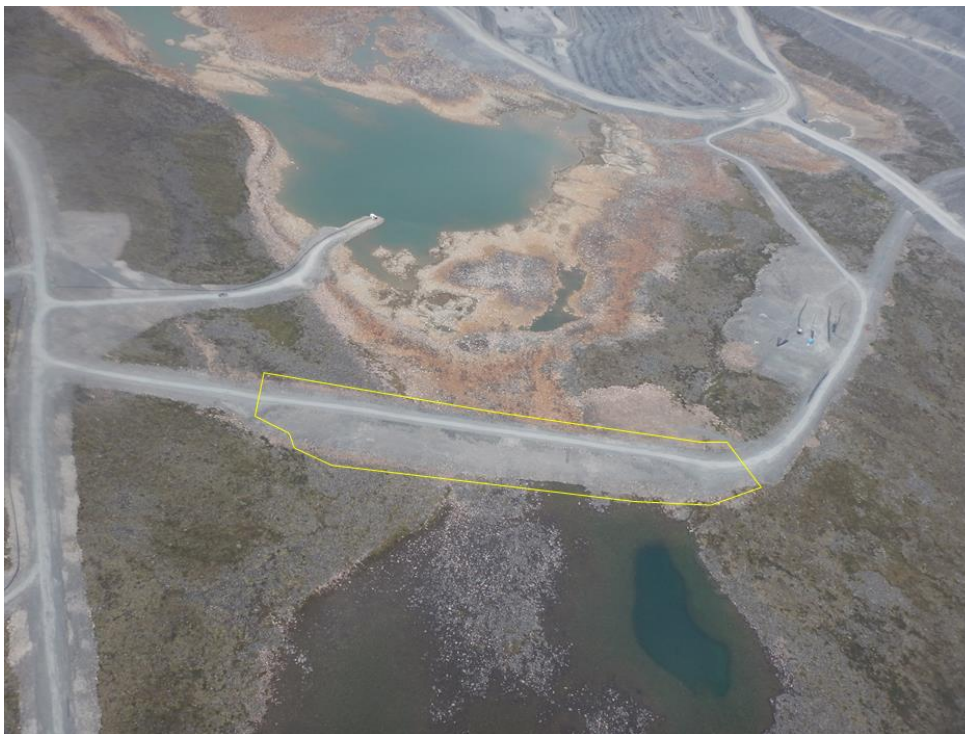
Figure 3-7 : Aerial View of Vault Dike
