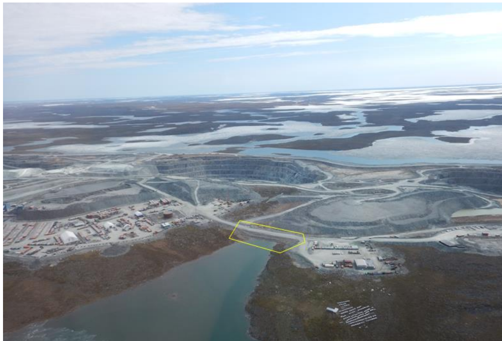
Figure 3-5 : Aerial View of South Camp Dike
