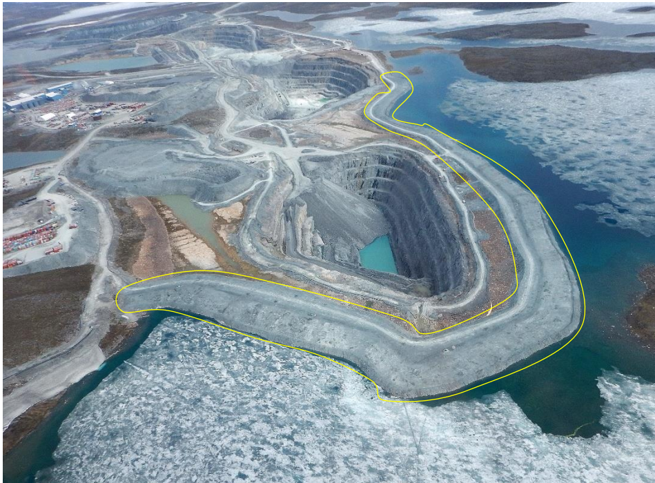
Figure 3-3 : Aerial View of Bay-Goose Dike
