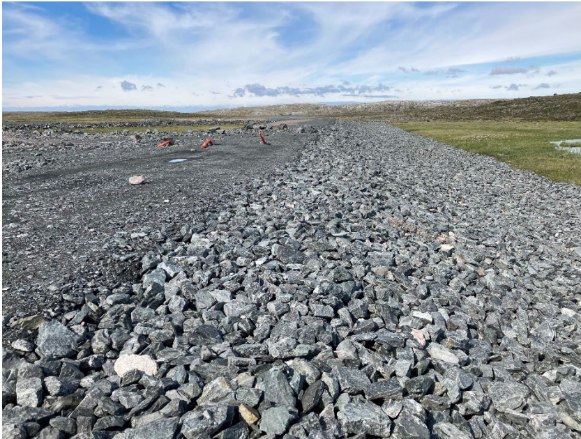
Photograph H12-1 IVR Diversion Channel
