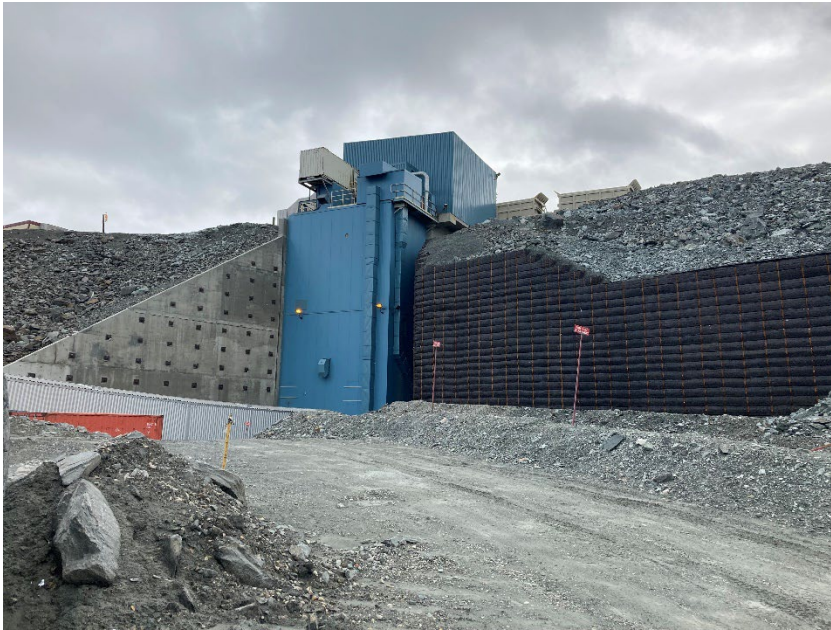
Photograph H6-1 Crusher Retaining Wall
