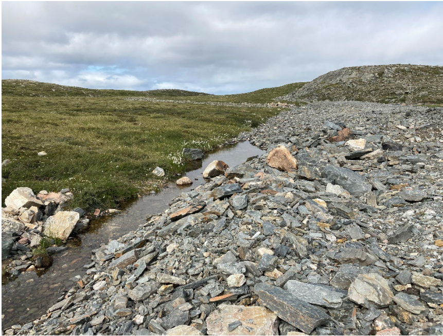
Photograph H2-13 Diversion Ditch and its Sediment and Erosion Protection Structure
