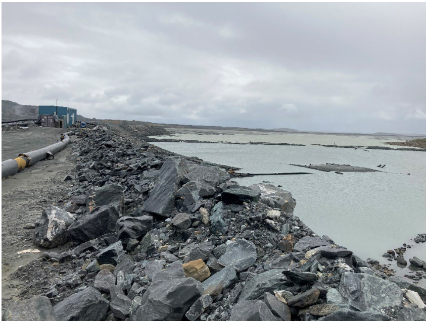
Photograph B4-8 Stormwater Dike
