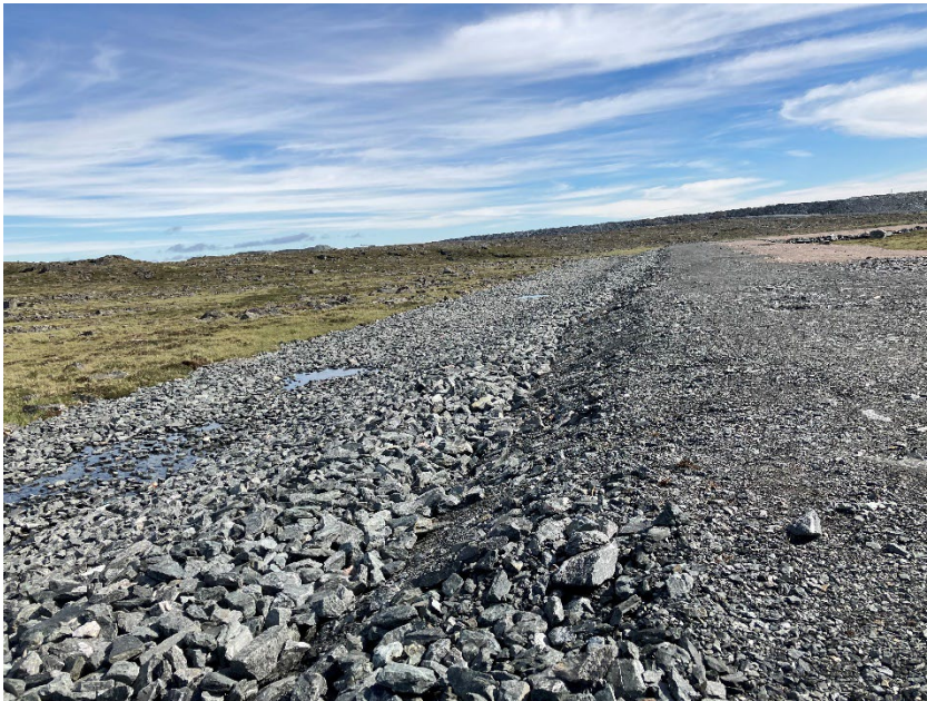
Photograph H12-6 IVR Diversion Channel
