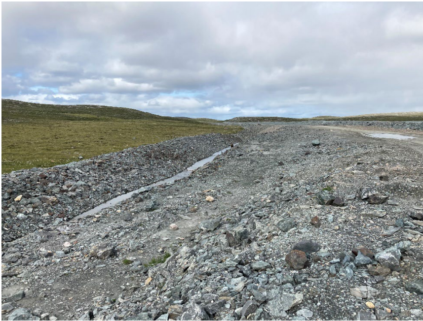
Photograph H2-15 Diversion Ditch and its Sediment and Erosion Protection Structure
