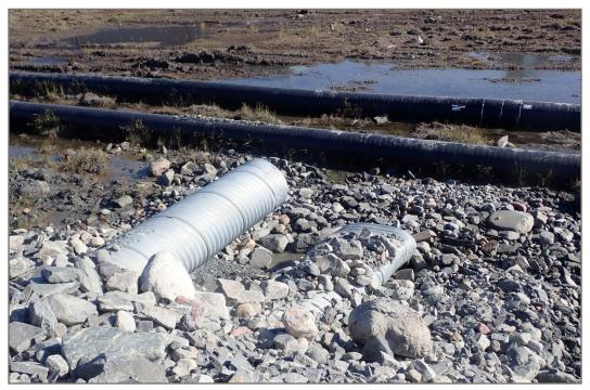
Photo 10: Site Roads—Culvert #18 Outlet. Lower pipe crushed.
