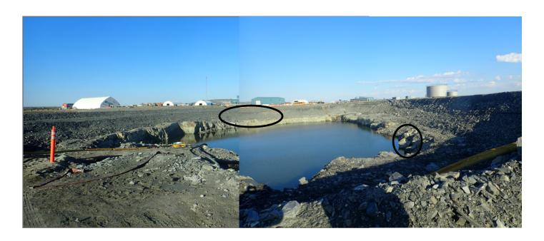
**Photo 1:** SP1 Saline Pond - looking towards the west. Pond in bedrock, ROM covered overburden slopes
