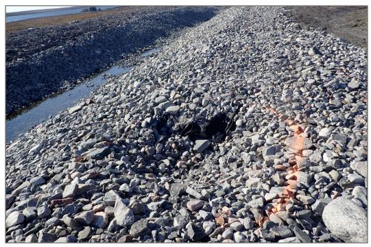
**Photo 24:** Channel 4 - Minor subsidence between original ground and channel rip rap.
