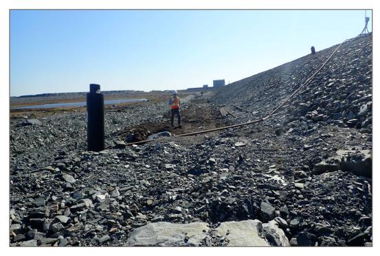
**Photo 14:** Dike D-CP1 - North end of disturbed ground between dyke toe and seepage collection channel.
