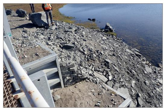
Photo 19: M-5 Bridge—Gabion North Abutment
