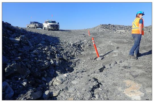
Photo 6: WRSF3—Settlement in access ramp from WRSF3 to CP6.
