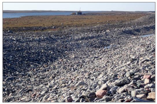
**Photo 25:** Channel 4 - Subsidence in upstream slope (east slope) of channel.
