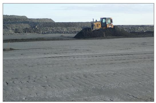
**Photo 5:** TSF - Spreading tailings.
