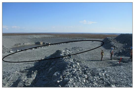
Photo 7: WRSF3—Thermal cover placed in 2021 between WRSF3 and CP6 due to significant settlement and erosion in area.
