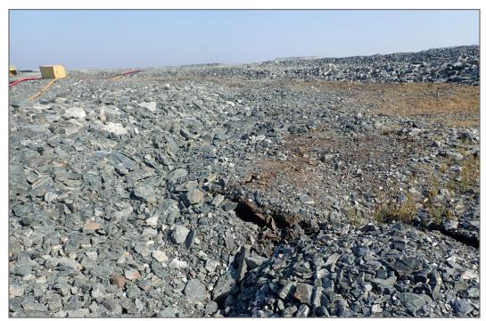
Photo 19: SP4 Saline Pond —Settlement in behind rockfill cover.
