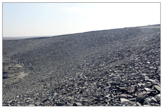
Photo 14: SP4—Rockfill covered overburden slope.
