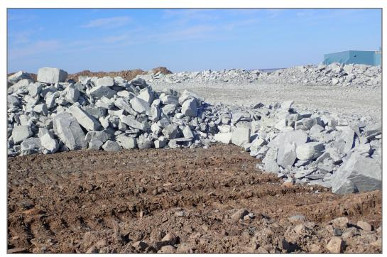
**Photo 13:** WRSF1—Waste rock plating in overburden for access.
