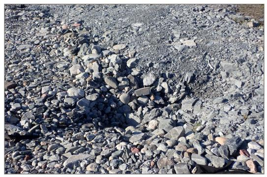
Photo 26: Channel 4 - Subsidence between overburden and rip rap.
