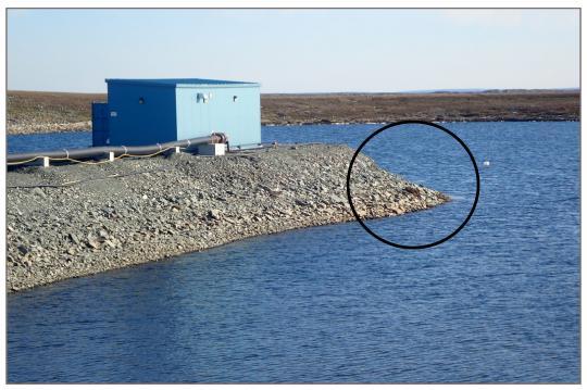
Photo 17: Dike D-CP1 Jetty 1 - Erosion at south east corner of Jetty 1
