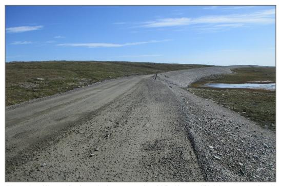
Photo 14: Water collection point between road and hill side near KM 2.35, overtopped road during 2021 freshet.
