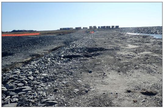
Photo 11: Berm CP4 - Settlement on surface of berm.
