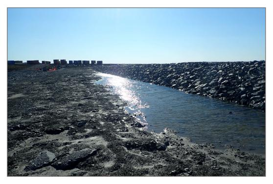
**Photo 12:** Berm CP4 - Pooling water on thermal berm.
