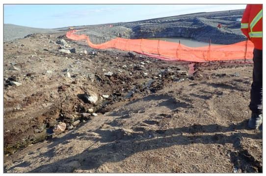
Photo 10: TSF - Drainage from Cell 1 directed to CP3
