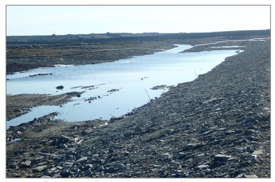
**Photo 34:** Channel 5—Water level in channel controlled by CP5, pooling in low area against Berm3, looking east. Berm 5 on the right of the photo.
