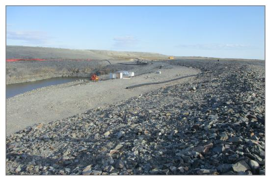
**Photo 9:** Berm CP3 - Berm crest, looking south. Undulations in crest 0.3 to 0.5 m.
