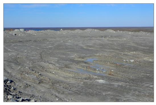
Photo 12: WRSF1—Condition of winter placement overburden on top bench.
