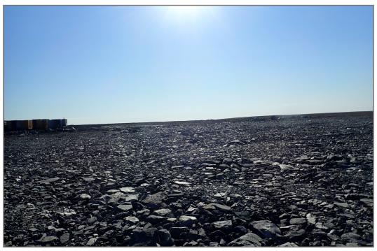
**Photo 13:** Berm CP4 - Undulating settlement up to 0.3 m throughout surface of berm.
