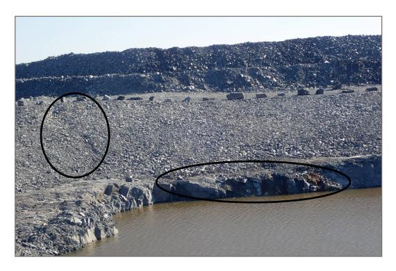
Photo 4: Pond CP6—South side of pond, WRSF3 above pond, water inflow on bedrock surface in southeast corner of pond, deformed ROM, may be indication of subsurface flow.
