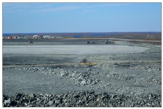
**Photo 4:** TSF - Placing tailings. White precipitate on some previously placed tailings.
