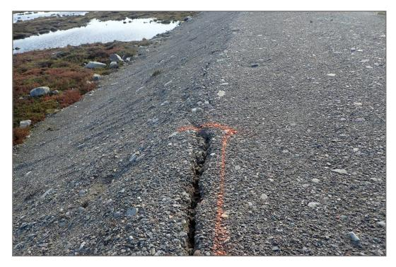
Photo 42: Berm 2—Cracking on upstream slope.
