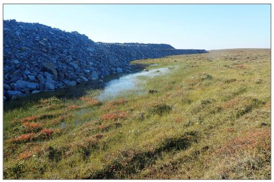
**Photo 3:** WRSF3—Ponding at the toe on east side of WRSF.
