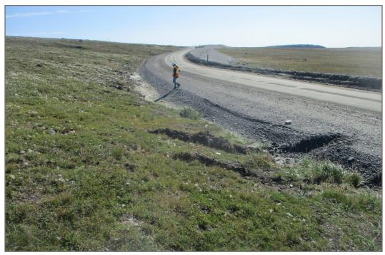
Photo 13: Water collection point between road and hill side near KM 2.35, overtopped road during 2021 freshet.
