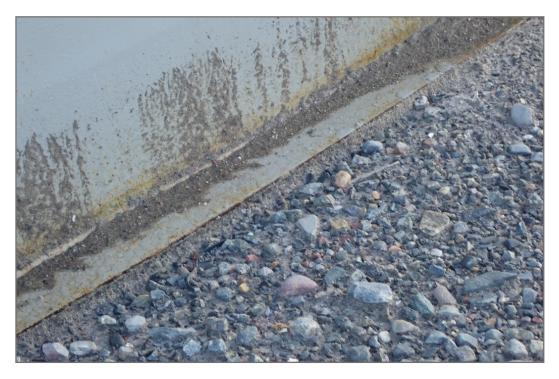
**Photo 24:** Industrial Fuel Storage Tanks. Small amount of erosion on tank pedestals. Fill generally still under tanks.
