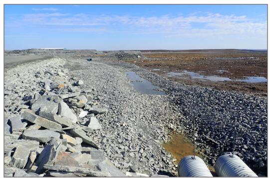
**Photo 37:** Channel 7—Upper reach, minor subsidence and pooling at bottom of channel, looking north.
