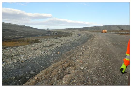
Photo 20: Channel 3—Cracking along road side berm.
