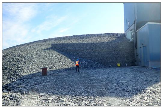
Photo 4: Crusher Pad—MSE Wall on the east corner.
