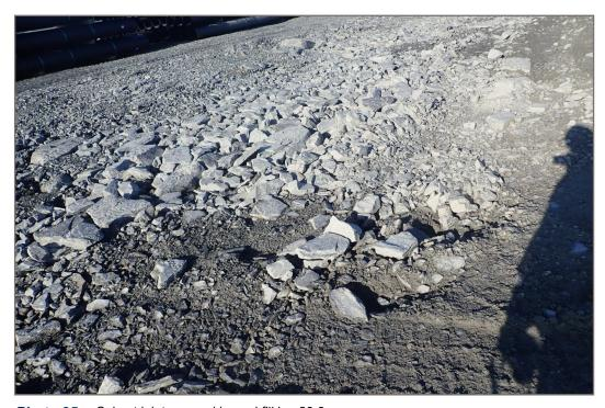
Photo 35: Culvert inlet covered by rockfill km 29.6
