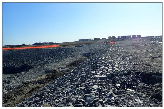
Photo 10: Berm CP4 - Upstream slope, thermal cover and original ground above Pond CP4
