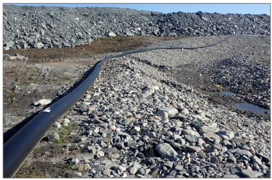
**Photo 27:** Channel 4 - Low point along upstream of channel crest with preferential flow paths into channel.
