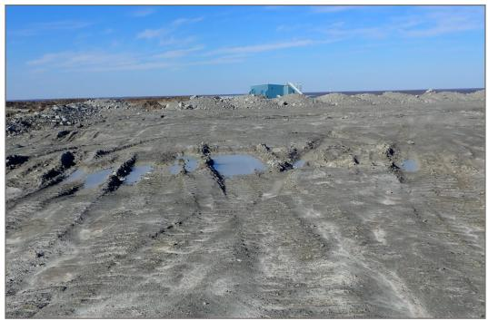
**Photo 11:** WRSF1—Condition of winter placement overburden on top bench.
