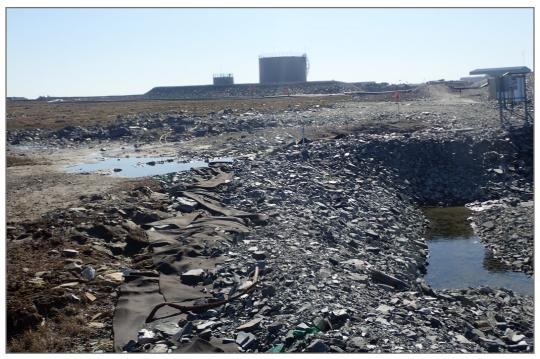
**Photo 11:** Dike D-CP1 - Water collection pond, southeast corner, deformed fill slope.
