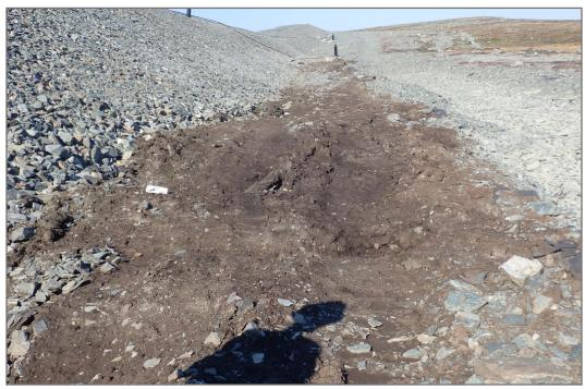
Photo 12: Dike D-CP1 - ground between the Dike toe and water collection channel, settlement and subsidence. Similar to 2020.
