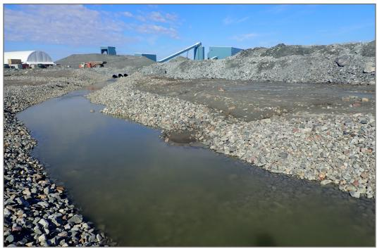
Photo 3: Channel 1—Downstream of crusher ramp, crest subsidence and erosion into channel.
