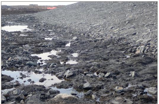
Photo 14: TSF - Sediment at toe of slope.
