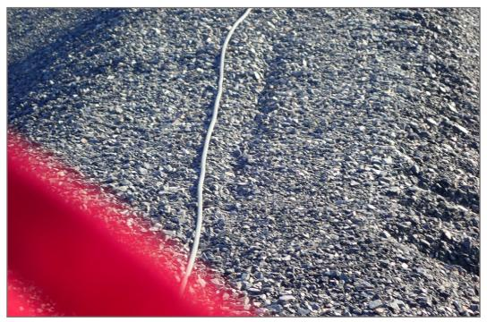
Photo 25: Industrial Fuel Storage Tanks. Exposed grounding cable.
