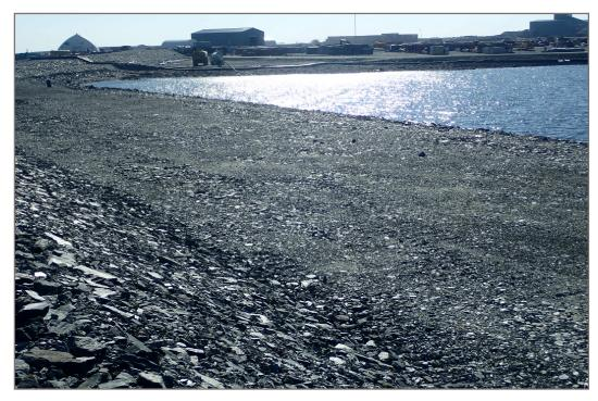
Photo 8: Dike D-CP1 - Upstream crest. Good conditions, west end of dyke.
