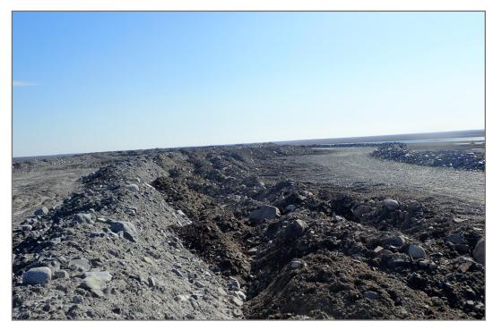
Photo 10: WRSF1—Recent overburden placement outside of WRSF overburden limits.
