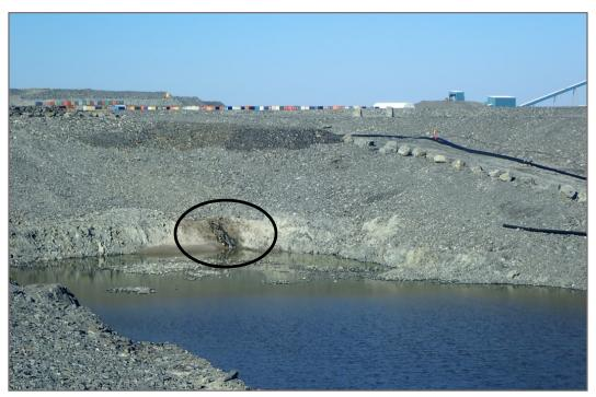
**Photo 3:** Pond CP6 - Exposed bedrock lower portion of pond, water inflow northwest corner.
