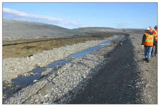
Photo 14: Channel 3—Undulating settlement along base of channel causing ponding.
