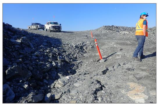
**Photo 13:** Pond CP6 - Settlement—on ramp from WRSF3 to CP6 area.
