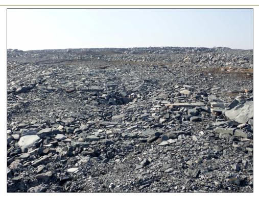
Photo 13: SP4 Saline Pond - Thaw subsidence in crest of rockfill cover.
