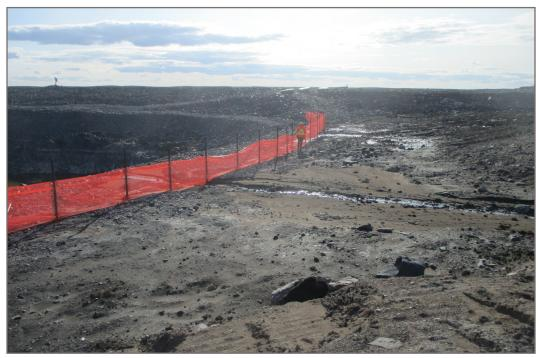
**Photo 5:** Pond CP3 - Runoff/erosion channels into pond from north end of TSF drainage, located on north side of pond.
