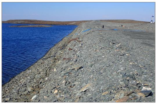
Photo 1: Dike D-CP1 - Upstream face—some wave erosion evident
