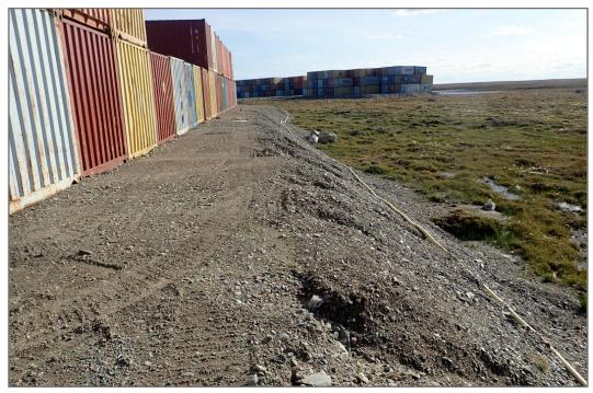
Photo 13: Emulsion Plant—north side of pad, erosion in pad slope.
