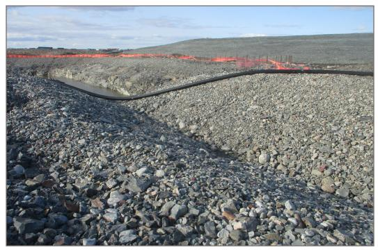
Photo 12: Channel 3—Discharge into CP3.
