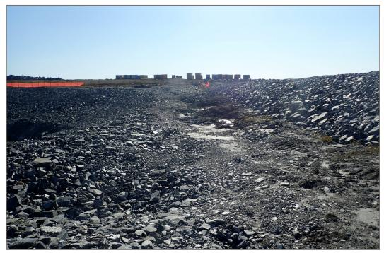
Photo 9: Pond CP4 - Settlement and subsidence between Berm CP4 and west pond slope.
