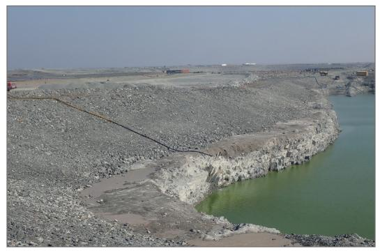
Photo 20: SP4 Saline Pond—Rockfill cover, no significant deformation. Bedrock below slope.
