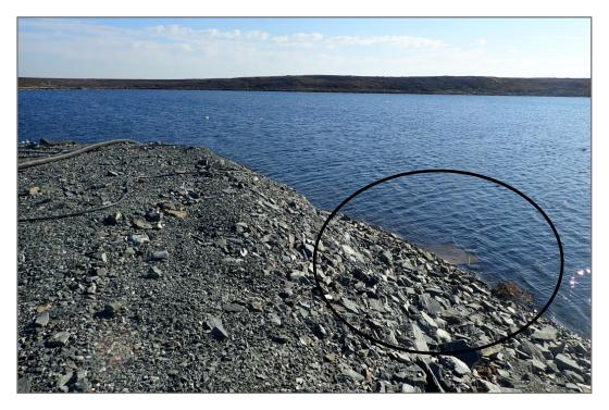
Photo 18: Dike D-CP1 Jetty 1—Erosion at southeast corner—under cutting top portion of fill.
