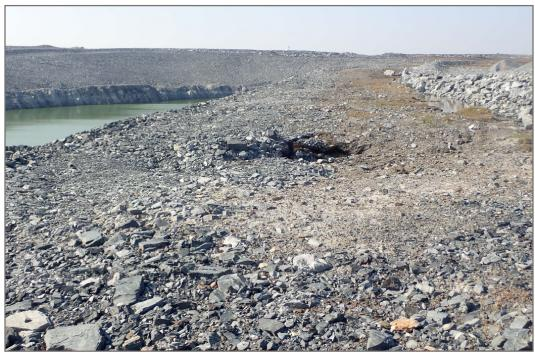
**Photo 15:** SP4 Saline Pond—Subsidence in original ground at crest of slope, behind rockfill cover.
