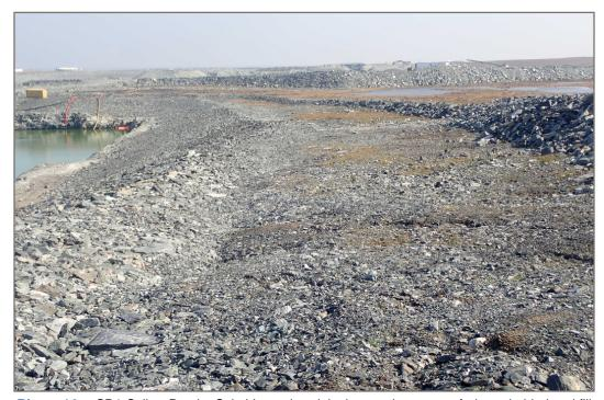
Photo 16: SP4 Saline Pond - Subsidence in original ground at crest of slope, behind rockfill cover.
