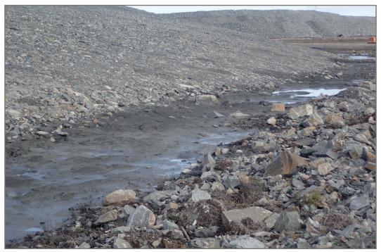
Photo 13: TSF - West slope. Sediment at toe of slope.
