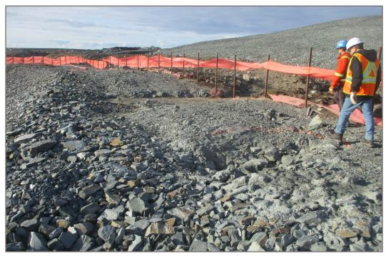
**Photo 10:** Pond CP3 - Looking north, settlement and erosion at overburden crest.
