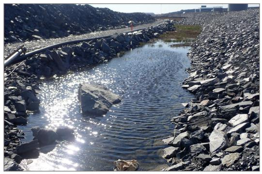
Photo 5: Pond CP6 - Ponded water adjacent to Berm CP6 and access road
