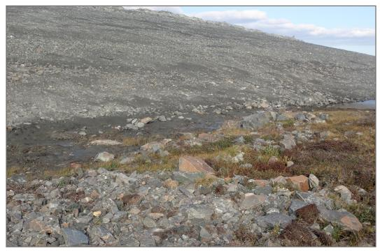
**Photo 12:** TSF - West slope of TSF. Sediment at toe of TSF slope.
