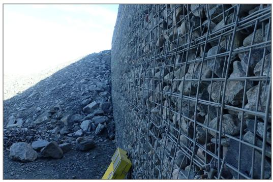
**Photo 5:** Crusher Pad—MSE wall, north east side. Slight bulge to gabion baskets
