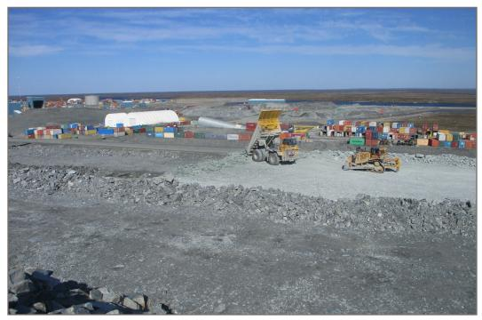
**Photo 6:** WRSF1—Waste rock placement—widening lower bench.
