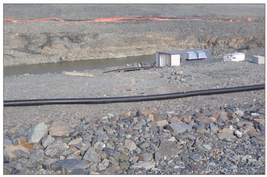
Photo 3: Pond CP3 - Looking east, CP3 berm and rockfill covered overburden in foreground. Settlement along the overburden between CP3 and berm.
