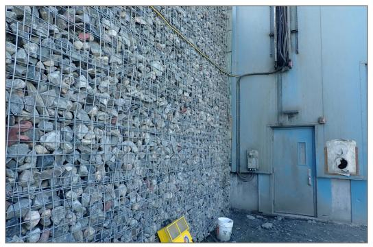
Photo 6: Crusher Pad—MSE wall, north east side. Slight inward slope to wall.
