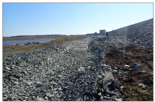
Photo 13: Dike D-CP1 - Seepage collection channel. Subsidence in ground between channel and downstream toe.
