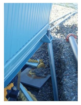
Photo 10: CP5 Jetty 5 - Footing Erosion—Southwest Corner
