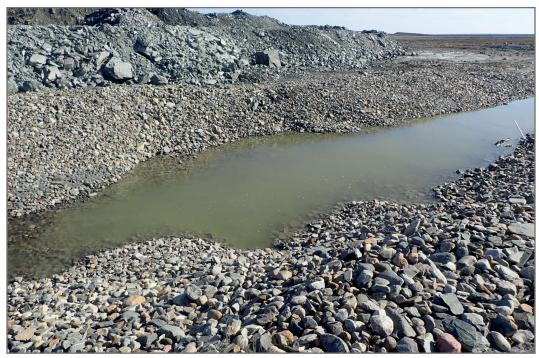
Photo 5: Channel 1—Subsidence of channel base and slopes.
