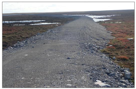
Photo 41: Berm 2— Esker and till berm upslope of TSF
