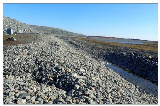
Photo 23: Channel 4 - Settlement in base of channel resulting in minor ponding.
