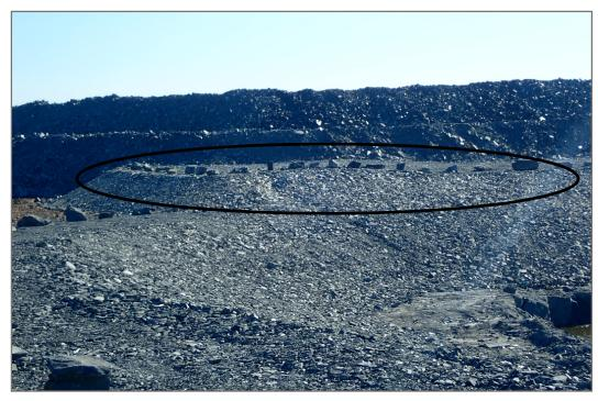
**Photo 8:** Pond CP6 - Ground between WRSF3 and CP6—filled with ROM June 2021. ROM placed to reduce erosion in former lakebed sediments.
