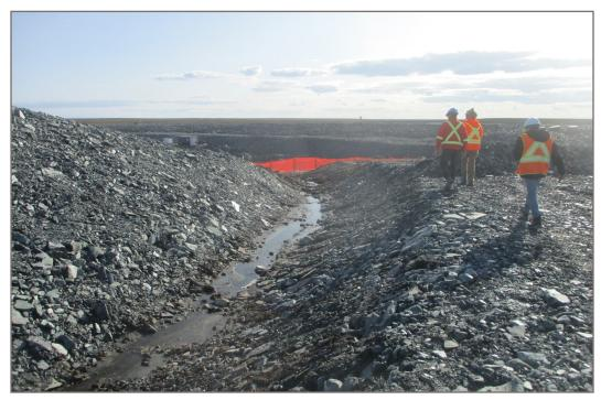
**Photo 6:** Pond CP3 - Improved runoff channel into pond from north end off TSF drainage , located on east side of pond.
