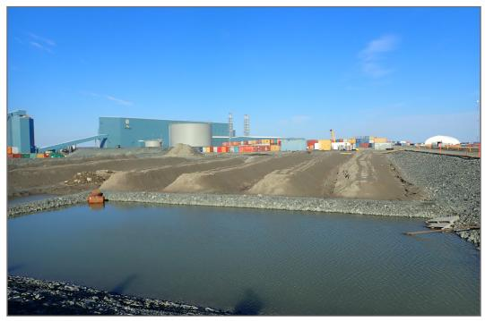
**Photo 15:** Landfarm– Windrows of contaminated soil. Water collection pond.
