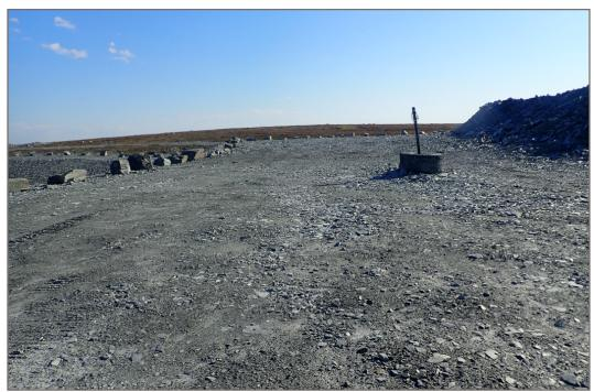
Photo 7: Pond CP6 - Ground between WRSF3 and CP6—filled with ROM June 2021. ROM placed to reduce erosion in former lakebed sediments.
