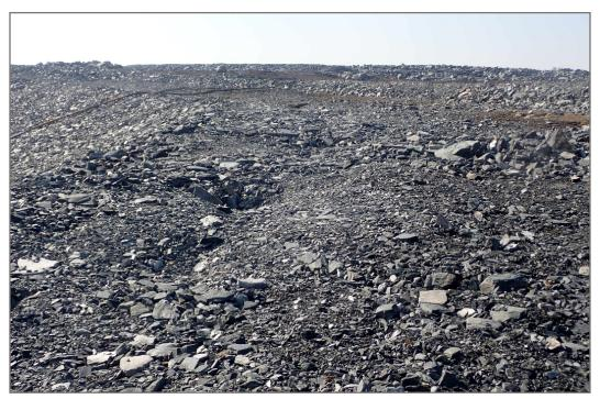
Photo 17: SP4 Saline Pond —Settlement in rockfill crest covering overburden slope.
