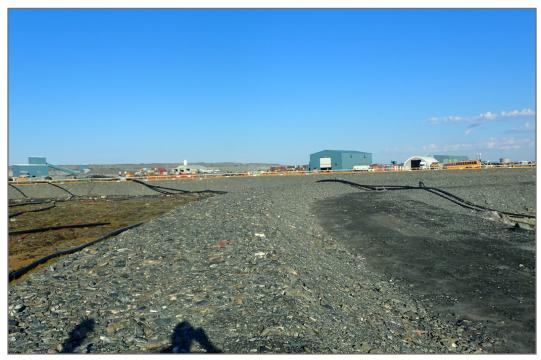
Photo 2: SP1 Saline Pond - Thermal Berm around the pond.
