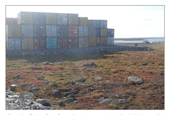
Photo 14: Emulsion Plant—Storage Area—slope on north edge of pad, slight lean to shipping containers.
