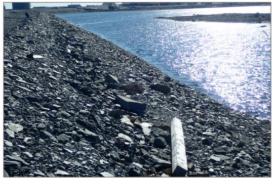
Photo 3: Dike D-CP1 - Upstream face—some wave erosion evident, scarp approximately 1 m high. Erosion also evident on lower portion of slope. Slope is self armouring with larger particles in ROM fill.
