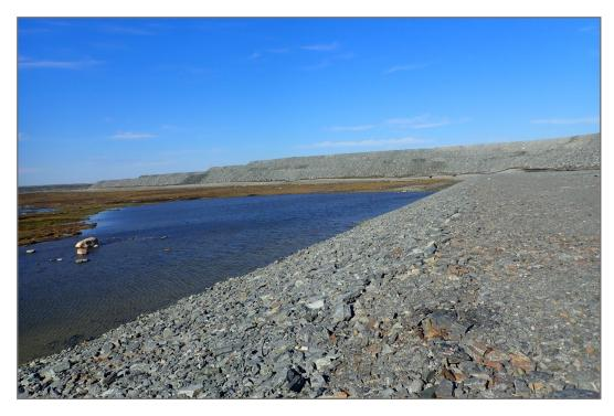
Photo 14: Berm CP4 - Downstream embankment of CP4 berm against lake B8.
