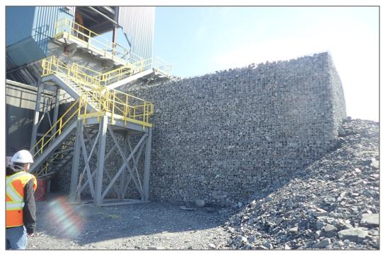
**Photo 3:** Crusher Pad—MSE Wall on the northwest corner.
