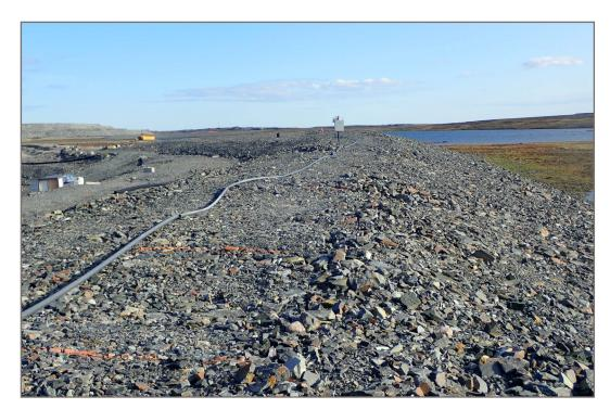
Photo 8: Berm CP3 - Looking south, surface of berm.. Settlement and subsidence.
