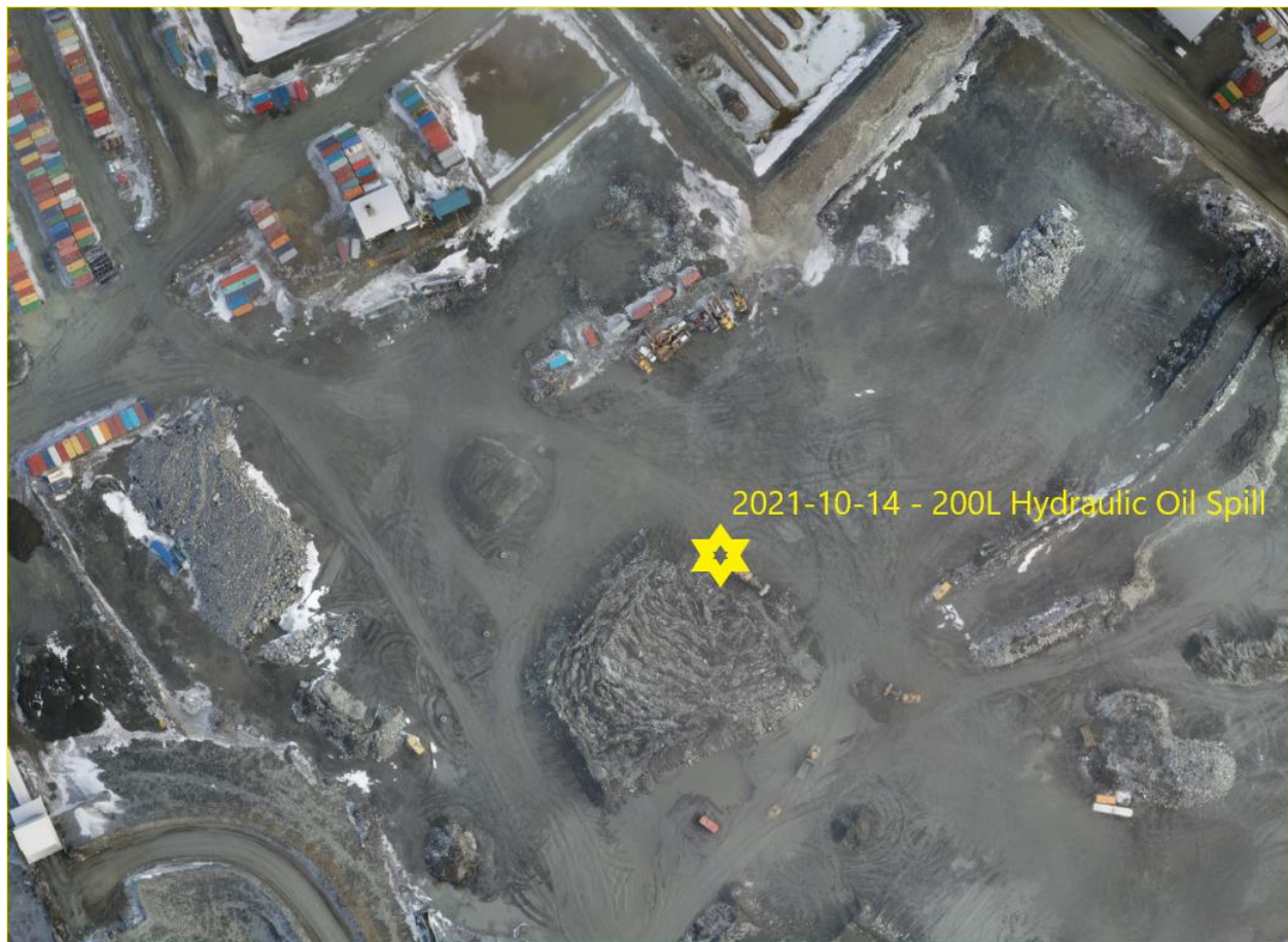
Figure 1: Location of the spill on ore pad
