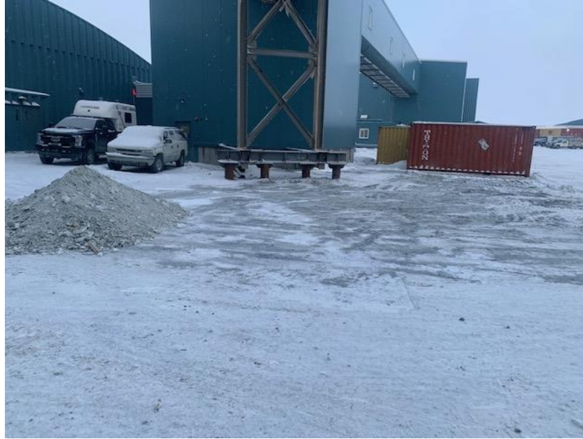
Figure 2: Final clean up.
