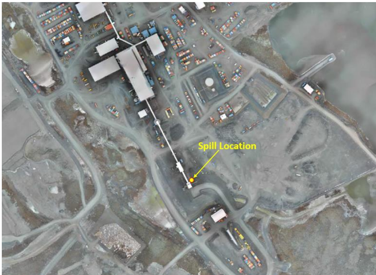
Figure 1: Location of the spill on East side of the apron feeder building.
