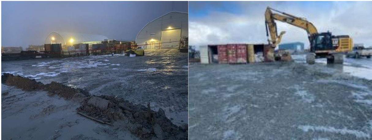
Figure 3: Containment berm and excavator clean up.
