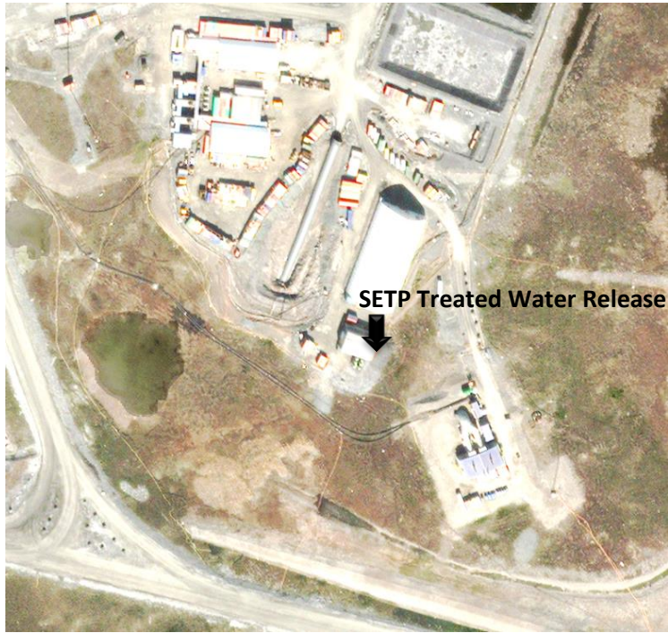
Figure 2: Location of SETP treated water spill within Meliadine's water management area.
