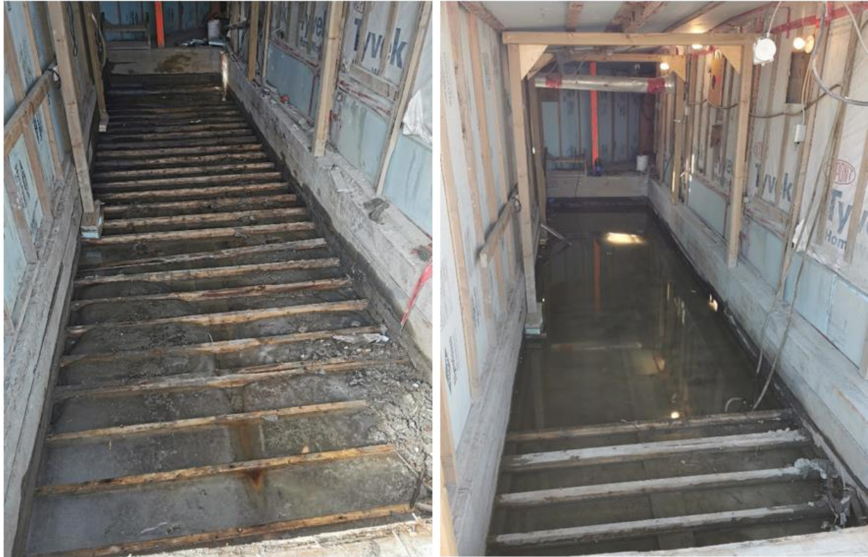
Figure 6: Removal of floorboards, joists, and final recovery of contaminated liquid.
