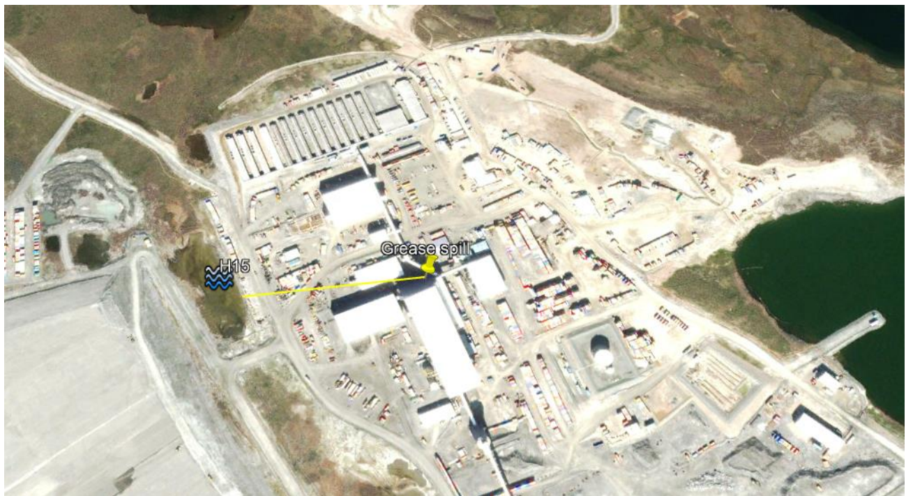
Figure 1: Location of spill.
