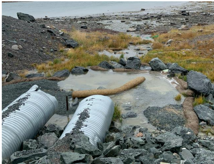
Figure 2: Sediment control at discharge
