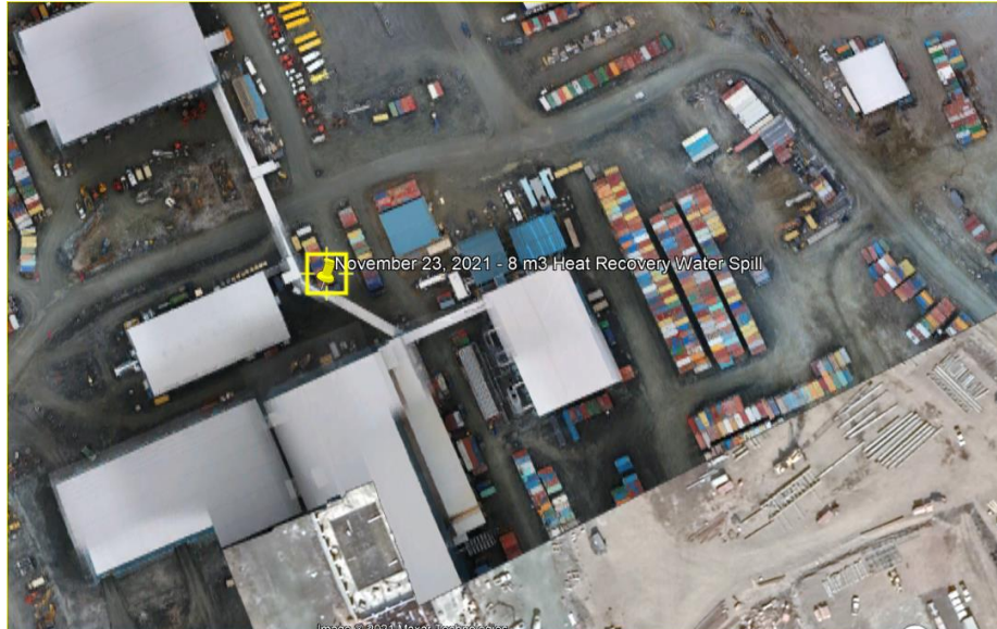
Figure 1: Location of the spill source was inside the elevated pedestrian corridor, which then leaked to the ground below on the Industrial Pad.
