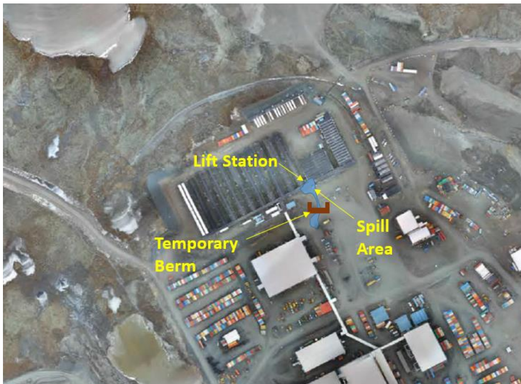
Figure 1: Location of the lift station and affected area in relation to the main camp.
