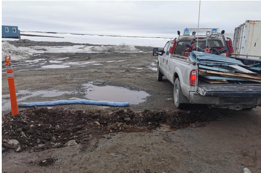
Figure 4: Trench dug to restrict potential flow further down slope.
