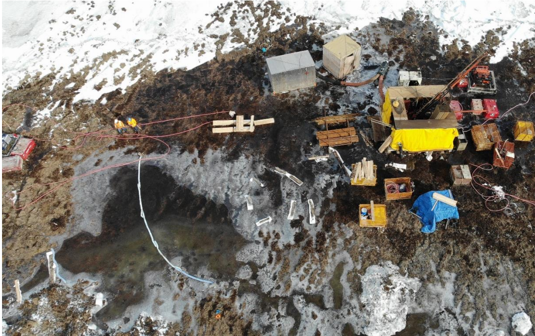
Figure 4: Absorbent pads and booms were deployed to capture the hydrocarbons at the surface of water.
