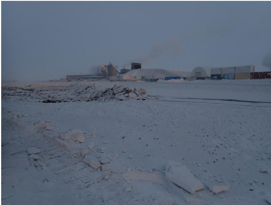
Figure 2: Snow pushed into heat recovery waterline.
