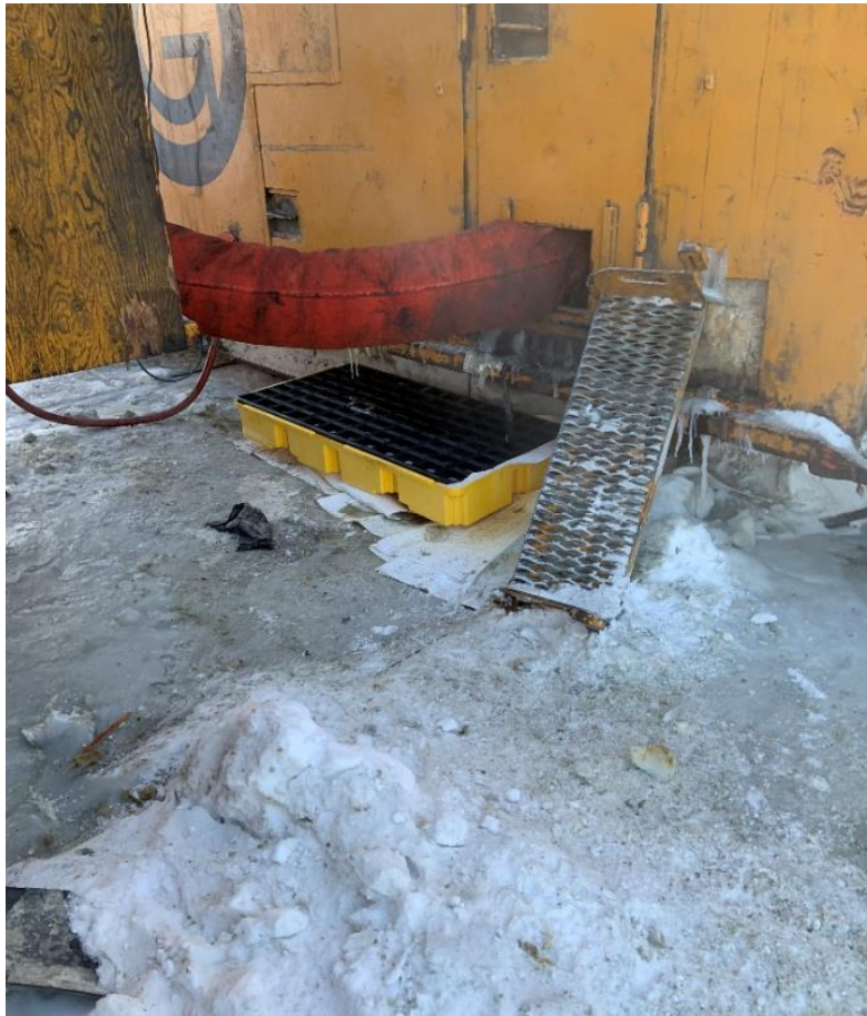
Figure 4: Drill #1 on March 30 after clean up and installation of drip pans and absorbents.
