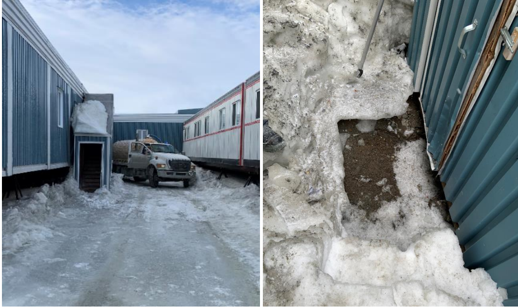
Figure 5: The sucker truck was utilized to empty the lift station holding tank and to collect pooling water outside of the lift station.
