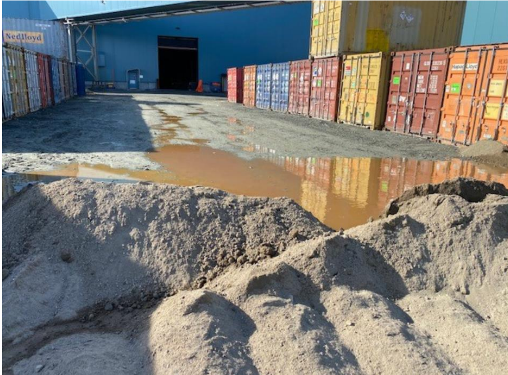
Figure 3: Sand berms constructed at the north end of the spill location.
