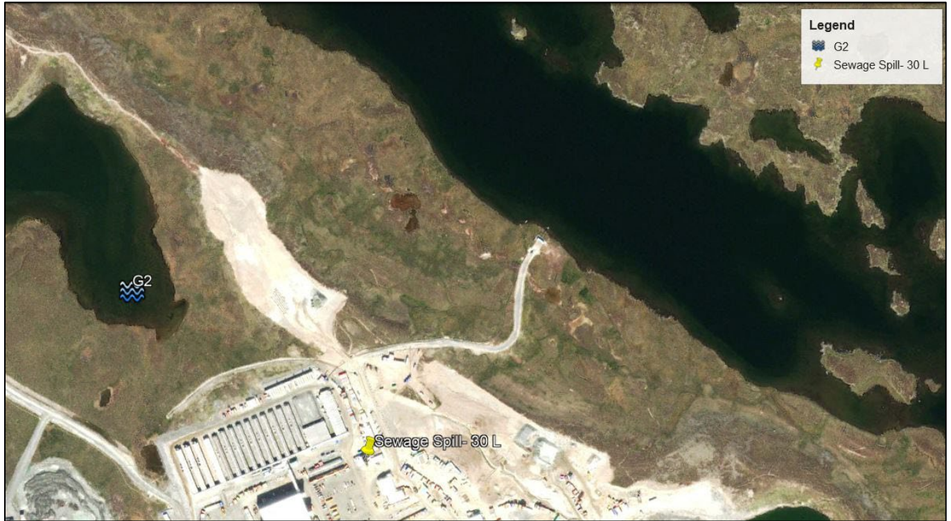
Figure 1: Location of the sewage spill and proximity to water bodies.
