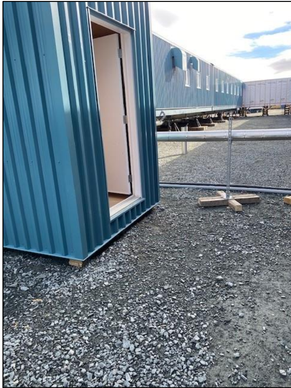
Photo 1: Wing 16 lift station (spill location)
