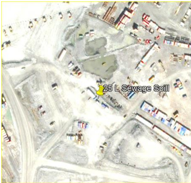
Figure 1: Location of the spill
