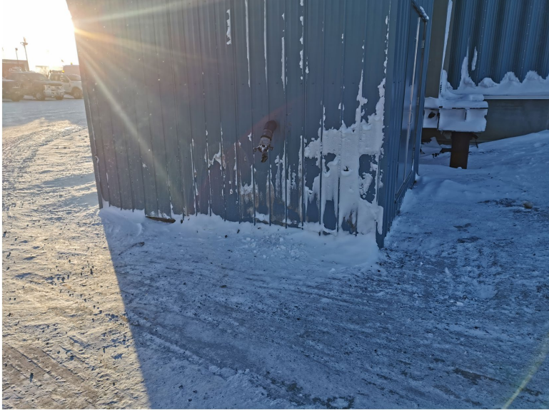
Figure 2: MSB lift station spill clean up
