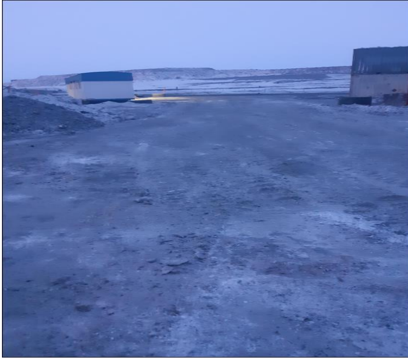
Figure 2: Thickener process water spill cleanup
