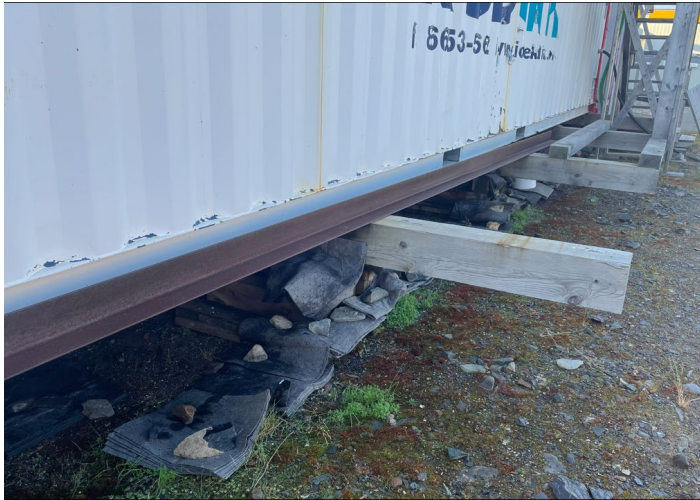
Photo 1: Bionest partially treated Effluent spill
