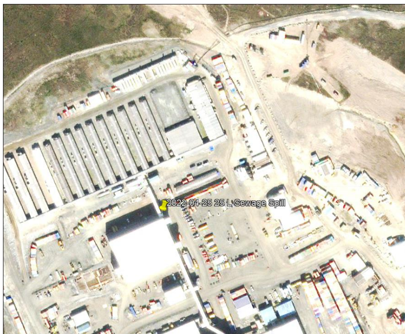
Figure 1: Location of the MSB lift station spill
