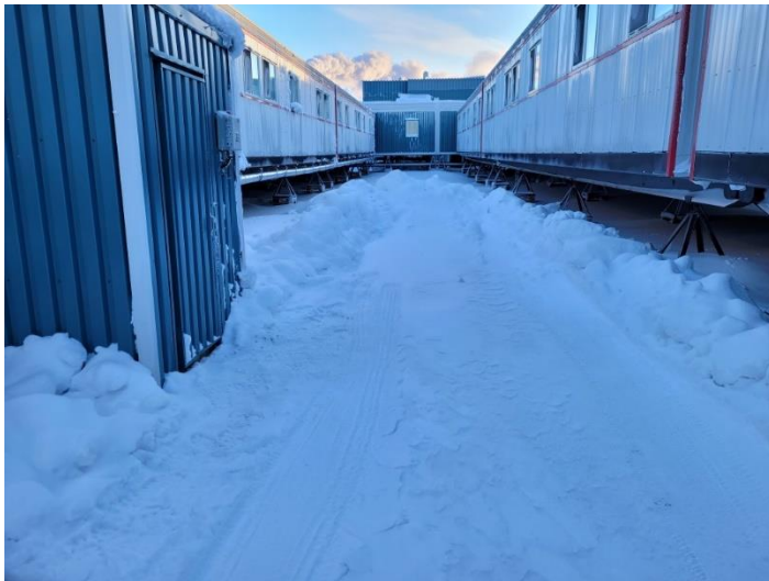
Photo 4: Ground area outside the wing three lift station.
