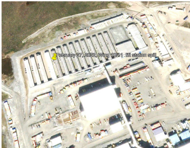
Figure 1: Location of the spill between wings 10 and 11.
