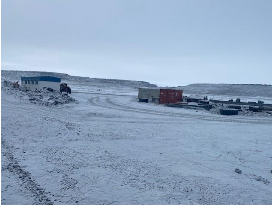
Figure 2: Thickener process water spill clean up area
