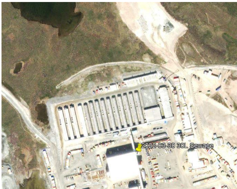
Figure 1: Location of the MSB lift station spill
