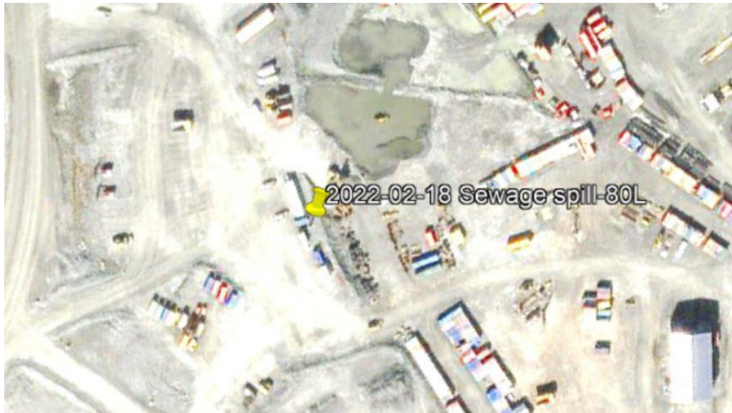
Figure 1: Location of the spill at KCG lift station
