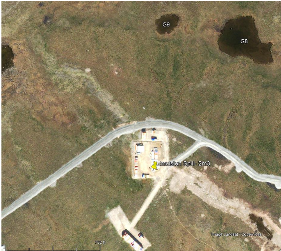
Figure 1: Location of emulsion spill and proximity to water bodies.
