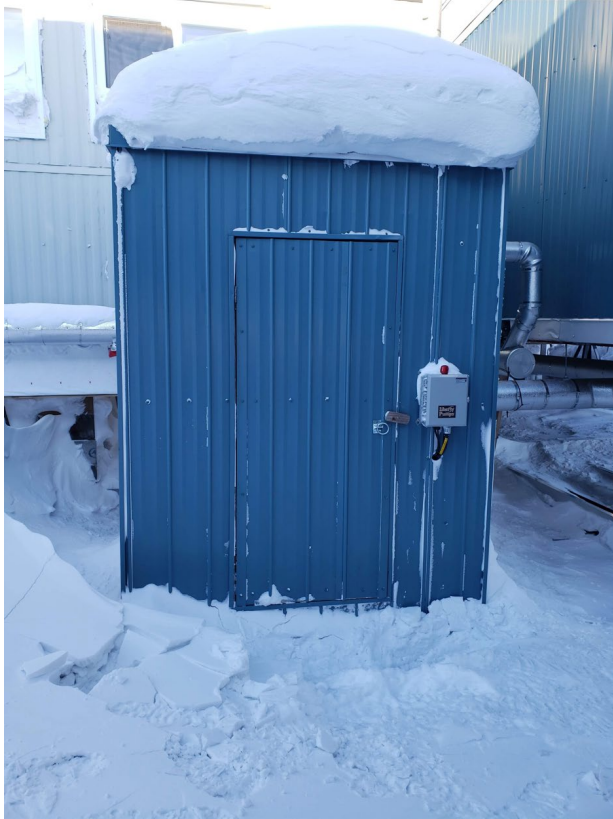
Figure 2: Lift station spill general area was cleaned with sucker truck and shovel
