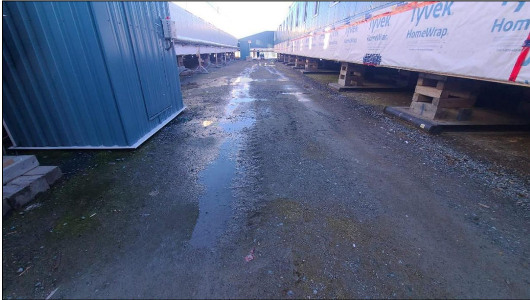
Photo 1: Wing 10 lift station untreated sewage spill.
