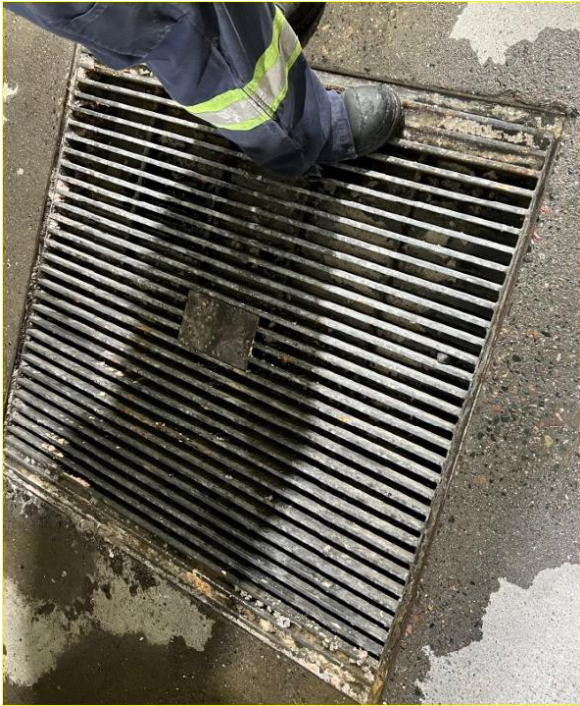
Figure 3: Dyno Equipment Shop collection sump
