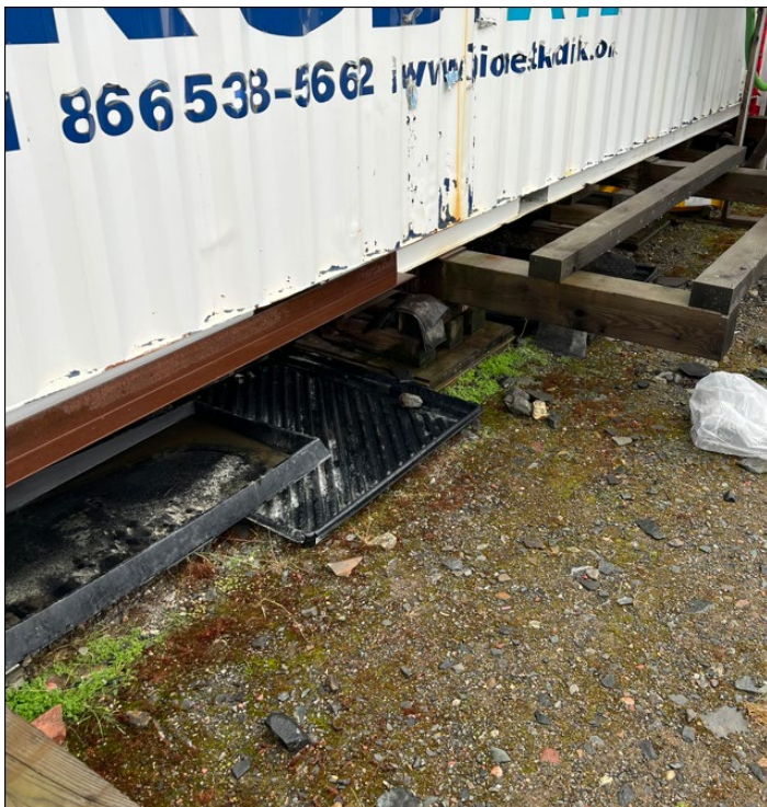
Photo 2: Bionest partially treated Effluent spill collection
