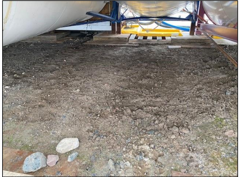
Photo 2: Spill remediation beneath tank RU7000
