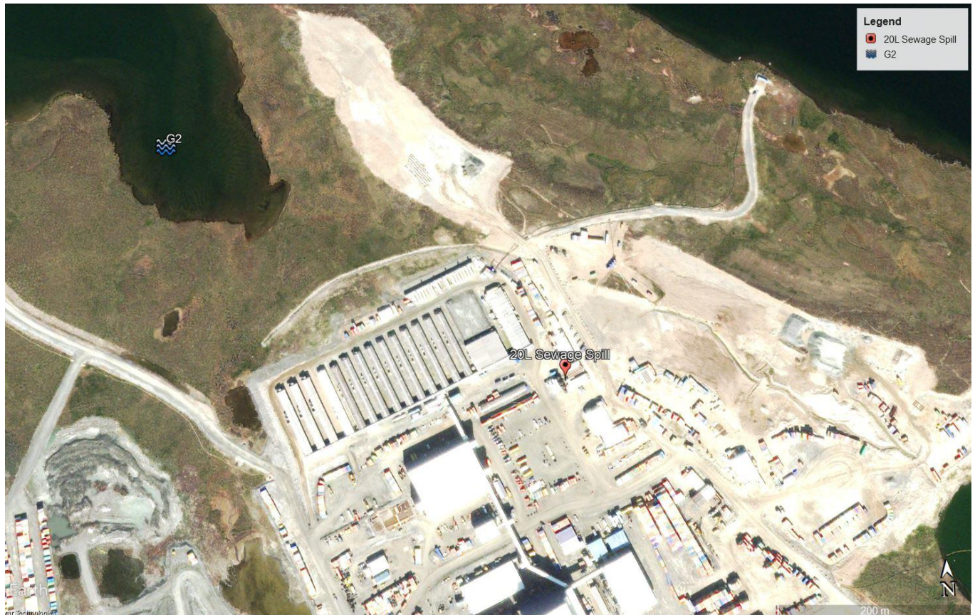
Figure 1: Location of sewage spill and proximity to water bodies.
