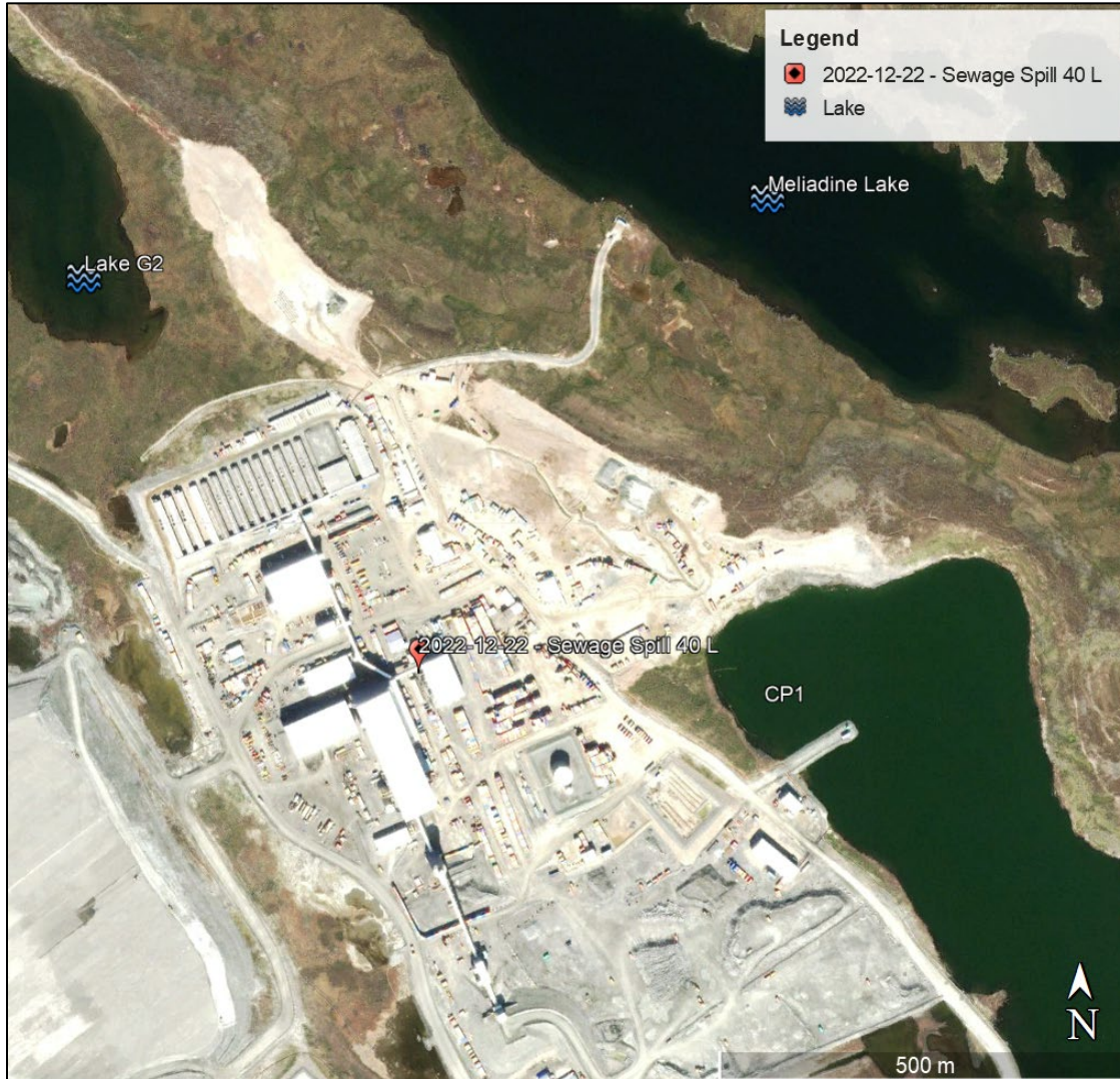
Figure 1: Location of the sewage spill and proximity to water bodies.
