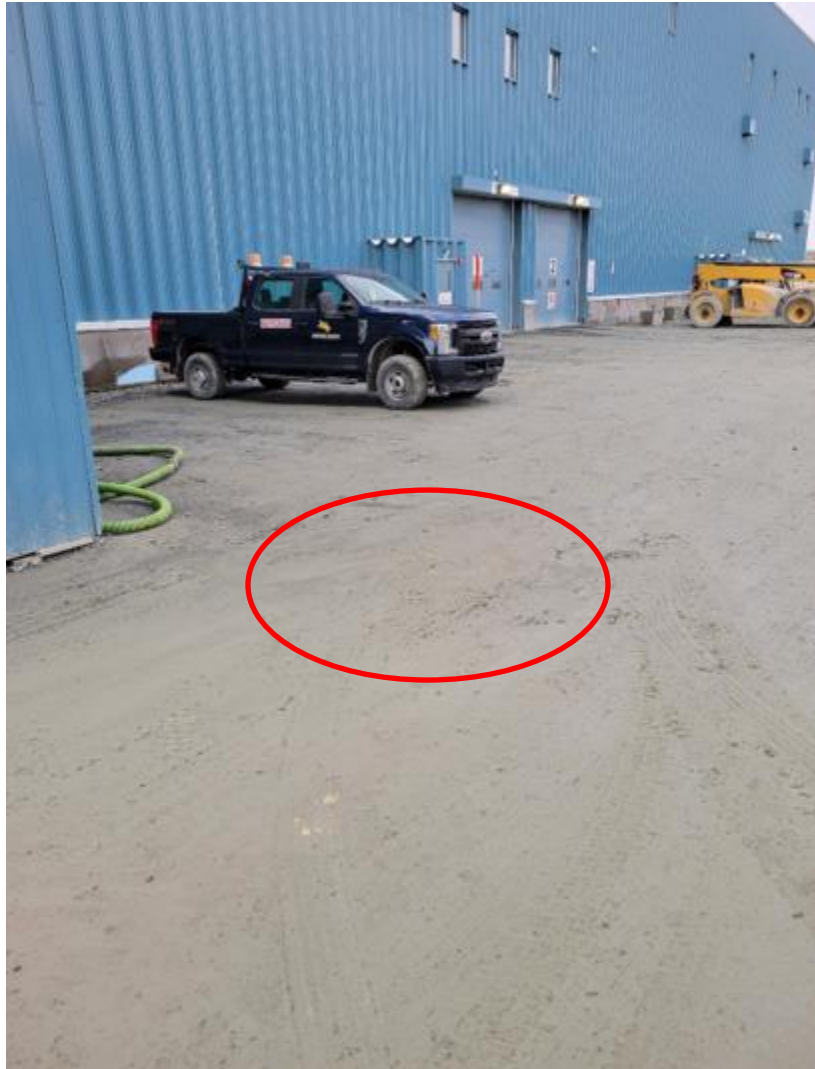
Photo 1: MSB lift station spill location (post-clean up)
