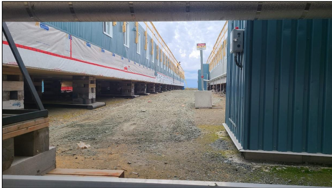
Photo 2: Spill remediation area.
