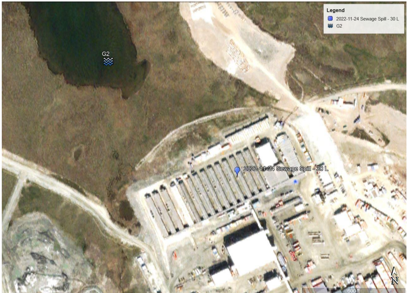
Figure 1: Location of sewage spill and proximity to water bodies.
