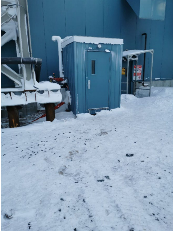
Figure 2: Power plant lift station spill clean up
