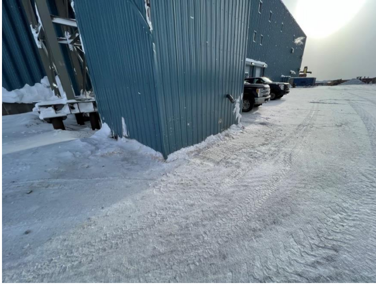
Figure 2: MSB lift station spill clean up
