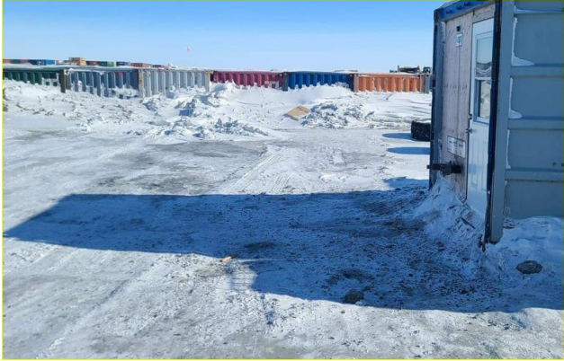
Figure 2: KCG sewage lift station tank spill cleanup
