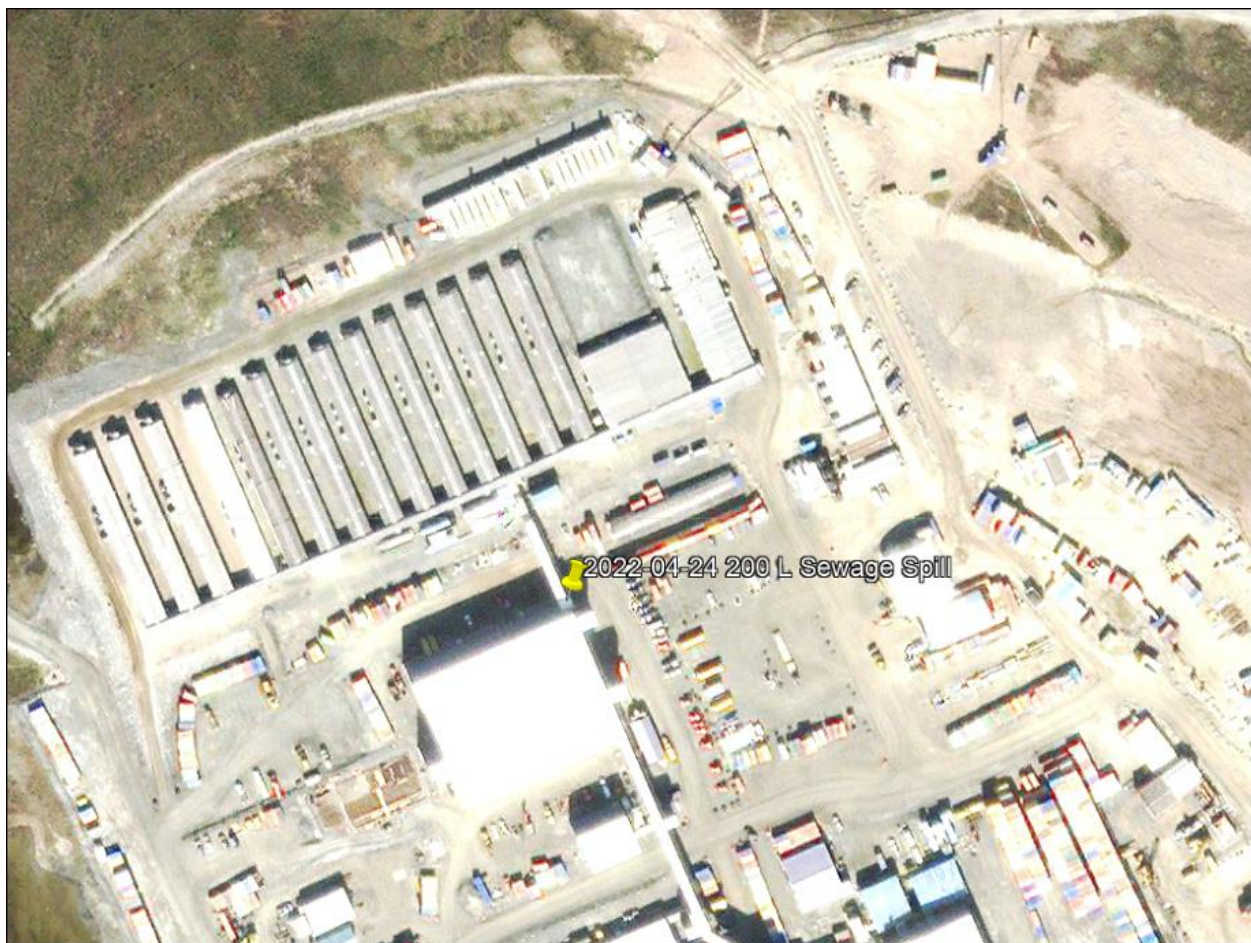
Figure 1: Location of the MSB lift station spill
