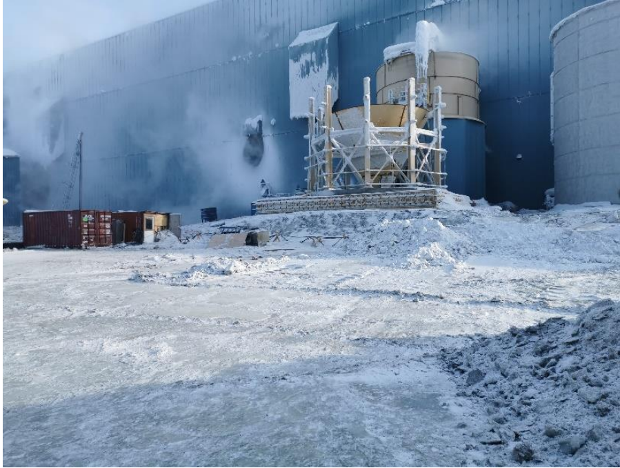
Figure 2: Thickener process water spill clean up
