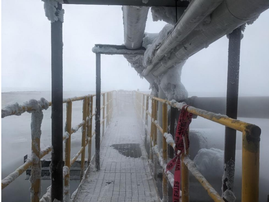
Figure 4: Post-clean up of the overhead ice on the thickener tank
