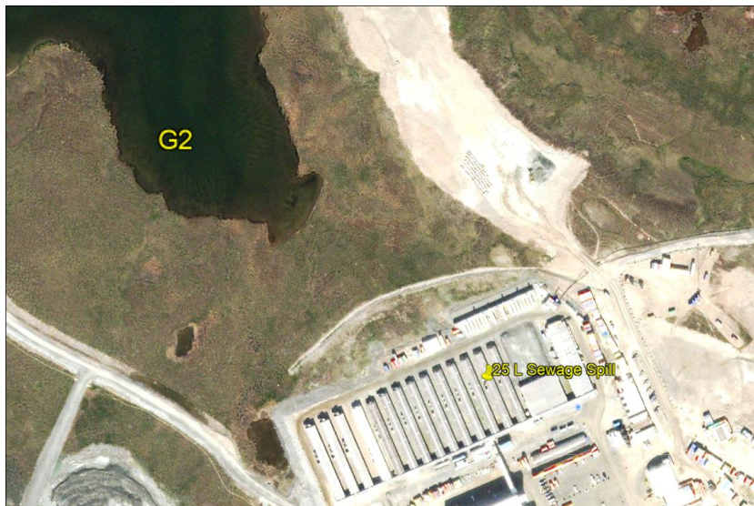
Figure 1: Location of sewage spill.
