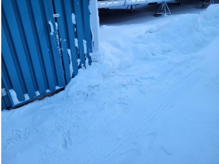
Photo 3: Ground area outside the wing three lift station, post cleanup.
