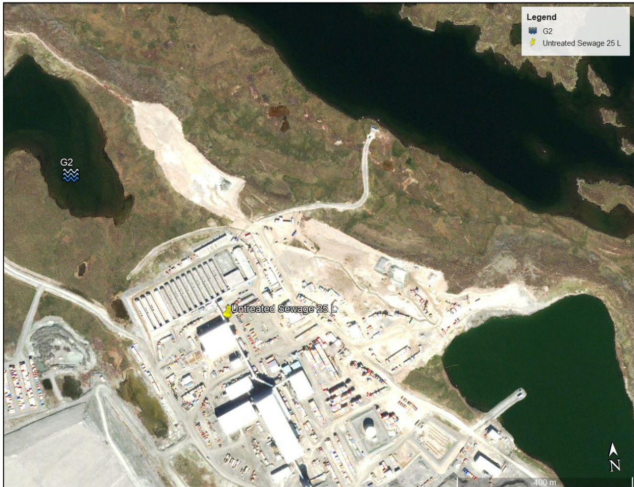
Figure 1: Location of sewage spill and proximity to water bodies.
