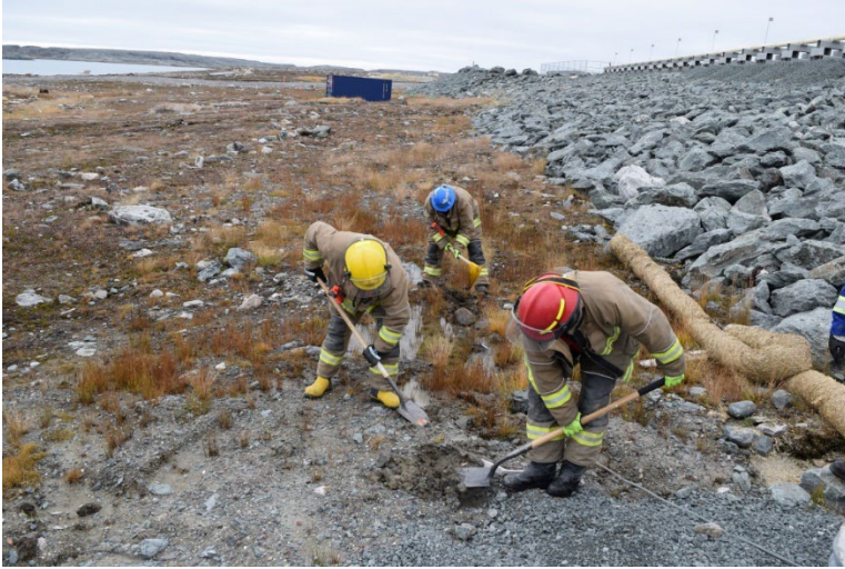
Photo 5: ERT attempting to build trench (surrounding terrain is bedrock)
