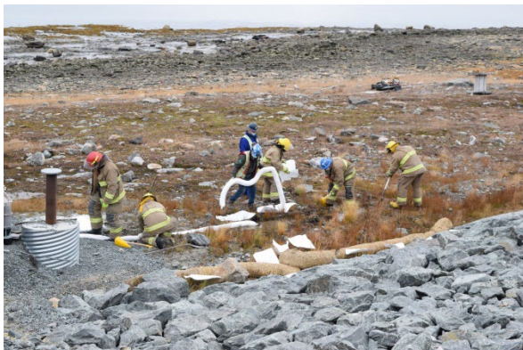
Photo 4: Deploying absorbent booms and sediment control logs
