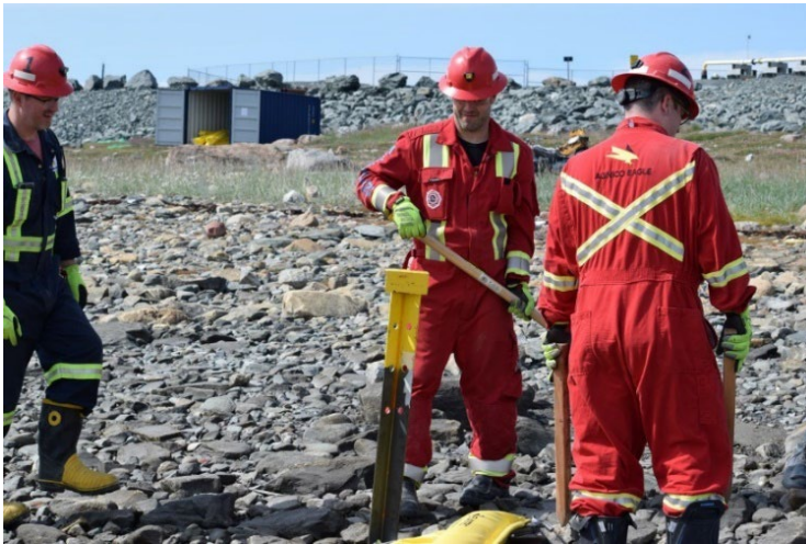
Photo 5: Post-pounding marine boom stakes into the ground with sledgehammer
