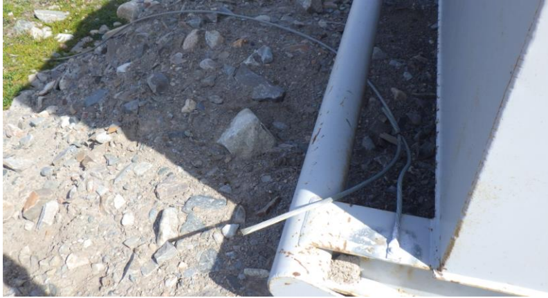
Figure 3-5 Surface Explosive Magazines – Grounding
