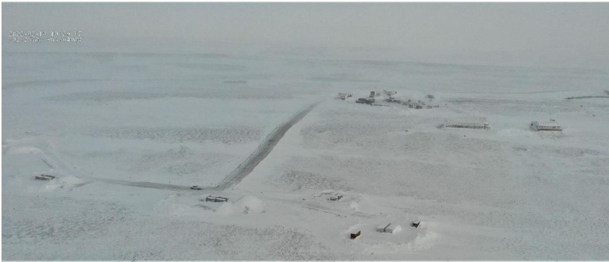
Figure 2-3 Permanent Surface Magazine Location - the Emulsion Plant Storage
