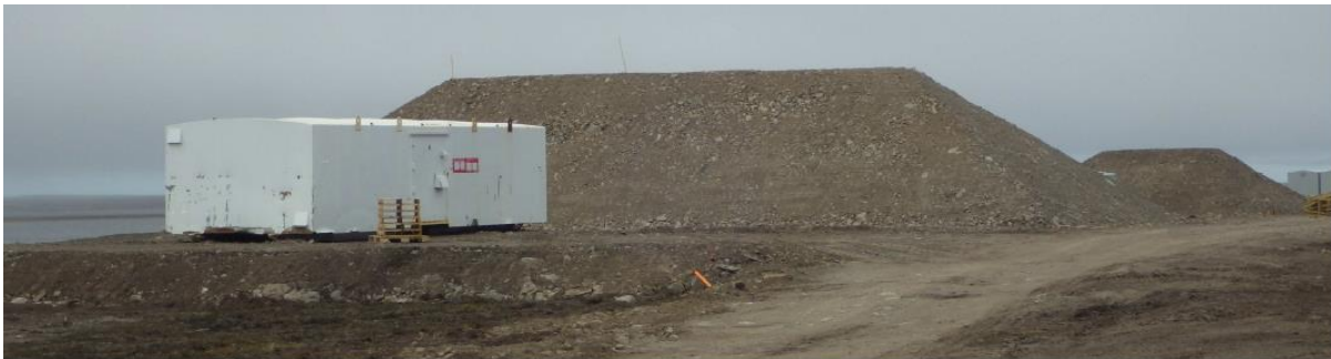
Figure 3-4 Surface Explosive Magazines and Berms
