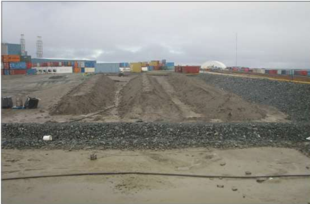
Photo 19: Landfarm— Windrows of contaminated soil.
