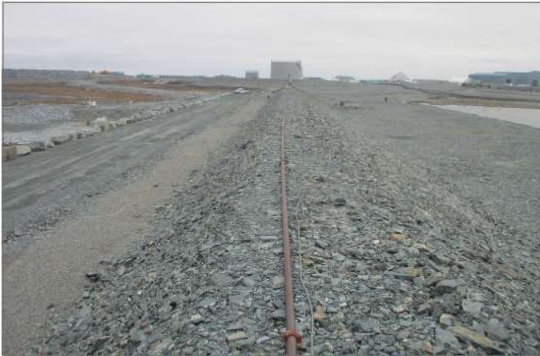
Photo 4: Dike D-CP1 - Crest. Upstream on right, downstream on left.
