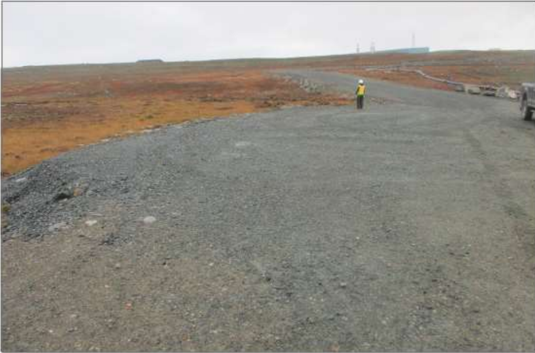
Photo 3: Freshwater Intake Road and turnaround.
