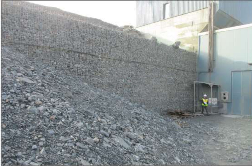
Photo 7: Crusher Pad—MSE wall, north east side.
