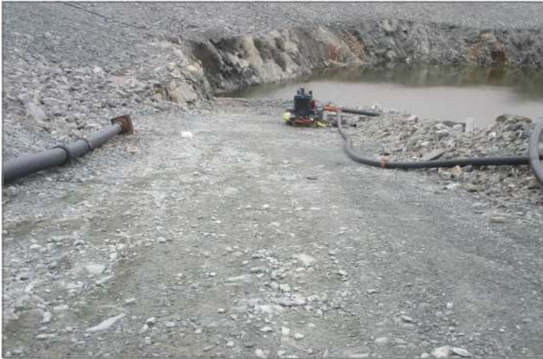
Photo 3: Pond CP4 - Looking north at the ramp into the pond.
