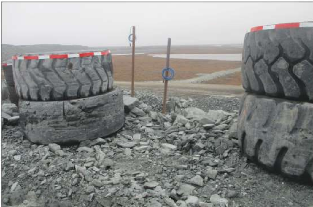
Photo 4: TSF - Thermistors located on edge of TSF embankment.
