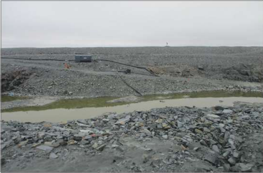
Photo 1: Pond CP3 - Looking southwest, bedrock overburden contact, access ramp into pond.
