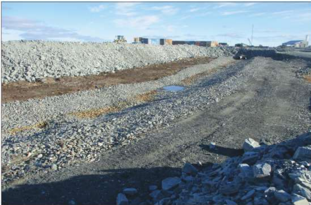
Photo 36: Channel 7—Lower reach, in good condition.
