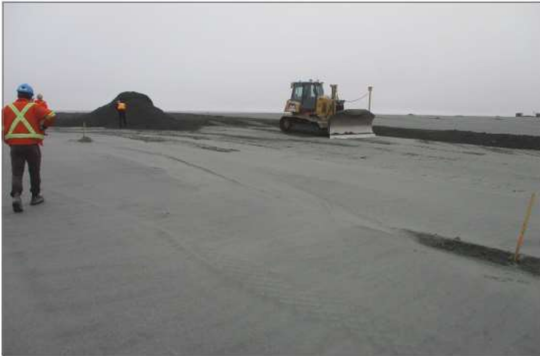
Photo 5: TSF - Spreading tailings.
