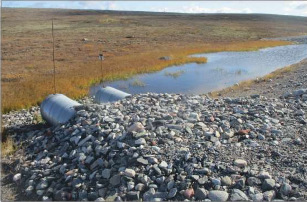
Photo 3: Culvert C09 (C10).
