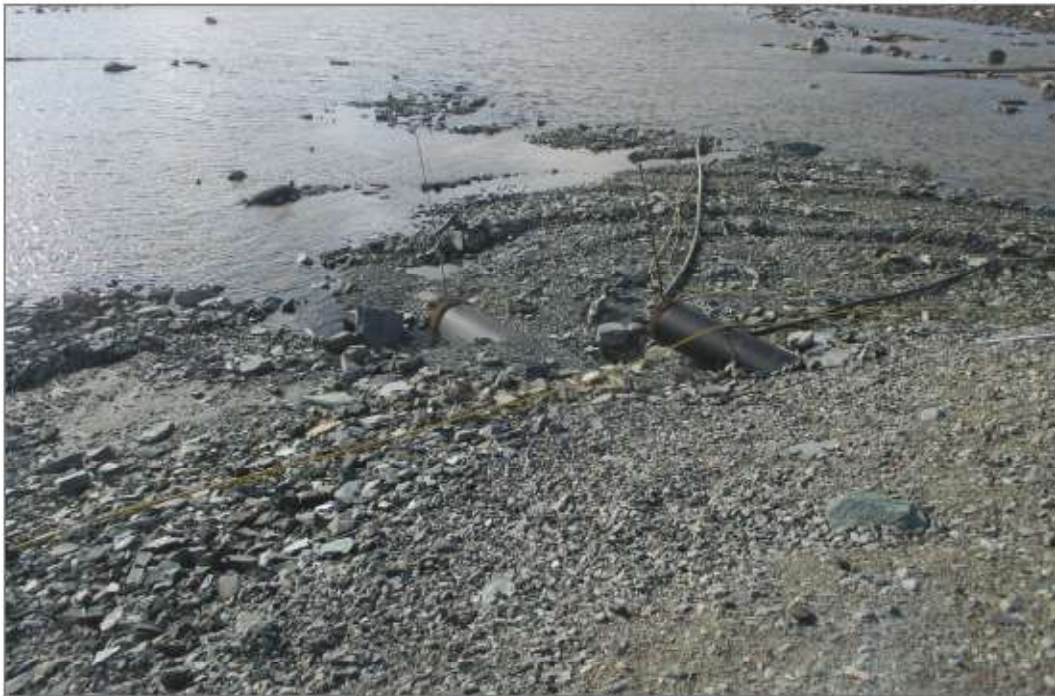
Photo 10: CP5 Jetty 5 - Exposed jetty pump intake in CP5
