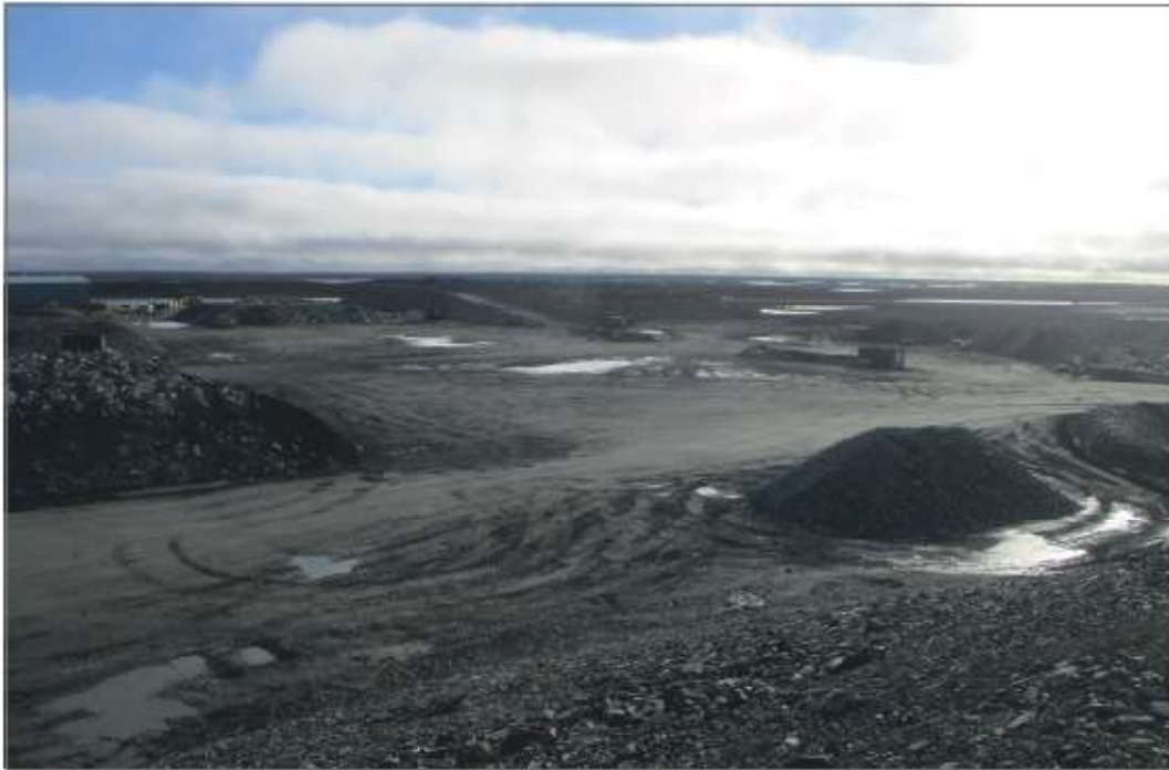
Photo 2: Ore Stockpile Area—Viewed from crusher ramp.
