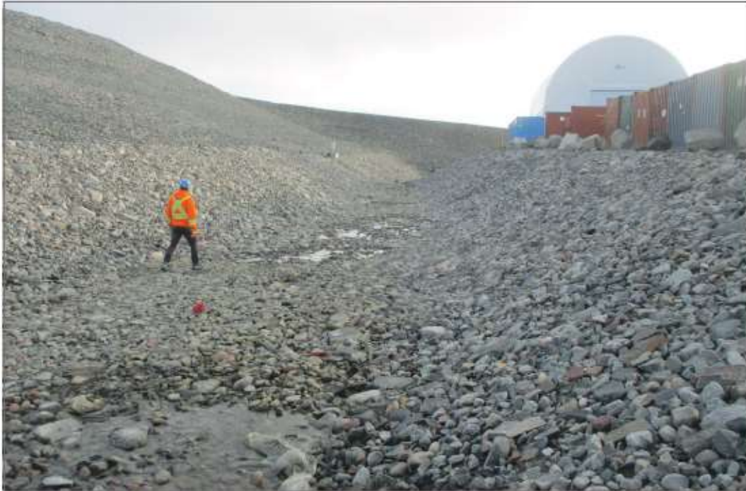
Photo 1: Channel 1—Upper reach, crusher ramp embankment to the left, looking east
