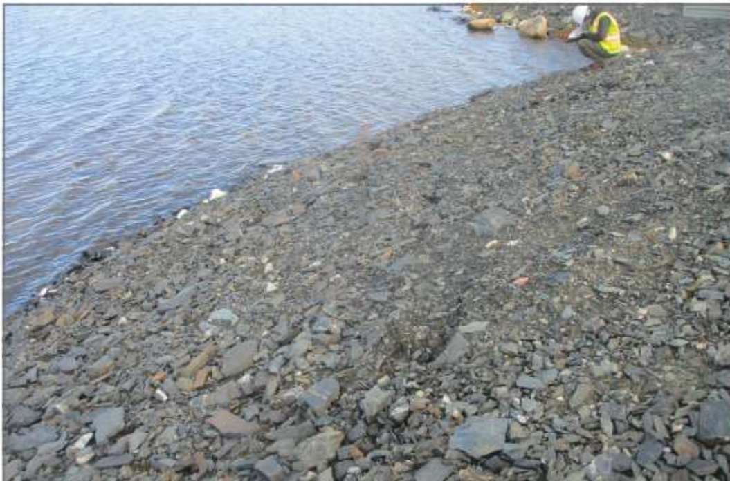
Photo 18: M-5 Bridge—South Abutment cracks along east side.
