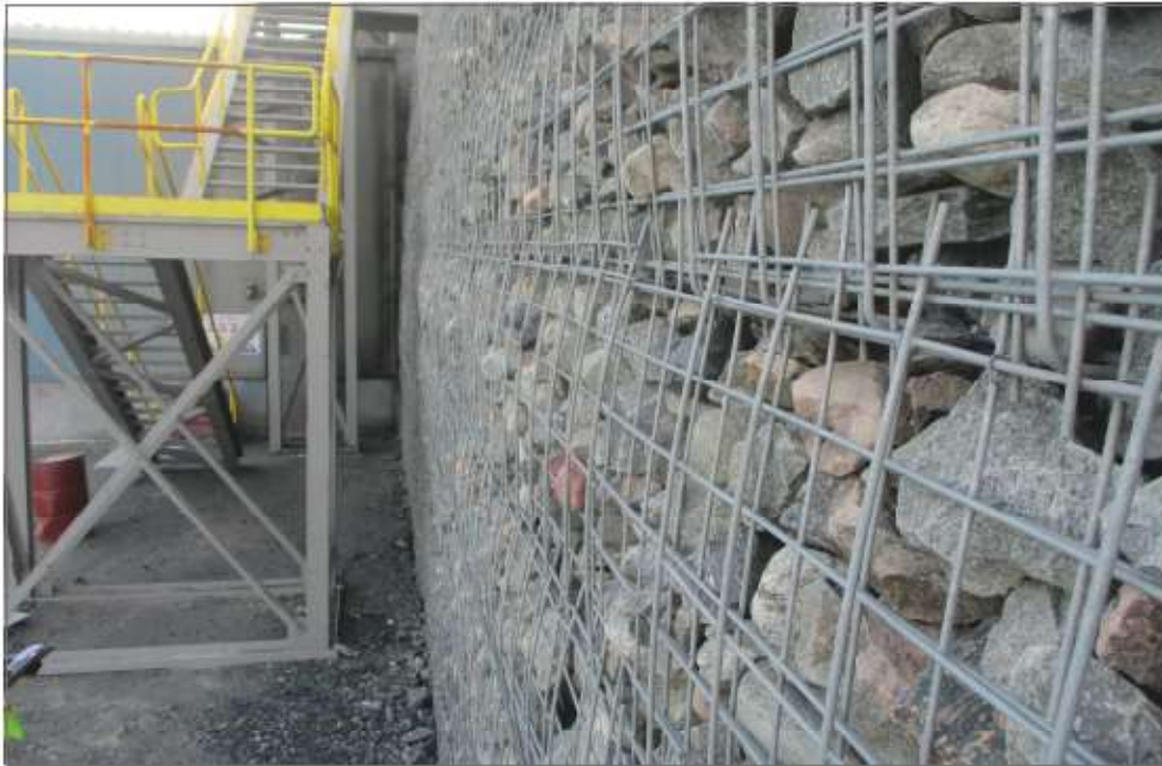
Photo 6: Crusher Pad—Closeup of MSE Wall on the northwest corner.
