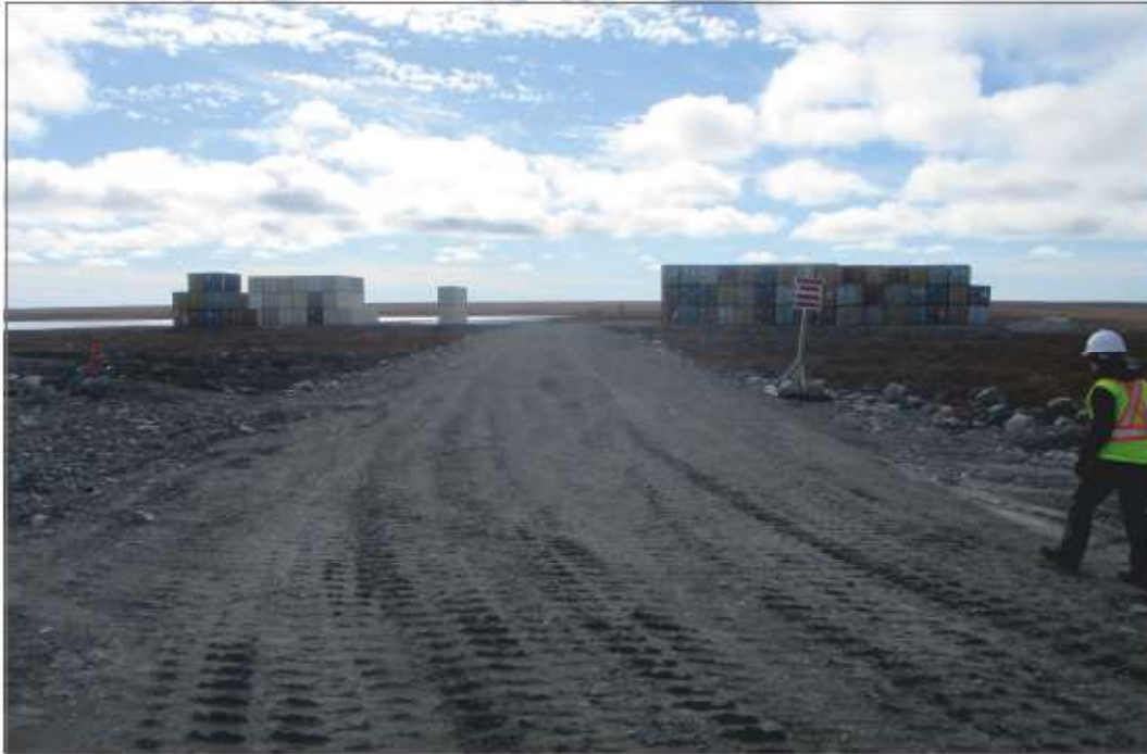
Photo 5: Emulsion Storage Pad access road.
