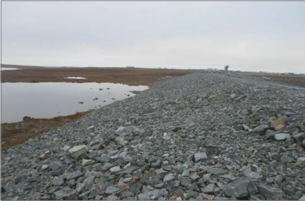
Photo 9: Berm CP3 - Berm downstream crest, looking North.
