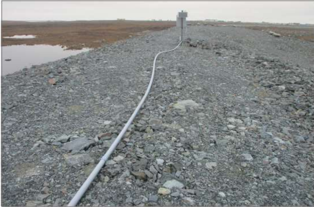
Photo 7: Berm CP3 - GTC instrumentation loggers installed on berm.
