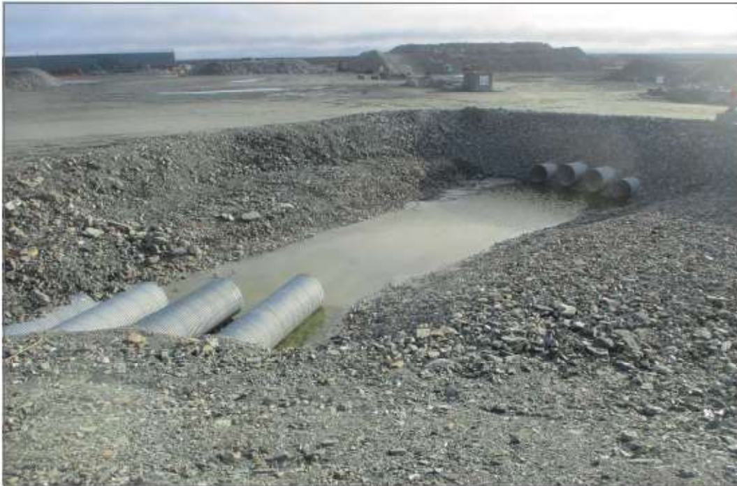
Photo 3: Channel 1—Channel length between crusher ramp and ore pad access.
