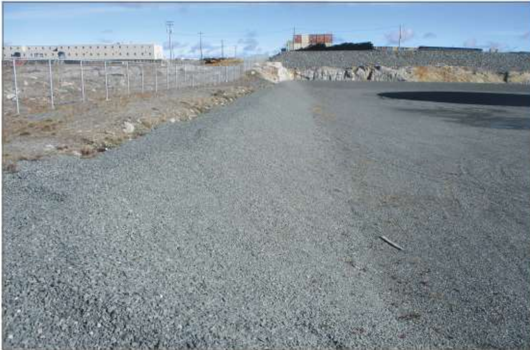
Photo 17: ITVIA Tankfarm—West berm of tankfarm
