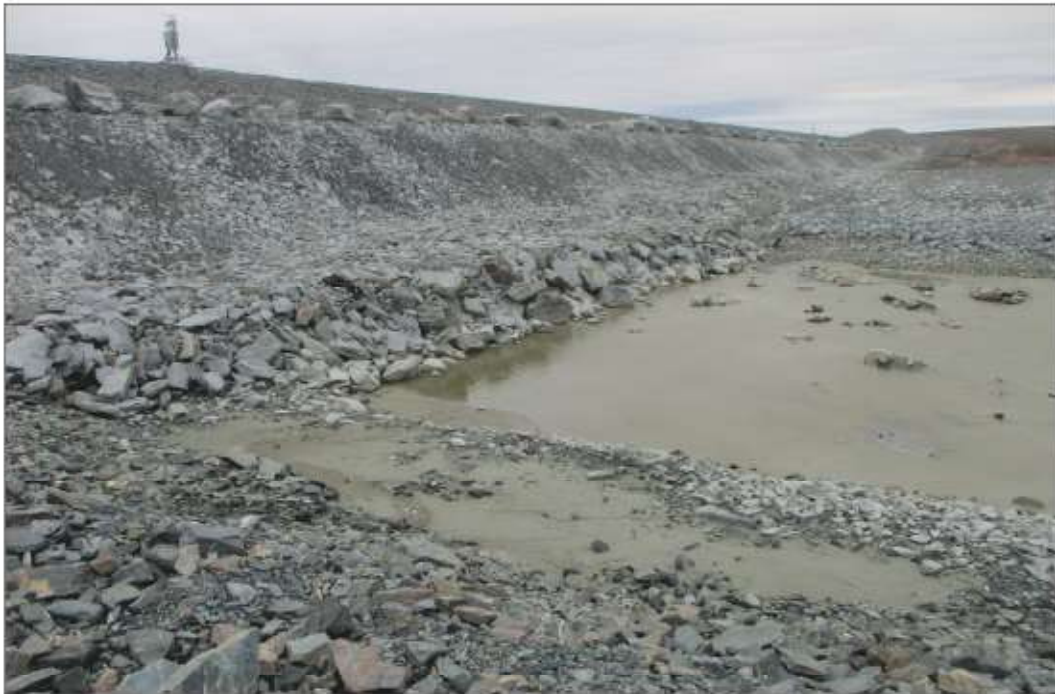
Photo 8: Dike D-CP1 - Downstream crest and sump built up with rockfill.
