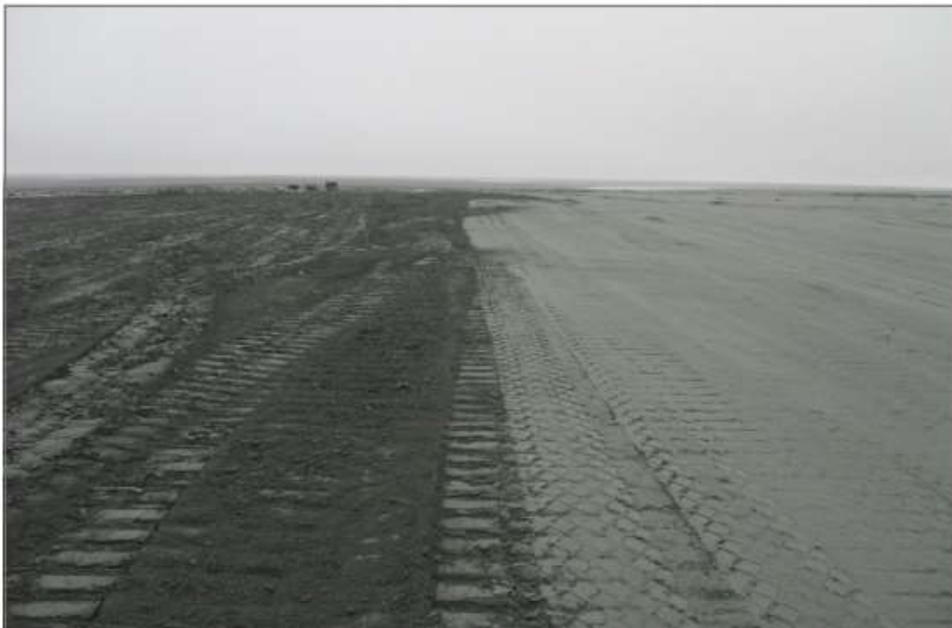
Photo 6: TSF - Compacting tailings.
