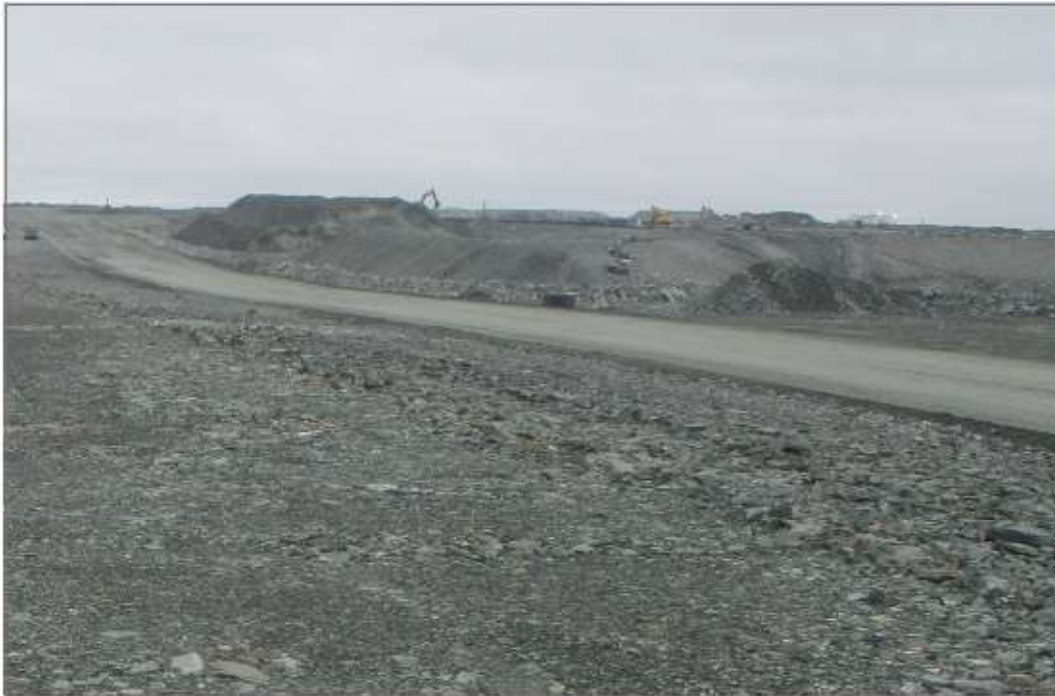
Photo 11: Site Roads—Haul road between Tiri1 and Tiri2 Pits, adjacent D-CP1.
