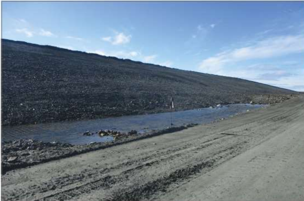
Photo 3: TSF - East slope, access road in foreground.
