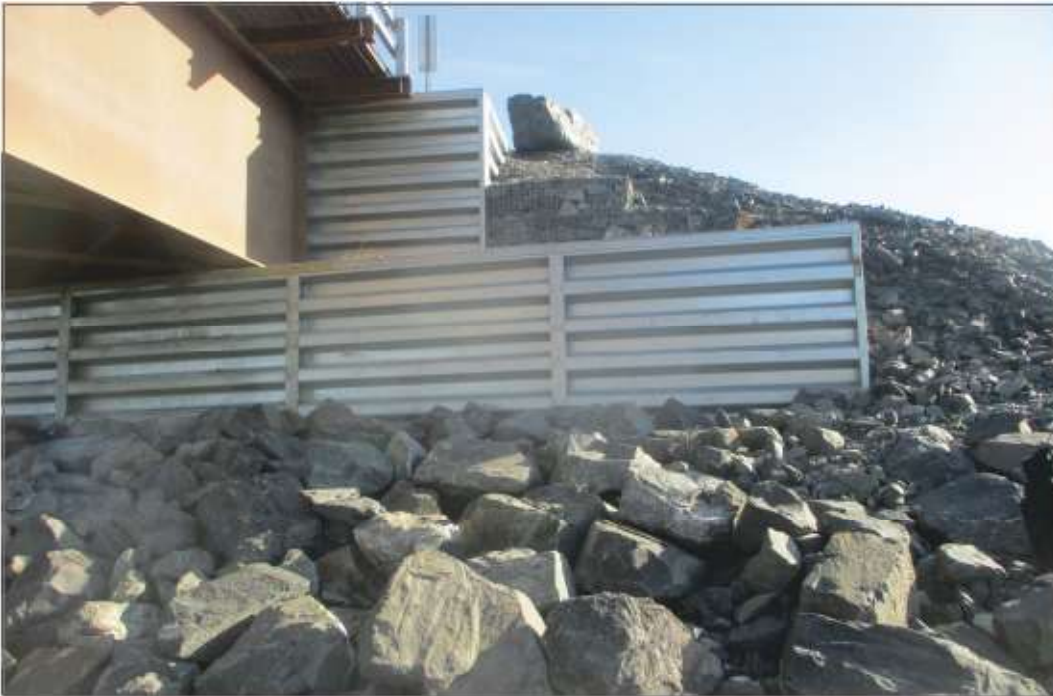
Photo 13: Meliadine River Bridge—North abutment.
