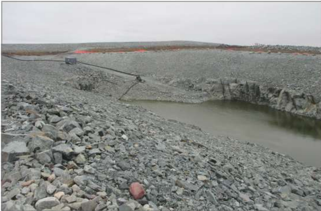
Photo 4: Pond CP4 - South slope—rockfill covered slope, no obvious signs of distress.
