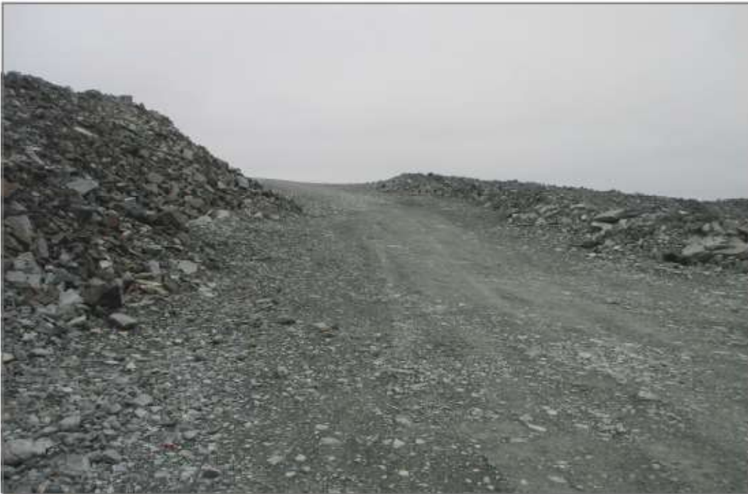
Photo 6: WRSF3—Access ramp from WRSF3 to CP6.
