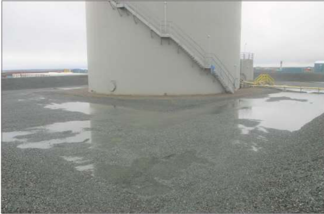
Photo 25: Industrial Fuel Storage Tanks.—Ponded water in tankfarm.
