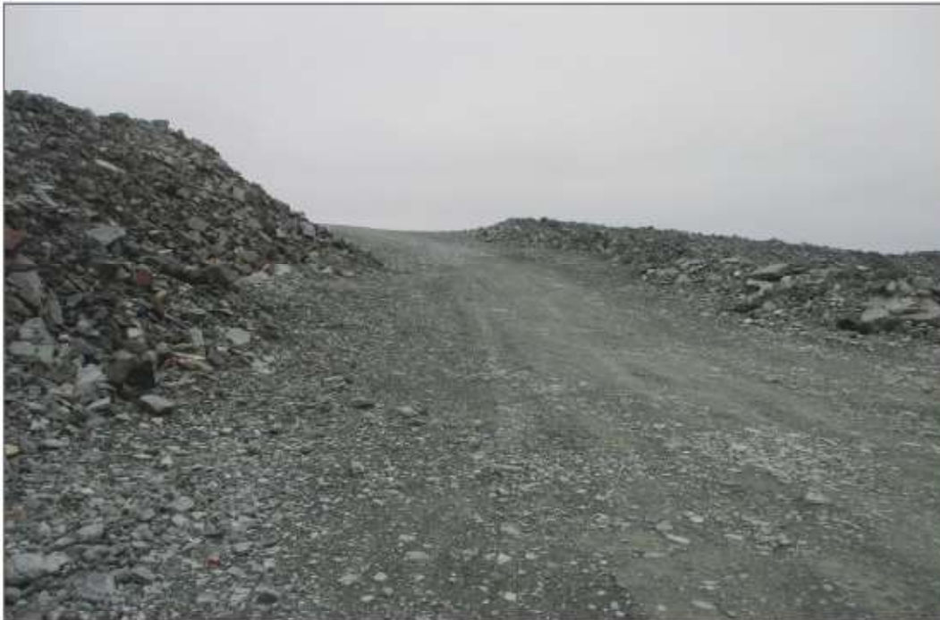
Photo 10: Pond CP6 - Ramp from WRSF3 to CP6 area.
