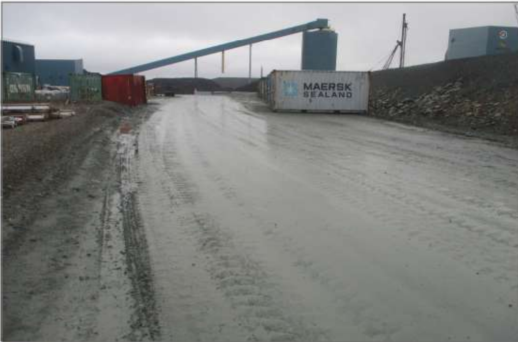
Photo 8: Site Roads—Service road adjacent landfarm and industrial tankfarm.
