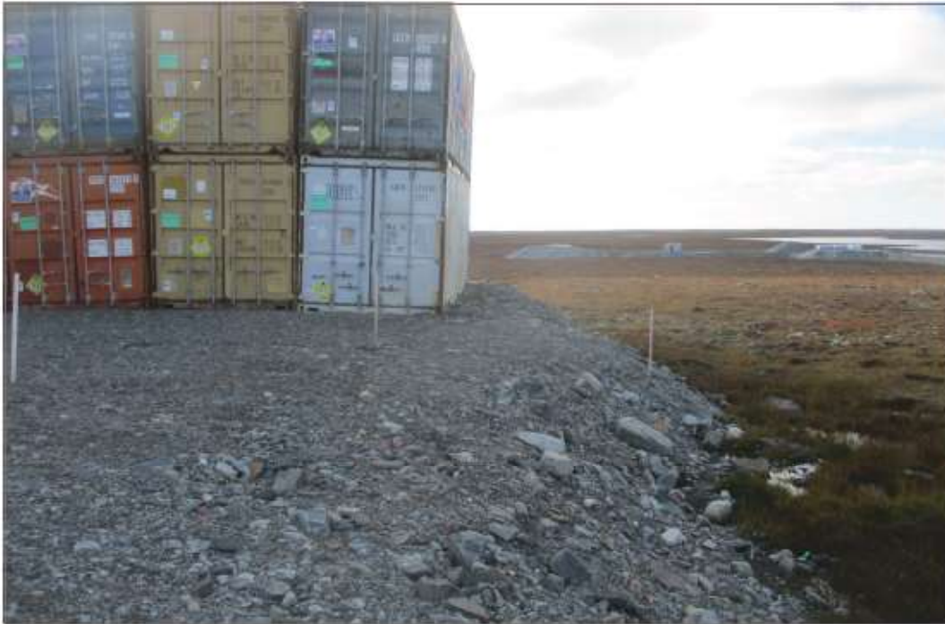
Photo 17: Emulsion Plant—Storage Area—slope on north edge of pad, slight lean to shipping containers.
