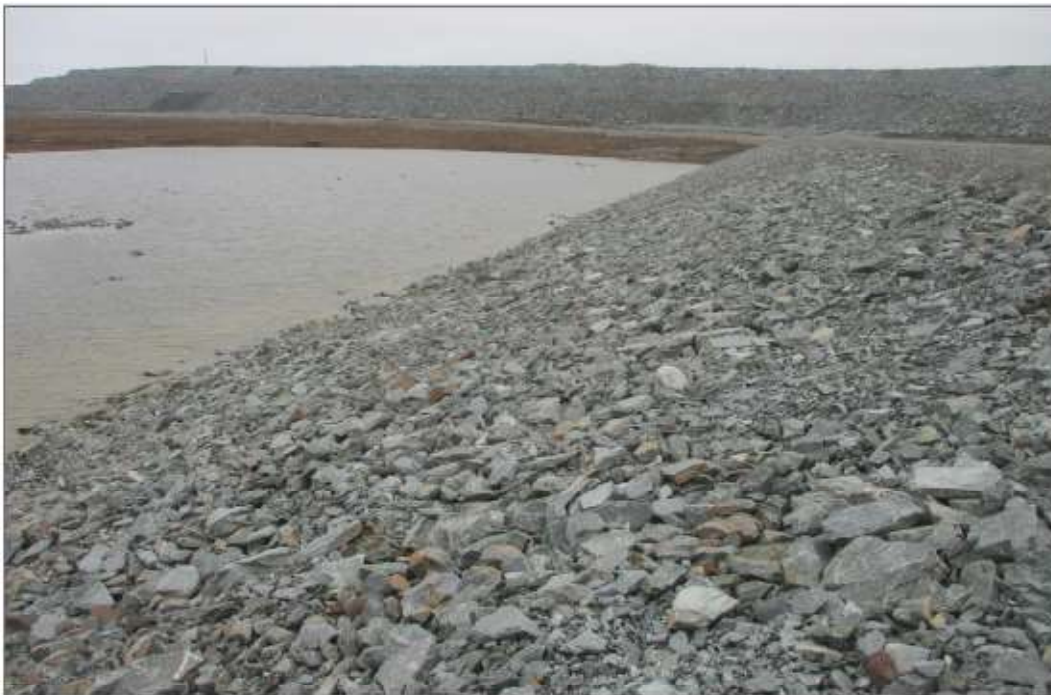
Photo 12: Berm CP4 - Downstream embankment of CP4 berm against lake B8.
