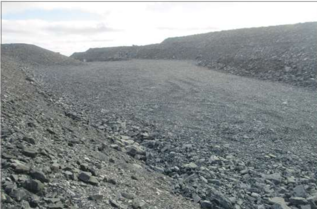
Photo 2: WRSF1—Viewed from Paste Plant Ramp— Backfilled low point along toe of WRSF.
