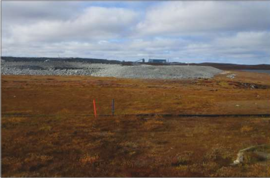
Photo 9: Berm CP2—Overview of berm and downstream area, looking north.
