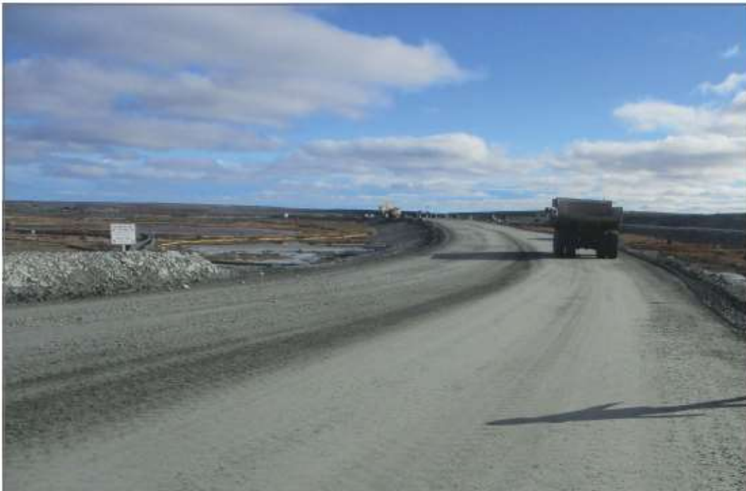
Photo 10: Site Roads—WRSF1 Haul Road, looking south.
