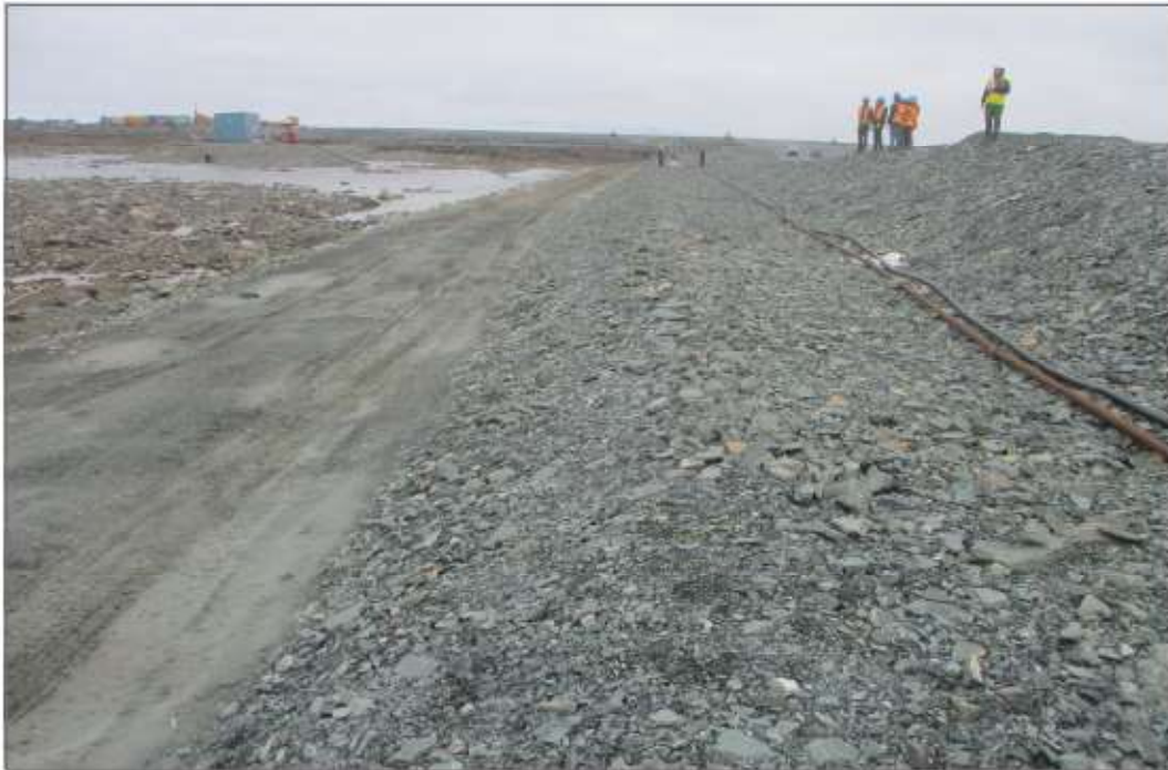
Photo 1: D-CP5 Dike - looking towards the northeast, upstream.
