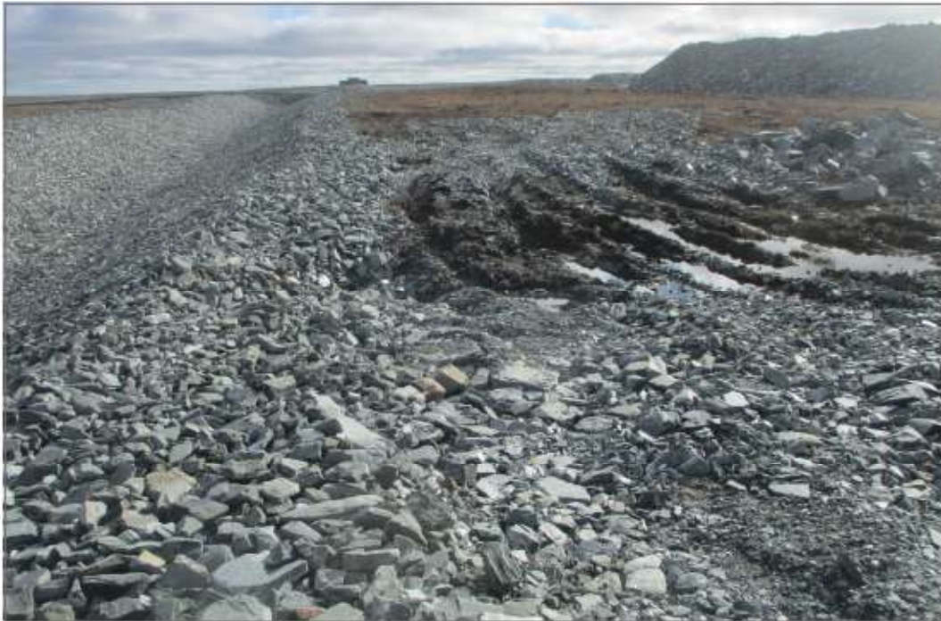
Photo 45: Channel 10—Disturbance to upstream original ground and thaw subsidence.
