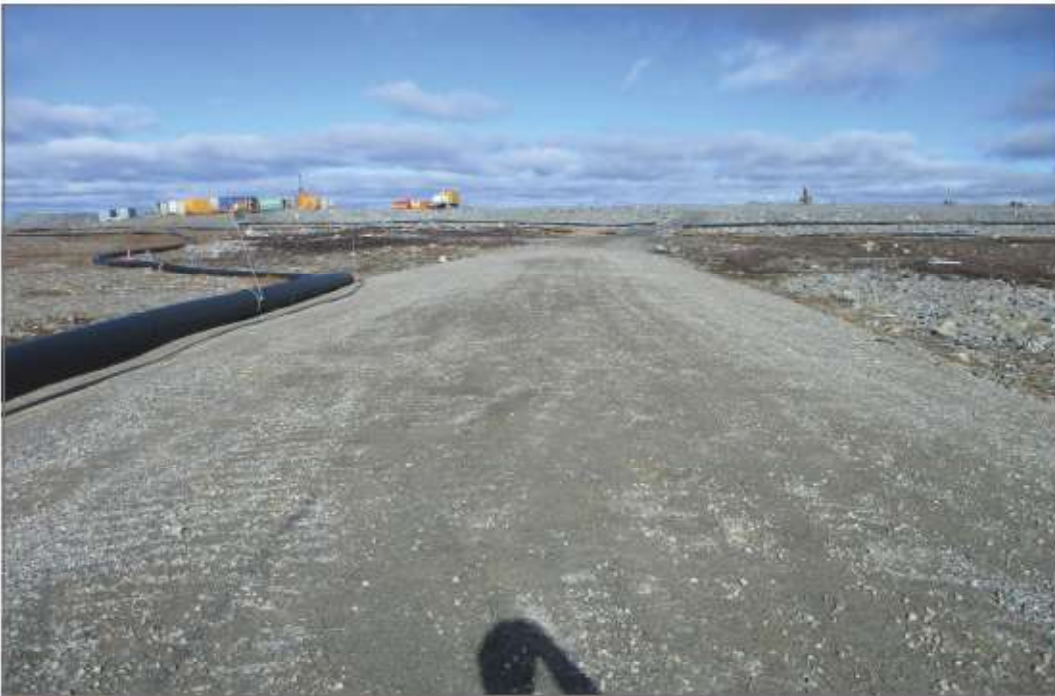
Photo 4: Site Roads—CP5 Jetty Road.
