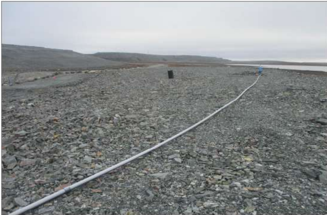
Photo 8: Berm CP3 - Looking south, surface of berm. Undulating settlement and subsidence.
