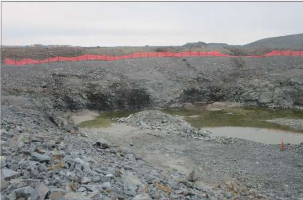
Photo 2: Pond CP3—Looking northeast, water running into CP3 along several points on north side.
