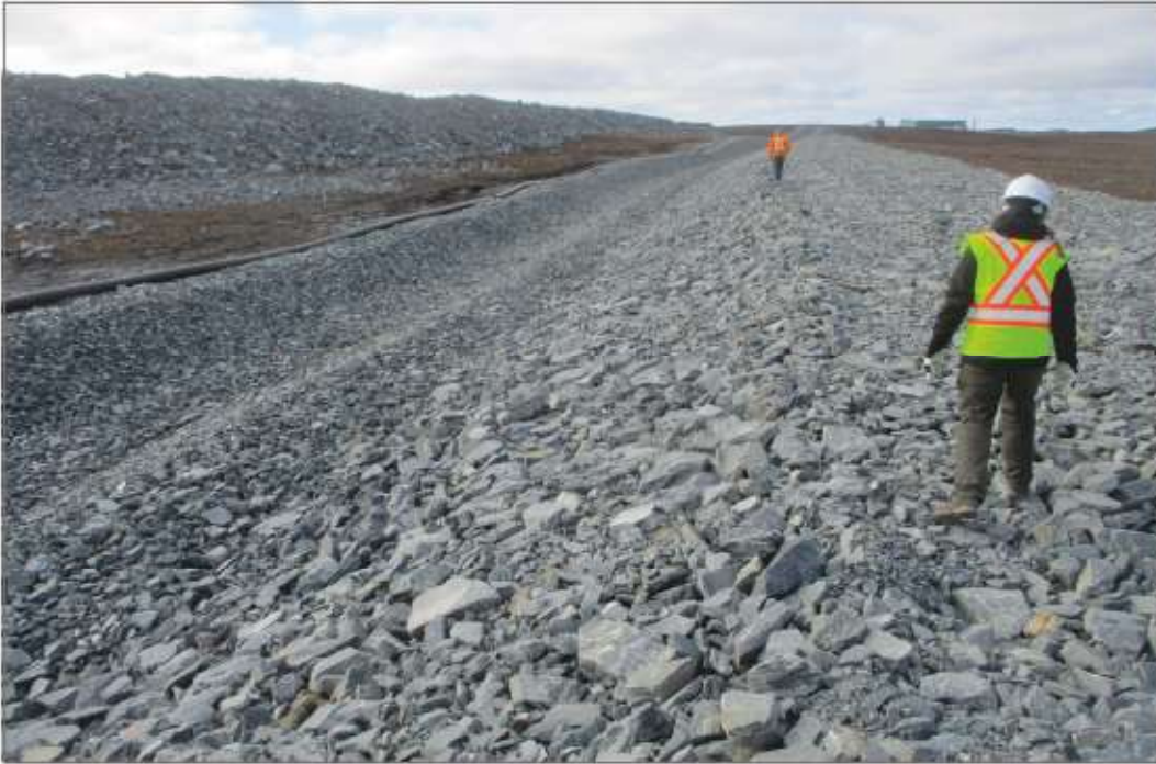
Photo 39: Channel 9—Armoured diversion berm downstream of channel.
