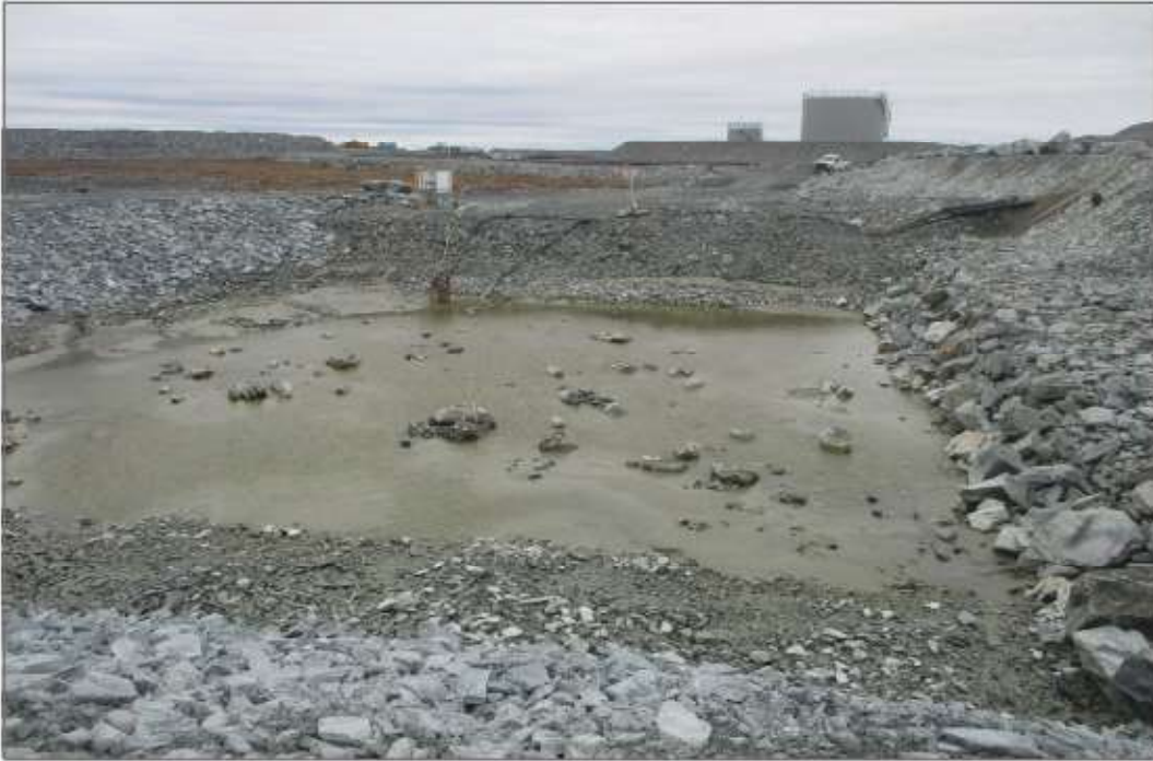
Photo 11: Dike D-CP1 - Water collection pond, east side, rockfill embankments restored.
