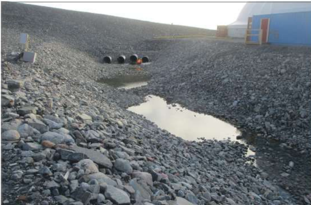
Photo 2: Channel 1—Culvert under the crusher ramp, Berm 1 on the right.
