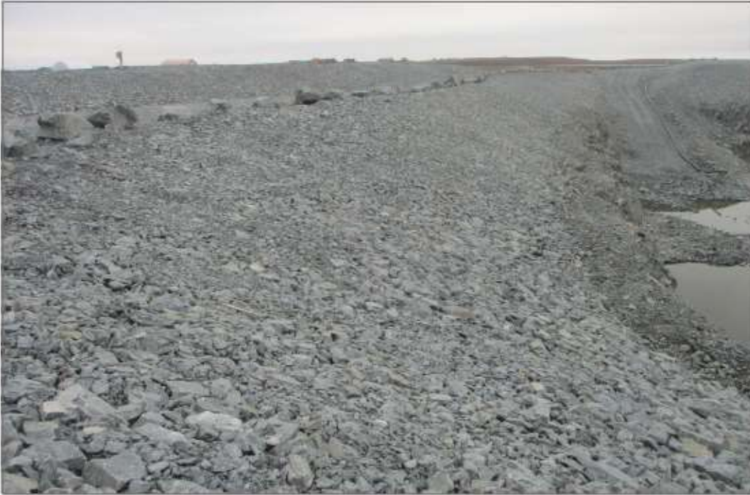
Photo 3: Pond CP2—Looking south, rockfill covered overburden along east side of CP2.
