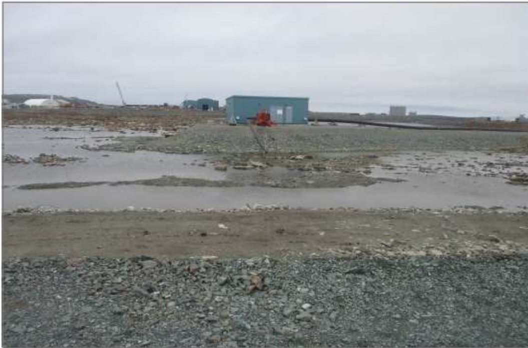
Photo 8: CP5 Jetty 5—Diesel Pumping into Jetty 5 pump well.
