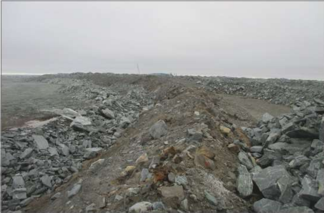
Photo 5: WRSF1—97 m bench surface, overburden placed within limits.
