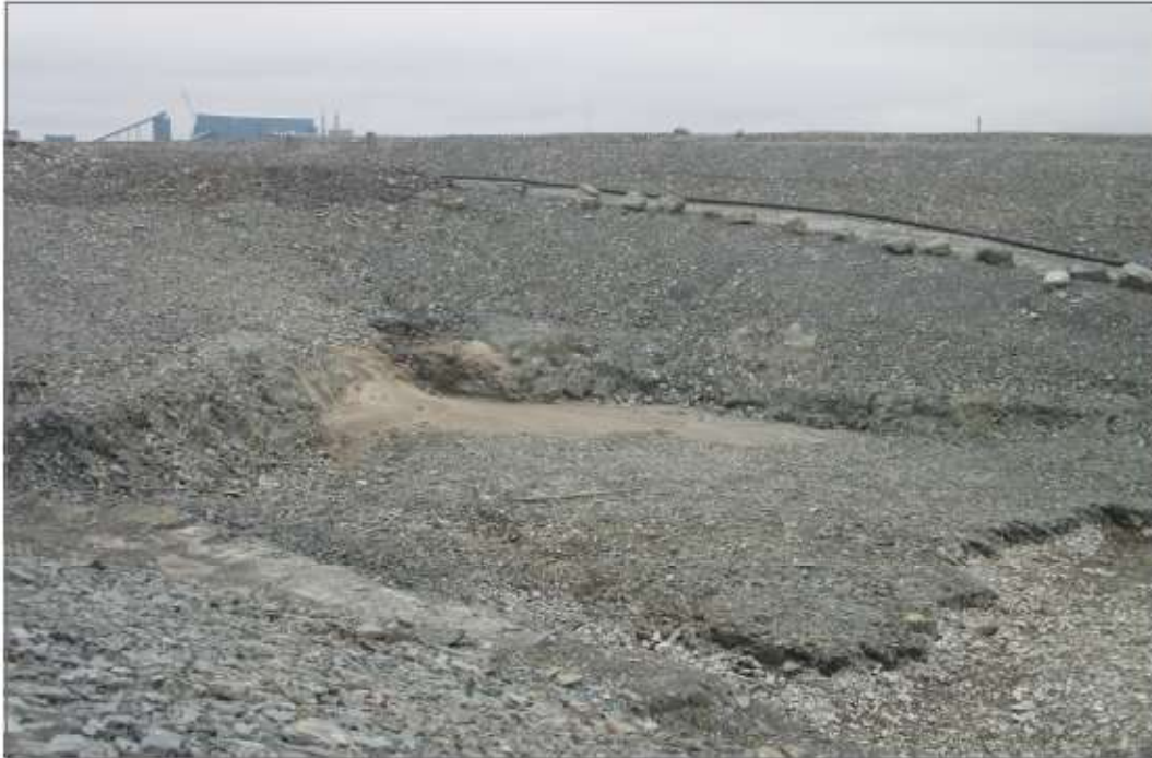
Photo 3: Pond CP6 - Significant sedimentation from water inflow at northwest corner.
