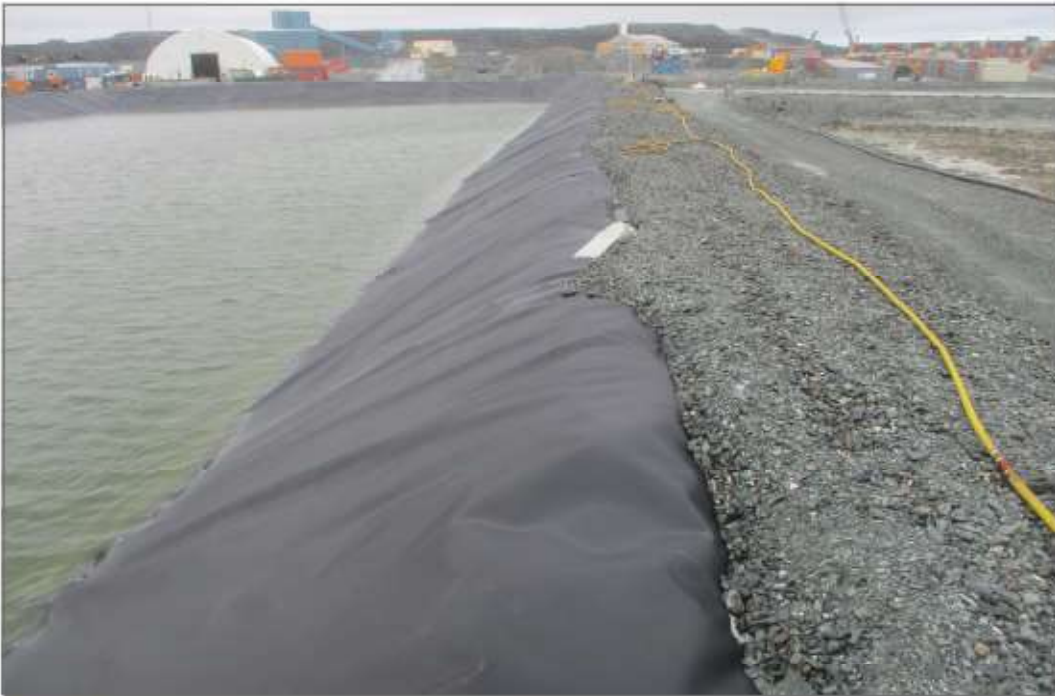
Photo 6: SP3 Saline Pond - looking west, north berm
