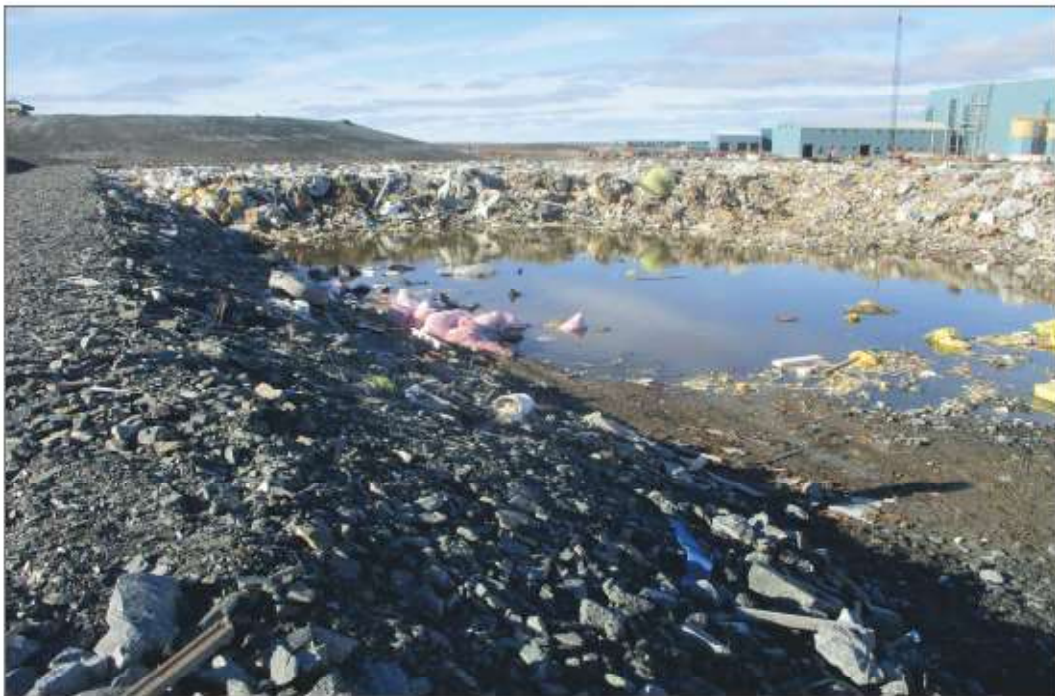
Photo 10: Landfill - WRSF1 Landfill with ponded water.
