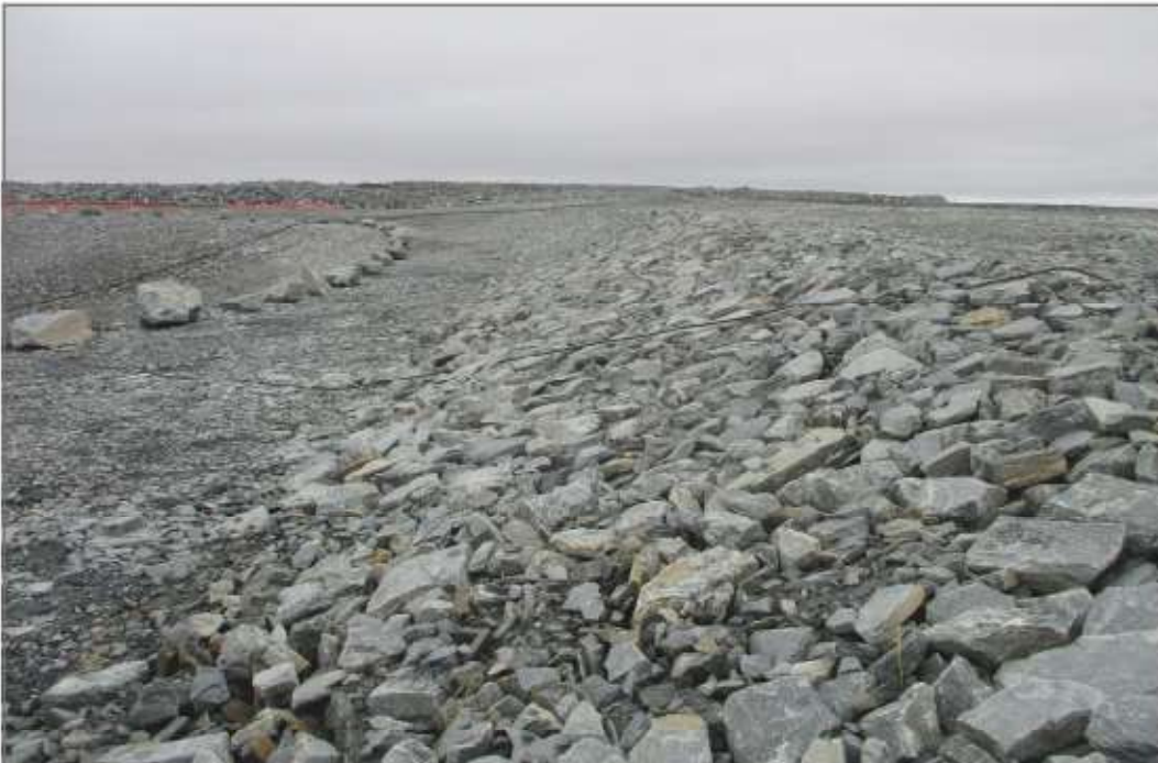
Photo 10: Berm CP4 - Upstream slope, thermal cover above Pond CP4
