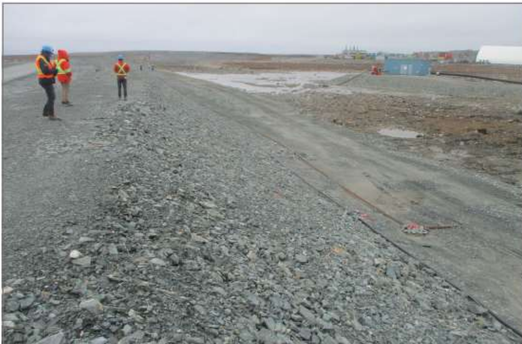
Photo 2: D-CP5 Dike - looking towards the southwest, upstream.
