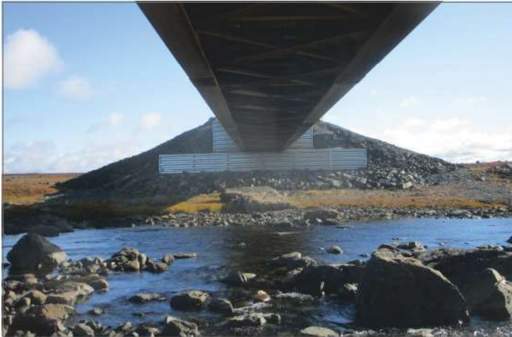
Photo 9: Meliadine River Bridge north abutment
