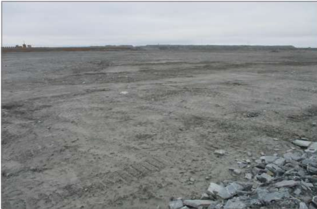
Photo 2: WRSF3 - Condition of overburden surface placed during west expansion.
