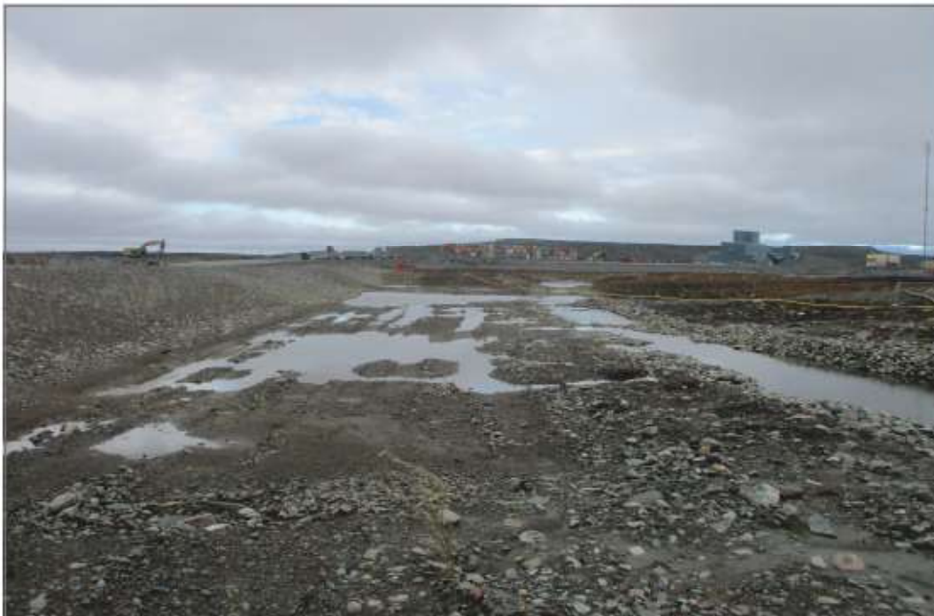
Photo 32: Channel 5—Water level in channel controlled by CP5, pooling in low area against Berm3, looking west.
