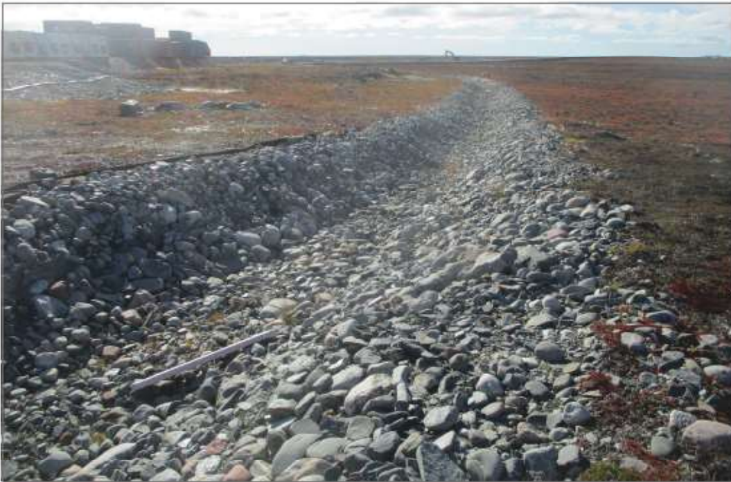
Photo 10: Channel 2—In good condition.
