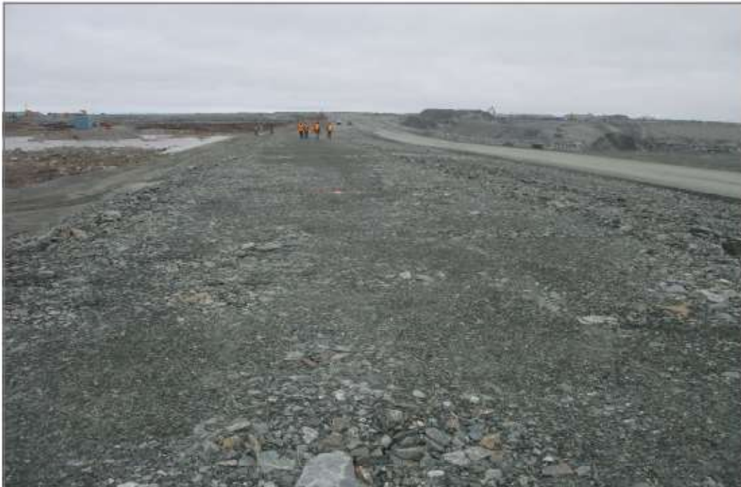
Photo 6: D-CP5 Dike - Crest of dike, looking northeast.
