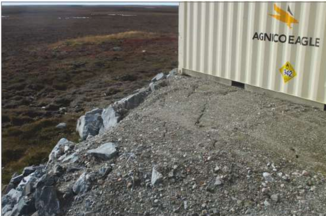
Photo 18: Emulsion Plant—Storage Area—Shipping container placed on edge of pad crest at south corner.
