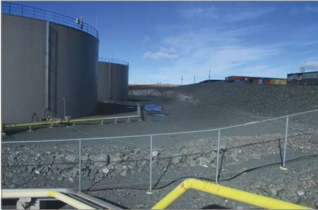
Photo 11: ITIVIA Tankfarm—North of tanks.
