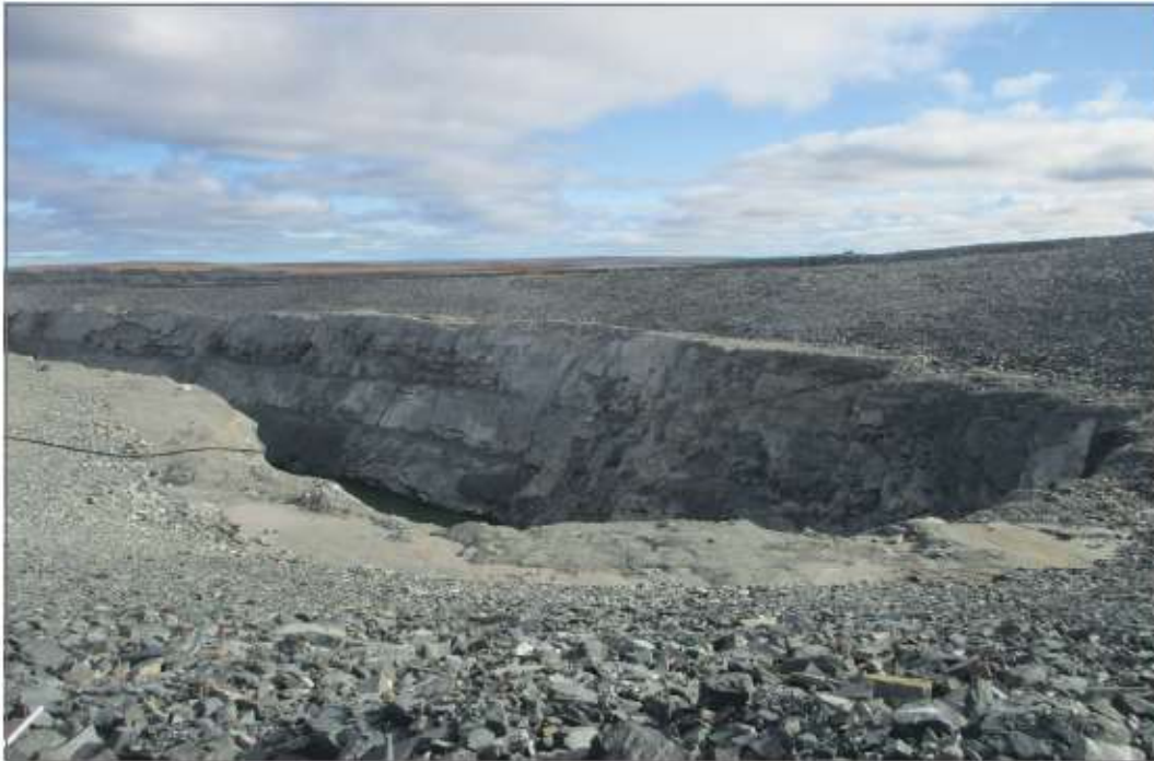
Photo 15: SP4 Saline Pond—Rockfill cover, no significant deformation. Bedrock below slope.
