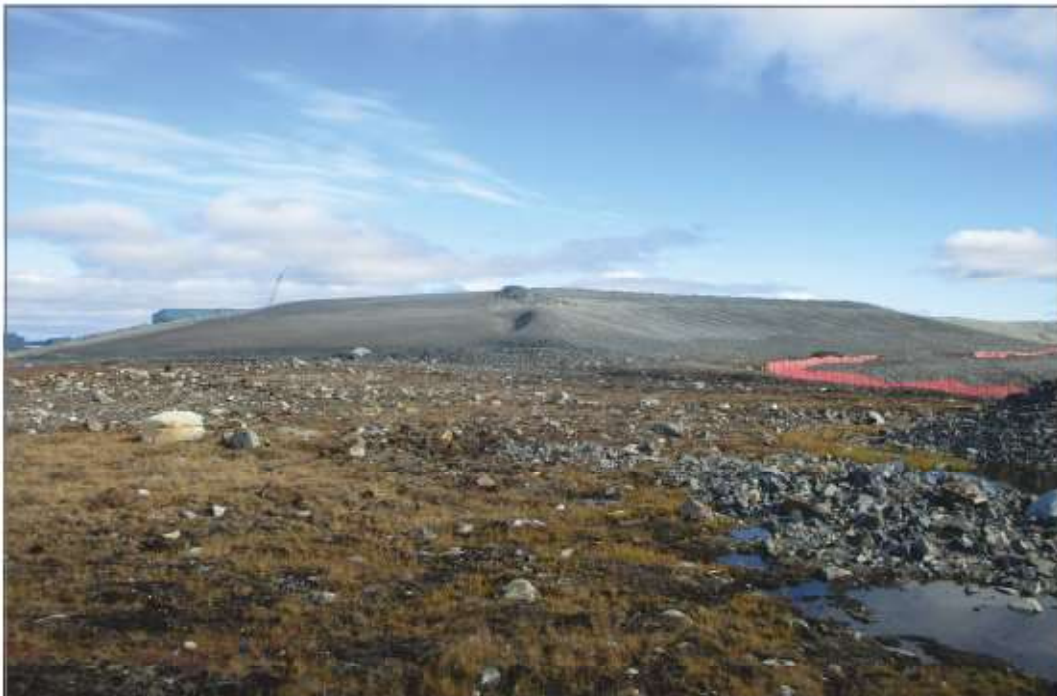
Photo 2: TSF—North side of Cell 1—Rockfill slope covering west side of TSF
