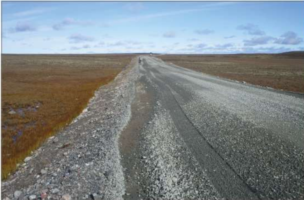
Photo 1: Overview of Bypass Road from KM 5.1 North
