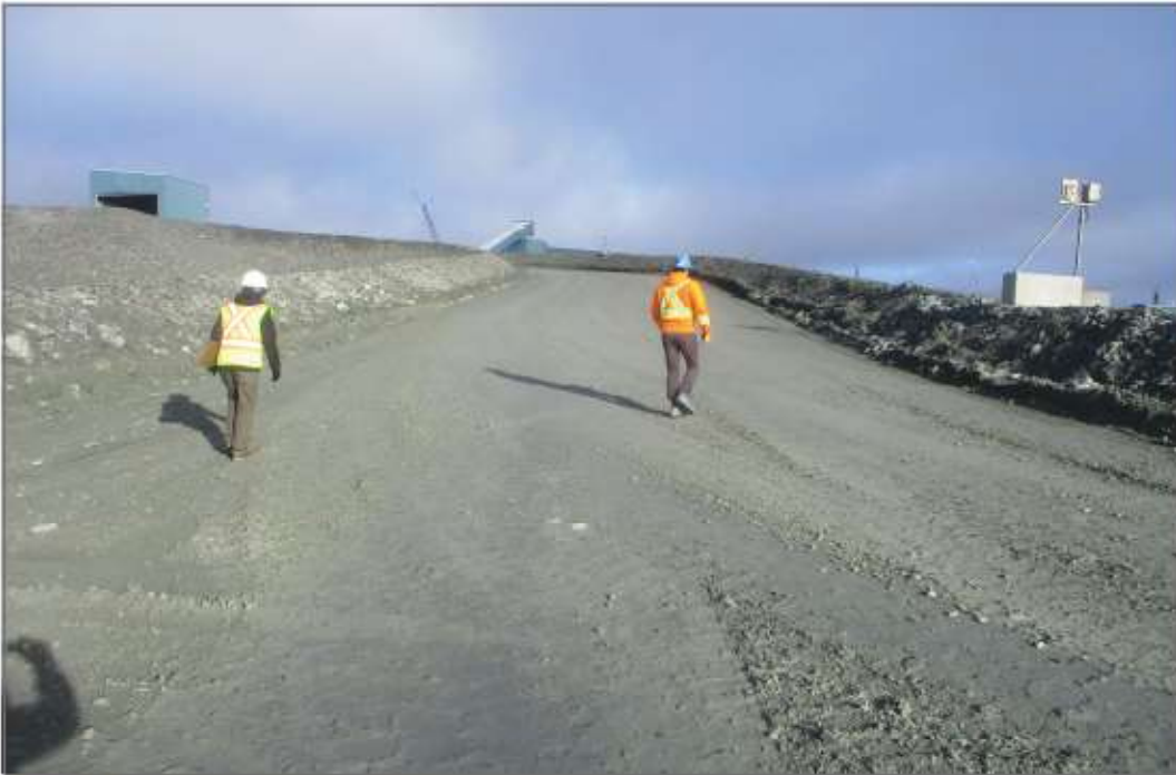
Photo 4: Crusher Pad —Ramp access.
