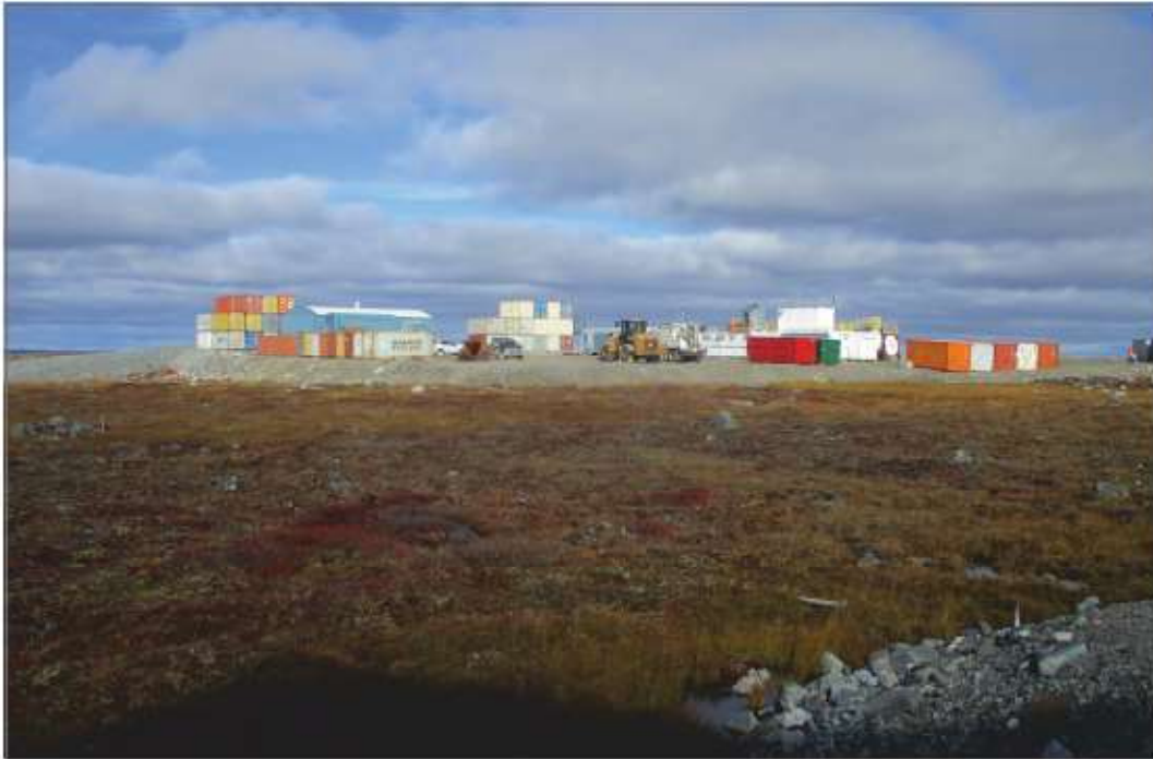
Photo 15: Emulsion Plant—Overview from southwest direction
