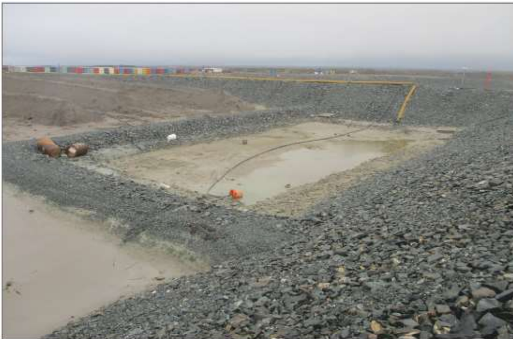
Photo 20: Landfarm—Water collection pond with low ponding and sedimentation.
