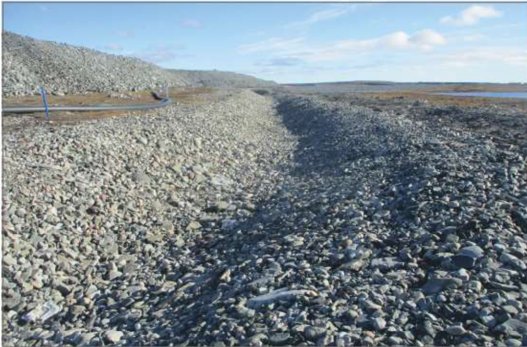
Photo 24: Channel 4—Looking south.
