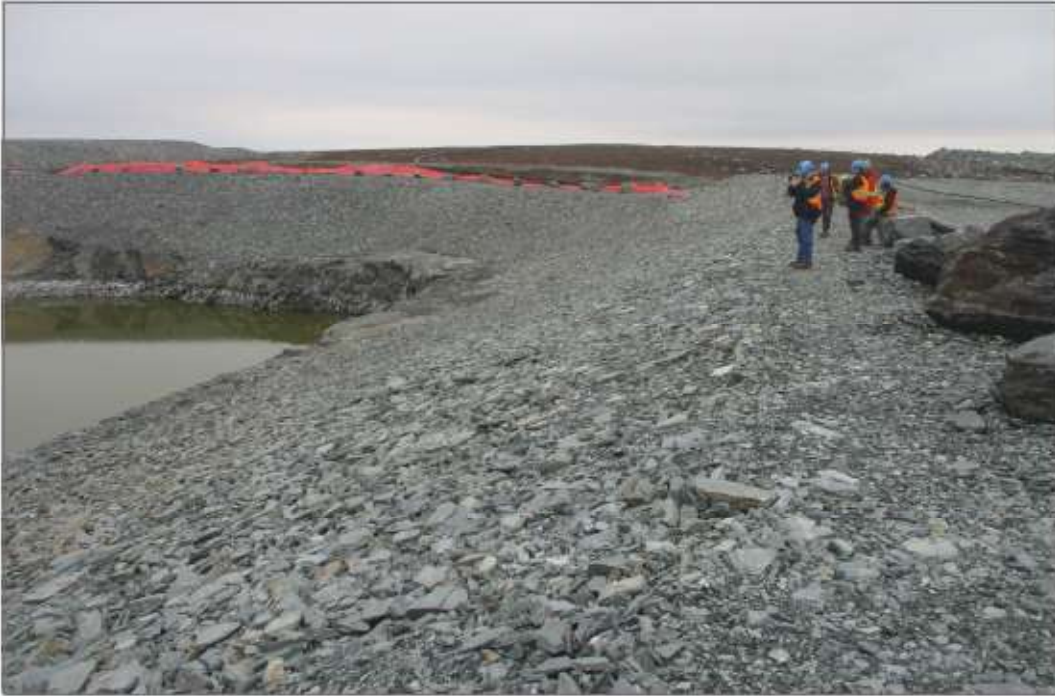
Photo 1: Pond CP6 - Looking east —Rockfill covered overburden, south embankment.
