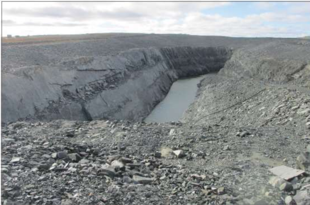
Photo 8: SP4 Saline Pond - Looking west, rockfill covered slopes.
