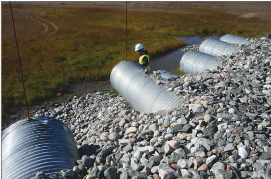
Photo 6: Culvert C10 (C11 on sign).
