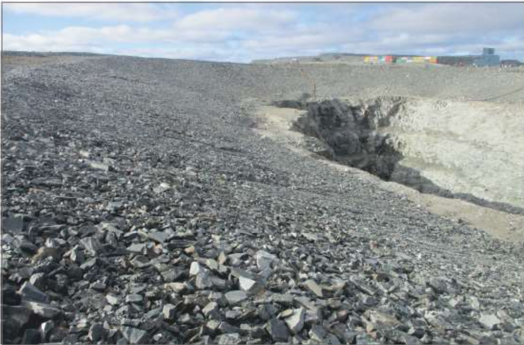
Photo 12: SP4 Saline Pond - Rockfill covered slope, looking northwest.
