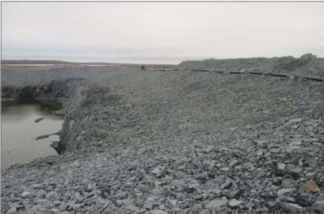
Photo 4: Pond CP2—Looking south, rockfill covered overburden along west side of CP2.
