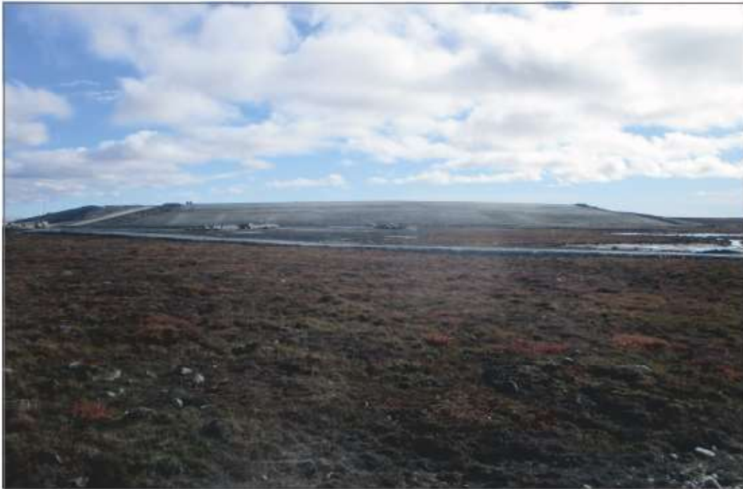
Photo 1: TSF - North side of Cell 1
