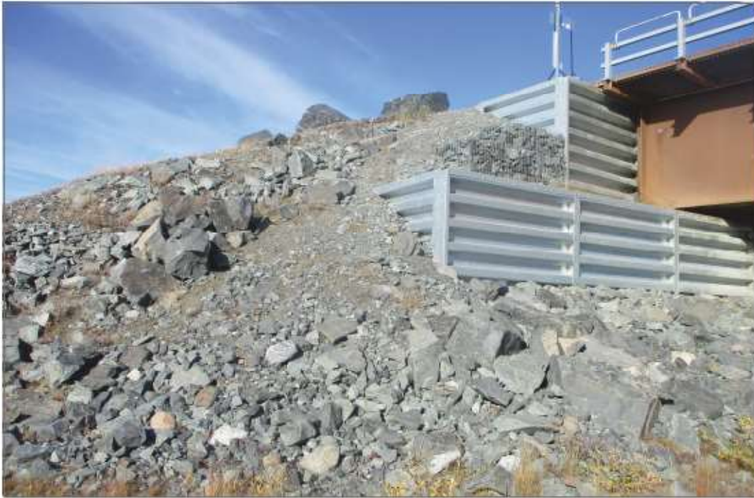
Photo 11: Meliadine River Bridge north abutment
