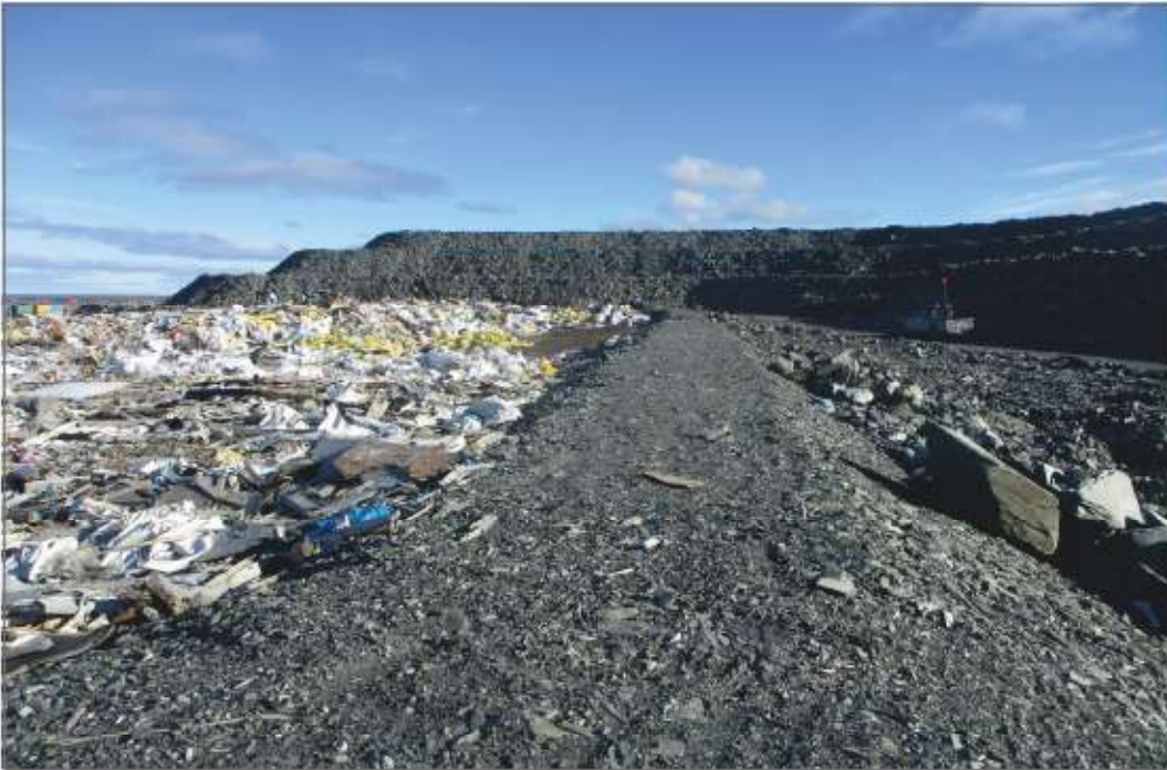
Photo 12: Landfill – WRSF1 Landfill—Southwest berm.
