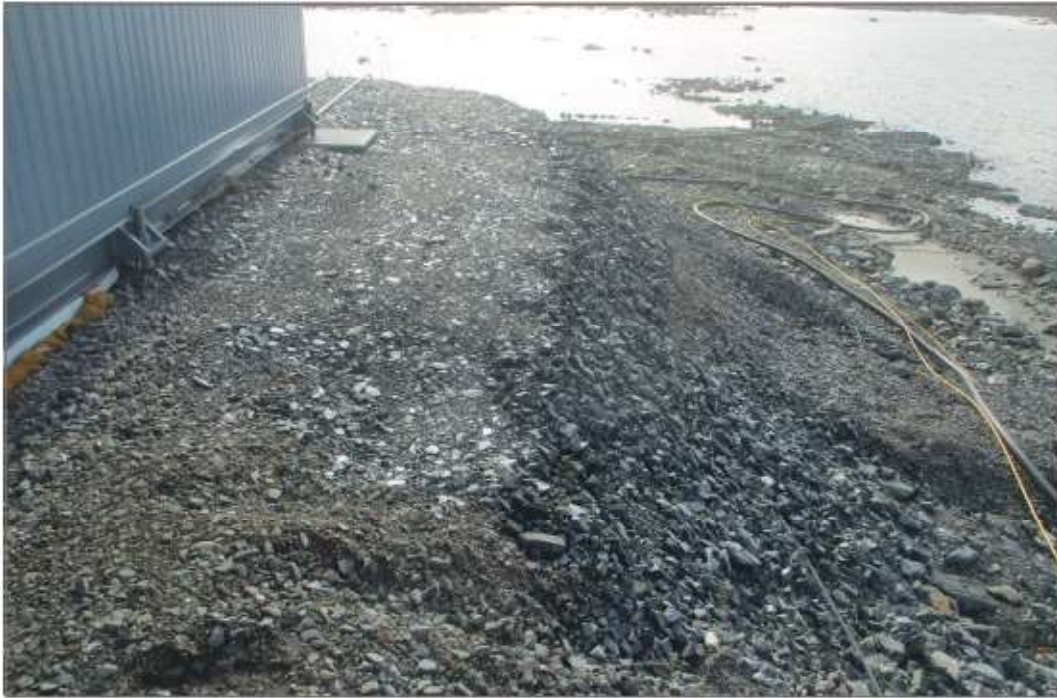
Photo 9: CP5 Jetty 5 - Repaired footing erosion from 2021.
