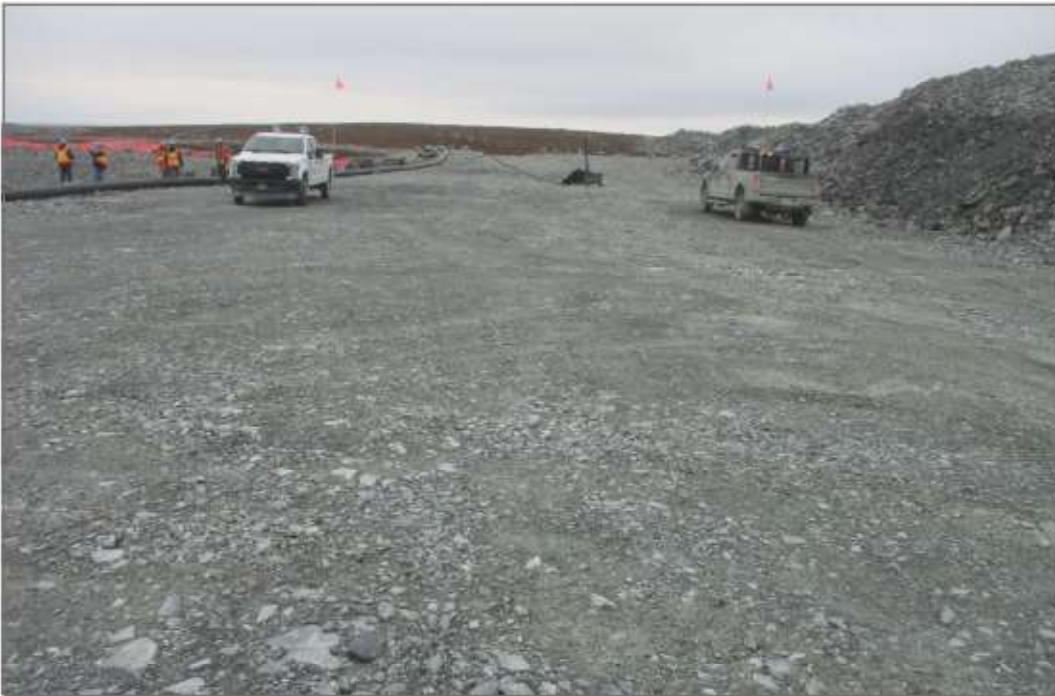
Photo 2: Pond CP6—Ground between WRSF3 and CP6—filled with ROM June 2021. ROM placed to reduce erosion in former lakebed sediments.
