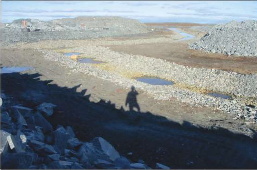
Photo 37: Channel 7—Outlet into Channel 1, ore stockpile in background.
