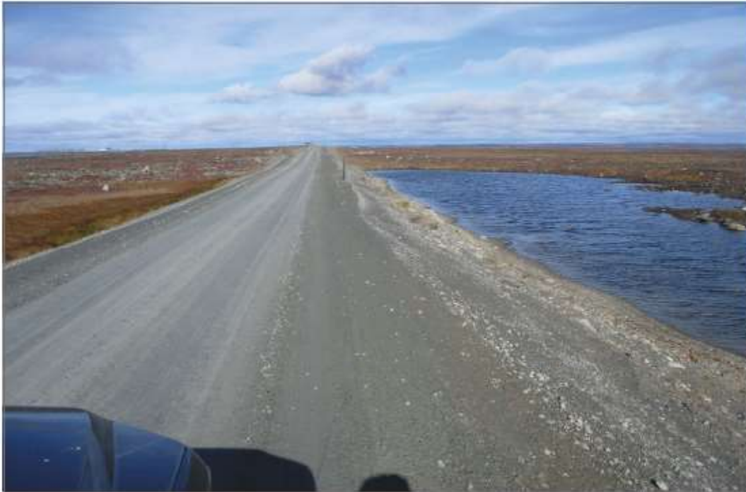
Photo 33: No culvert km 28.7
