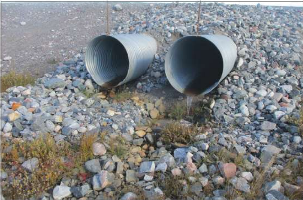
Photo 4: Culvert C09 (C10).
