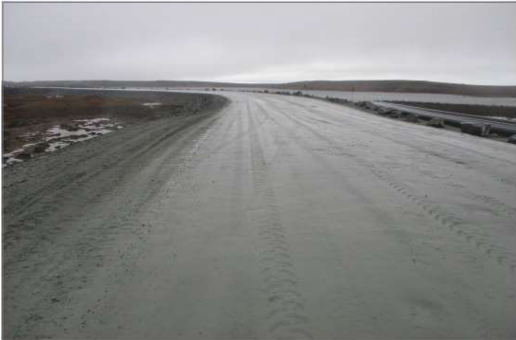
Photo 9: Site Roads—Service road adjacent CP1, looking north.
