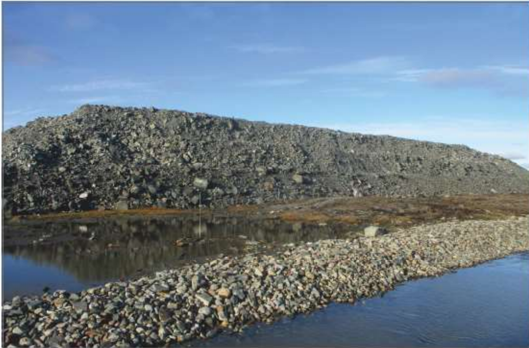
Photo 5: Ore Stockpile—South side viewed from Channel 1.
