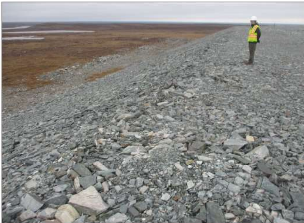
Photo 8: Pond CP6 - Berm CP6—downstream crest.
