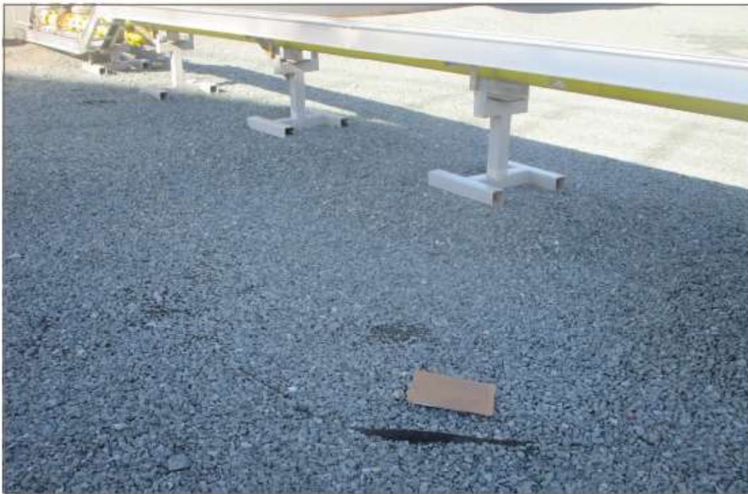
Photo 16: ITIVIA Tankfarm—Geotextile exposed in pad base.
