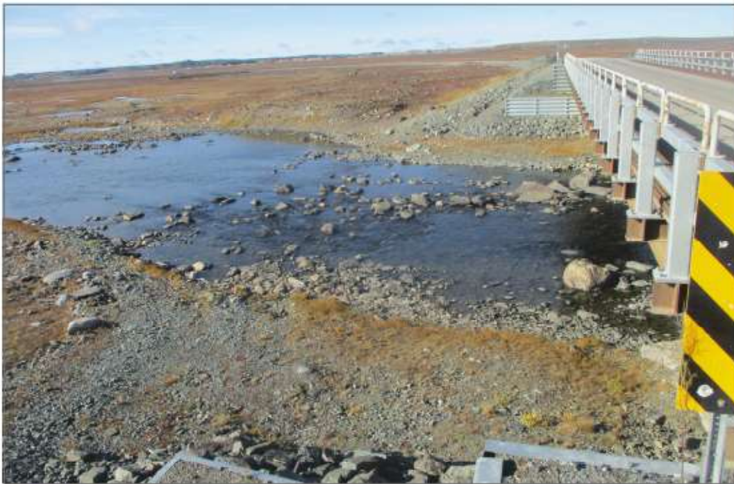
Photo 12: Meliadine River Bridge—Shoreline downstream of bridge
