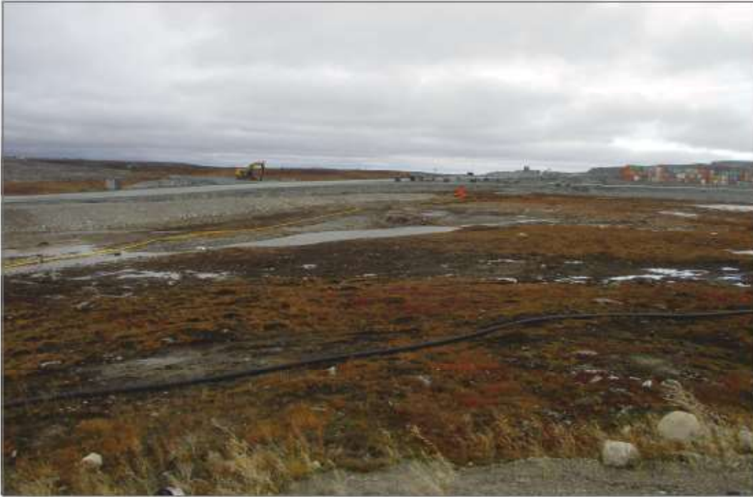
Photo 33: Channel 5—Upper reach looking southwest.
