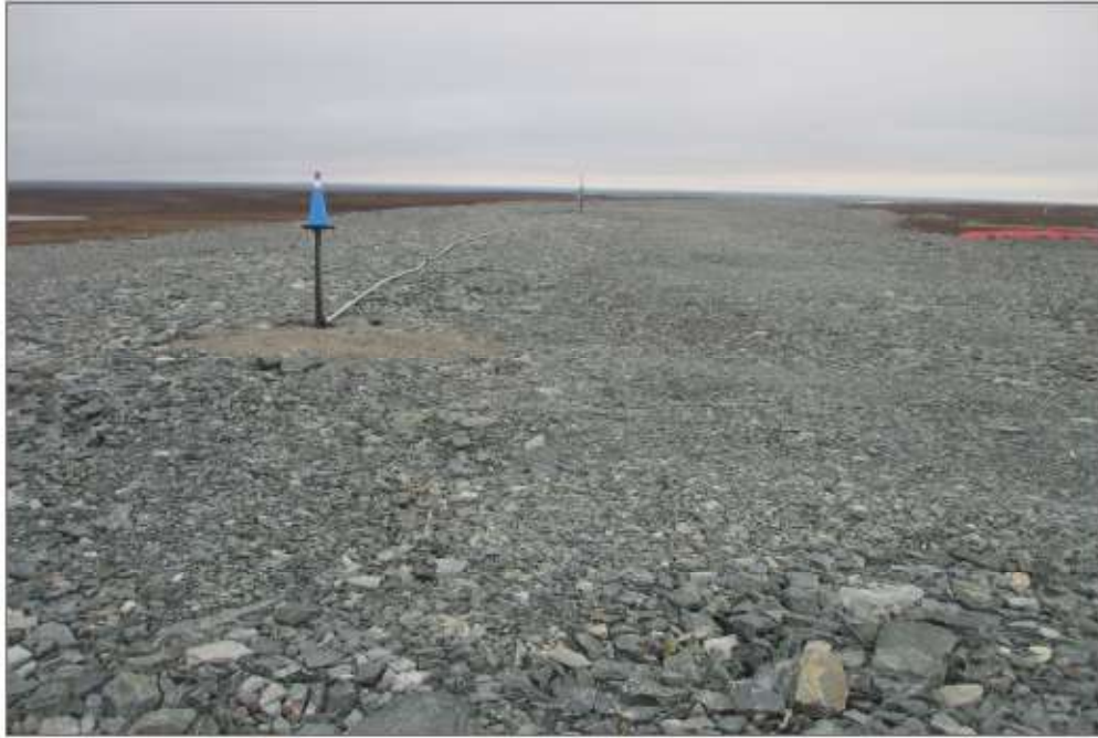
Photo 7: Pond CP6 - Berm CP6 crest. Minimal settlement.
