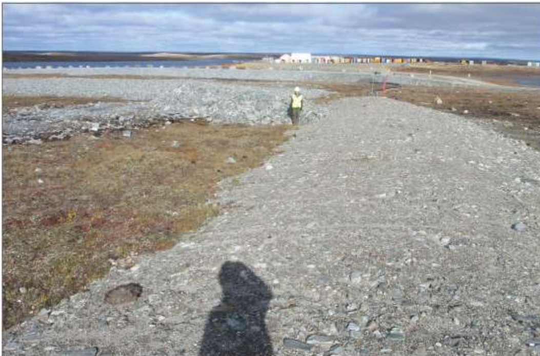
Photo 46: Channel 10—Channel inlet diversion berms, low area in berm tie-in .
