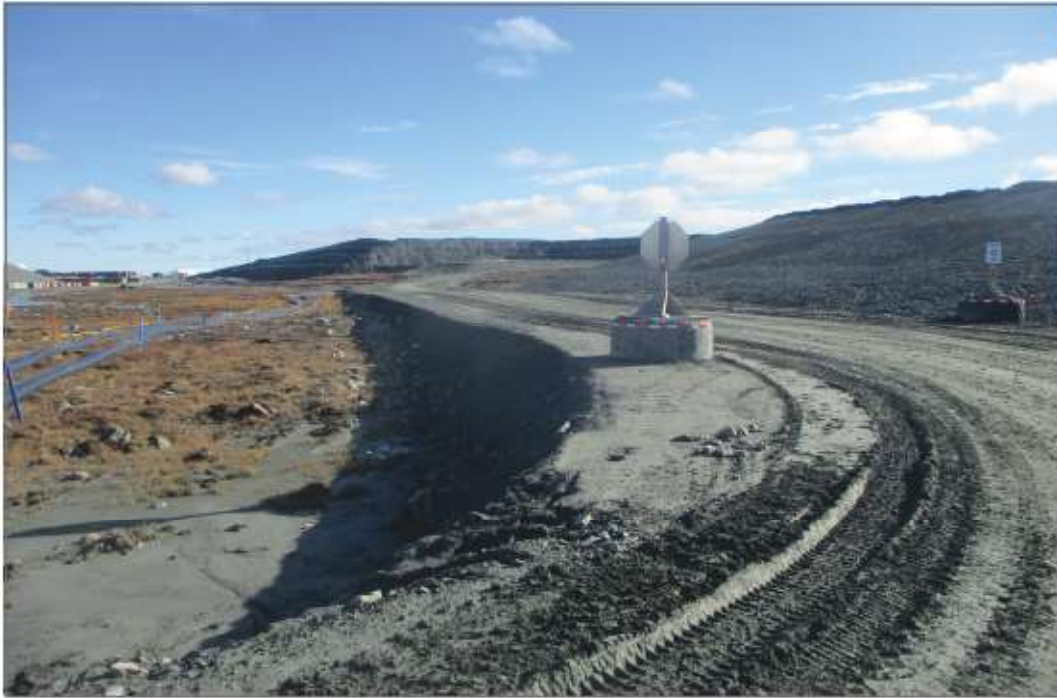
Photo 1: Site Roads—Road to landfill adjacent the TSF.
