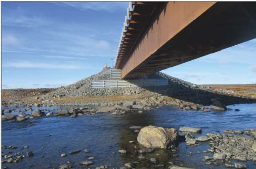
Photo 10: Meliadine River Bridge South Abutment
