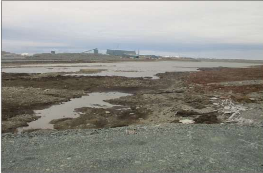
Photo 3: Dike D-CP1 - Upstream area of CP1, water levels well managed.
