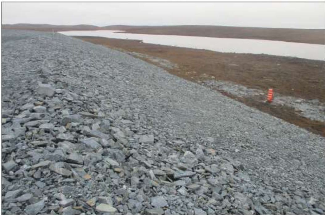
Photo 8: Berm CP2—Downstream crest of berm looking north.
