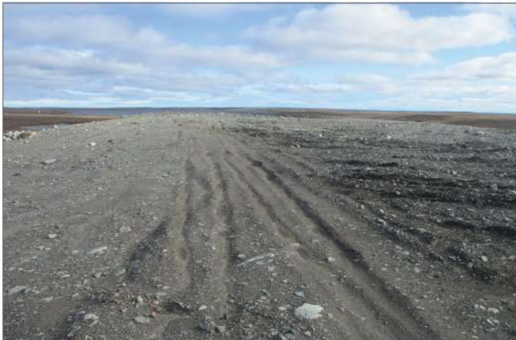
Photo 4: Wesmeg Esker—Access, looking northwest.
