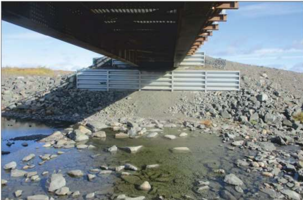
Photo 3: Char River Bridge—North abutment
