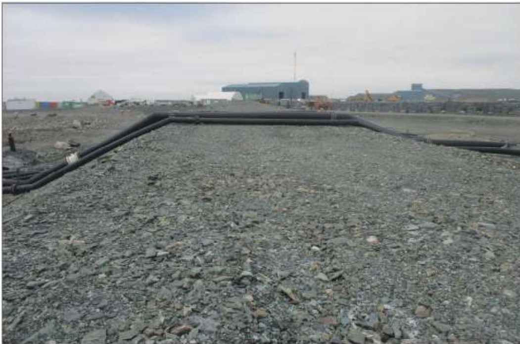
Photo 16: Dike D-CP1 - Multiple pipelines crossing D-CP1 at west abutment.
