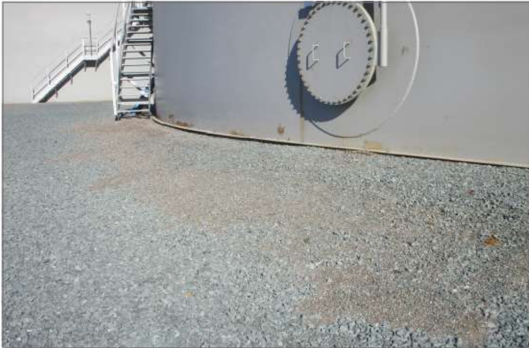
Photo 14: ITIVIA Tankfarm—Perimeter of tank base on pedestal.
