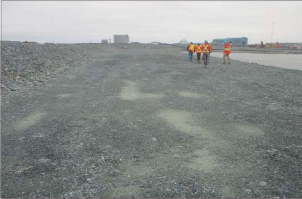
Photo 9: Dike D-CP1 - Upstream crest in good condition.
