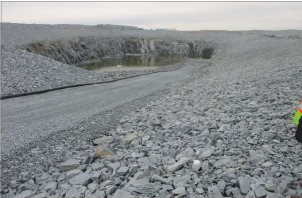
Photo 11: Pond CP2 - Access ramp, looking north.
