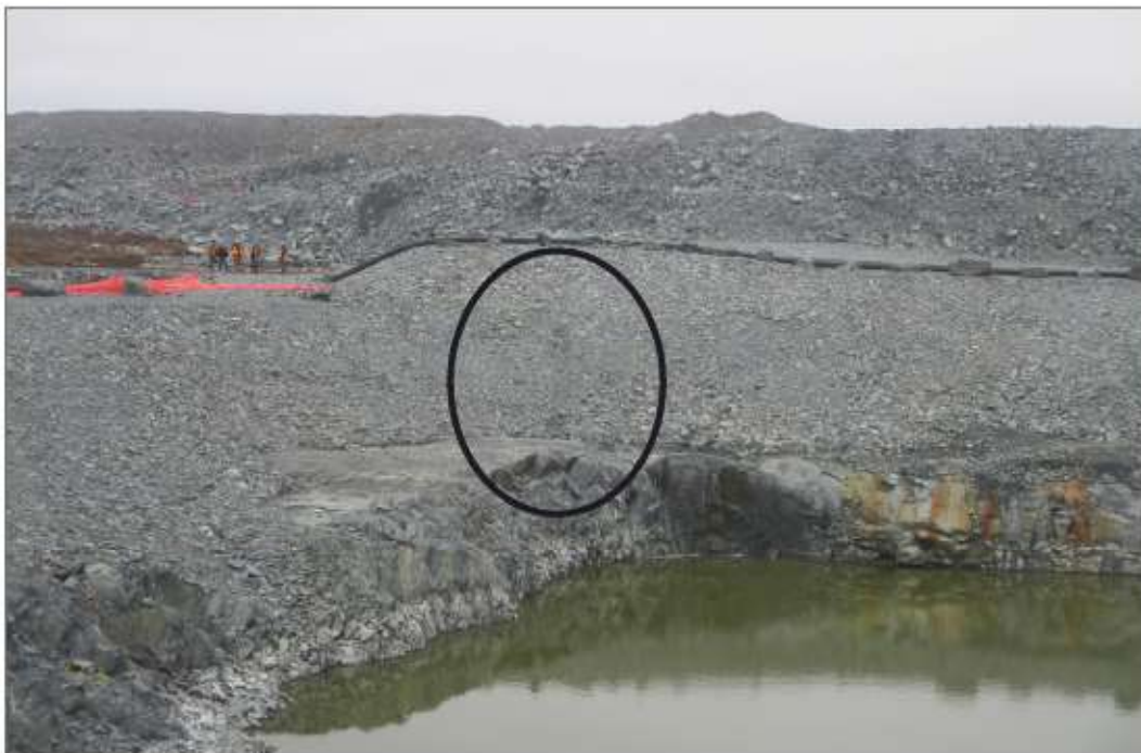
Photo 4: Pond CP6—South side of pond, WRSF3 above pond, water inflow on bedrock surface in southeast corner of pond, deformed ROM, indication of subsurface flow.
