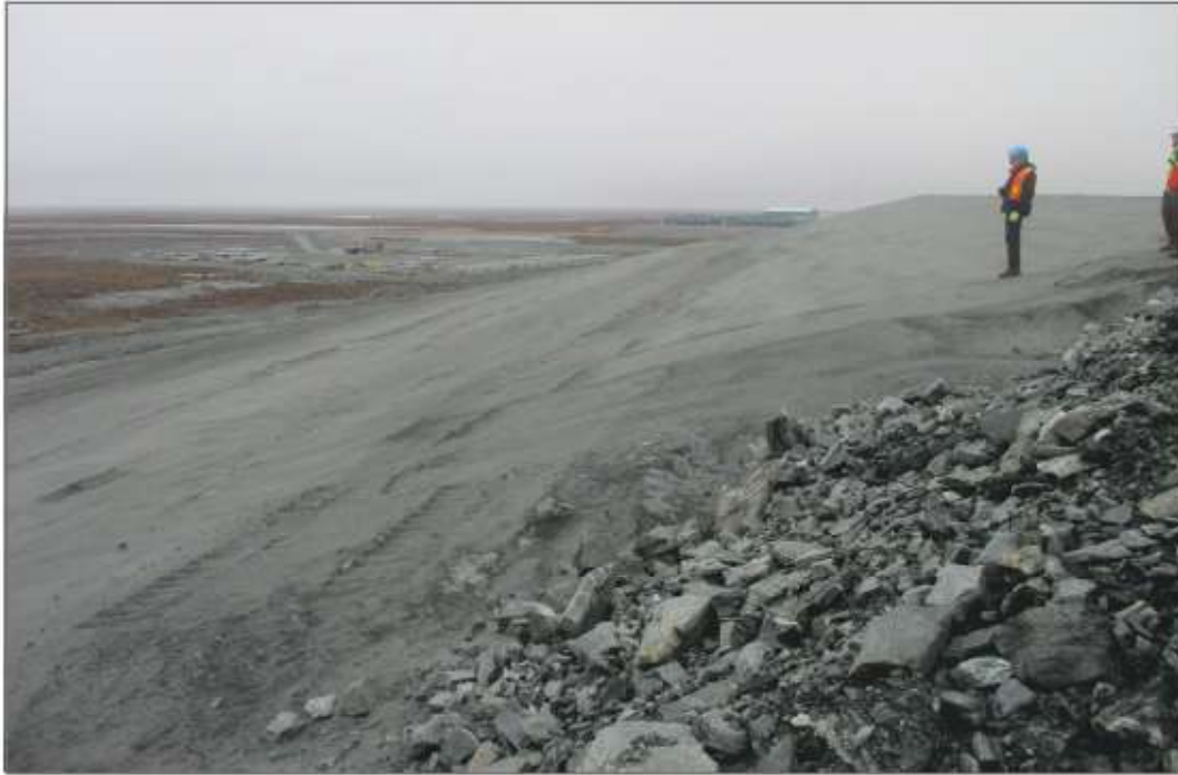
Photo 7: TSF - Slope between Cell 1 and future Cell 2.
