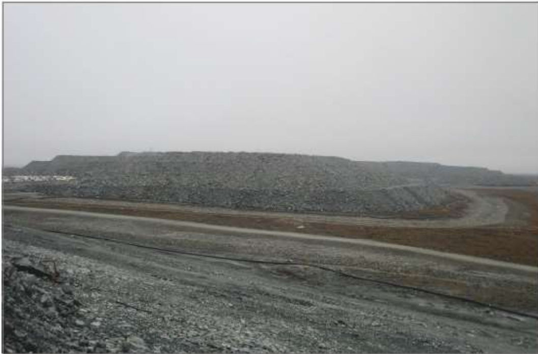
Photo 4: WRSF1—North side of WRSF, viewed from TSF.
