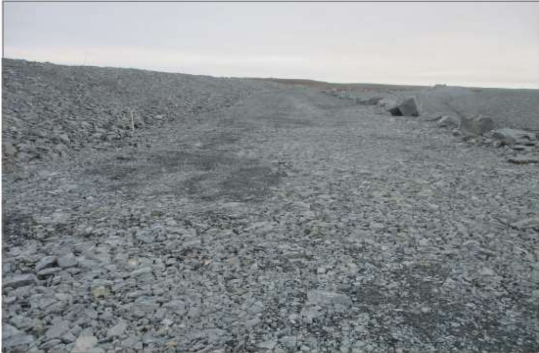
Photo 5: Pond CP2—Rockfill covering original ground between CP2 and berm.
