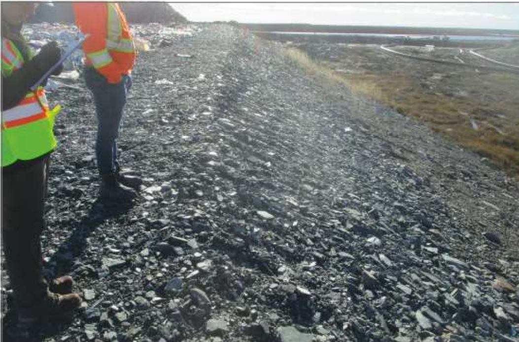
Photo 14: Landfill - WRSF1 Landfill—Northwest berm—some revegetation.
