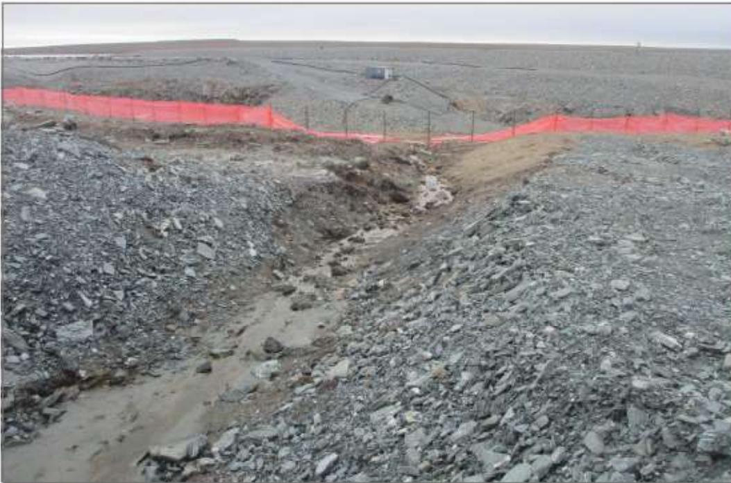
Photo 6: Pond CP3 - Constructed runoff channel into pond from north end of TSF drainage, located on east side of pond.
