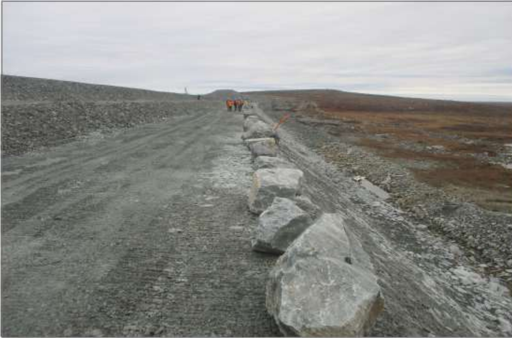
Photo 7: Dike D-CP1 - Downstream crest of toe berm constructed in fall of 2021.
