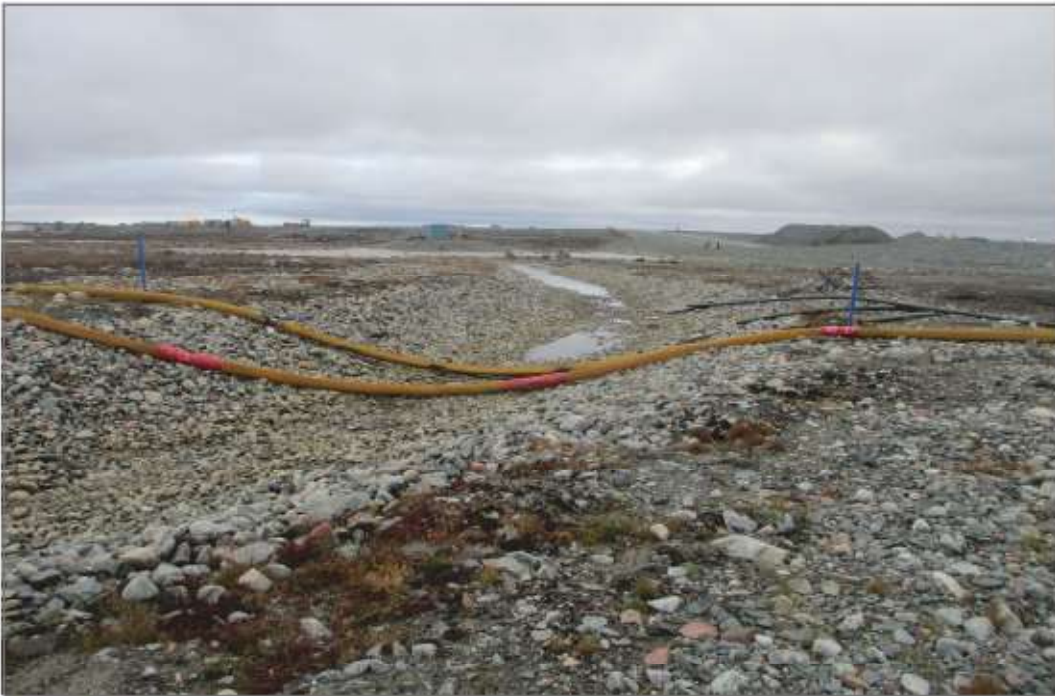
Photo 34: Channel 5—Lower reach, outlet into CP5, looking northeast.
