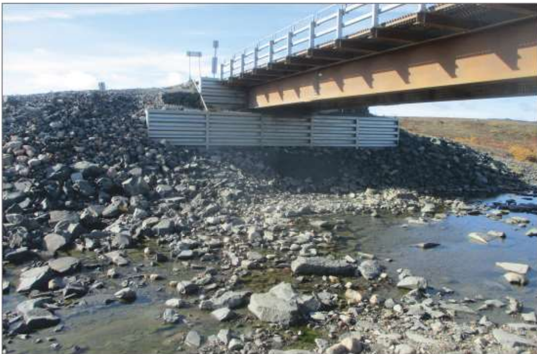
Photo 4: Char River Bridge—South Abutment
