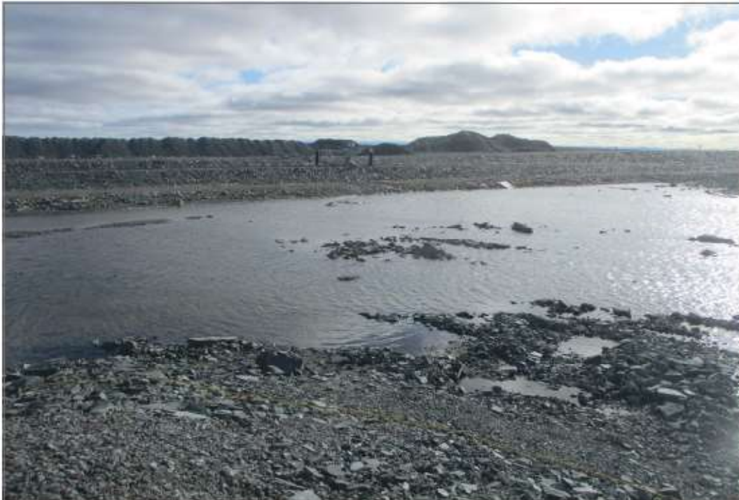
Photo 3: D-CP5 Dike - Looking towards upstream embankment from Jetty.
