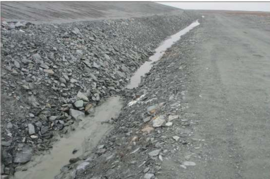
Photo 12: TSF - Swale along toe of north embankment directed to CP3.
