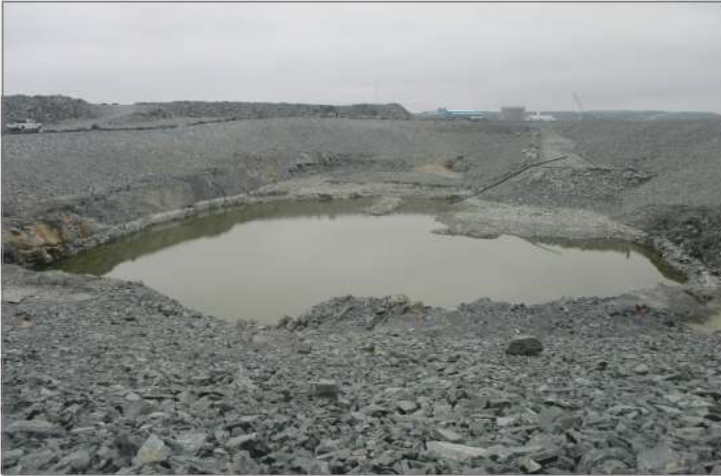
Photo 9: Pond CP6 - Embankments of CP6 showing no significant deformation.
