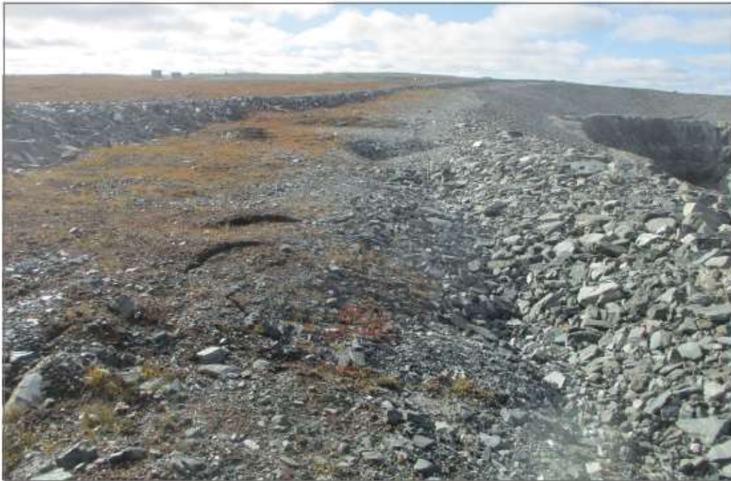
Photo 10: SP4 Saline Pond—Looking west General subsidence between overburden and rock-fill cover.
