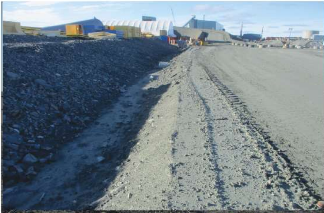
Photo 2: Site Roads—Drainage swale and road to ore stockpile.
