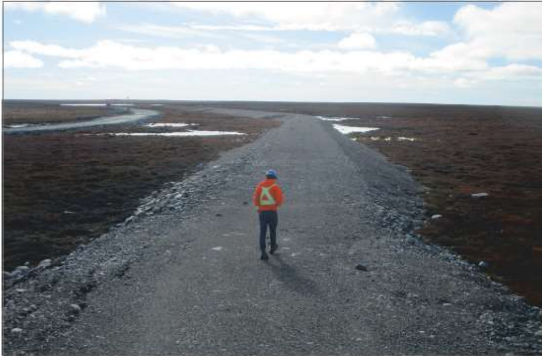
Photo 47: Berm 2—East abutment.
