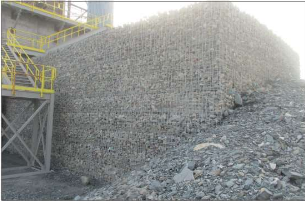
Photo 5: Crusher Pad—MSE Wall on the northwest corner.
