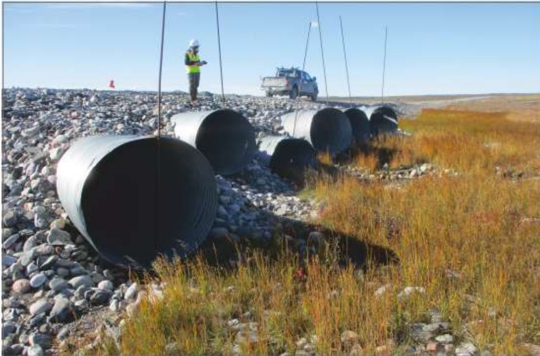
Photo 5: Culvert C10 (C11 on sign).
