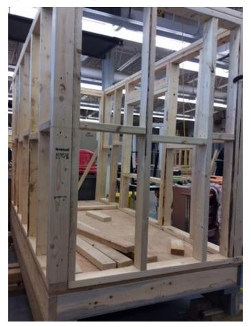
Figure 36. Cabin being built by carpentry students of Jonah Amitnaaq Secondary school with recycled wood.
