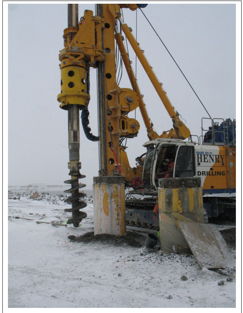
Photo No. 2 Auger for caisson clean-out
