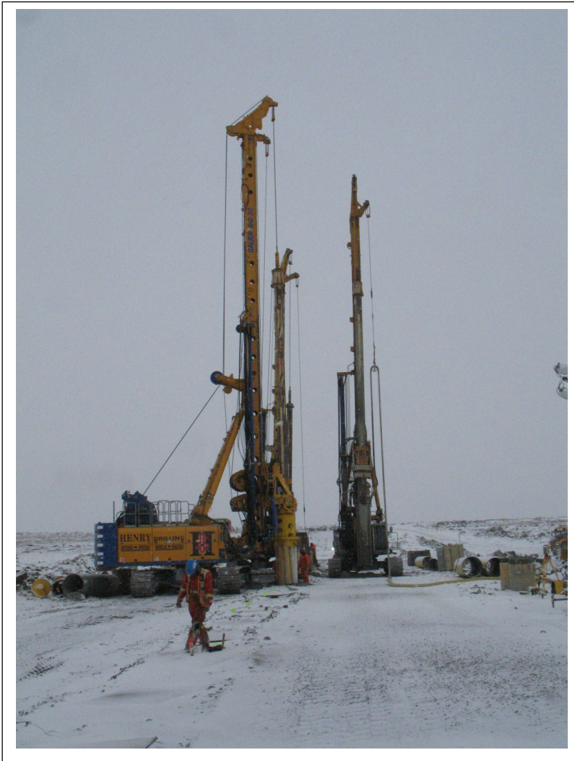
Photo No. 1 Caisson drilling machines on Whale Tail Dike
