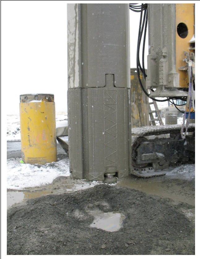
Photo No. 3 Rock socket drill
