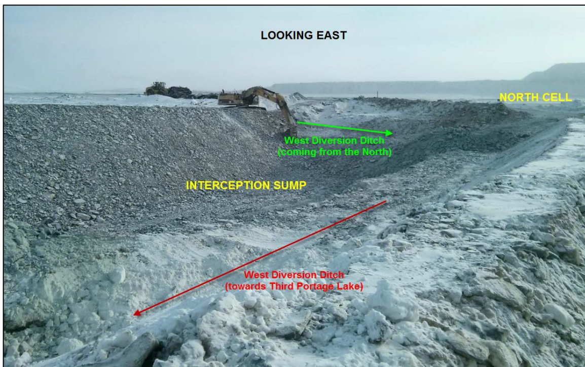
Figure 2-5: North Cell West Diversion ditch interception sump
