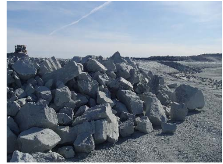
NCIS-120 (2018-07-26), looking NE from Sta. 1+830/-27 m (approx.). View of an accumulation of boulders on the upstream slope of the NCIS.
