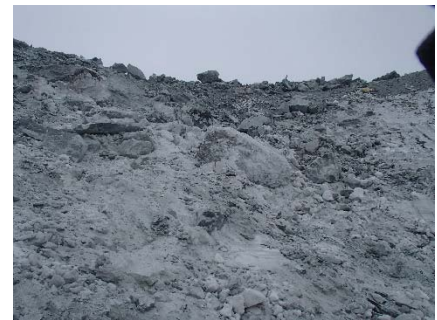
CD-1804 (2018-04-28), looking S from Sta. 40+790/-2 m. Presence of oversize boulders on the existing slope at the junction between SD5 and Central Dike.
