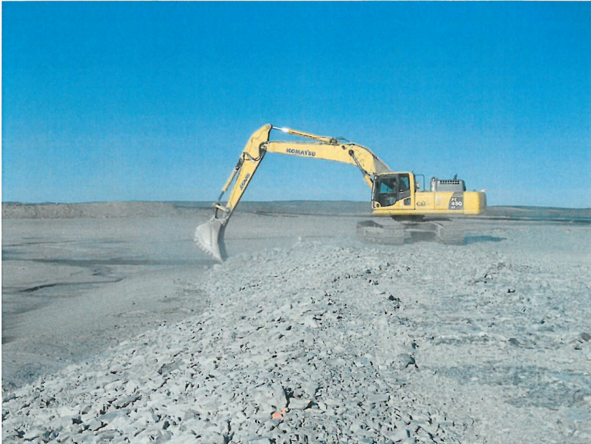
Photograph NCIS-094: From Sta 1+125/-109 m (approx.), looking SW. Profiling of the upstream slope (3H:1V) from El. 150 to 152 m with an excavator from Sta. 1+135 m to 1+100 m
