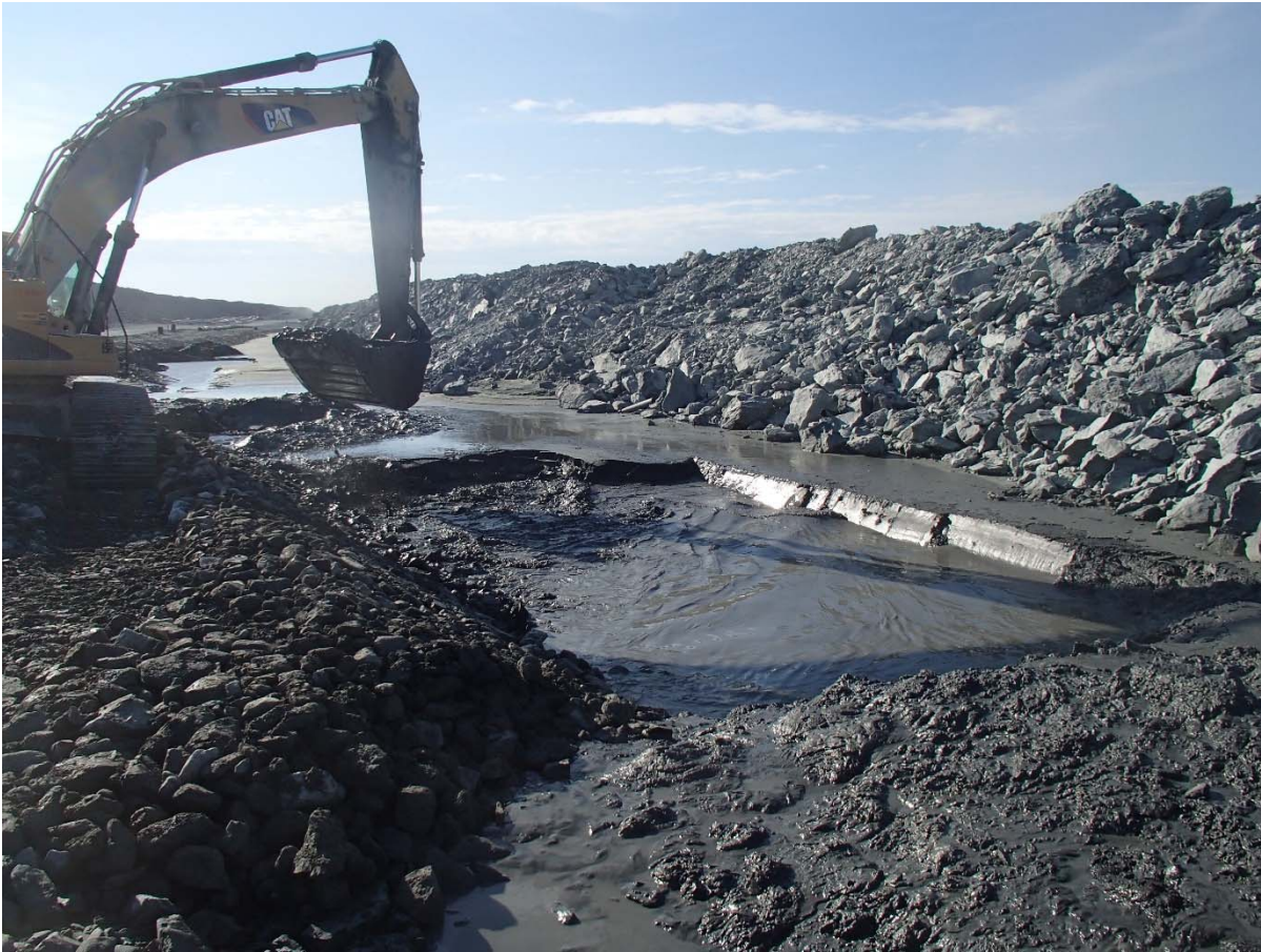
Photograph NCIS-123: From Sta. 3+340/+33 m (approx.), looking S. Excavation of a 1 m (approx.) deep sump (south sump) in the tailings with an excavator from Sta. 3+345 m to 3+365 m (o.s. +24 to +32 m). The bottom of the excavation was frozen.
