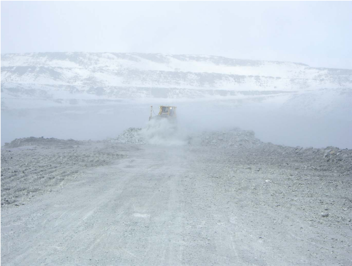
Photograph CD-1800: From Sta. 0+500/-14 m looking N. Placement of a 2 m thick (approx.) lift of intermediate volcanic (IV) rockfill from El. 143 m to El. 145 m from 0+435 to 0+535m (o.s. -28 to -18 m).
