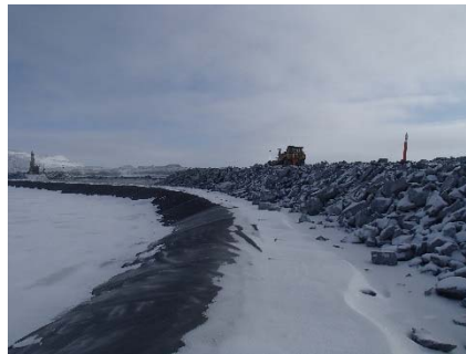
CD-1818 (2018-05-03), looking NE from Sta. 40+770/-25 m. Placement of a 2 m thick (approx.) lift of intermediate volcanic (IV) rockfill from El. 143 m to El. 145 m from approx. Sta. 0+980 m to 0+880 m (o.s. -28 to -11 m).
