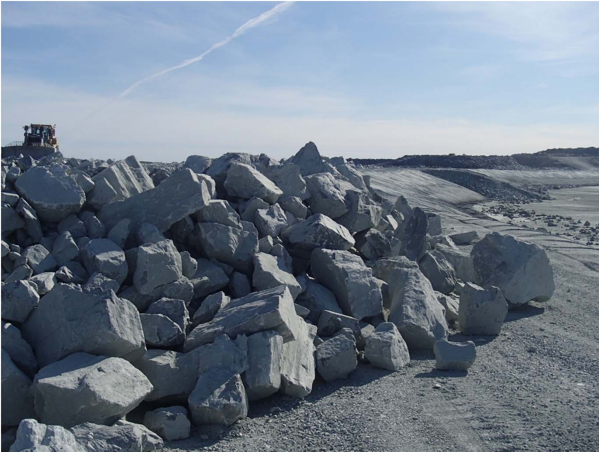
Photograph NCIS-120: From Sta. 1+830/-27 m (approx.), looking NE. View of an accumulation of boulders on the upstream slope of the NCIS.
