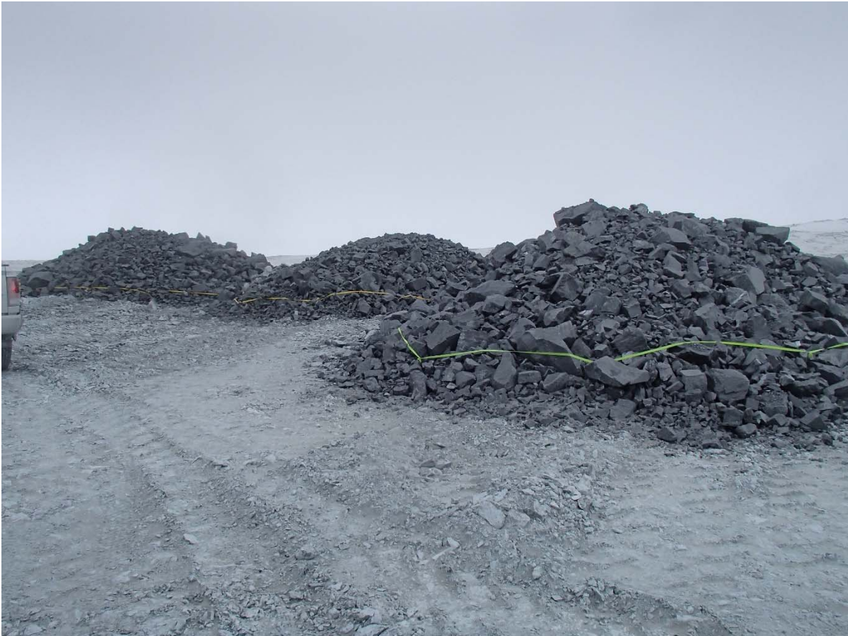
Photograph NCIS-016: From Sta. 1+750 m (approx.), looking SE. View of the Iron Formation rockfill (PAG material) piles on the North Cell Internal Structure.
