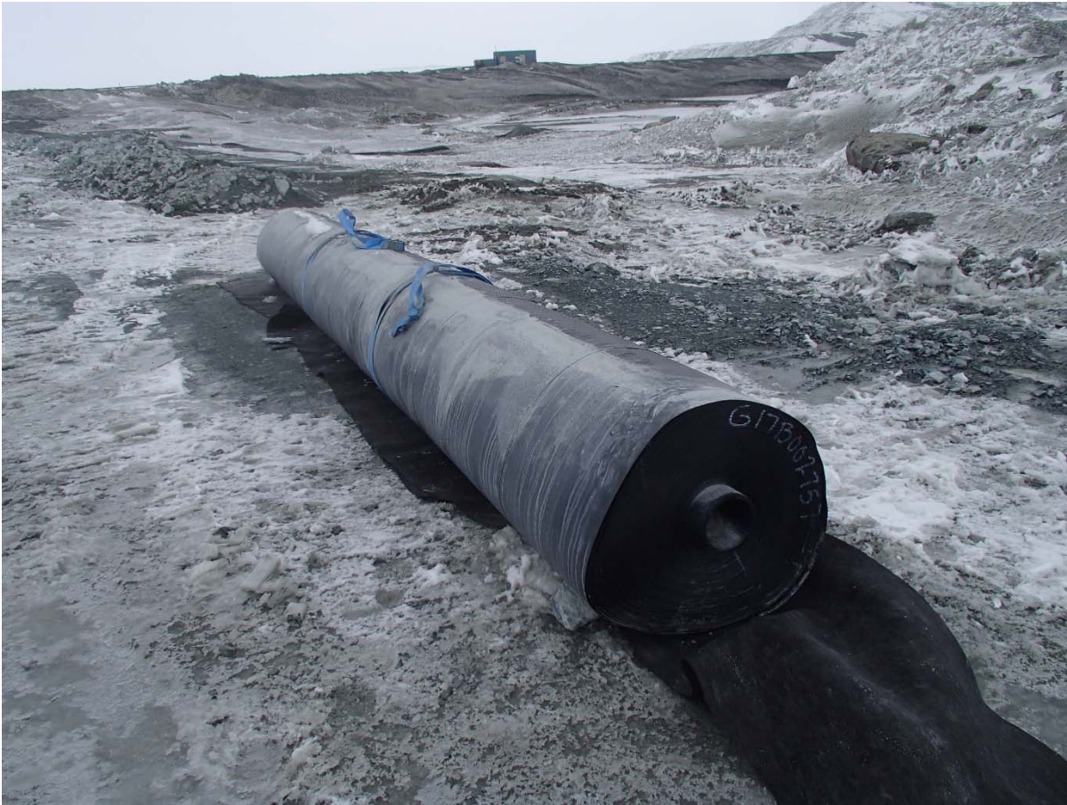
Photograph SD3-303: From Sta. 20+780/-15 m, looking N. View of an LLDPE liner roll stored on geotextile.
