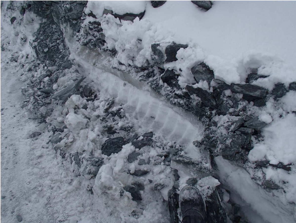
Photograph NCIS-004: View of the scraped upstream side of the UM rockfill lift at El. 152 m further to the north: the snow layer is only observed at the toe and is approximately 0.5 m thick.
