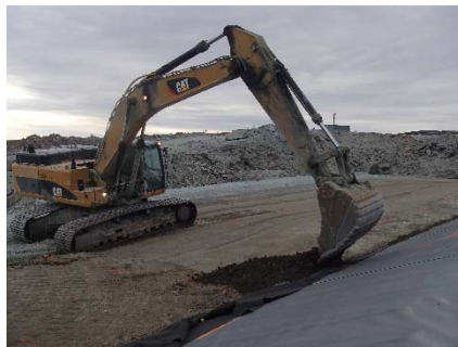
SD3-347 (2018-07-18), looking W from Sta. 20+640/-41 m. Placement of a third 0.5 m thick lift of fine UM rockfill (0-500 mm) upstream of the low quality till (0-150mm) from El. 143 m to 143.5 m from Sta. 20+688 m to 20+619 m.
