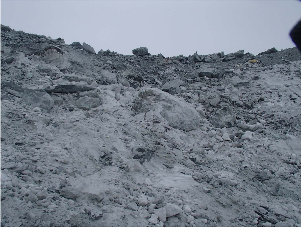
Photograph CD-1804: From Sta. 40+790/-2 m looking S. Presence of oversize boulders on the existing slope at the junction between SD5 and Central Dike.
