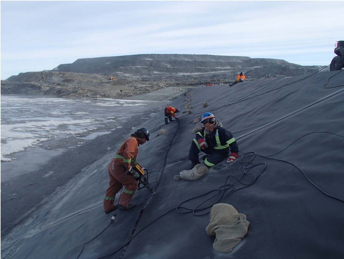
Photograph CD-1890: From Sta. 0+310/-26 m, looking N. View of the extrusion welding.
