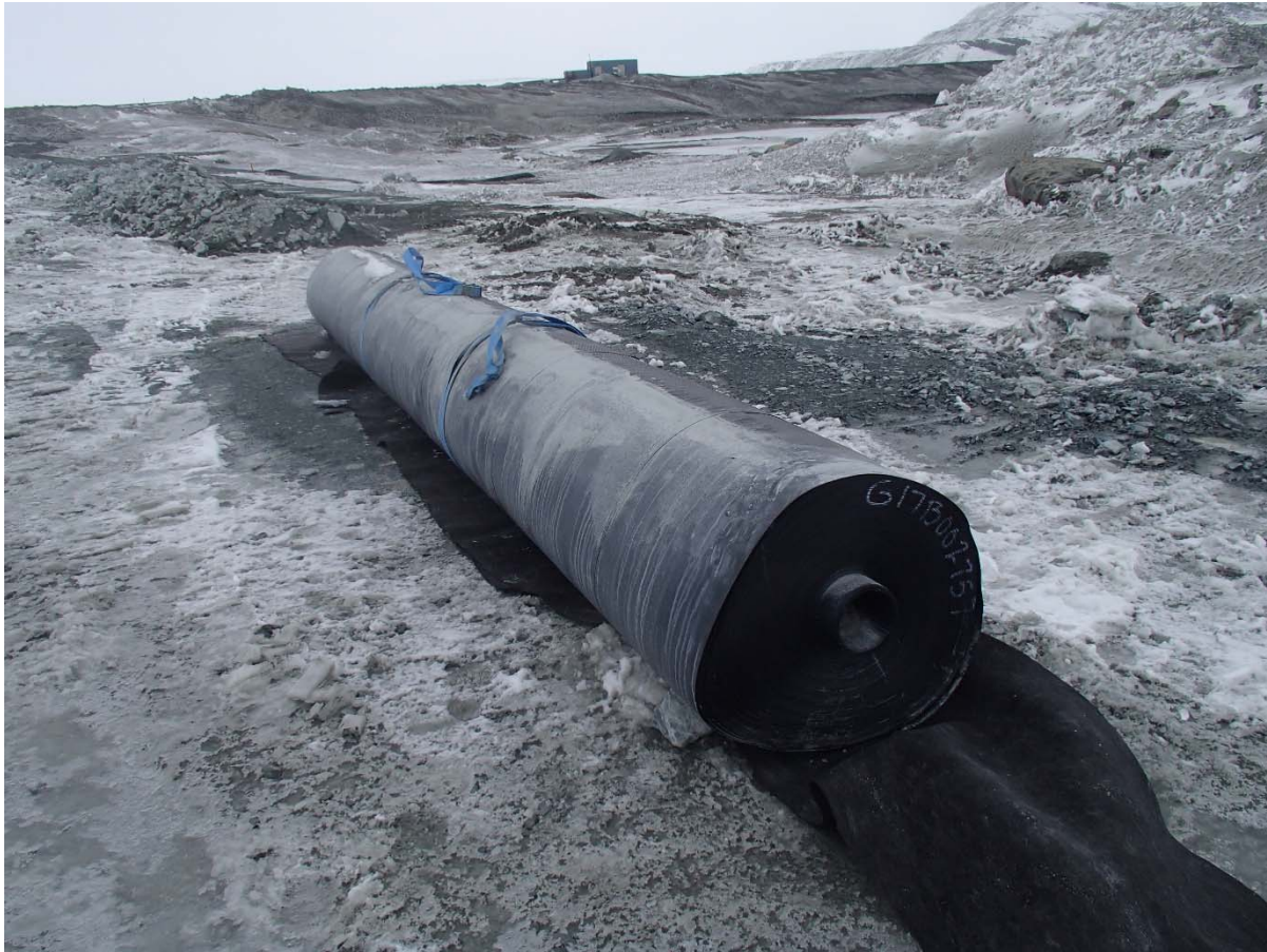
Photograph SD3-303: From Sta. 20+780/-15 m, looking N. View of a LLDPE liner roll stored on geotextile.
