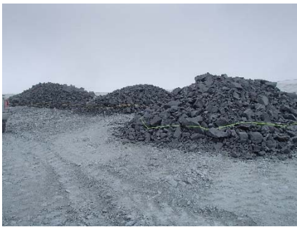
NCIS-016 (2018-05-23), looking SE from Sta. 1+750 m. View of the Iron Formation rockfill (PAG material) piles on the North Cell Internal Structure.
