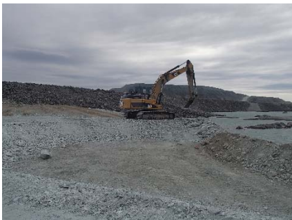
SD3-347 (2018-07-18), looking W from Sta. 20+640/-41 m. Placement of a third 0.5 m thick lift of fine UM rockfill (0-500 mm) upstream of the low quality till (0-150mm) from El. 143 m to 143.5 m from Sta. 20+688 m to 20+619 m.
