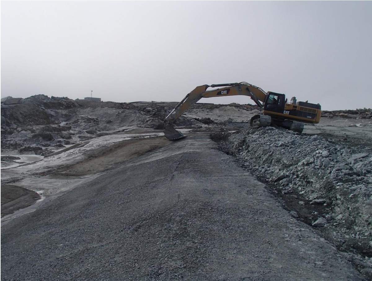
Photograph SD3-306: From Sta. 20+780/-25 m, looking S. Correction of the surface of the fine filter in the upstream slope and the top of the first class compacted sieved till layer with an excavator from Sta. 20+803 m to 20+793 m.
