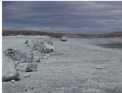
NCIS-032 (2018-06-20), looking N from Sta. 1+400/-24 m. Compaction of the 2 m lift (approx.) of ultramafic (UM) rockfill at El. 152 m with a 10-tonne smooth-drum compactor with vibration (6 passes) between the haul truck traffic lane and the upstream slope from Sta. 1+660 to 1+380 m (o.s. -45 to -24 m).
