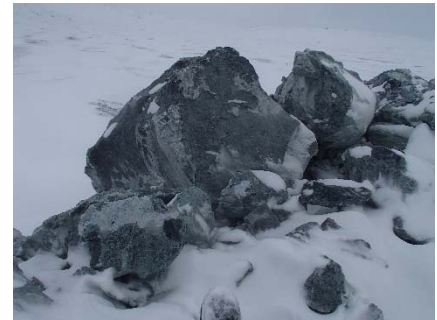
NCIS-006 (2018-05-19). View of oversized boulders on the UM rockfill lift at El. 152 m.
