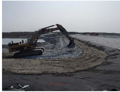
SD3-325 (2018-07-10), looking S from Sta. 20+610/-43 m. Placement of a first 0.5 m thick lift of fine rockfill (0-500 mm) upstream of the low quality till from El. 142 m to 142.5 m from Sta. 20+610 m to 20+760 m.
