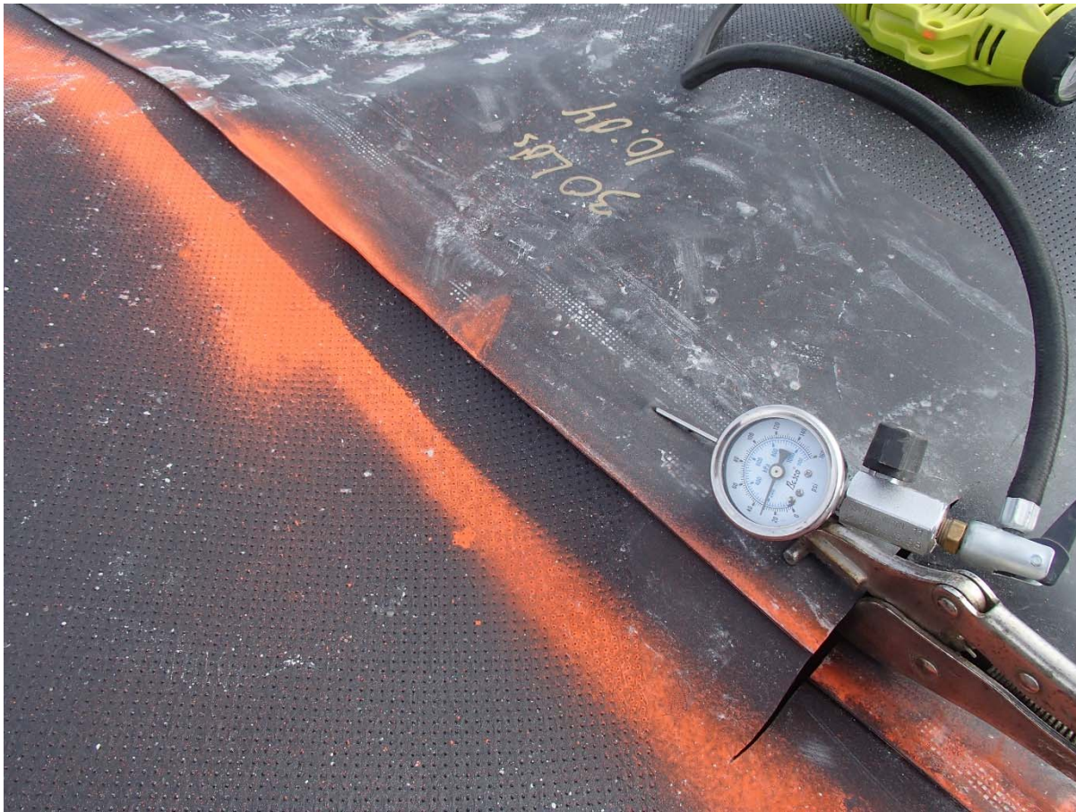
Photograph CD-1862: From Sta. 40+960/-24 m. View of an air channel test.
