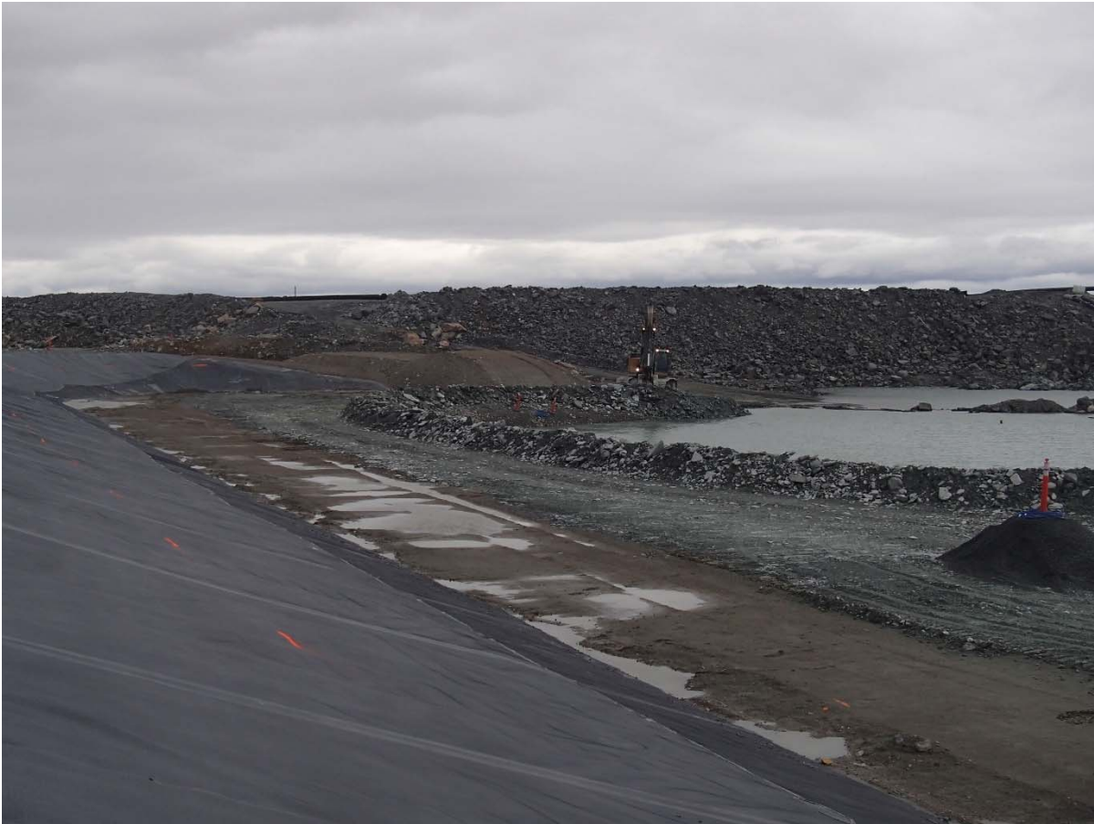
Photograph SD3-319: From Sta. 20+740/-31 m, looking SE. Placement of IV rockfill in the water up to El. 142 m with an excavator from Sta. 20+730 m to 20+610 m, at the bottom of the upstream slope of SD3 to widen the rockfill layer and allow access to the erosion protection.
