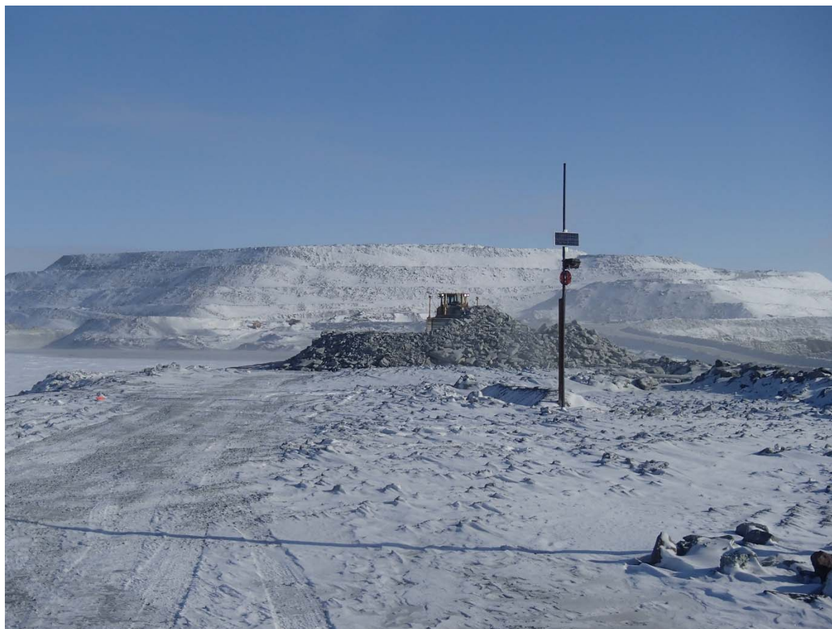
Photograph CD-1809: From Sta. 0+870/-16 m looking N. Placement a 2 m thick (approx.) lift of intermediate volcanic (IV) rockfill from El. 143 m to El. 145 m from approx. Sta. 0+760 to 0+835 m (o.s. -28 to 3 m).
