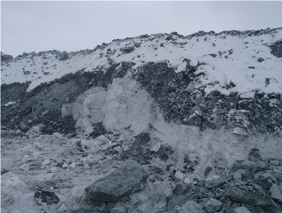
Photograph NCIS-002: View of the scraped upstream side of the UM rockfill lift at El. 152 m: a thick layer of snow (1.5 m) underlies the rockfill.
