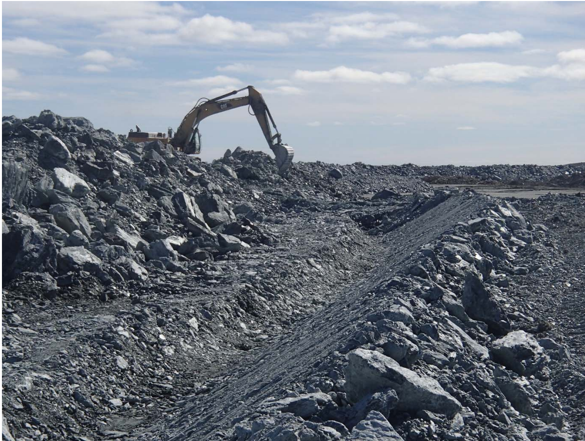
Photograph NCIS-130: From Sta. 1+446/+16 m (approx.), looking S. Excavation of a 0.8 m (approx.) deep, 1 m wide shallow ditch in the rockfill capping with an excavator from Sta. 1+380 m to 1+300 m.
