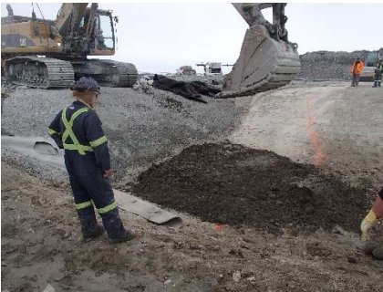
SD3-312 (2018-06-08), looking W from Sta. 20+610/-48 m. Placement of a 0.15 m thick lift of compacted sieved till from Sta. 20+596.4 m to 20+601.6 m (o.s. -42.6 to -46.3 m) to fill the depression in the compacted sieved till layer.
