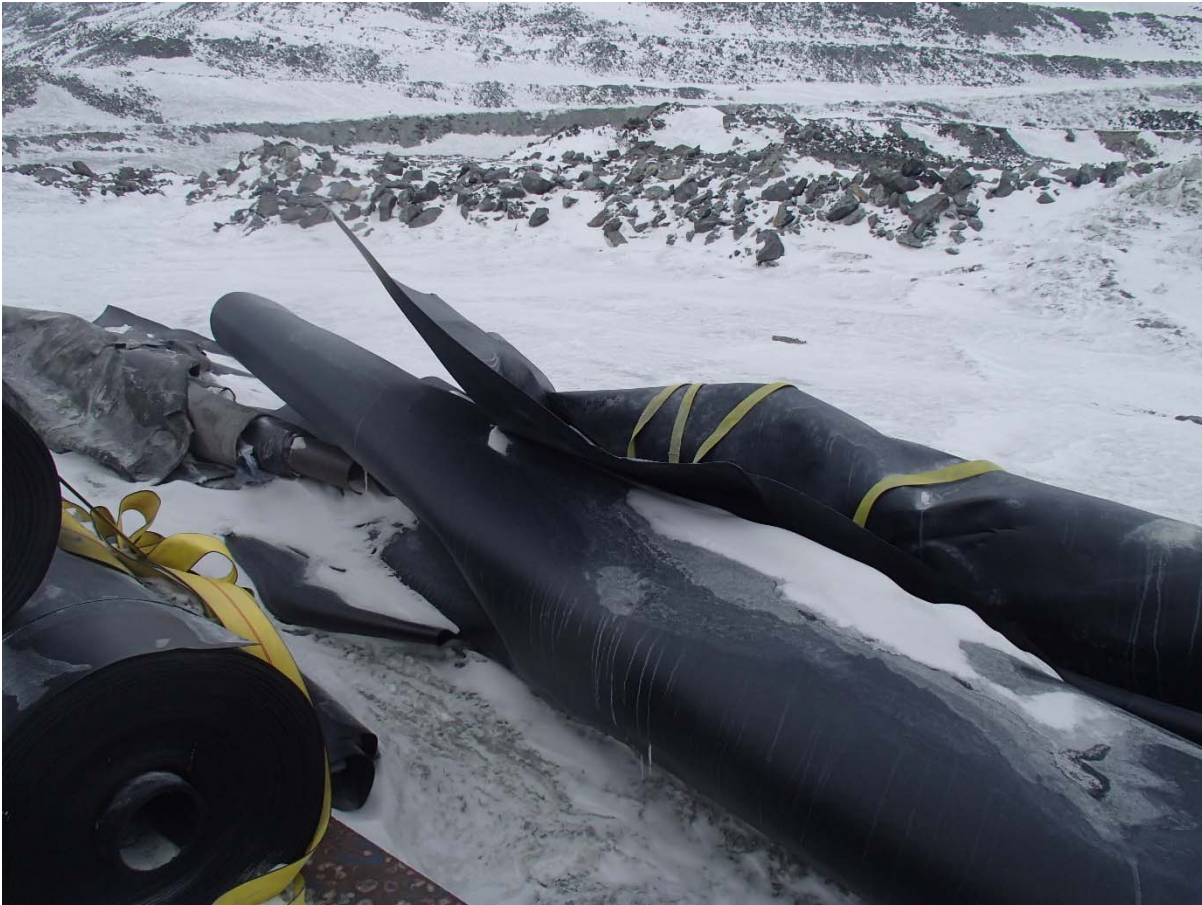
Photograph from the LLDPE storage site: View of old rolls stored on the ground.
