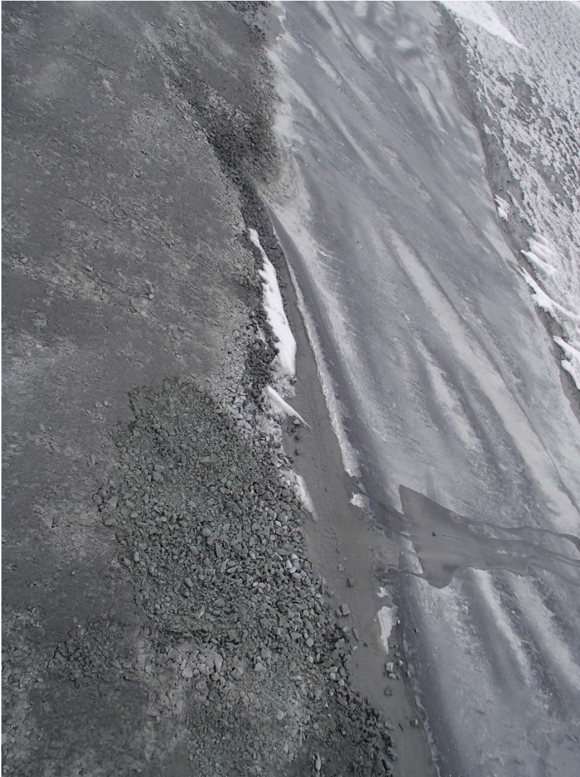
Photograph CD-1858: From Sta. 0+970/-45 m, looking S. View of the bottom of the fine filter upstream slope. Some material is missing to achieve a smooth slope.
