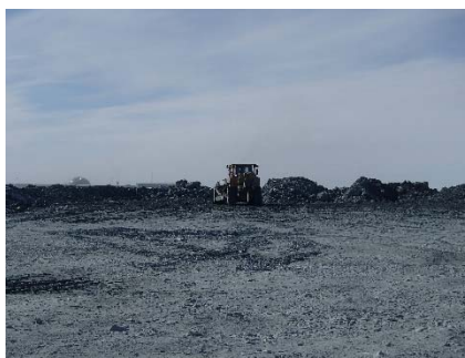
NCIS-026 (2018-06-06), looking S from Sta. 1+440/+2 m. Placement of a 2 m thick (approx.) lift of UM rockfill from El. 150 m to El. 152 m (approx.) with a dozer from Sta. 1+390 m to 1+365 m (+10 m to -29 m).
