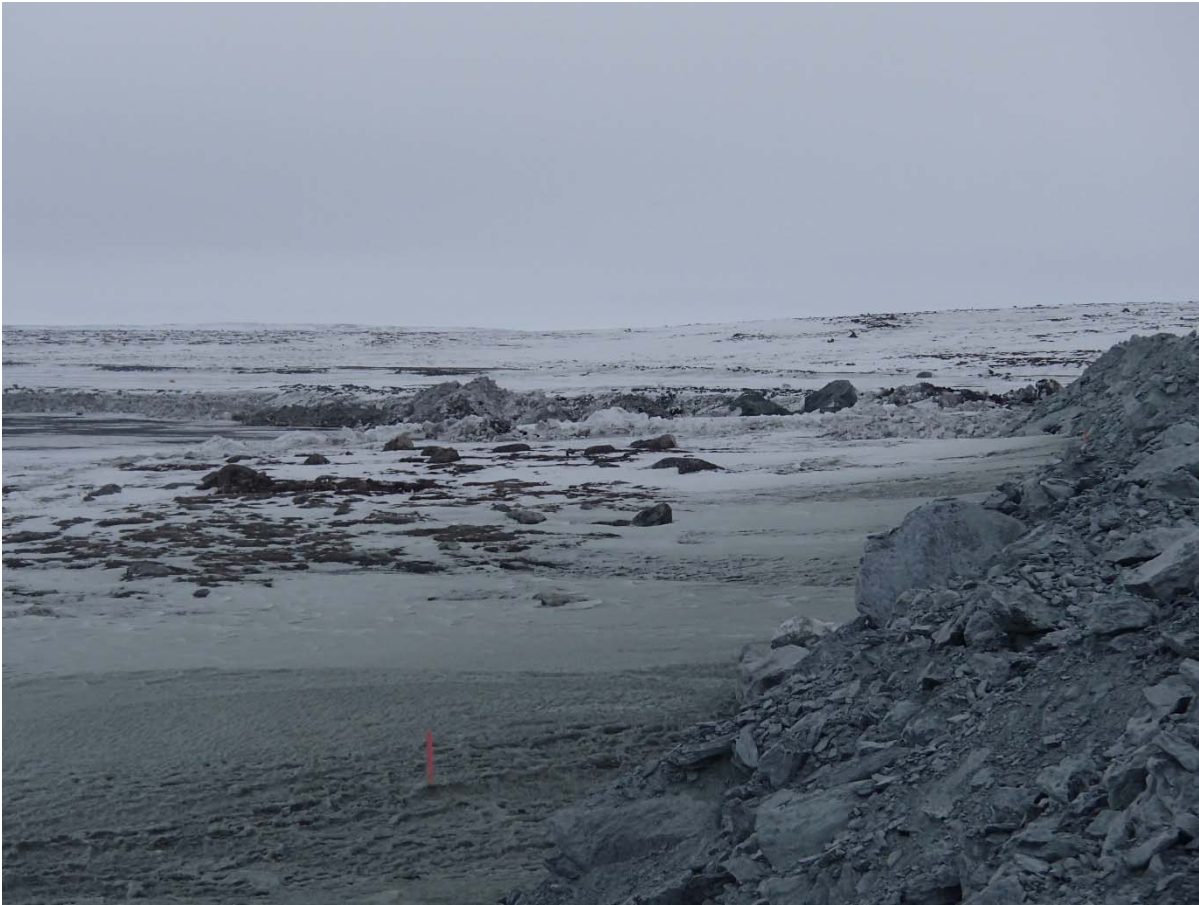
Photograph NCIS-014: From Sta. 1+900 m (approx.), looking SE. View of the natural soil on which the 2015 capping is built.
