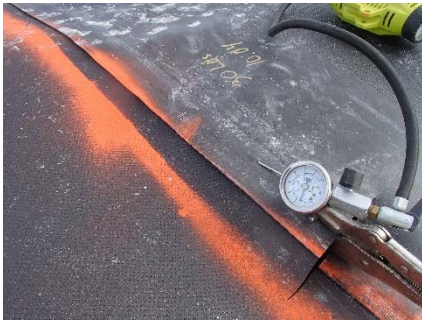
CD-1862 (2018-05-24), looking from Sta. 40+960/-24 m. View of an air channel test.
