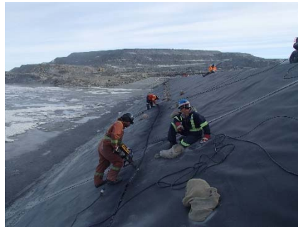
CD-1890 (2018-06-05), looking N from Sta. 0+310/-26 m. View of the extrusion welding.
