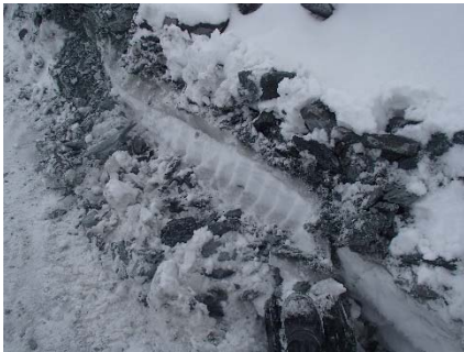
NCIS-004 (2018-05-19). View of the scraped upstream side of the UM rockfill lift at El. 152 m further to the north: the snow layer is only observed at the toe and is approximately 0.5 m thick.
