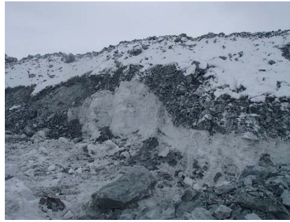
NCIS-002 (2018-05-19). View of the scraped upstream side of the UM rockfill lift at El. 152 m: a thick layer of snow (1.5 m) underlies the rockfill.
