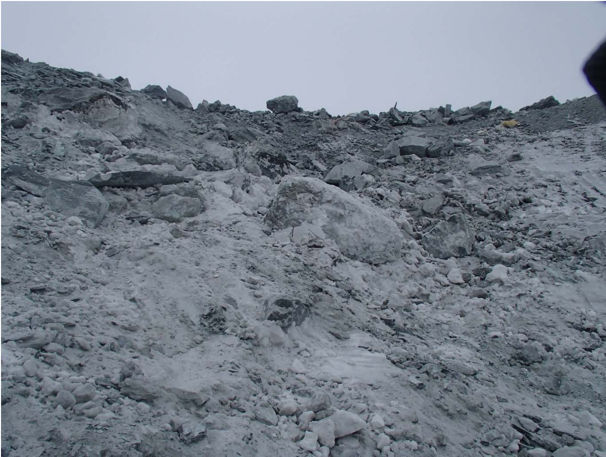
Photograph CD-1804: From Sta. 40+790/-2 m looking S. Presence of oversize boulders on the existing slope at the junction between SD5 and Central Dike.
