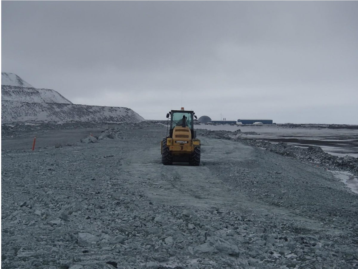
Photograph NCIS-022: From Sta. 2+245 m (approx.), looking SE. Compaction of the 2 m lift (approx.) of ultramafic (UM) rockfill at El. 152 m with a 10-tonne smooth-drum compactor with vibration (6 passes) between the haul truck traffic lane and the upstream slope from Sta. 2+625 to 1+625 m (o.s. unavailable).
