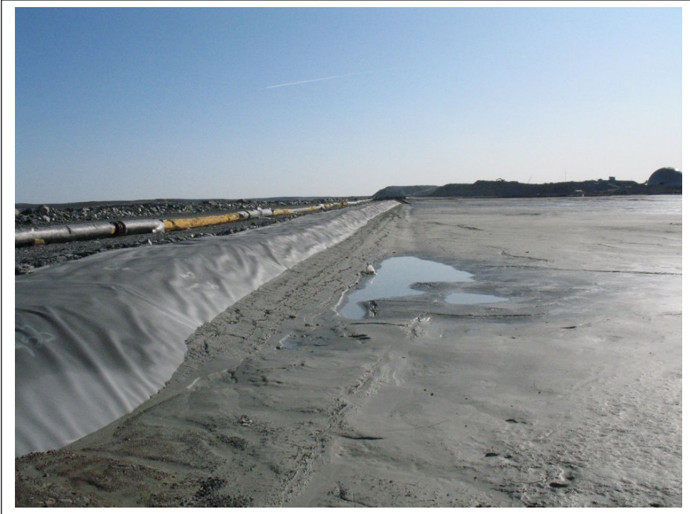
Photo No. 5 Tailings beach against Central Dike
