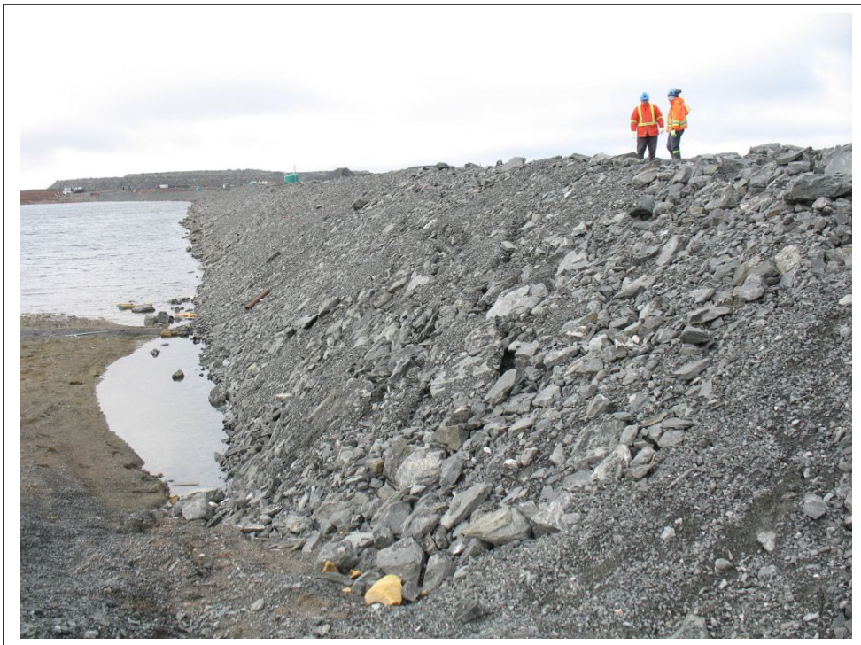
Photo #22 East abutment U/S slope
