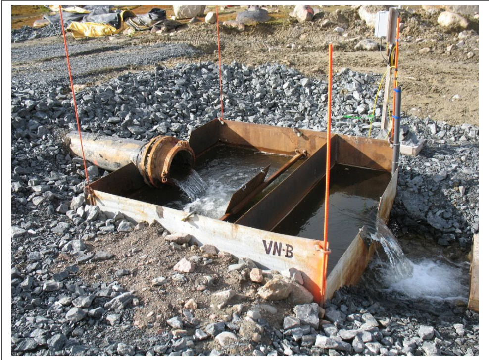
Photo #19 V-notch Weir B
