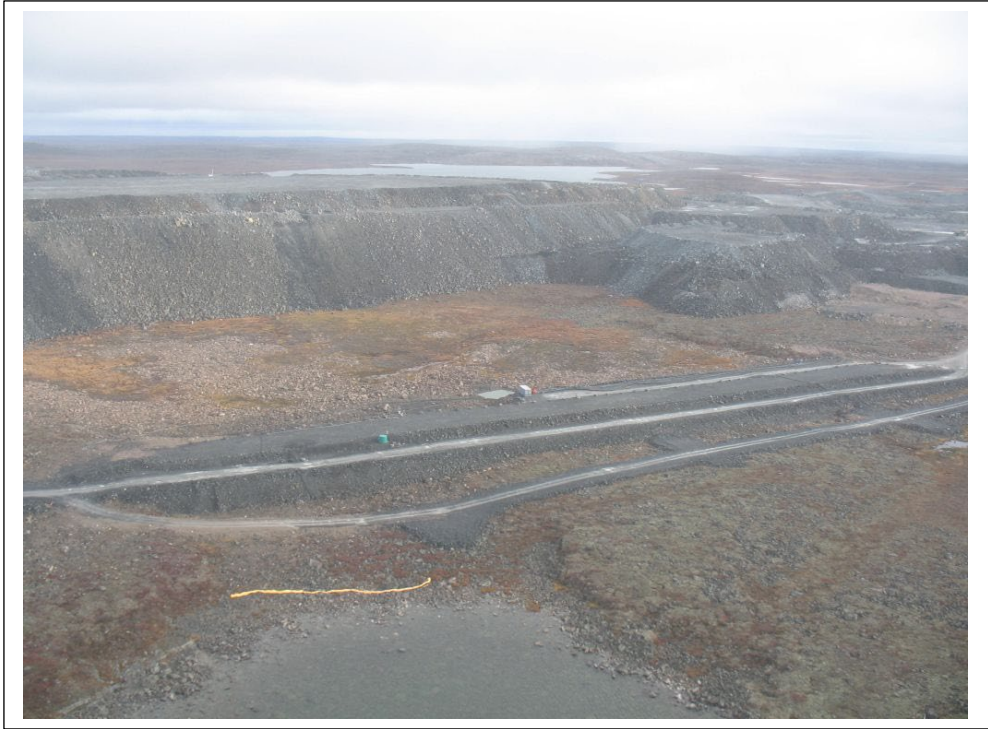
Photo #15 WRSF Dike
