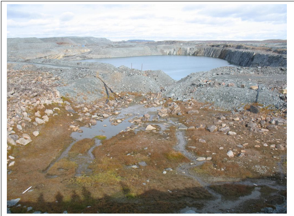
Photo #10 Seepage from Bay-Goose Dike
