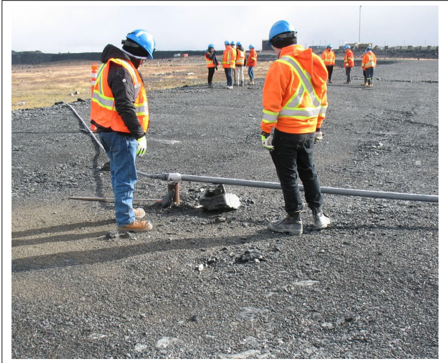
Photo #13 IVR Dike Crest
