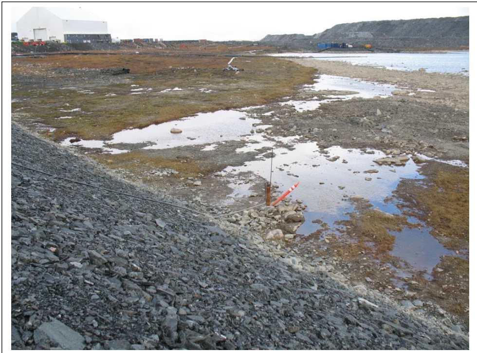
Photo #14 IVR Dike D/S toe
