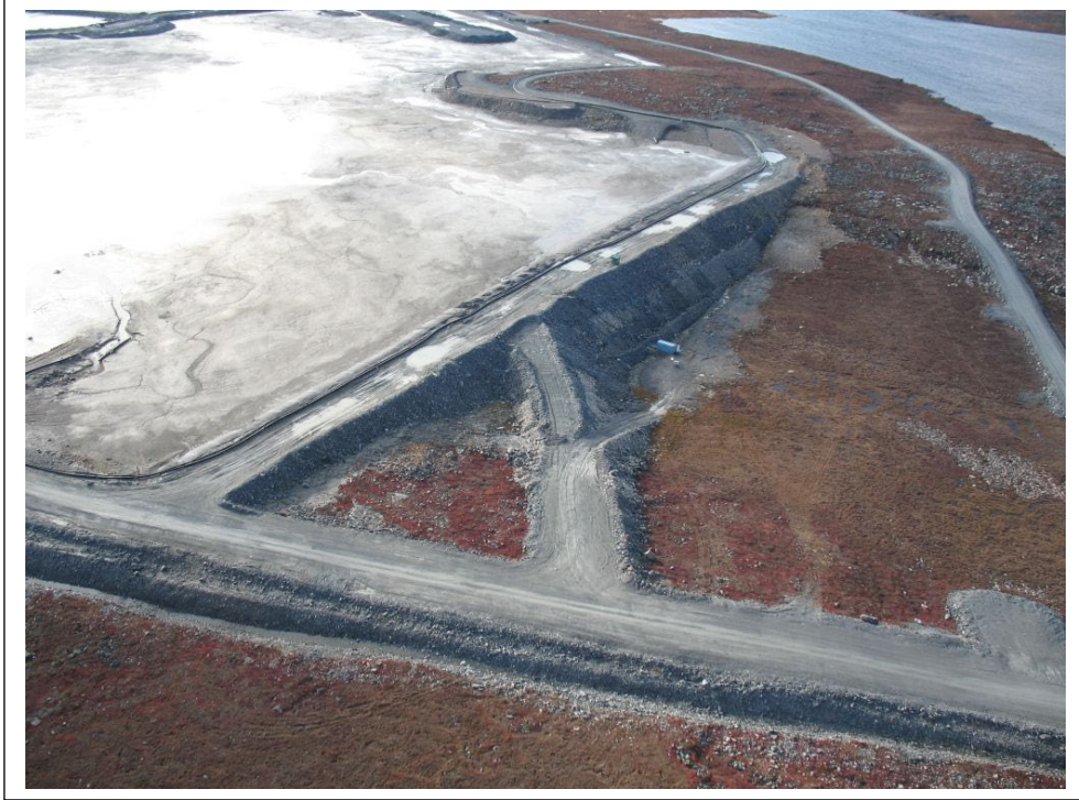
Photo #5 Saddle Dam SD-1
