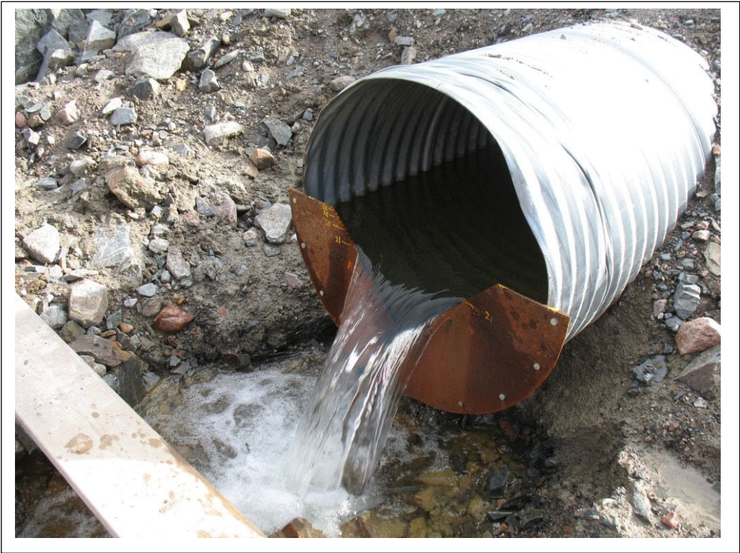
Photo #18 V-notch Weir A
