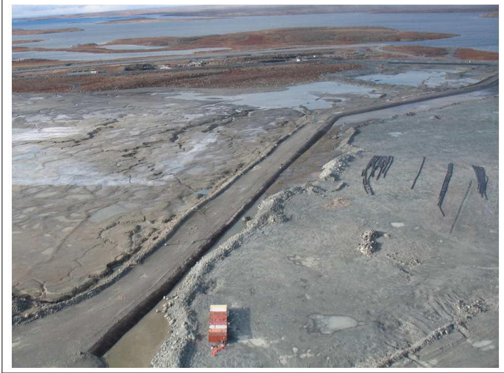
Photo #7 Stormwater Dike
