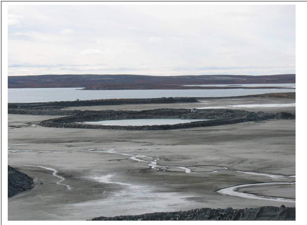
Photo #4 Reclaim sump in North Cell
