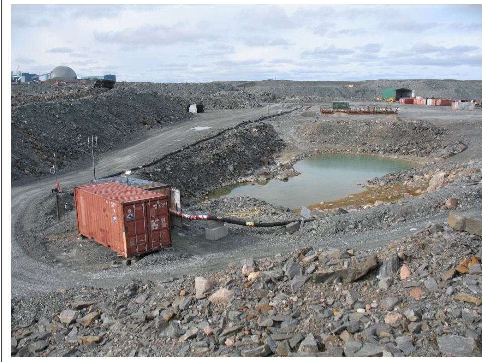
Photo #11 Pump installation at East Dike south channel
