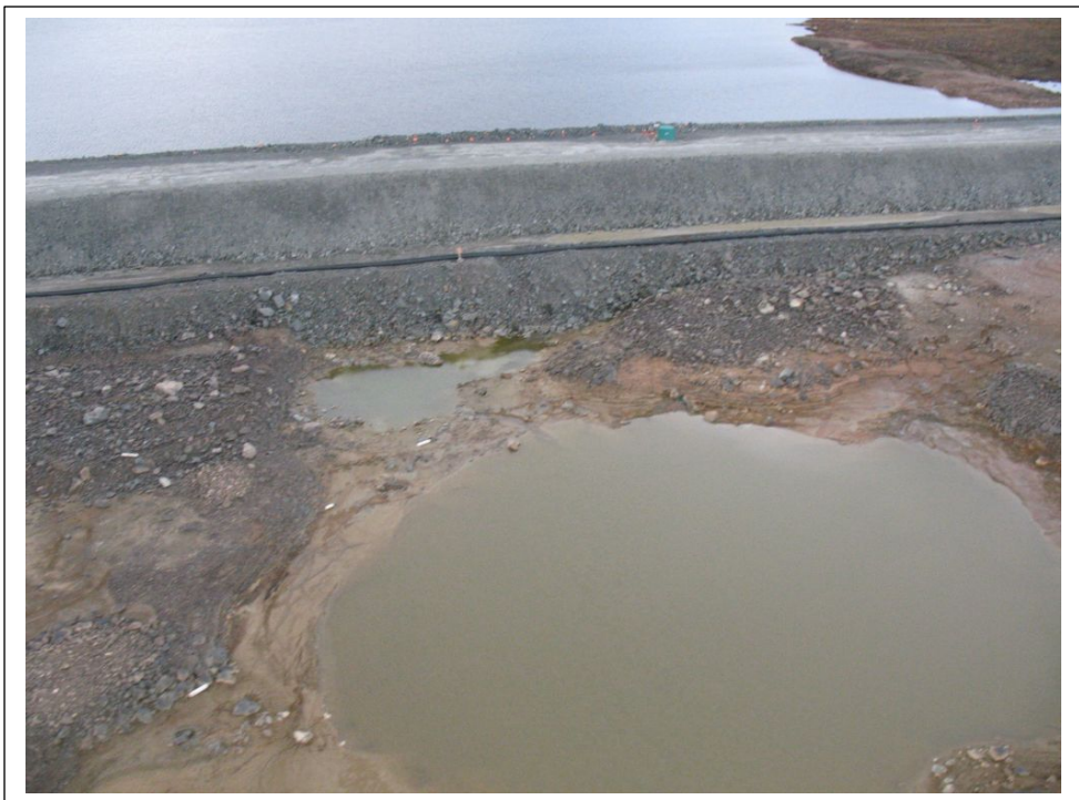
Photo No. 10 Western sector of Whale Tail Dike
