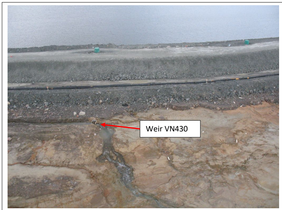
Photo No. 8 Central sector of Whale Tail Dike
