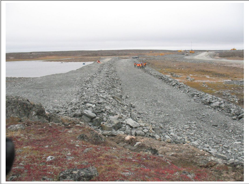
Photo No. 15 North East Dike from west abutment
