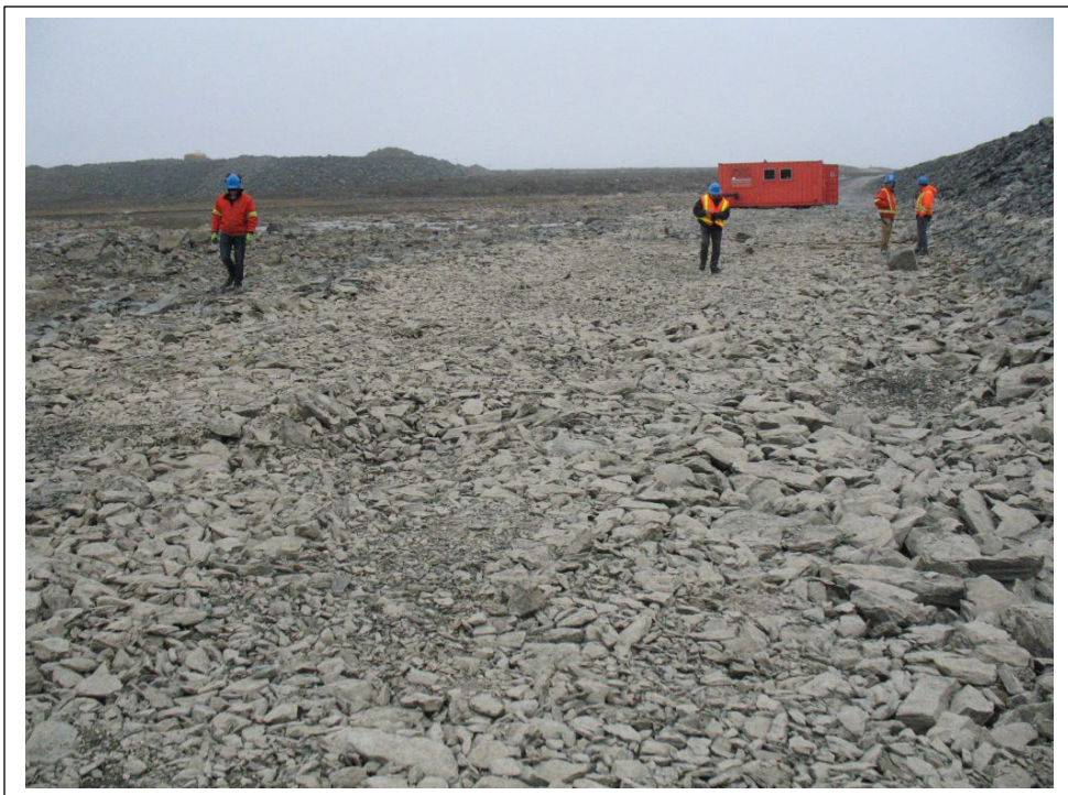
Photo No. 20 Upstream berm of WRSF Dike
