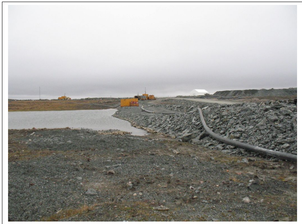
Photo No. 16 Pond upstream of eastern sector of North East Dike
