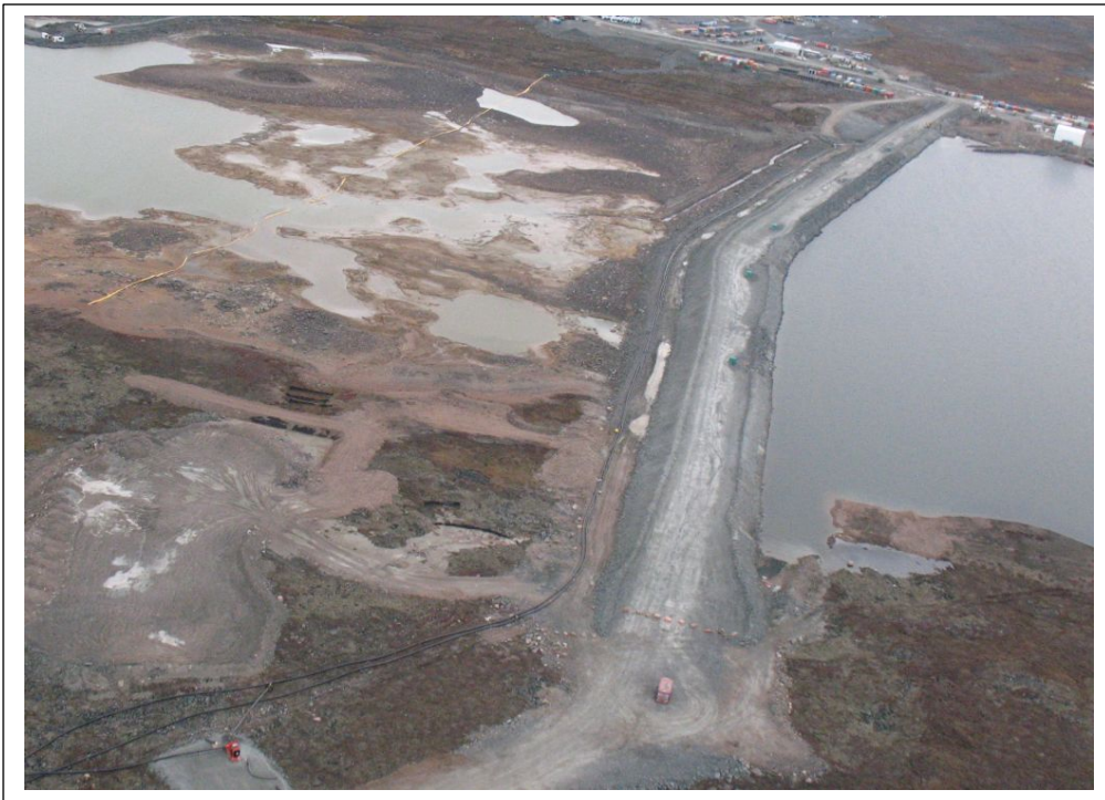
Photo No. 2 Whale Tail Dike viewed from the West (Increasing station)
