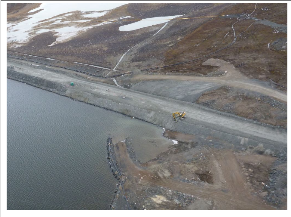
Photo No. 13 South Whale Tail Pond in vicinity of east abutment
