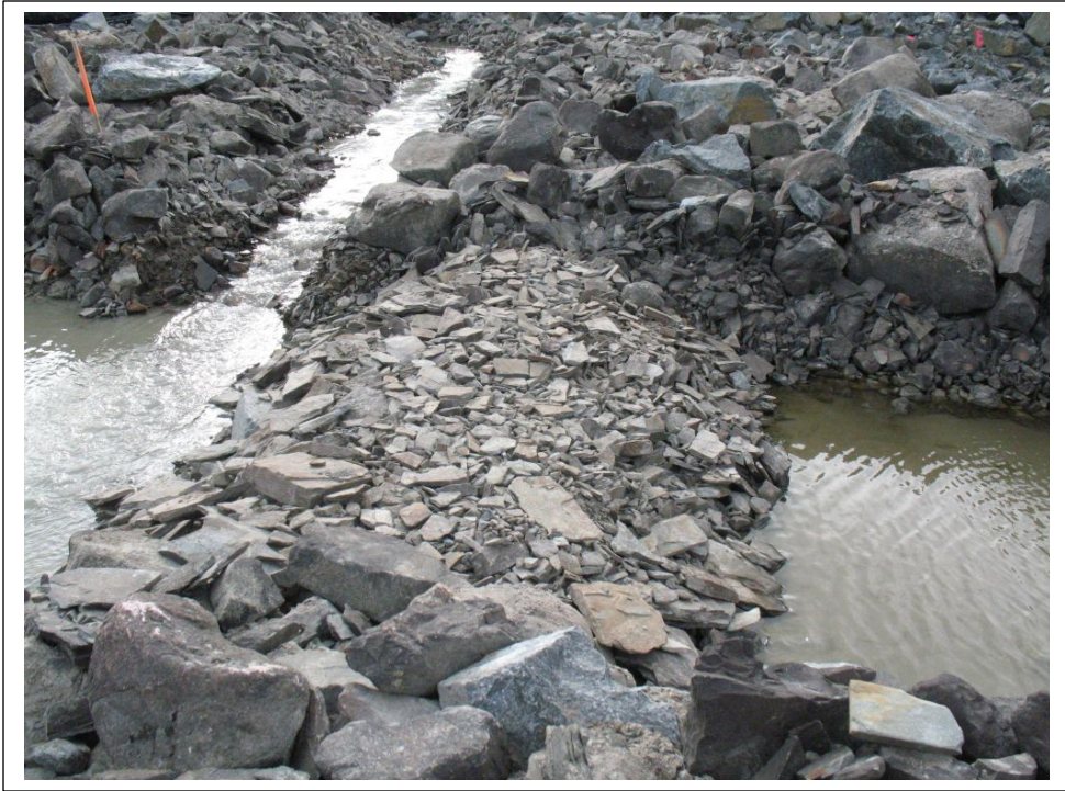
Photo No. 5 Dike to separate clean flow from turbid flow
