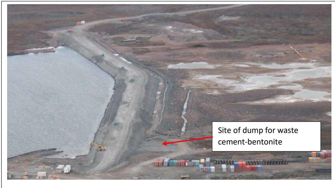
Photo No. 1 Whale Tail Dike viewed from the East (Decreasing station)
