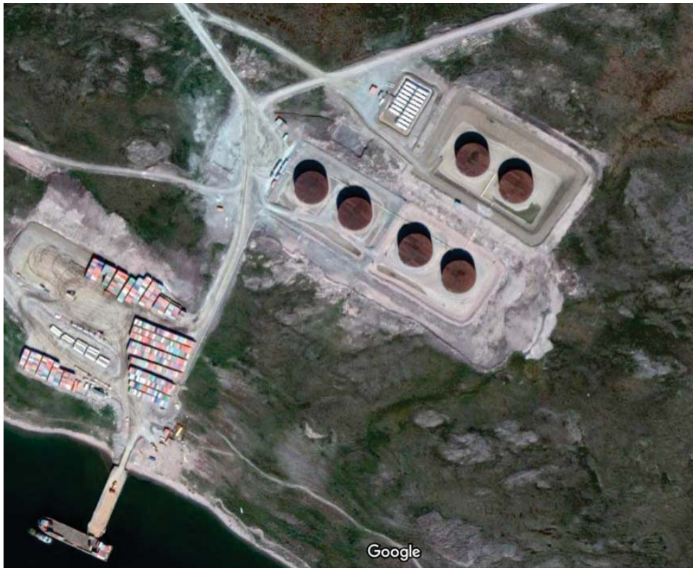
General site view before tank and containment construction
