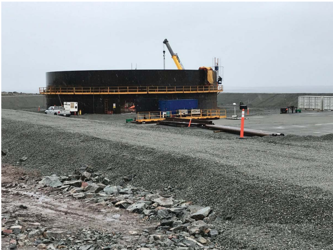
Tank wall welding
