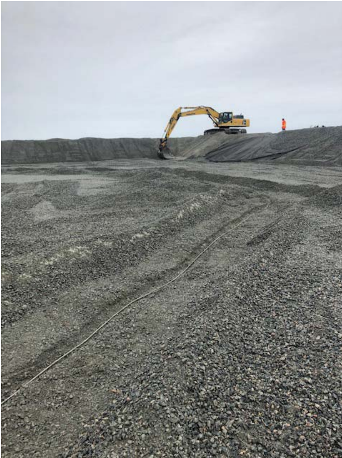
Pad and Berm construction
