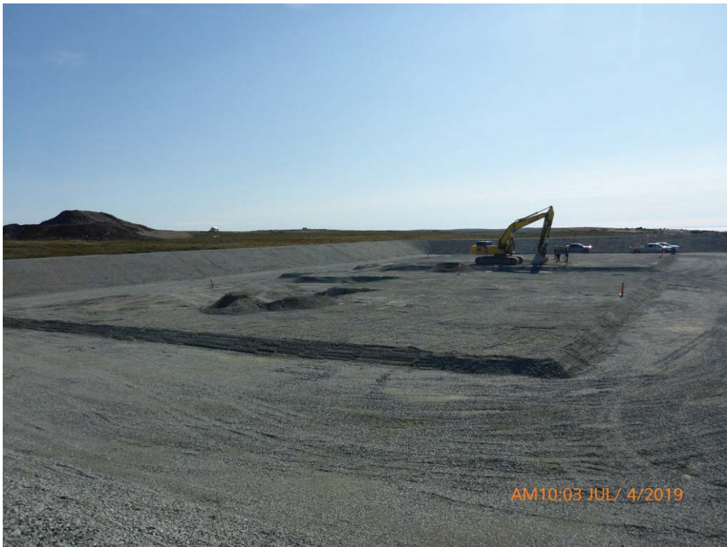
Tank pad construction
