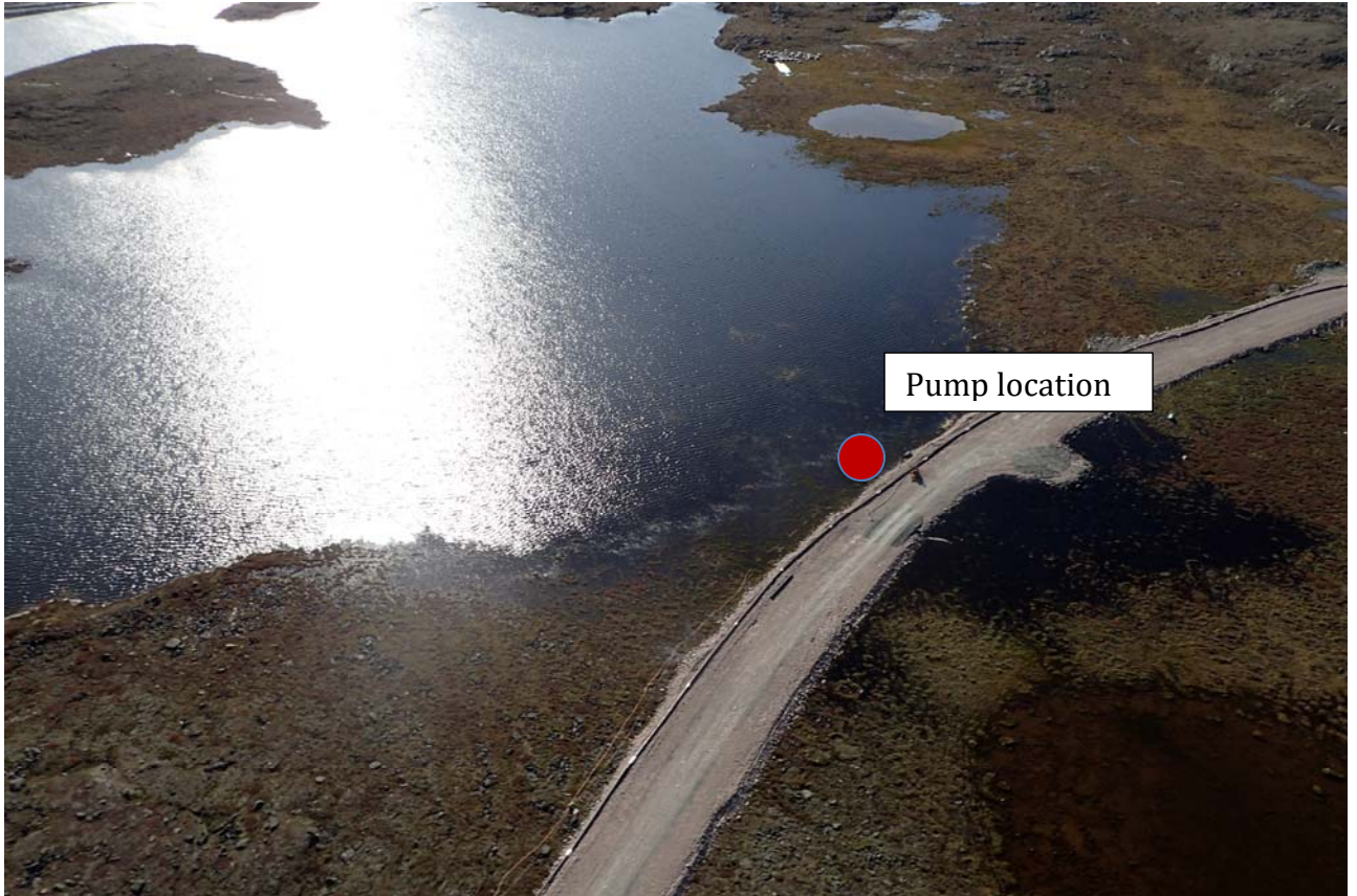
Figure 2: Pump Location (on road) at the north side of NE Pond
