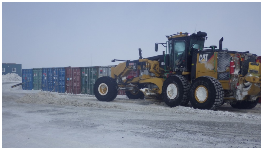
Figure 1: Grader scrapping up the frozen ground
