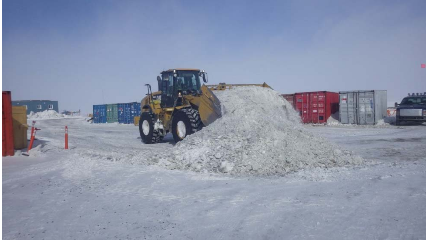
Figure 2: Loader piling up the frozen waste water
