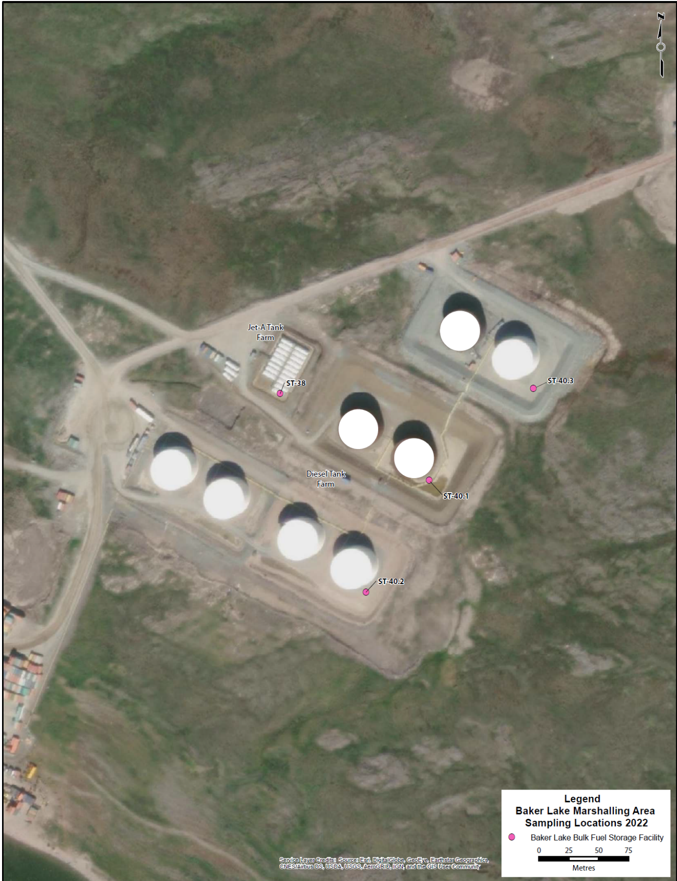
Figure 2: Baker Lake Diesel and Jet-A Fuel Tank Farm
