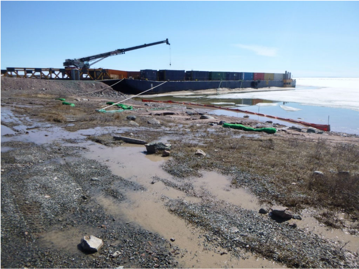
Figure 4. Mitigation Measures at BL-BARGE (2022/06/07)
