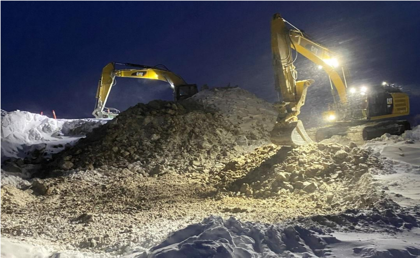
Figure 16. Excavation of spill area 2022-12-12
