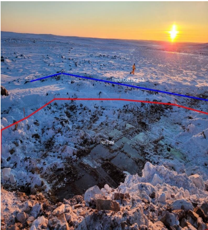
Figure 2. General view of incident from the road (2022-11-29)
