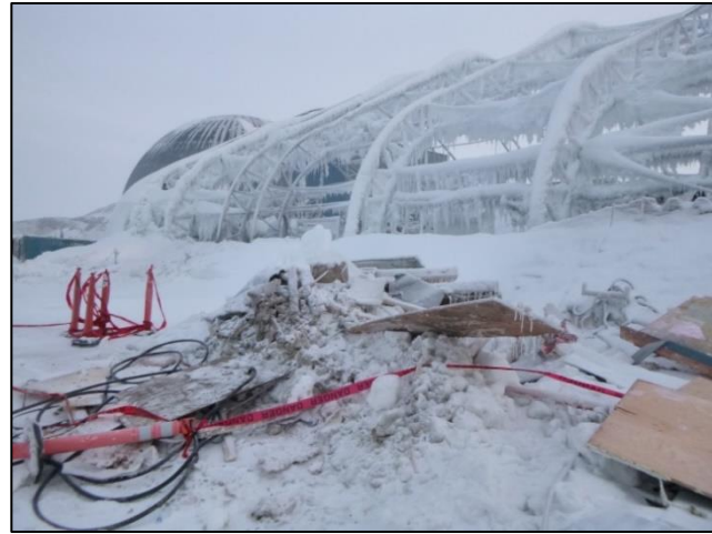
Photo 4: Taken facing Northeast of the Fire
