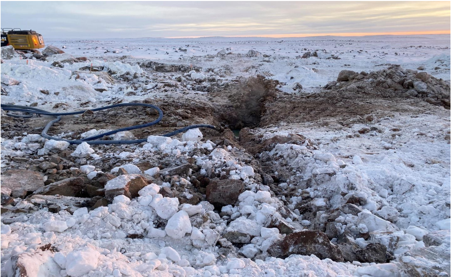
Figure 9. Surface drainage trenches -2022-12-02
