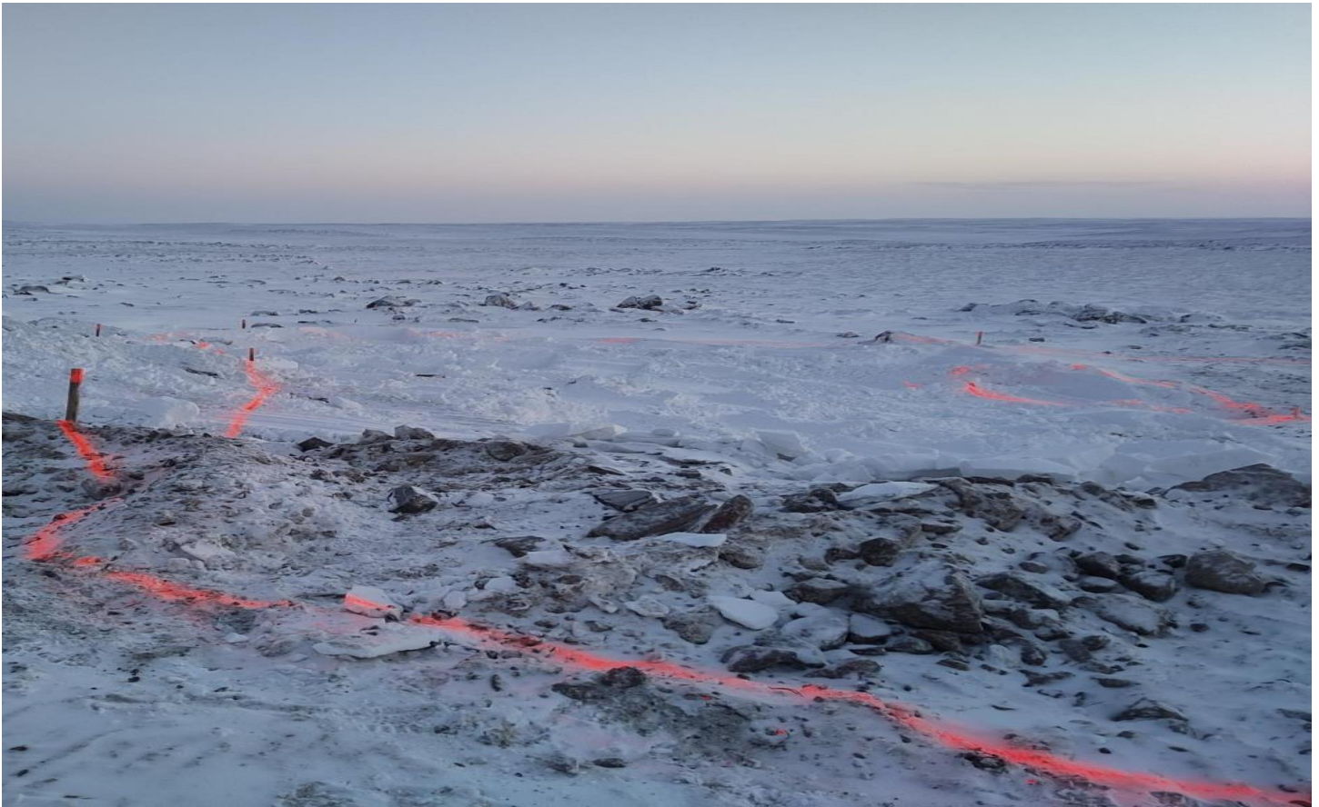
Figure 13. Spill zone delineated for snow removal after blizzard and additional excavation 2022-12-07
