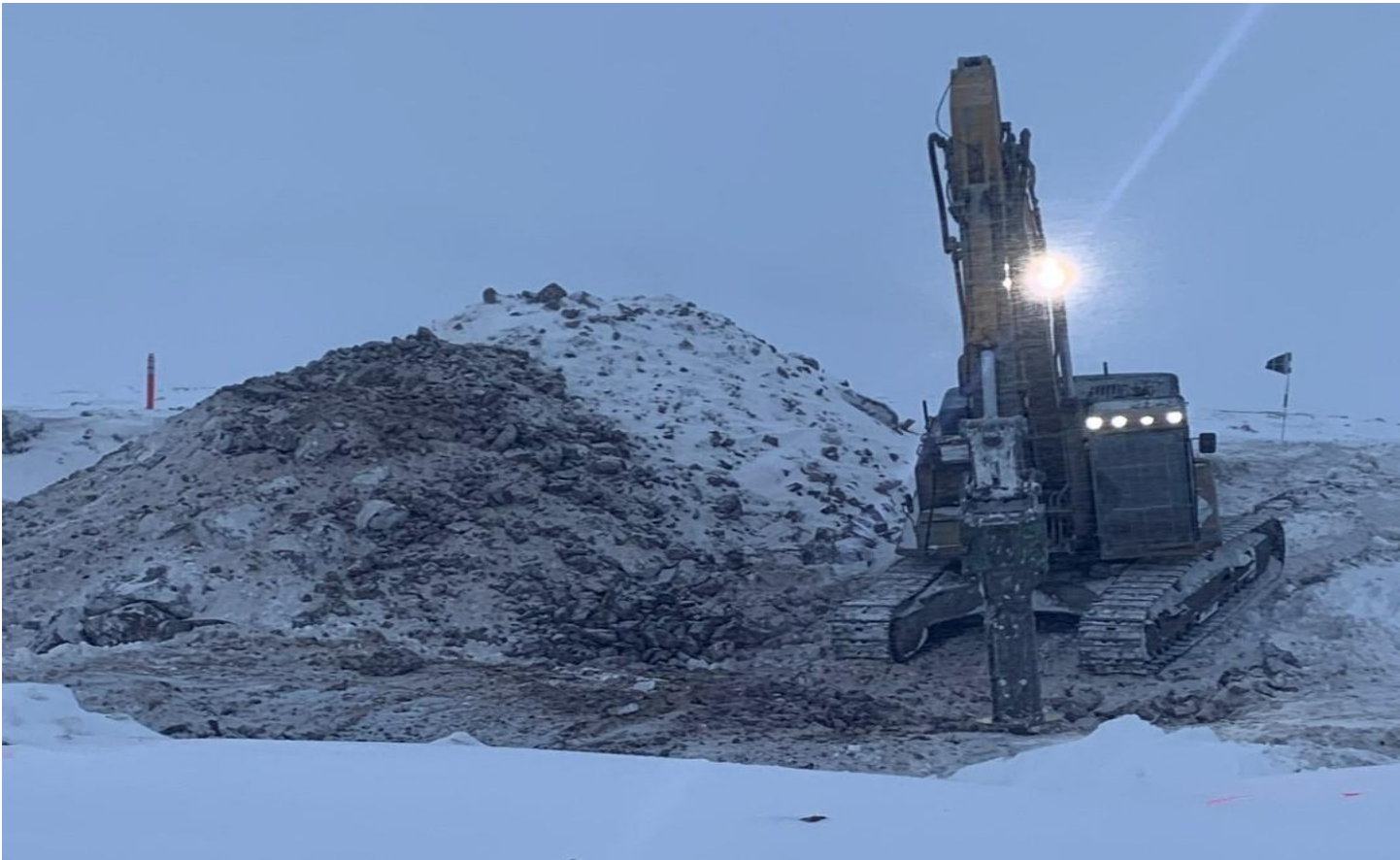
Figure 15. Excavation of spill area 2022-12-12
