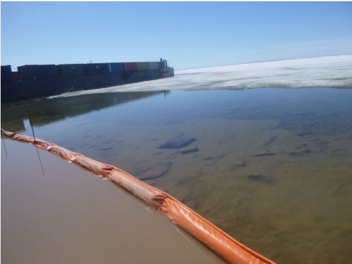
Figure 5. Contained turbidity & sediments at BL-BARGE (2022/06/10)
