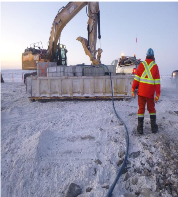
Figure 4. Pumping to totes (2022-11-29)
