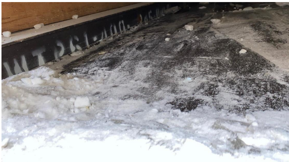
Figure 4. Grease Spill after cleanup efforts
