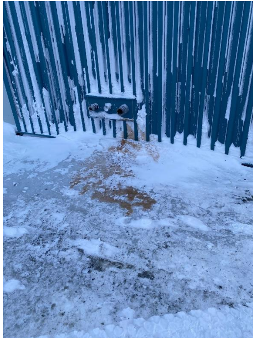
Figure 1. Emulsion facility, dated January 6th
