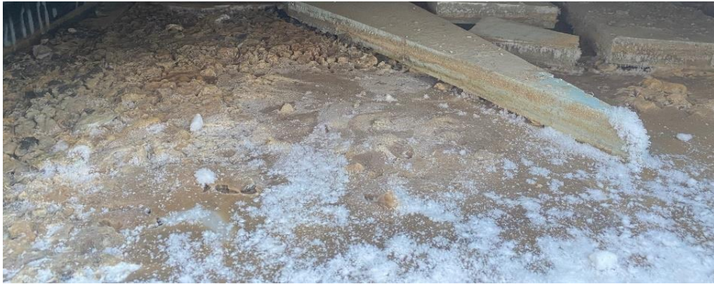
Figure 3. Grease under the wing ~24 hours post spill – 2022-02-04
