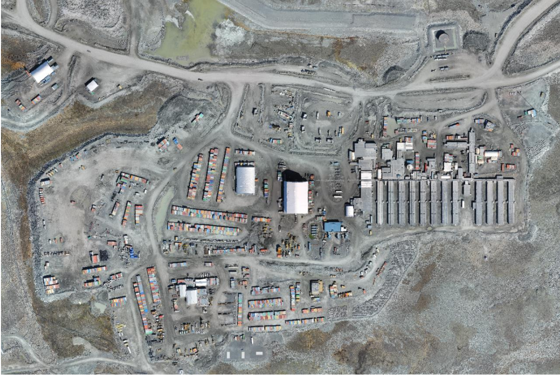
Figure 1-3 Aerial photo showing Whale Tail camp infrastructure (Summer 2022)
