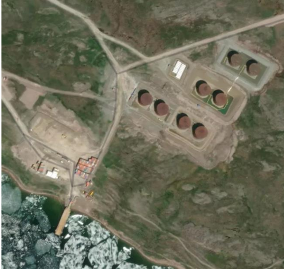
Figure 2-1 - Agnico's Baker Lake Oil Handling Facility – Ship to Shore Transfer Area
