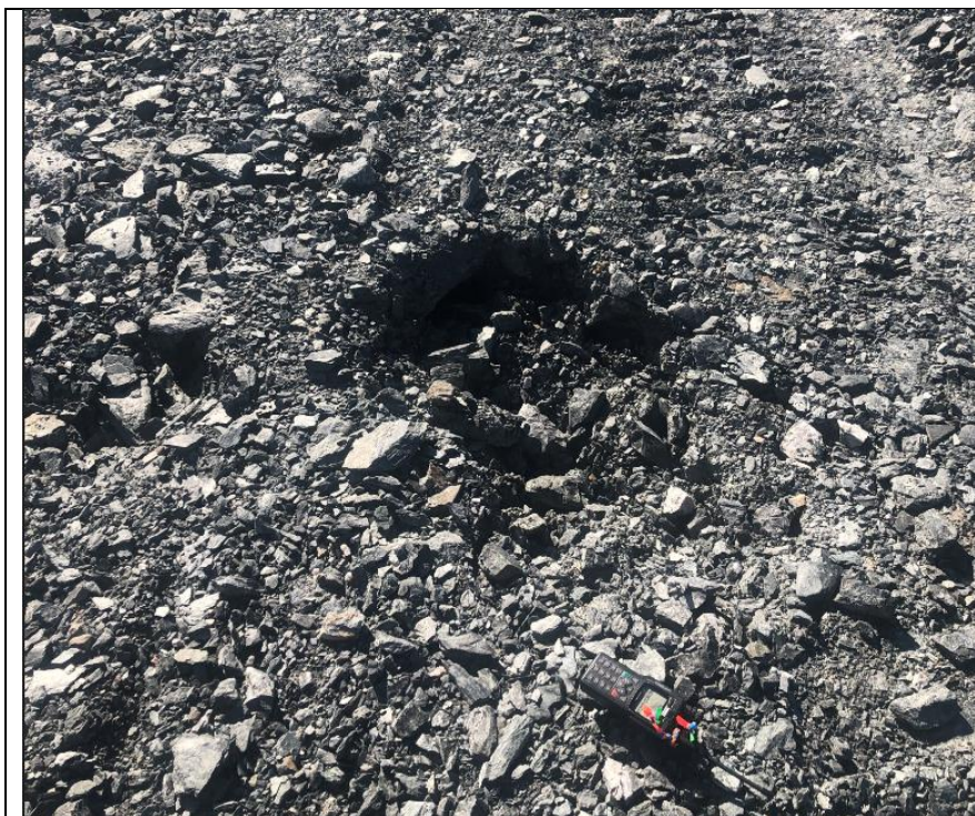
CR2: Rolling surface. Small puddles at surface, no damages
