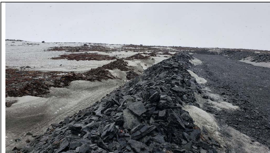
DS1: Downstream slope and berm.
