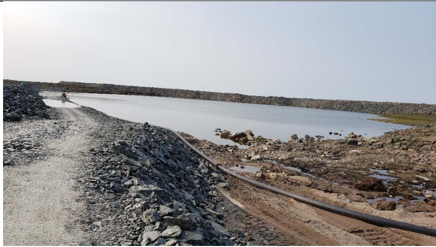
US1: Upstream slope. Water elevation at 156.02m.
