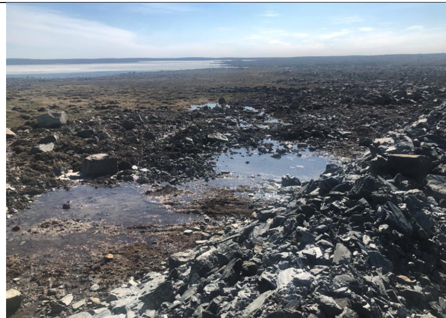
DS2: Downstream slope and berm.
