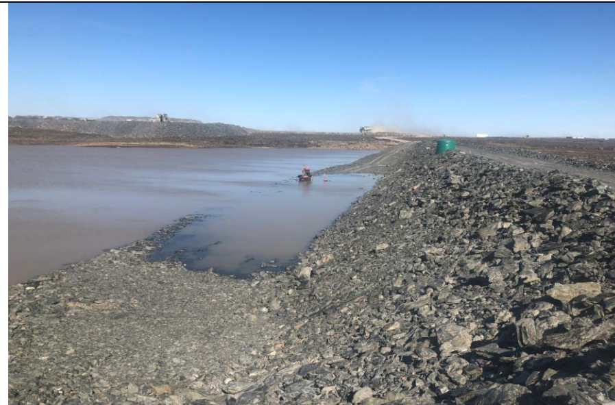
US1: Upstream slope. Water pond far from structure & frozen.
