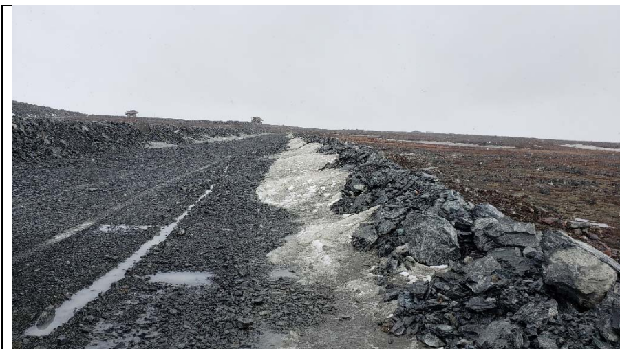
DS2: Downstream slope and berm.
