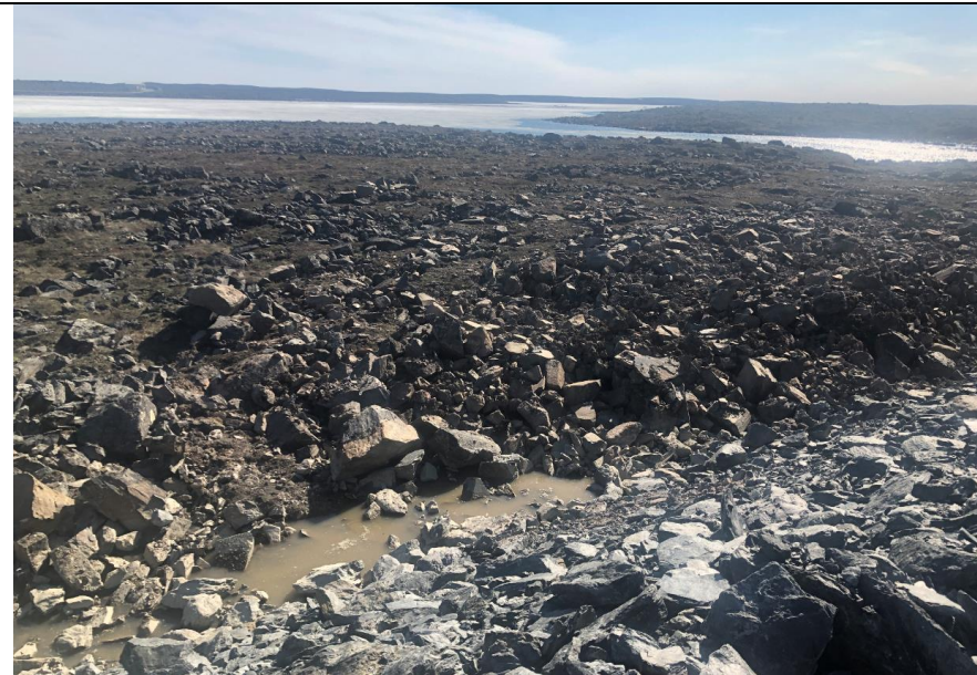
DS1: Downstream slope and berm.
