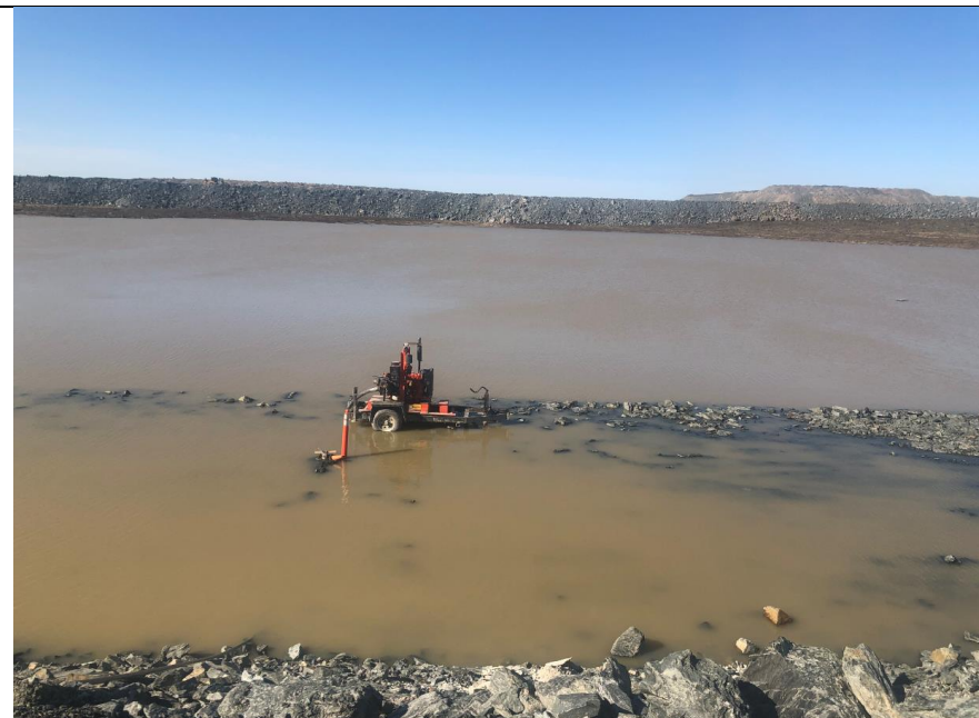
US2: Upstream slope.
