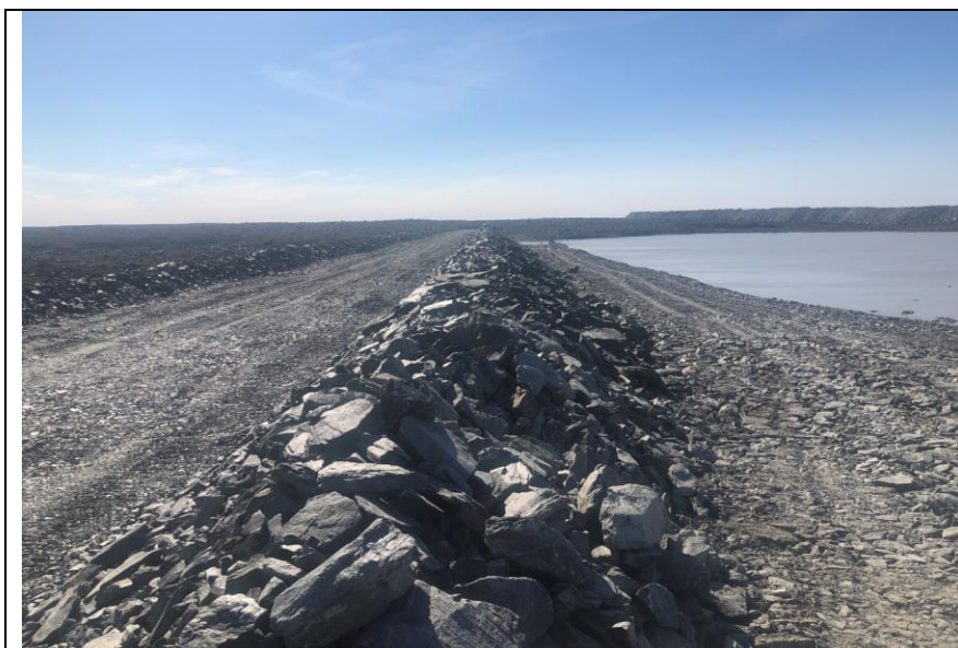
CR1: Rolling surface. Small puddles at surface, no damages
