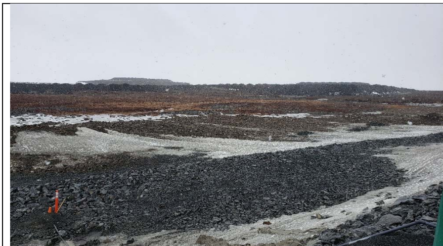
US2: Upstream slope.
