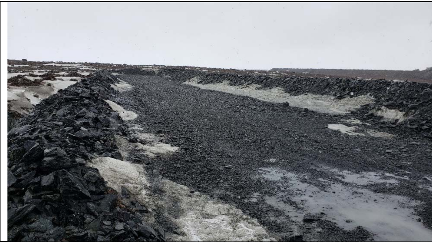
CR1: Rolling surface. Small puddles at surface, no damages
