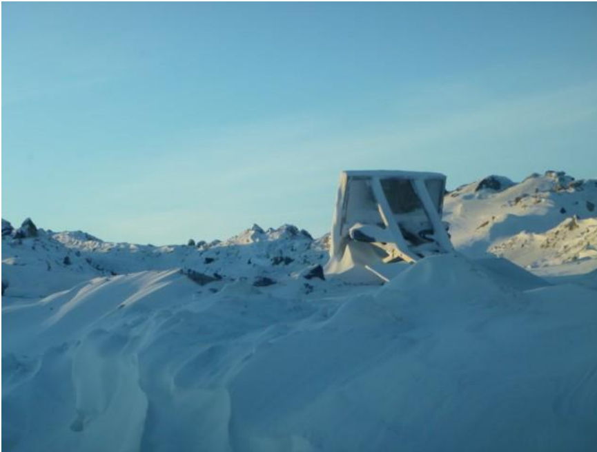
Photo 1: Sign posted to inform of a waste disposal facility fell down.
