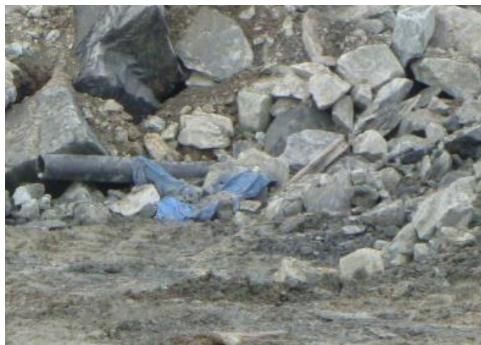
Picture 1: Plastic pipe and tarp
