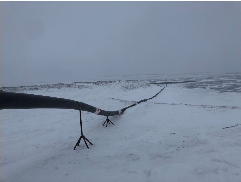
Picture 9 Final suction line installation
