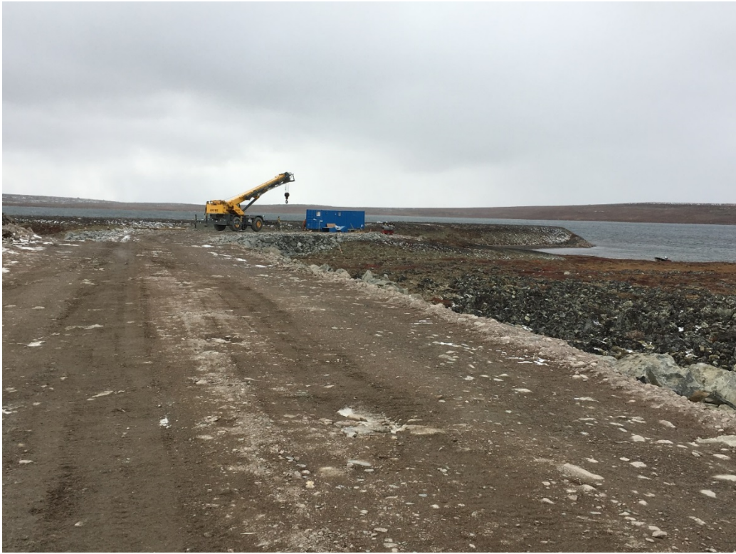
Picture 1 Pumping station installation
