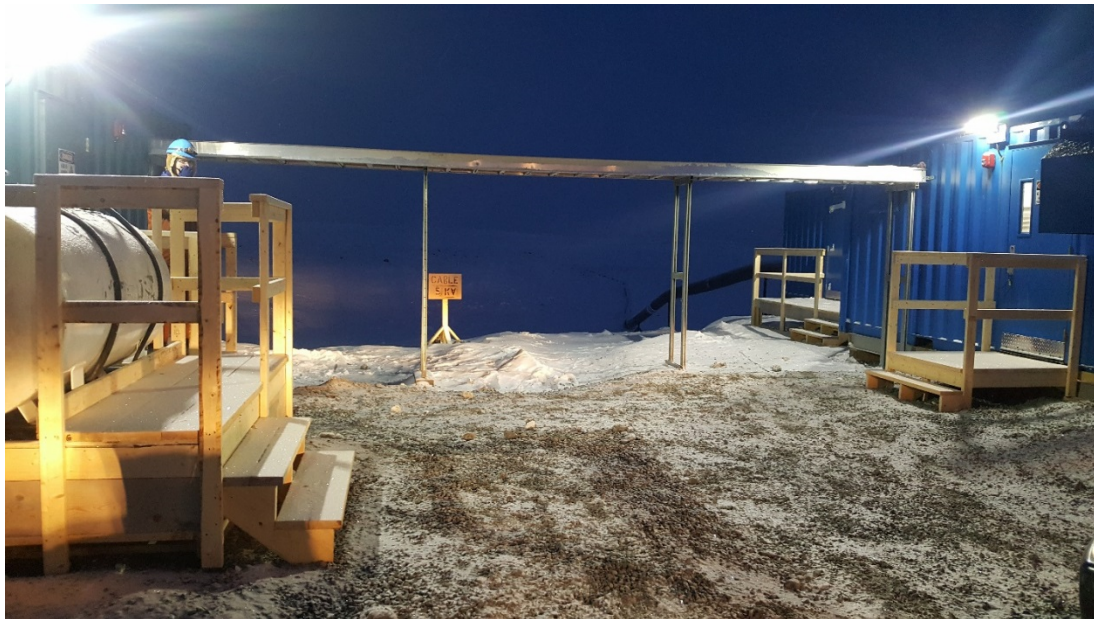
Picture 4 Pumping station after construction
