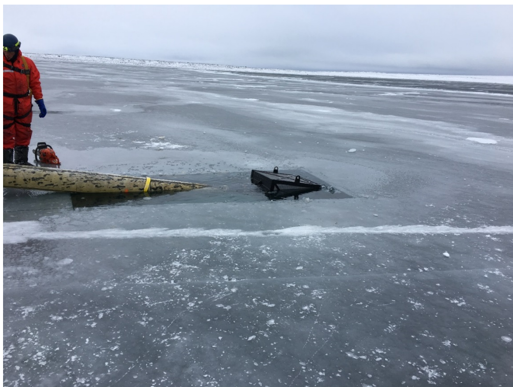
Picture 8 Suction line sinking
