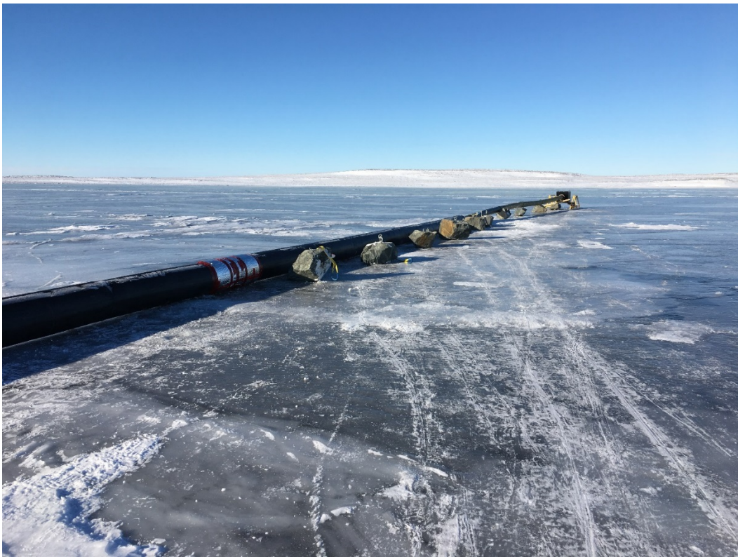
Picture 6 suction line with ballast on lake ice
