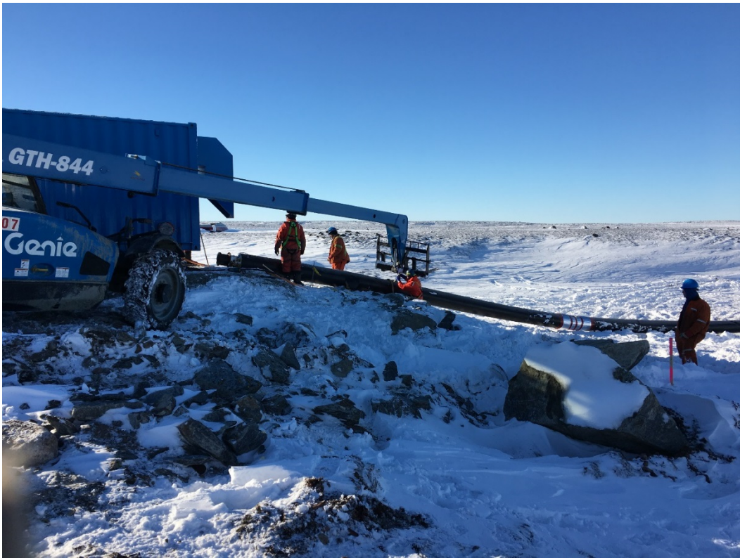
Picture 5 Telehandler pushing pipe with boom
