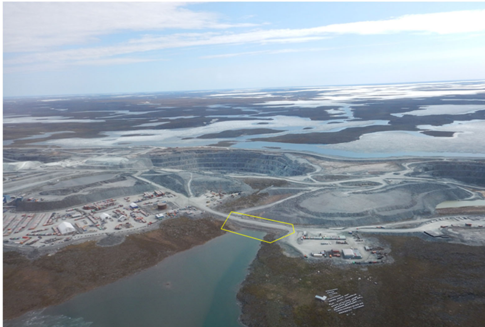
Figure 3-5 : Aerial View of South Camp Dike
