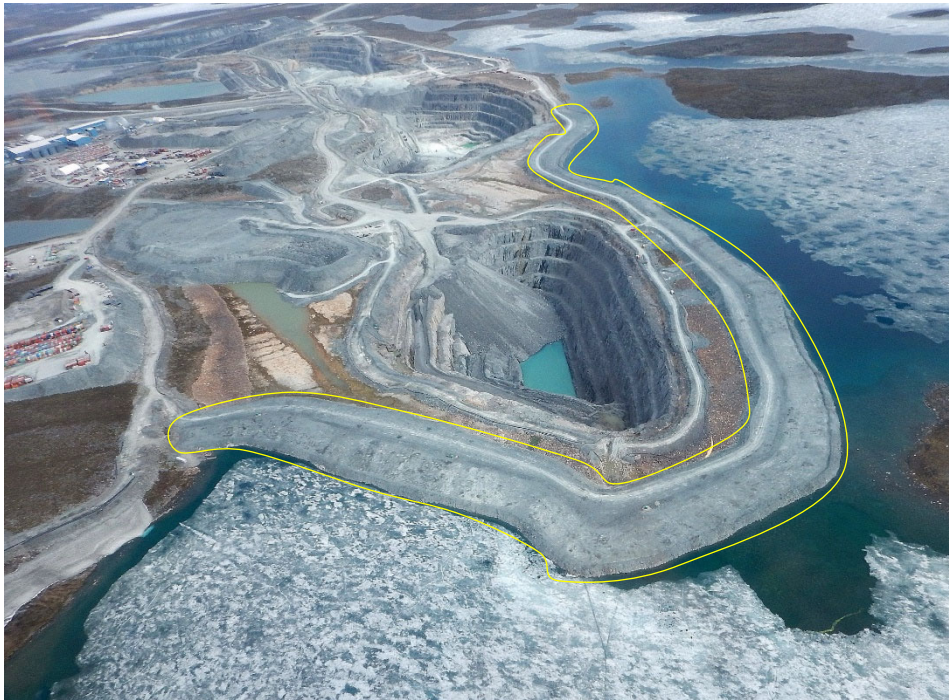
Figure 3-3 : Aerial View of Bay-Goose Dike
