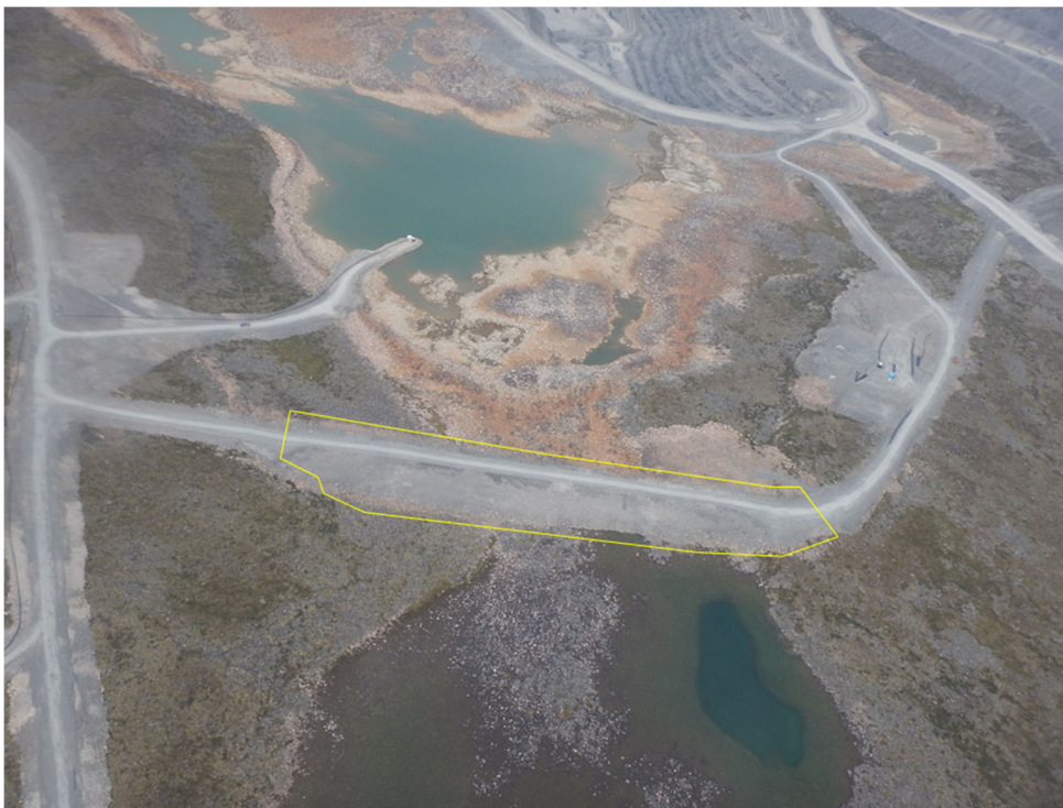
Figure 3-7 : Aerial View of Vault Dike
