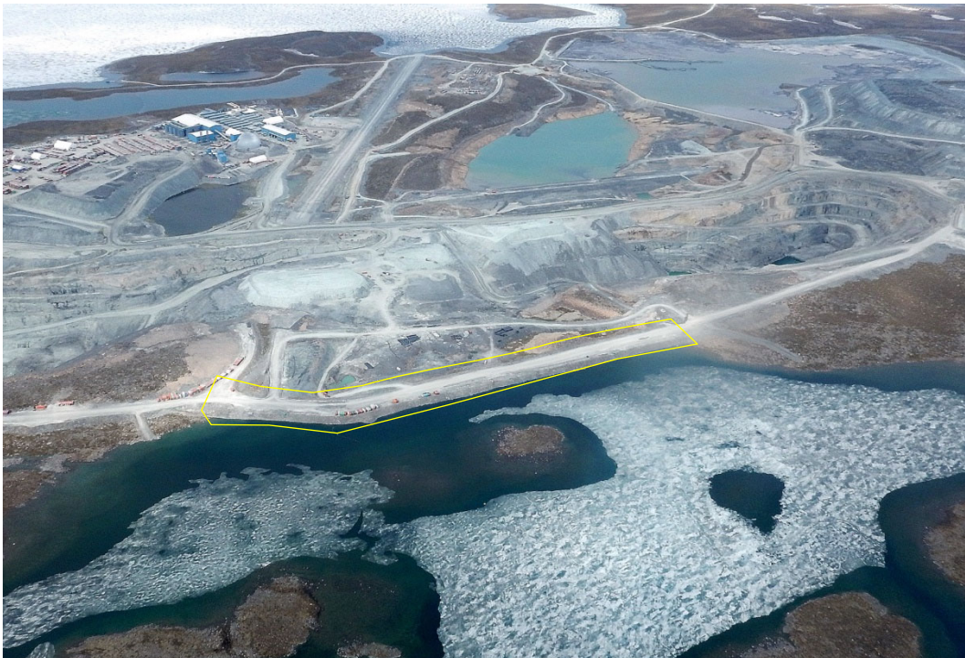
Figure 3-1 : Aerial View of East Dike
