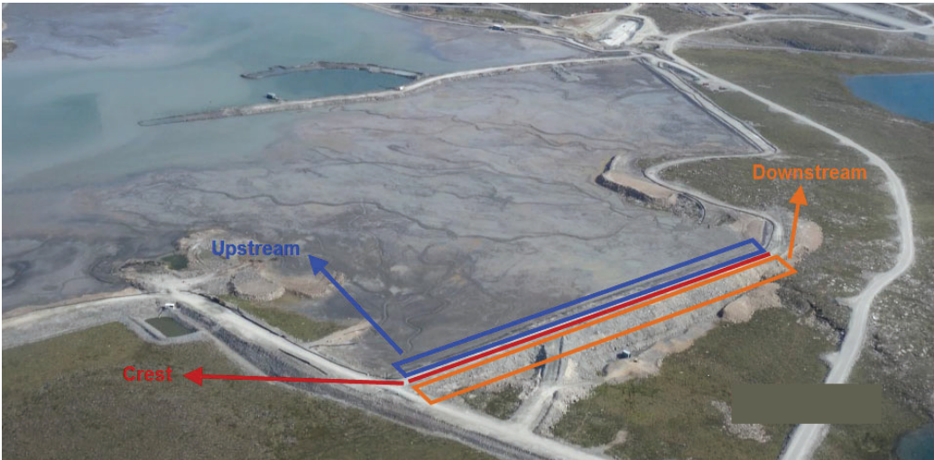
Figure 3-2: Aerial View of Saddle Dam 1
