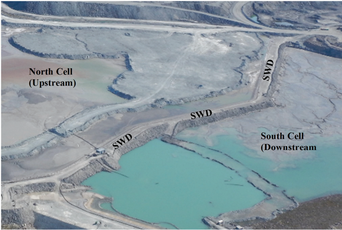
Figure 3-15: Aerial View of Stormwater Dike (2019)
