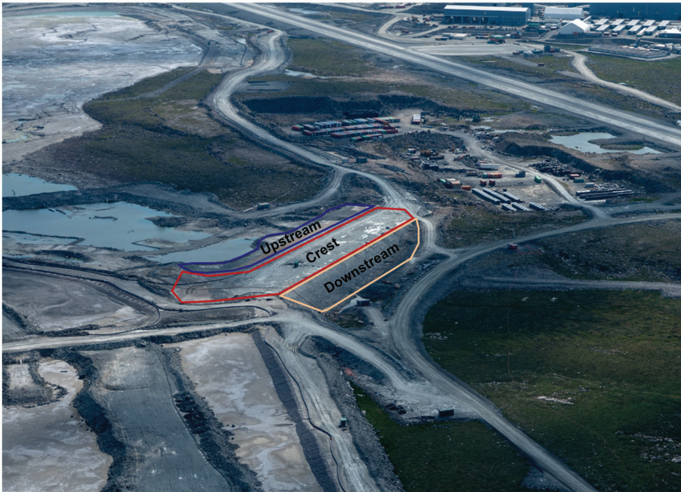
Figure 3-10: Aerial View of Saddle Dam 3
