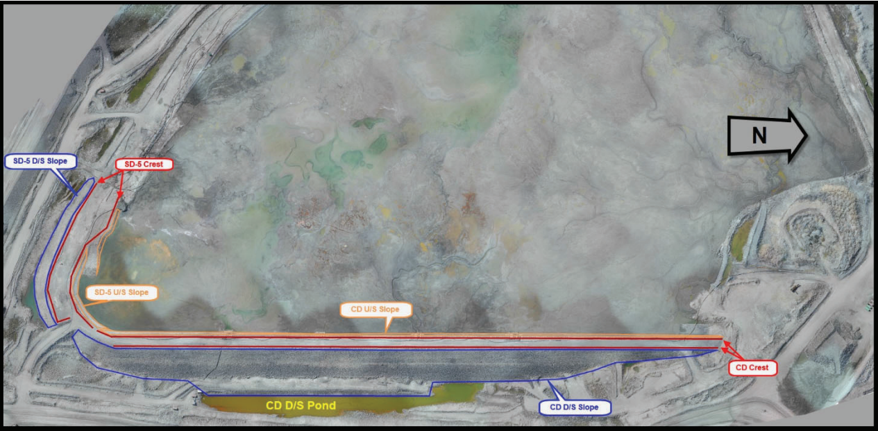
Figure 3-13: Aerial View of Central Dike and SD5
