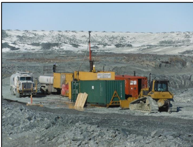
Drilling installation at monitoring well MW-IDP-09.
