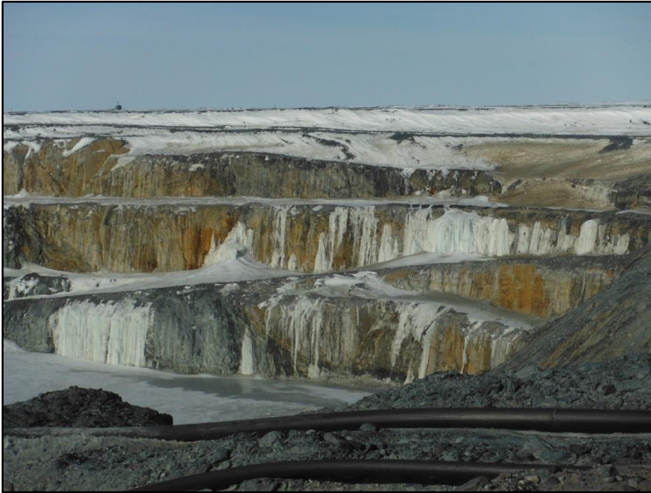
Goose Pit view looking southwest. All wall faces show frozen ice sheets at seepage areas.
