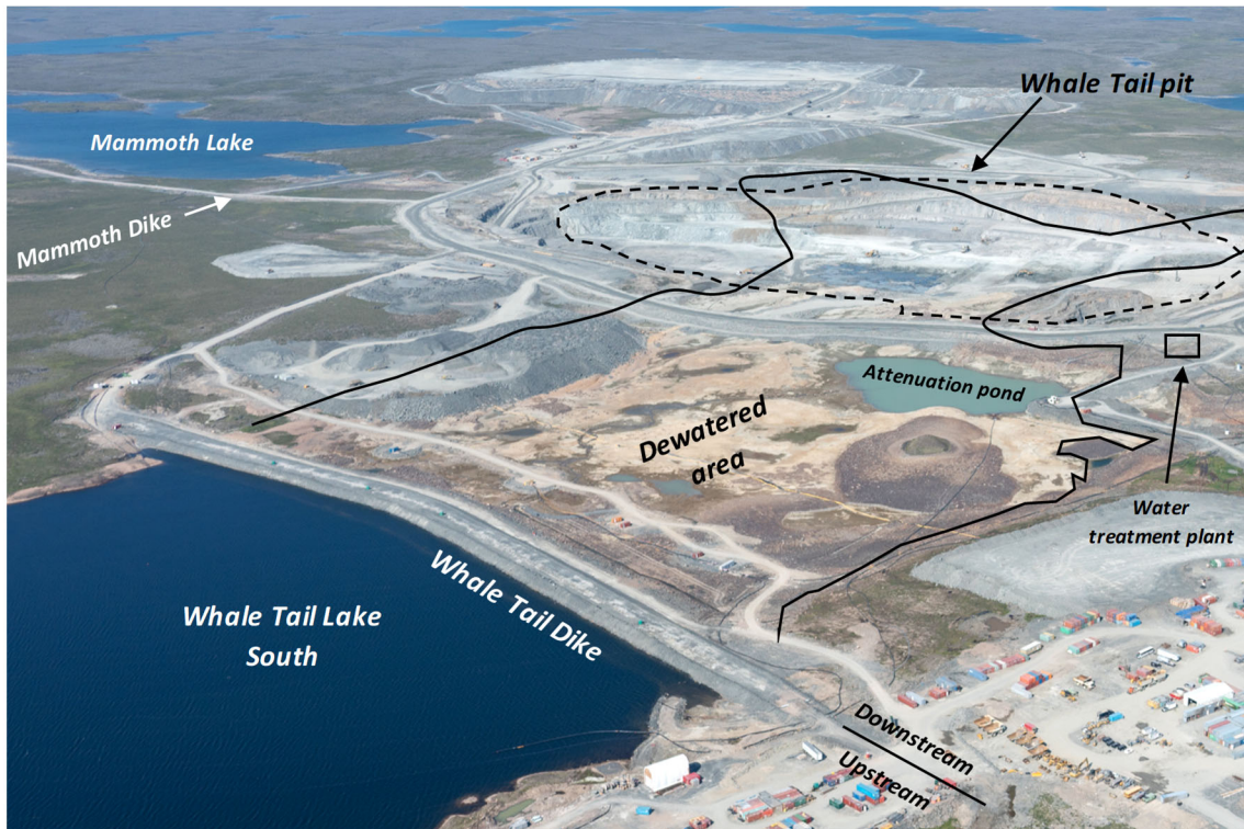
Figure 3-1 : Aerial View of Whale Tail Dike
