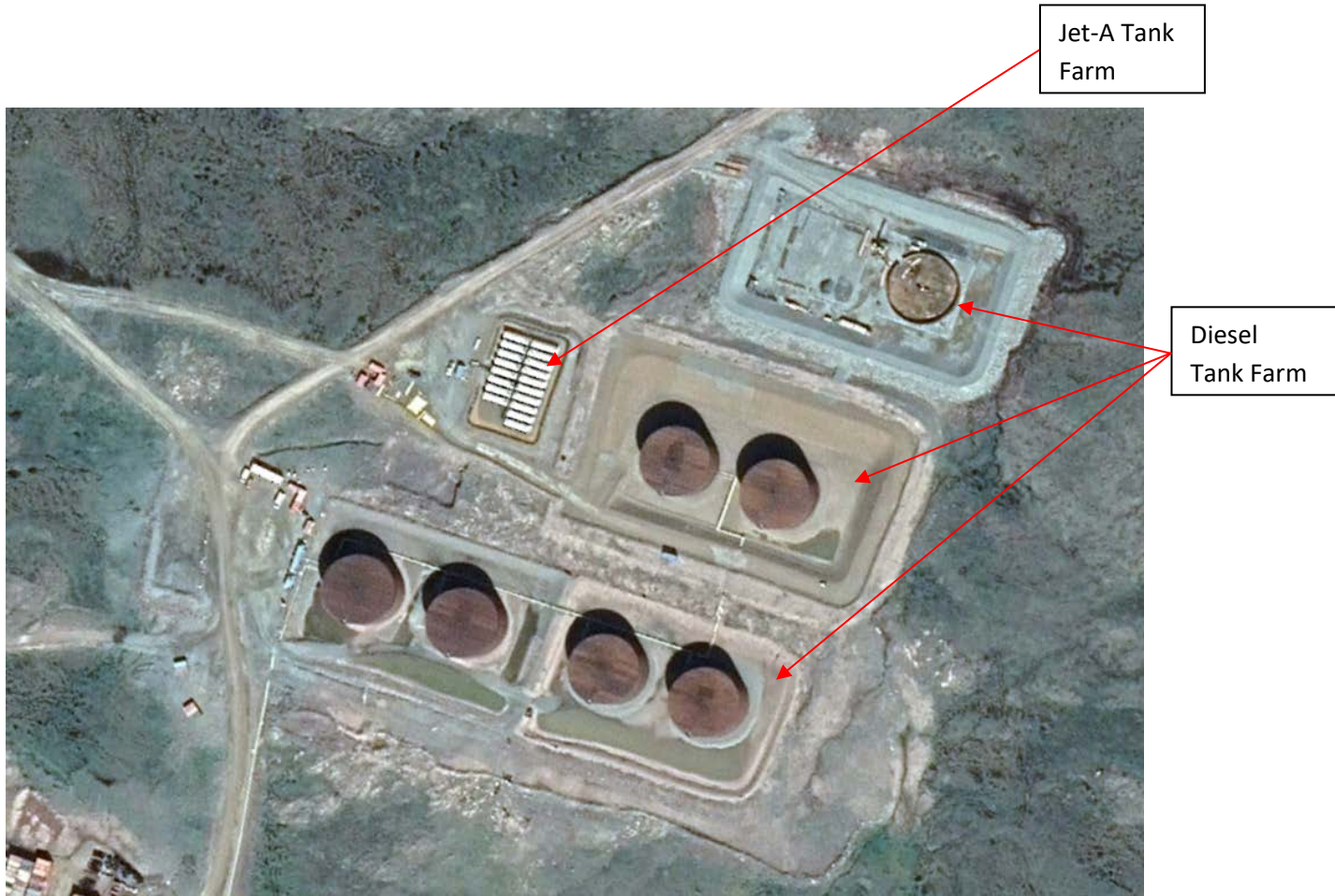
Figure 2 – Agnico’s Baker Lake Bulk Fuel Storage Facility Site Layout (including secondary containment for Tank no.8 to be added in following year)
