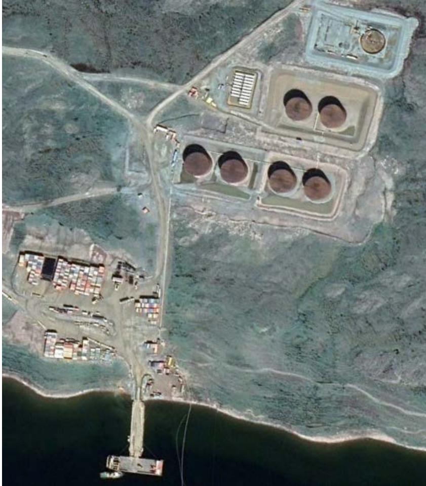
Figure 2-1 - Agnico's Baker Lake Oil Handling Facility – Ship to Shore Transfer Area
