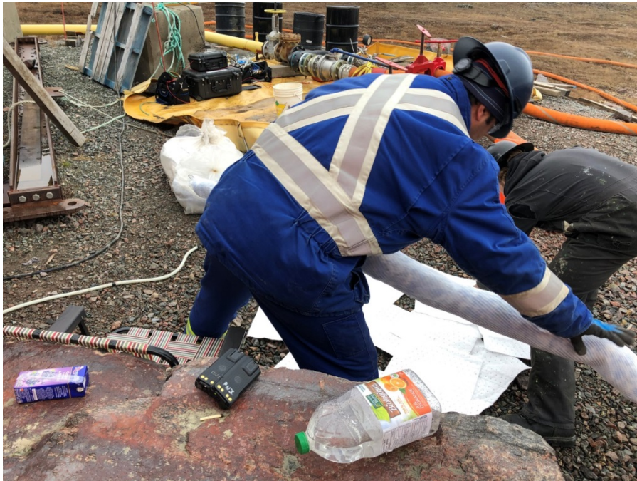
Photo 4 - Absorbent sheets and booms applied downstream and on the contaminated area
