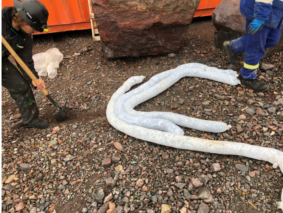
Photo 5 - Trench dug downstream of the spill to contain de spilled fluid
