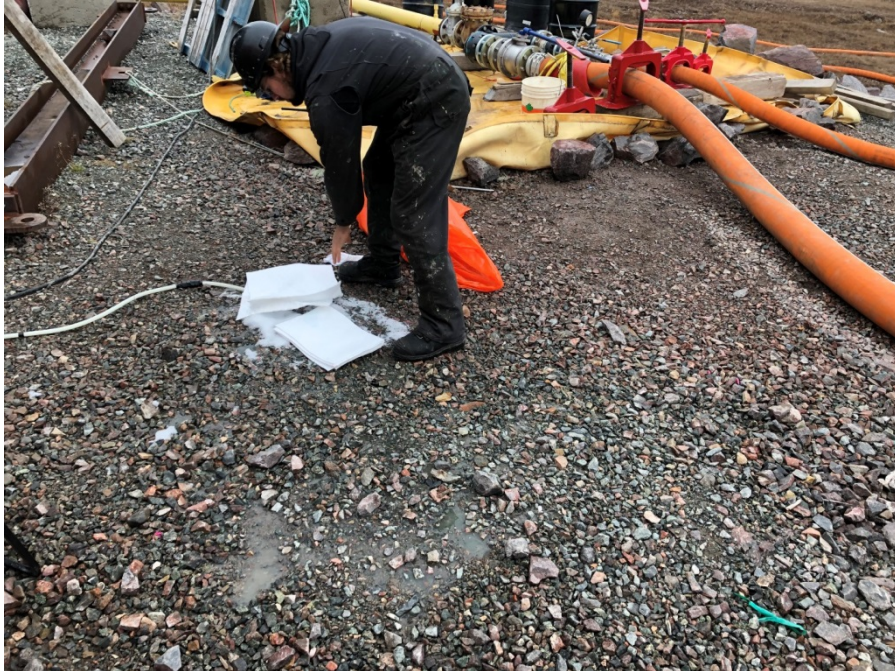
Photo 3 - Absorbent sheets applied on the contaminated area
