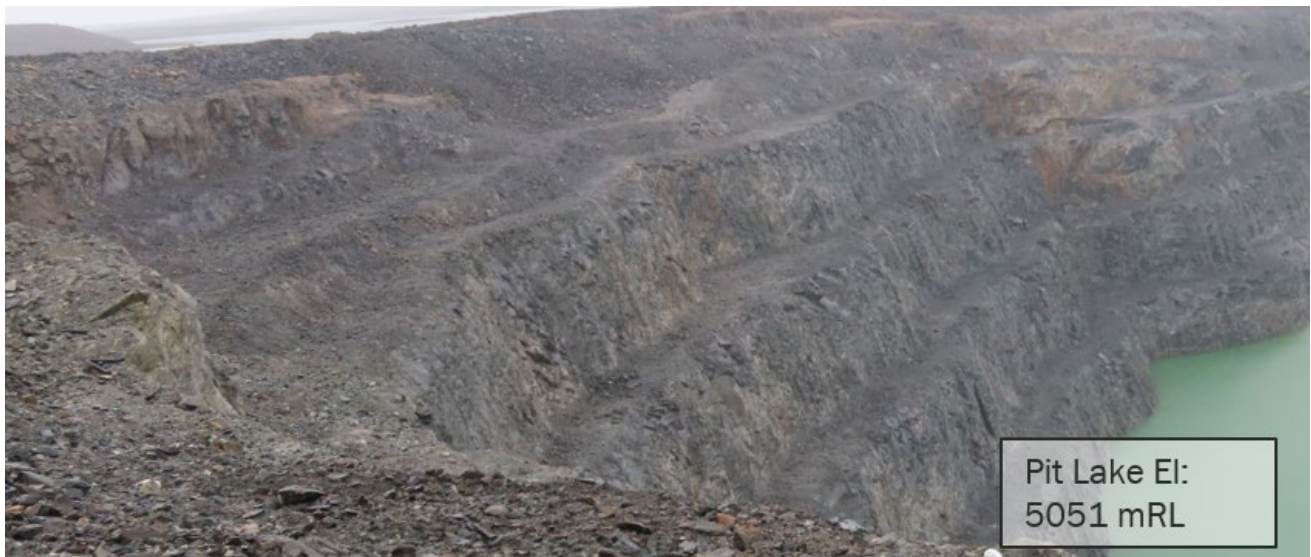
Photograph 4-6: Pit A East wall upper benches (2019)
