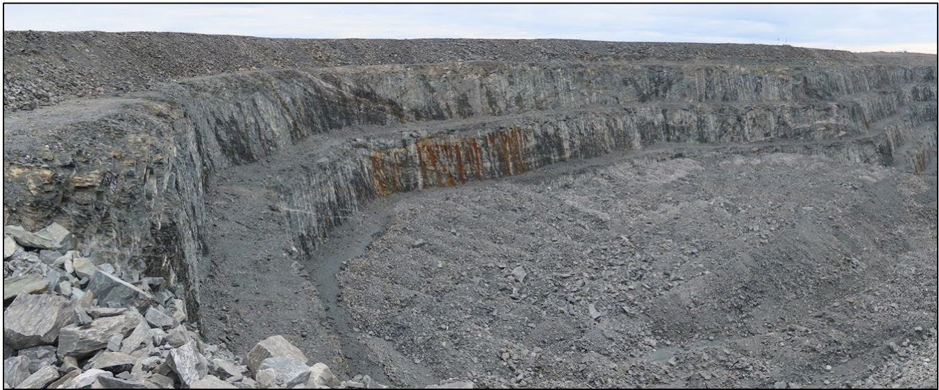
Photograph 8-16: Vault Pit northeast wall bench performance and 5088 mRL dump platform
