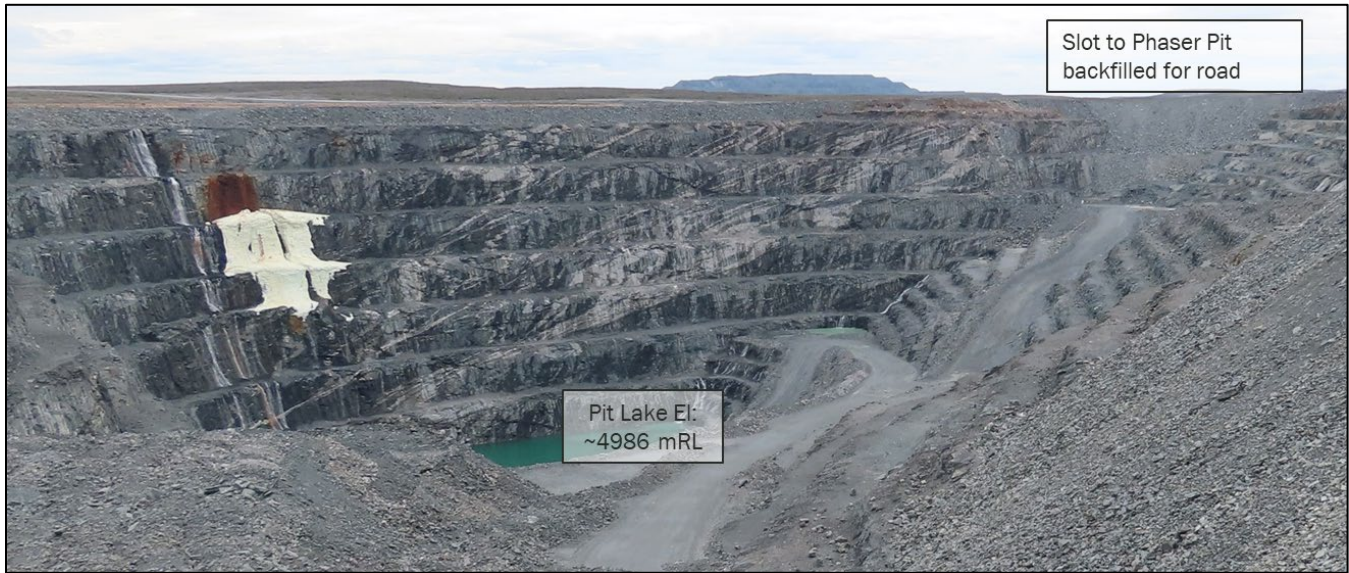
Photograph 8-8: Vault Pit sump and water flow from Phaser Pit
