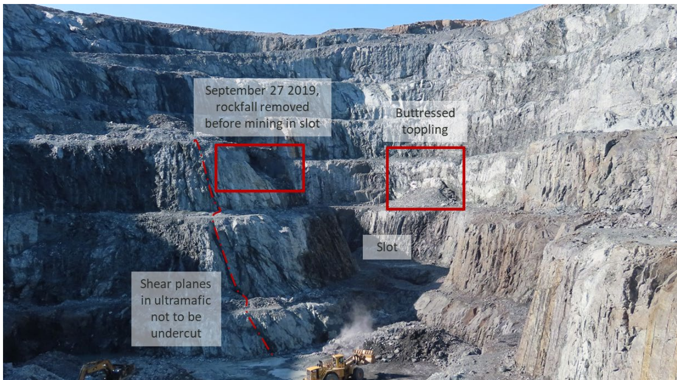
Photograph 6-22: Pit E slot (2019)
