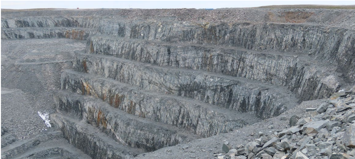
Photograph 8-10: Vault Pit east highwall bench performance, southeast end looking north (2019)
