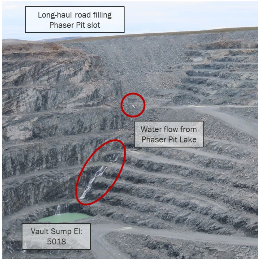
Photograph 8-4: Inflow to Vault Pit from Phaser Pit
