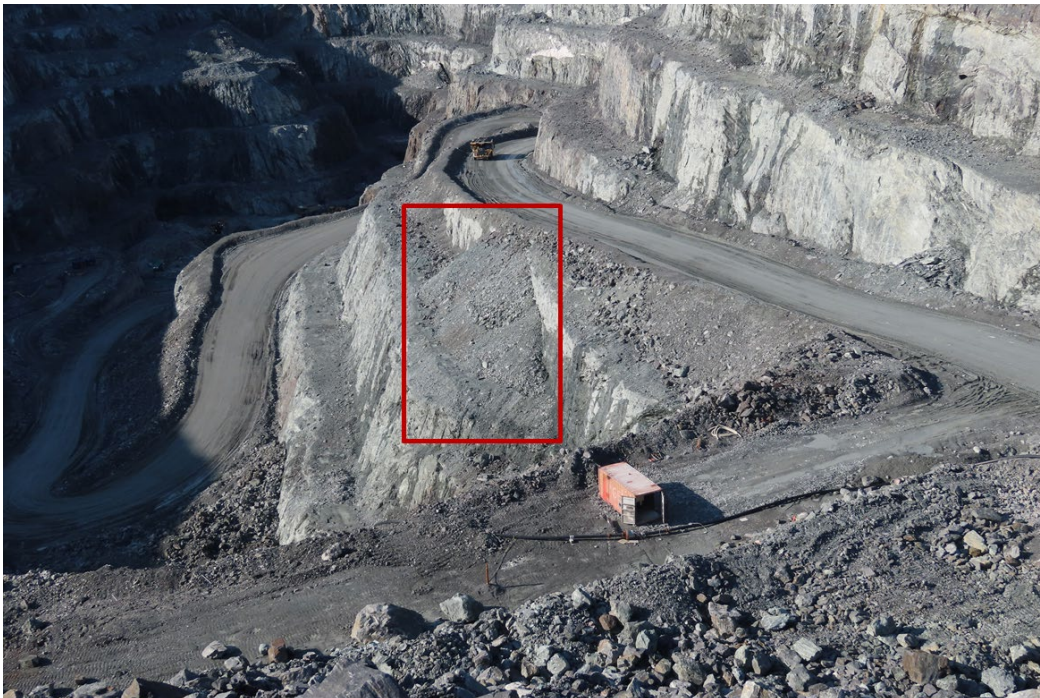
Photograph 6-21: Buttress support of ramp on west wall of Portage Pit
