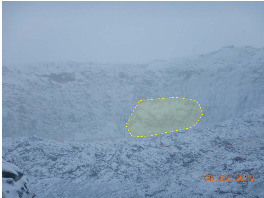
Zone BB13: BB Phaser, North East Wall: Fair dimension toe covering the corner; Hammering is recommended if possible.
