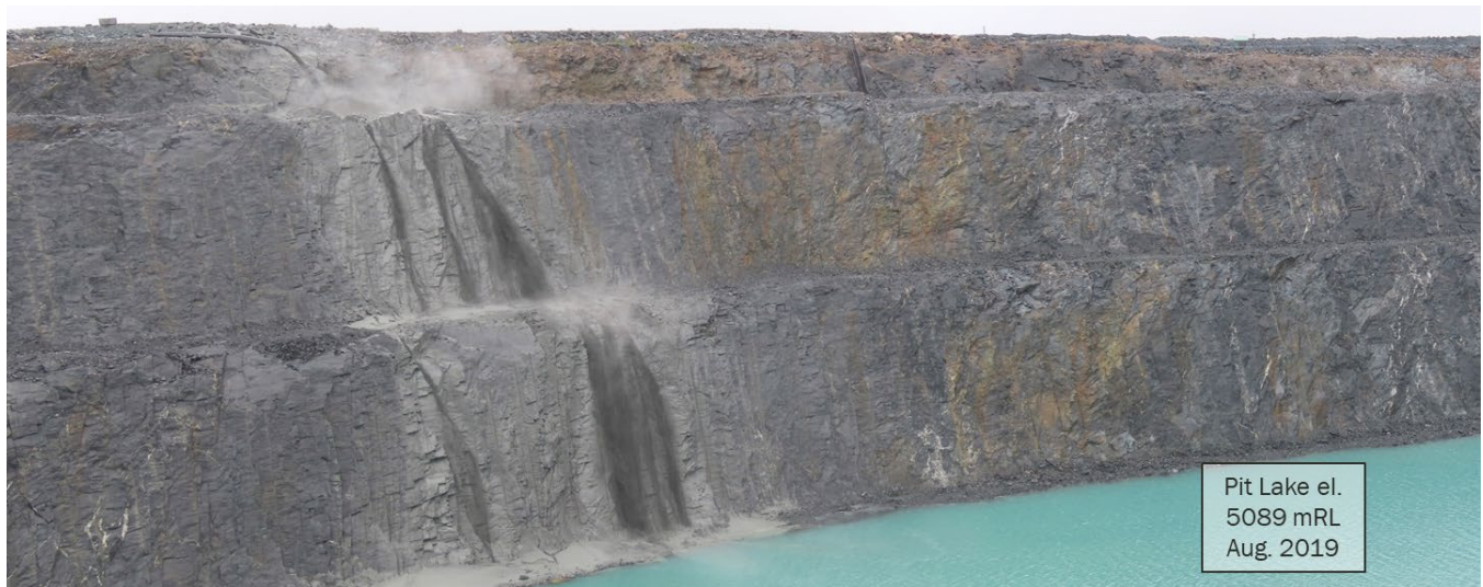
Photograph 7-2: Tailings discharge to Goose Pit from north end of east wall
