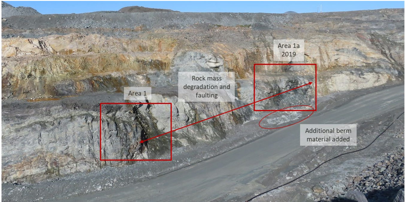
Photograph 6-15: Portage Pit West Ramp Area 1a instability
