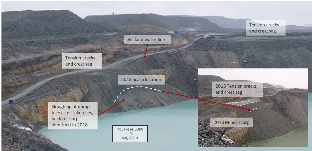
Photograph 7-10: Sloughing of Goose Pit South Dump face (2019)
