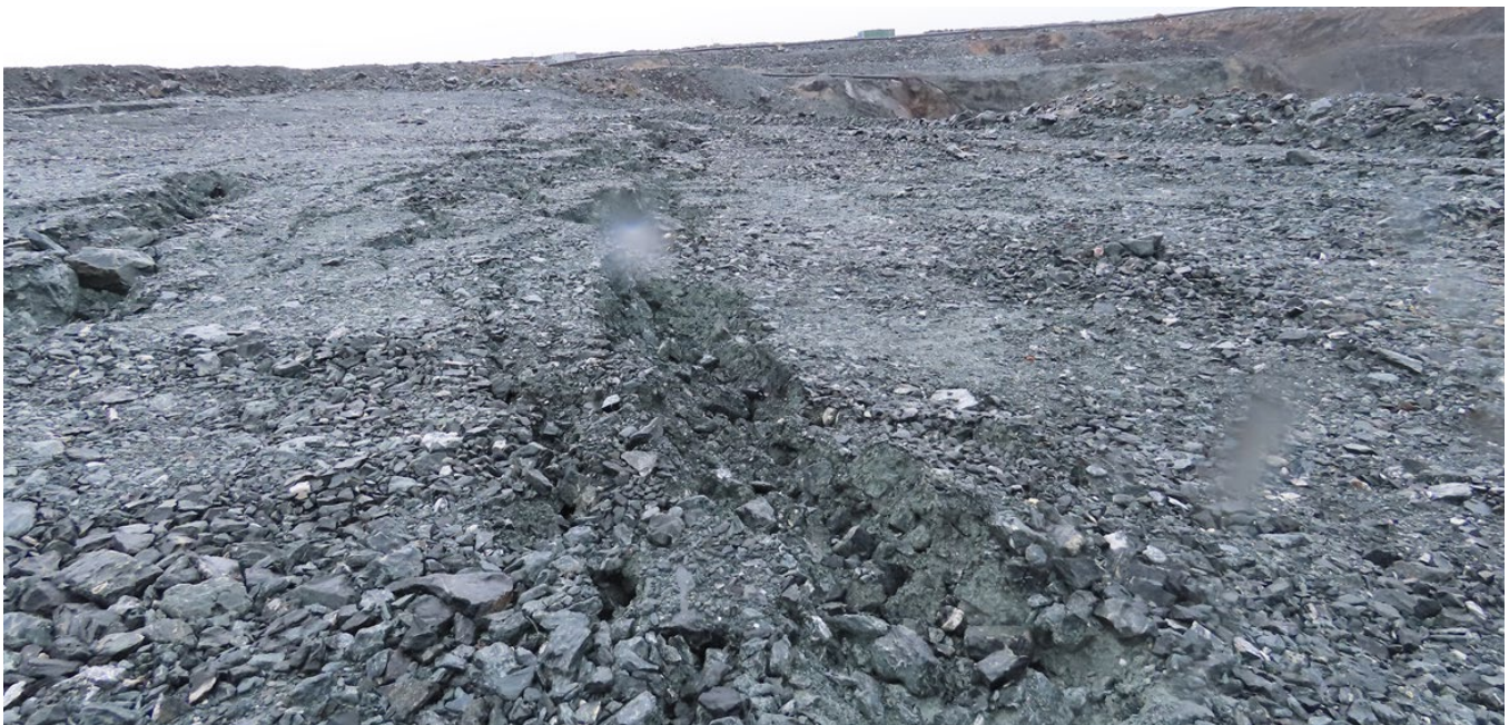
Photograph 7-9: Tension cracks and crest sag Goose Pit North Dump (2019)
