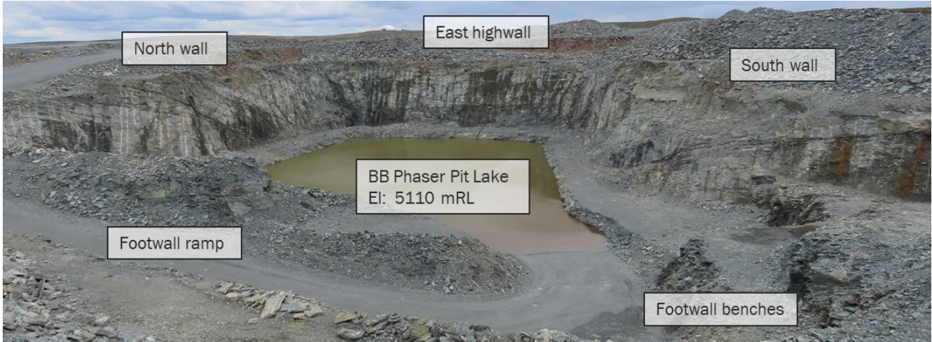
Photograph 8-20: BB Phaser Pit east highwall, endwalls and pit lake (2019)
