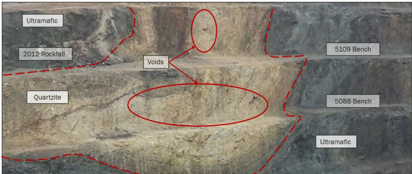
Photograph 4-4: Voids in quartzite above Pit A west ramp (2019)
