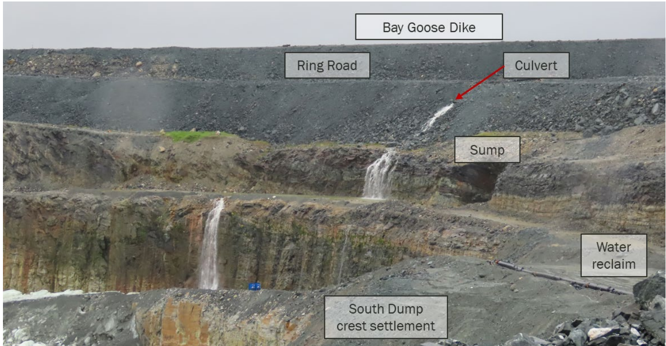
Photograph 7-4: Discharge of water from the water management pond between the ring road and Bay Goose Dike
