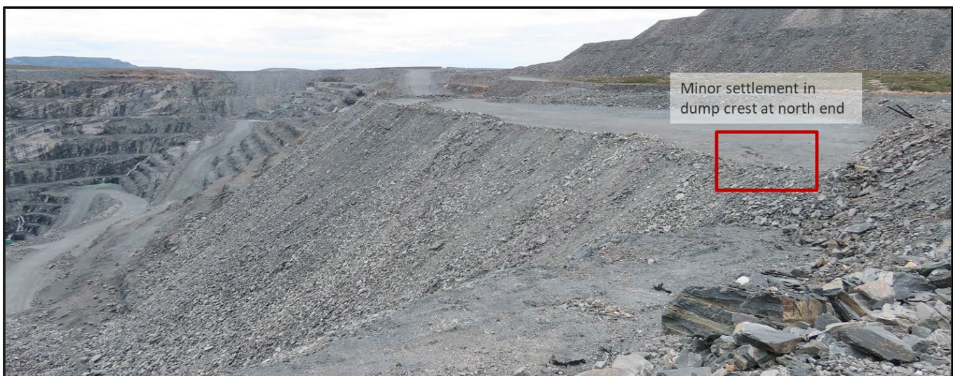
Photograph 8-17: Minor settlement of dump crest at north end
