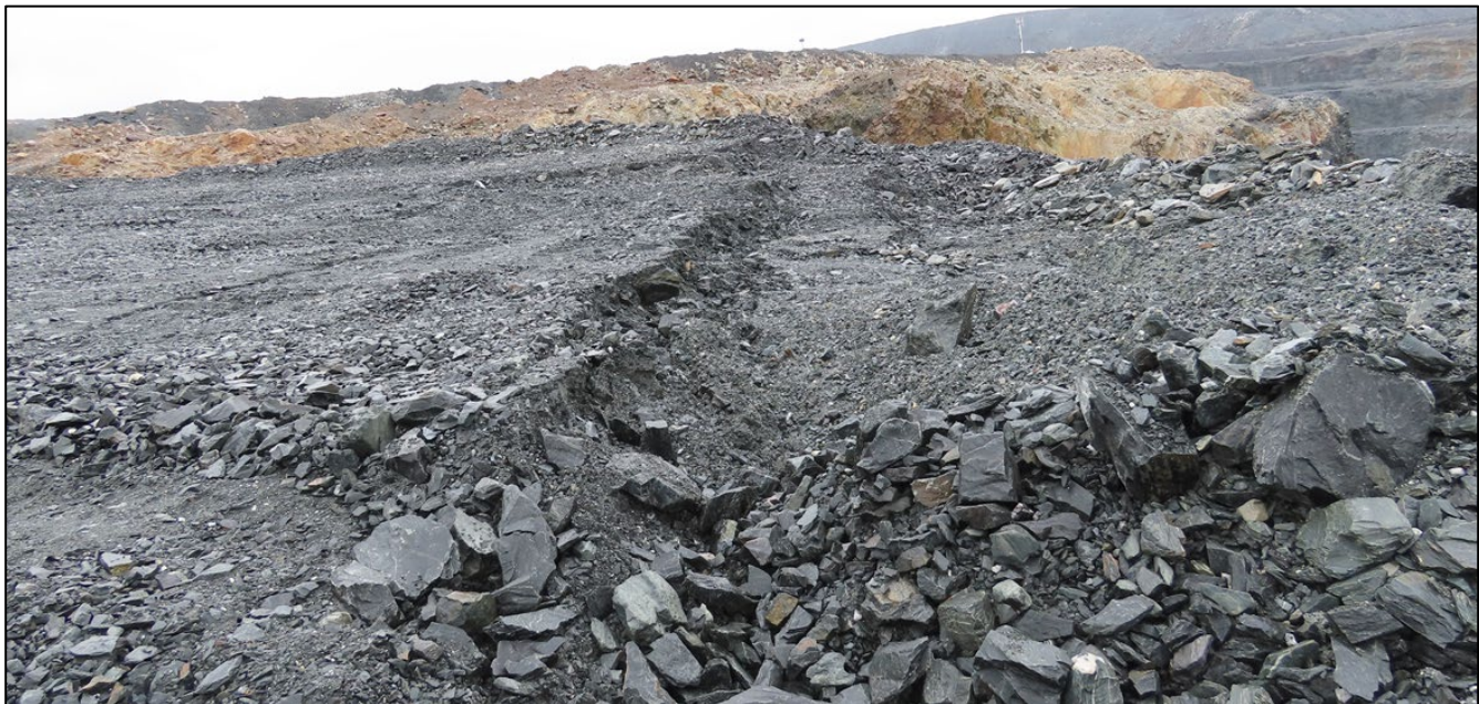
Photograph 4-11: B Dump showing settlement at north end of dump platform
