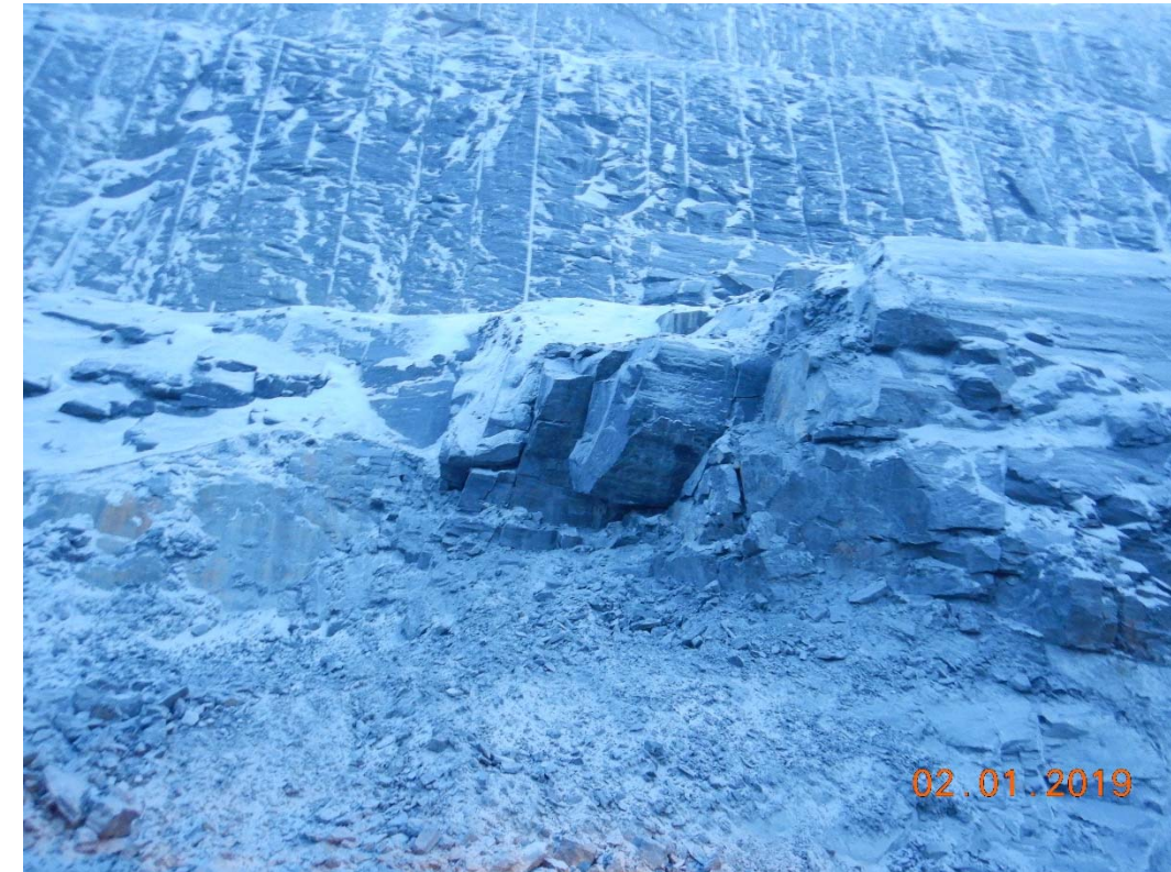
Zone E53: E5, East Wall: to be monitored with the radar.
