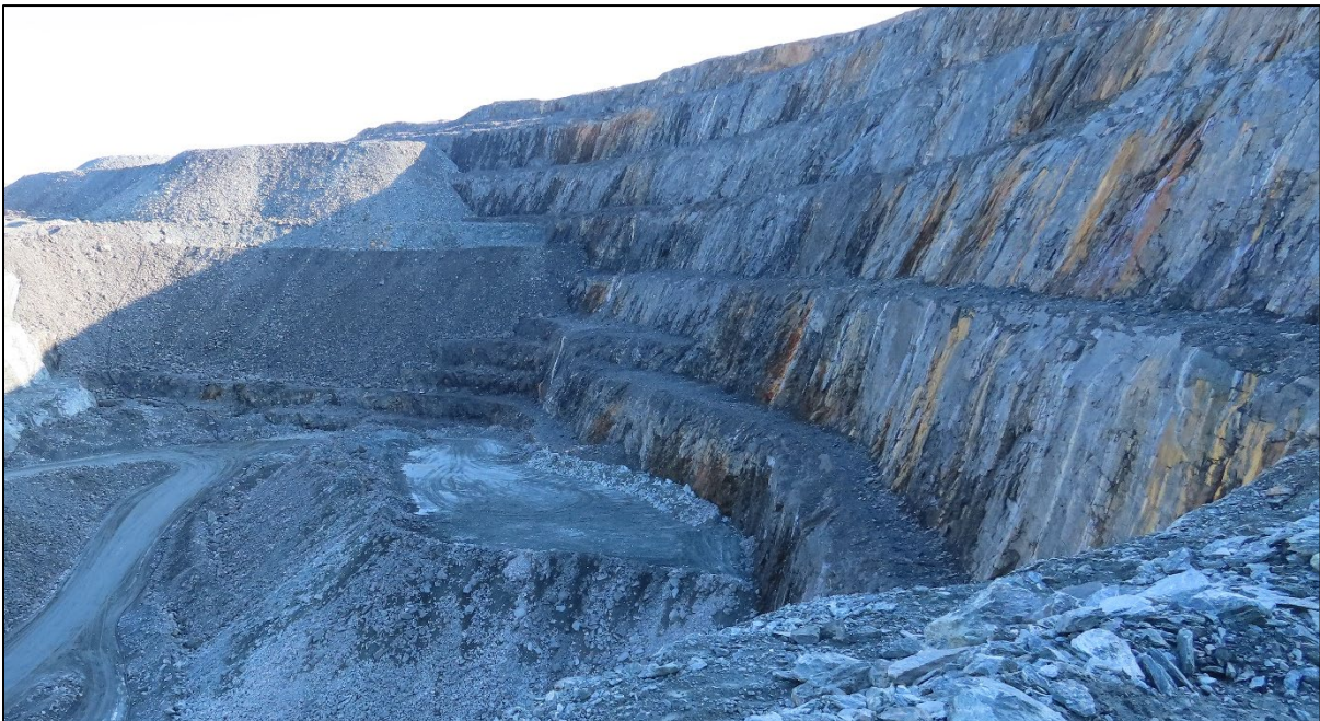
Photograph 6-2: Pit E east wall performance (2019)
