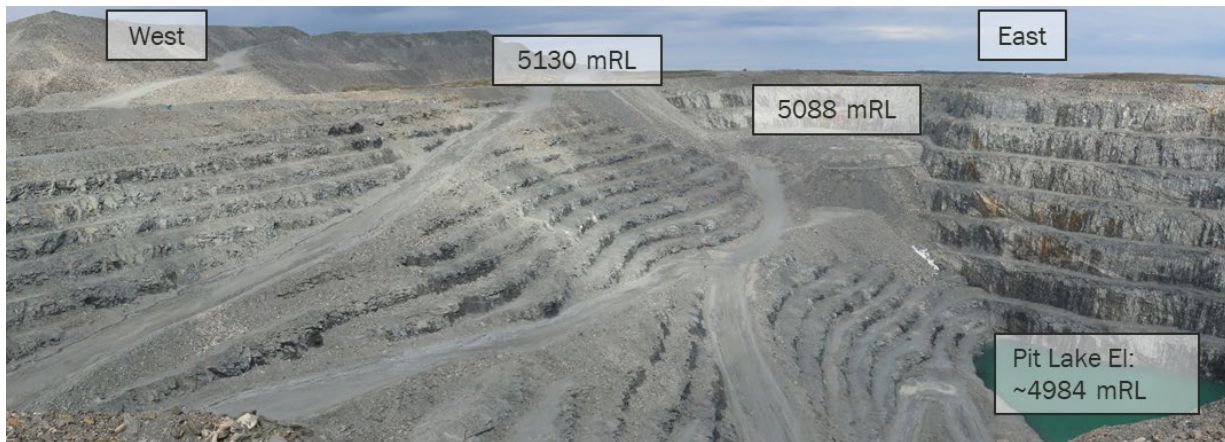
Photograph 8-5: Vault Pit west wall looking north (2019)
