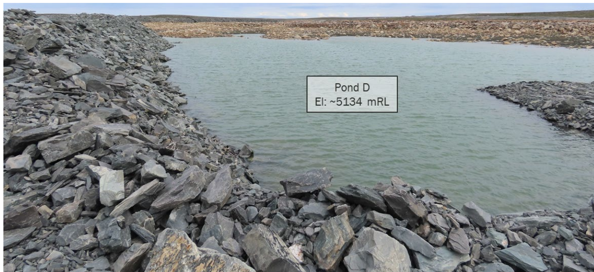
Photograph 8-3: Pond D attenuation storage (2019)
