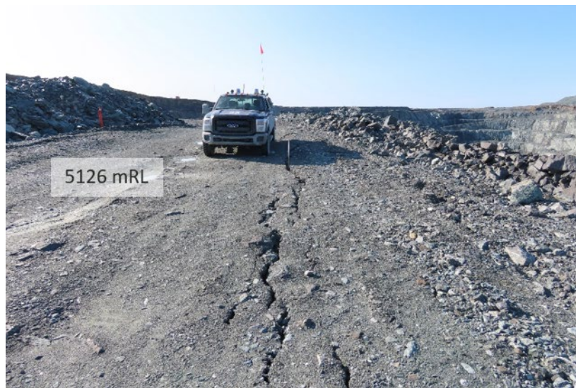
Photograph 5-6: Pit D Dump 5126 platform above haul road
