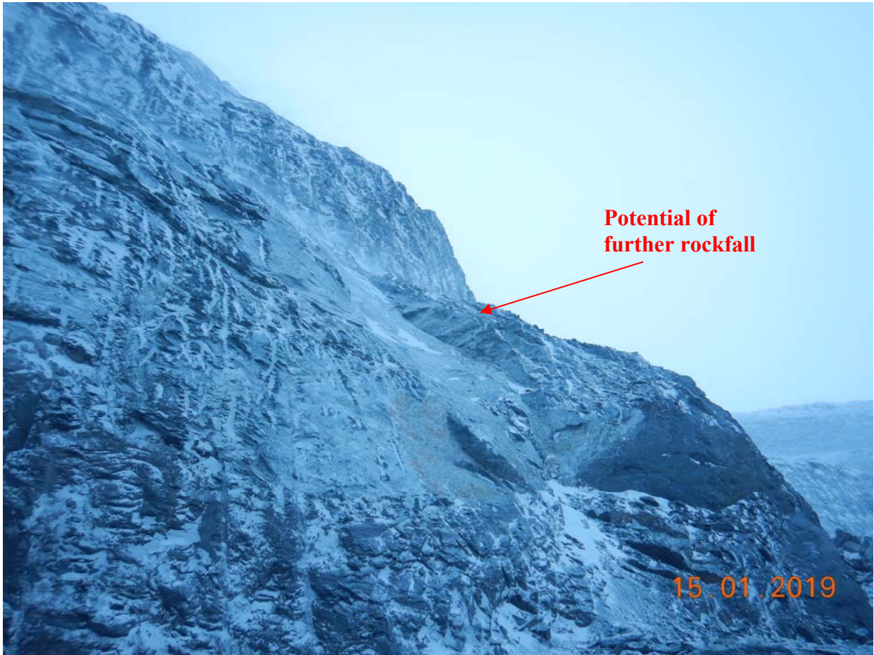
Fig.2: Photo showing potential of further material becoming loose.
