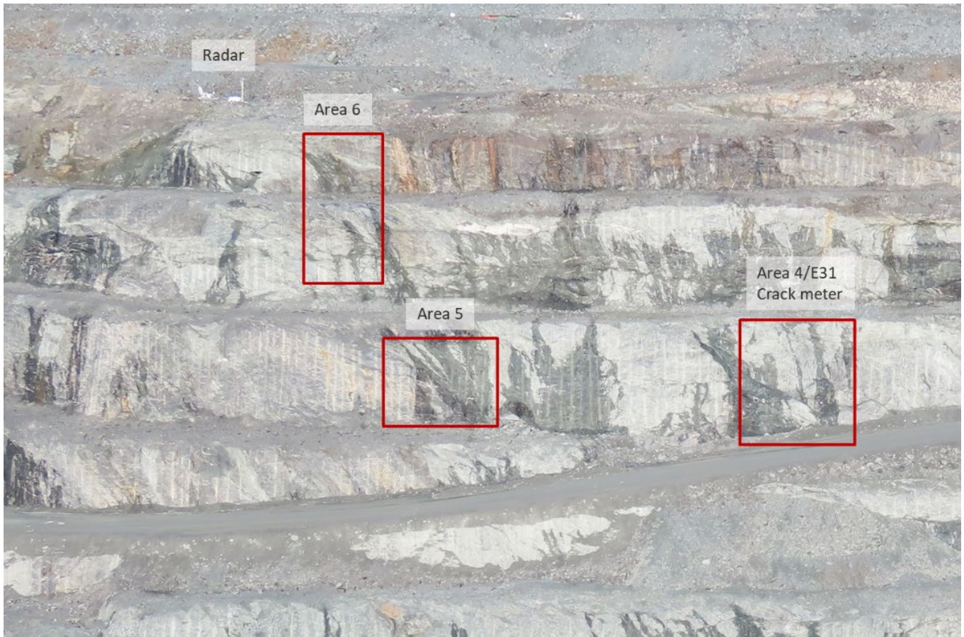
Photograph 6-18: Pit E Ramp Areas 4,5, and 6 (2019)
