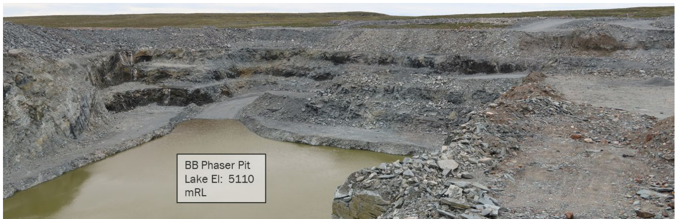
Photograph 8-21: BB Phaser Pit south through east highwall showing south end wall and west footwall slope performance (2019)
