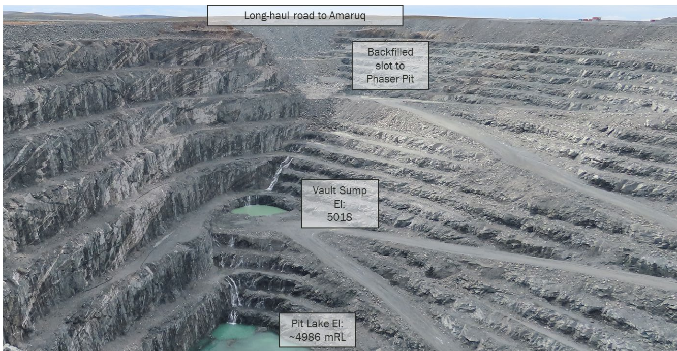
Photograph 8-7: Vault Pit grid south wall (2019) and backfilled slot cut to Phaser Pit
