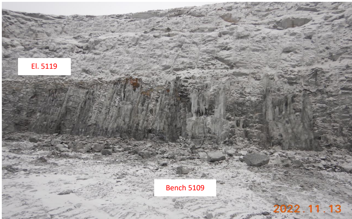
Photo 7: Whale Tail Pit P3, looking south-southwest; water flowing from a fault or brittle structure (November 13, 2022).
