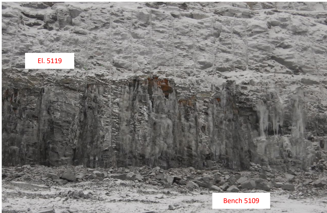
Photo 8: Whale Tail Pit P3, looking south-southwest; water flowing from a fault or brittle structure (November 13, 2022).
