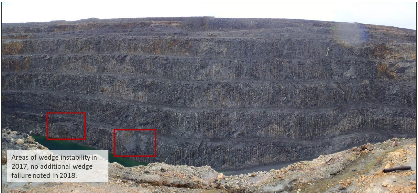
Photograph 4-10: Pit A east wall, north end additional wedges (2018)
