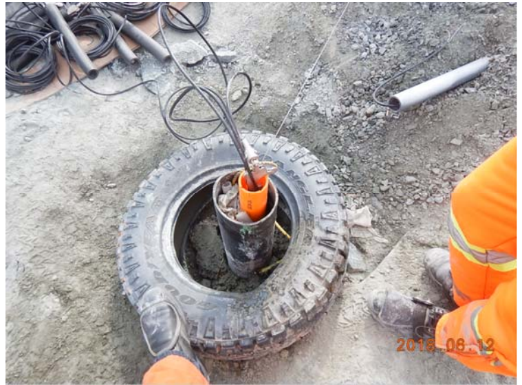
Photo 3.6: Connecting tube gently slid down the casing.
