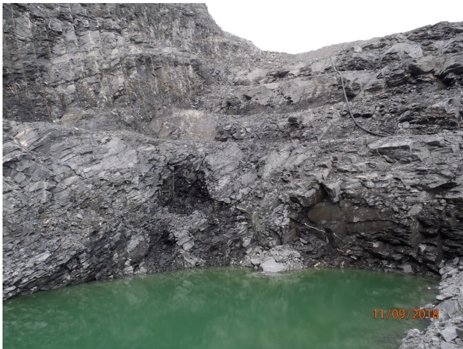
Photograph 8-5: Vault Pit south ramp sump and out dipping planes
