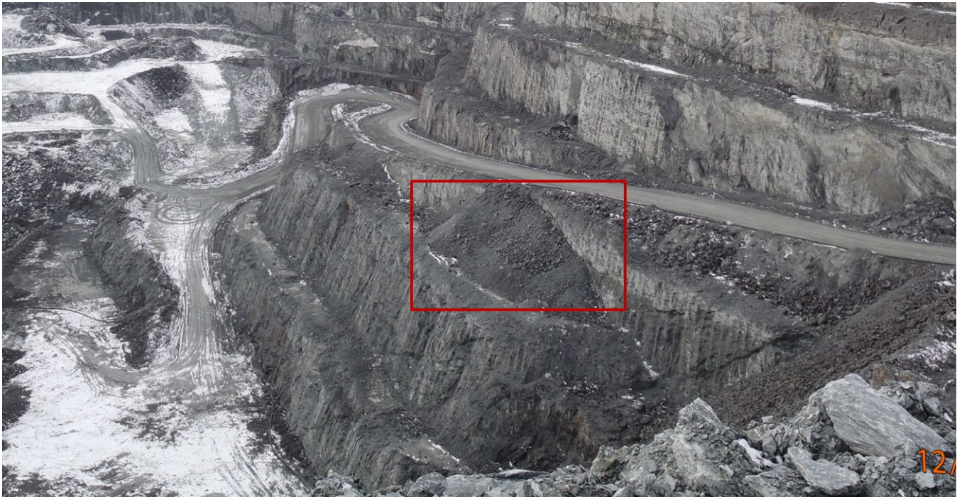
Photograph 6-23: Pit E west wall ramp buttress and step-in (2018)
