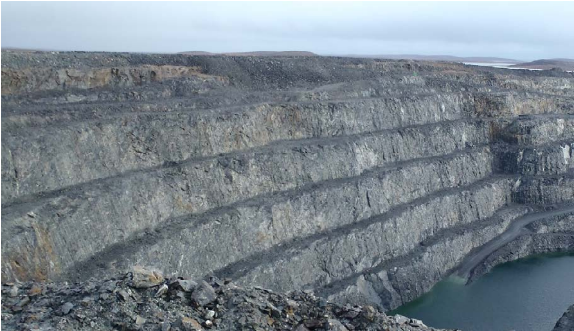
Photograph 4-9: Pit A East wall upper benches (2018)
