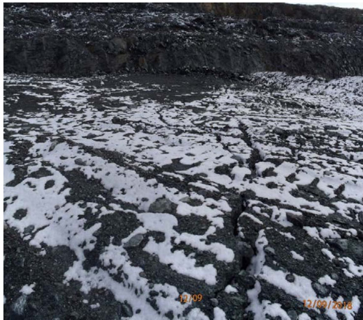
Photograph 5-5: D Dump transverse tension cracks
