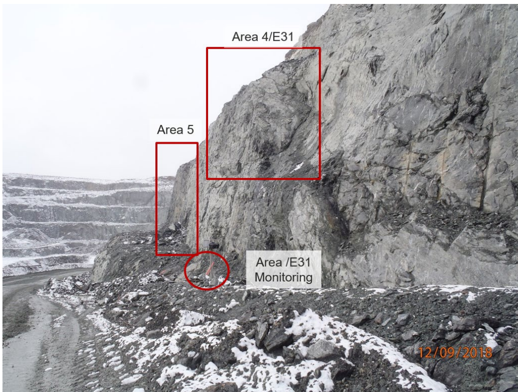
Photograph 6-21: Area 4/Zone E31 crack meter monitoring
