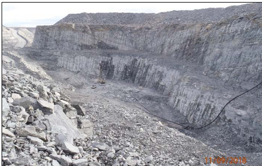
Photograph 8-14: Phaser Pit east-southeast highwall performance (2018)
