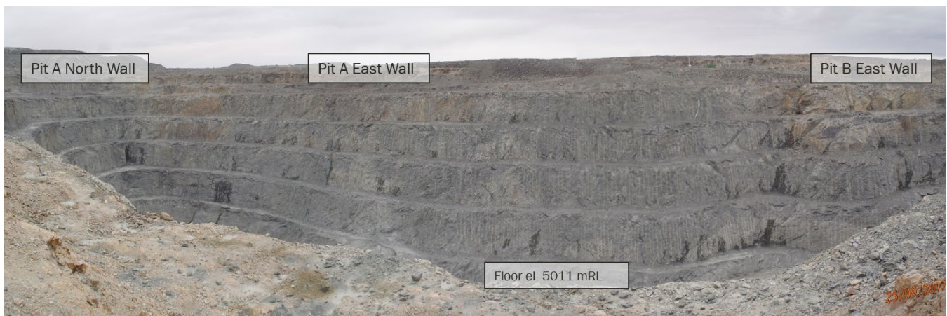
Photograph 4-2: Pits A and B looking north from west crest (2018)
