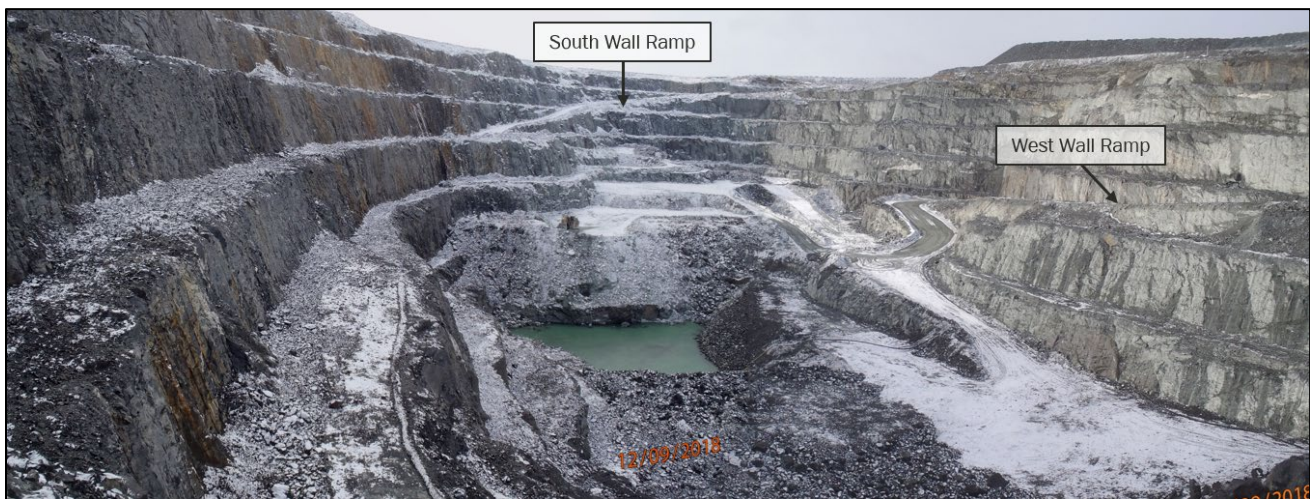
Photograph 6-2: Pit E viewing south (2017)
