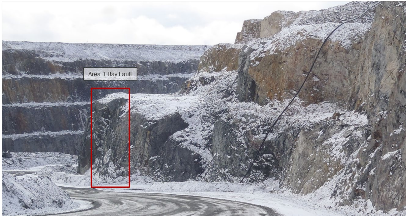
Photograph 6-16: Pit E Ramp Area 1 above ramp - Bay Fault or splay (2018)
