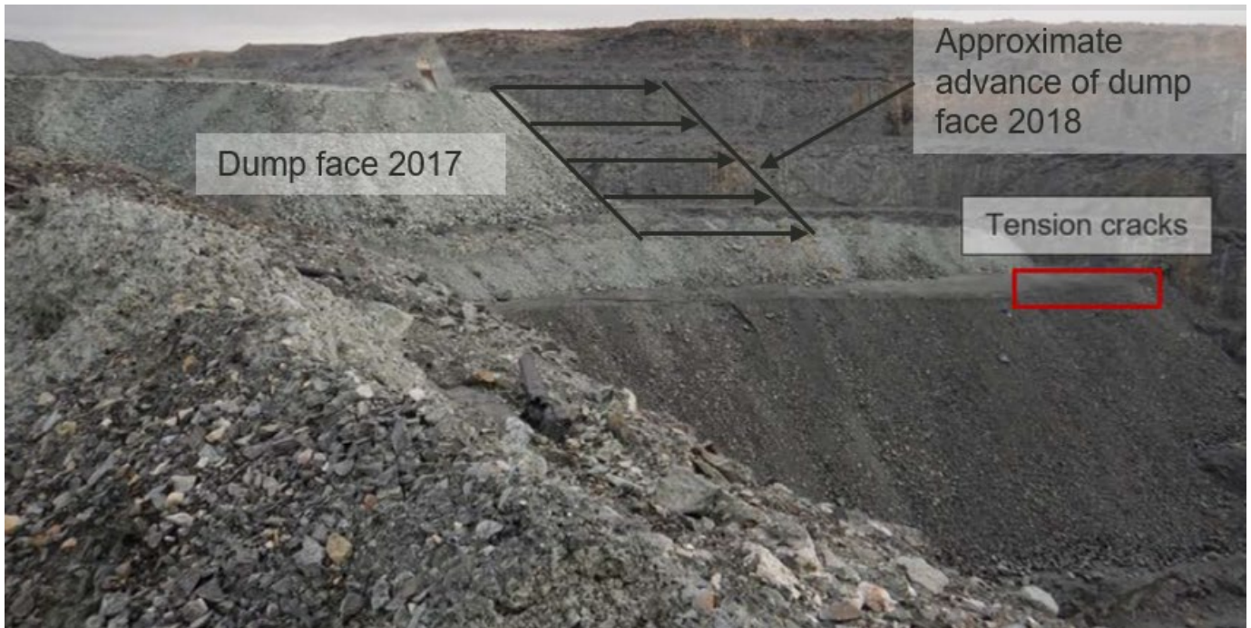
Photograph 5-2: Pit D dump showing 2017 dump face and approximate advance 2018 dump face location
