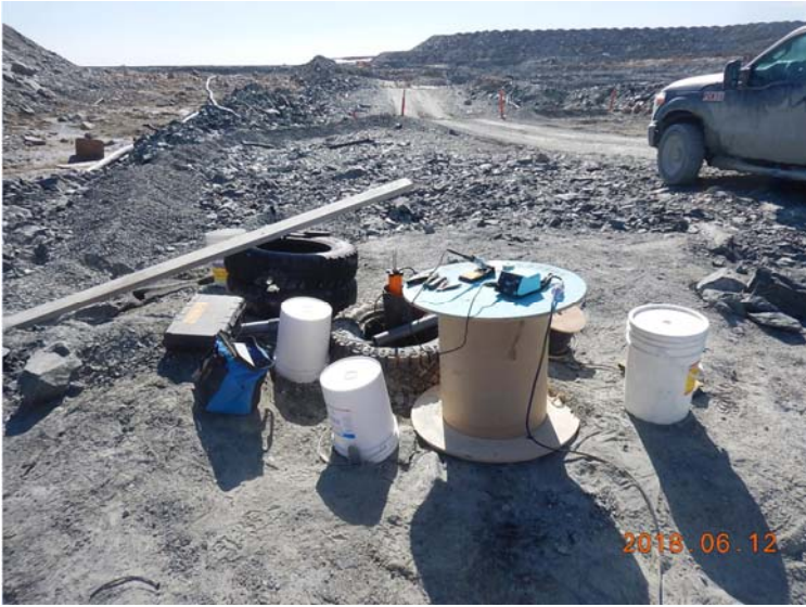
Photo 3.8: Preparation and set-up for the cable splicing
