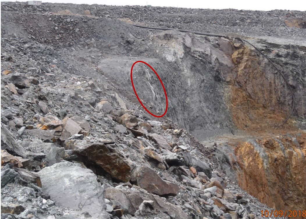
Photograph 7-11: Goose Pit uncontrolled water discharge on north pit wall
