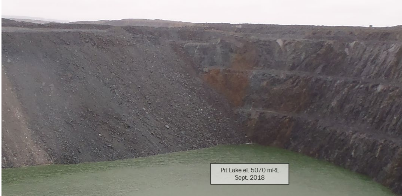
Photograph 7-9: Goose Pit northwest through northeast wall (north end wall 2018)
