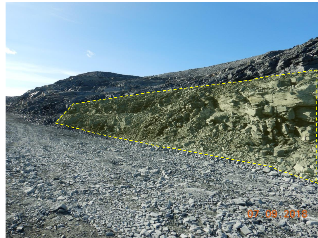
Zone P30: Phaser, West Wall: Lightly scale the wall.
