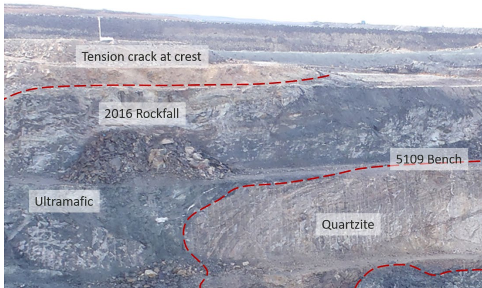
Photograph 4-5: Pit A West Wall 2016 rock fall and tension cracks (2018)
