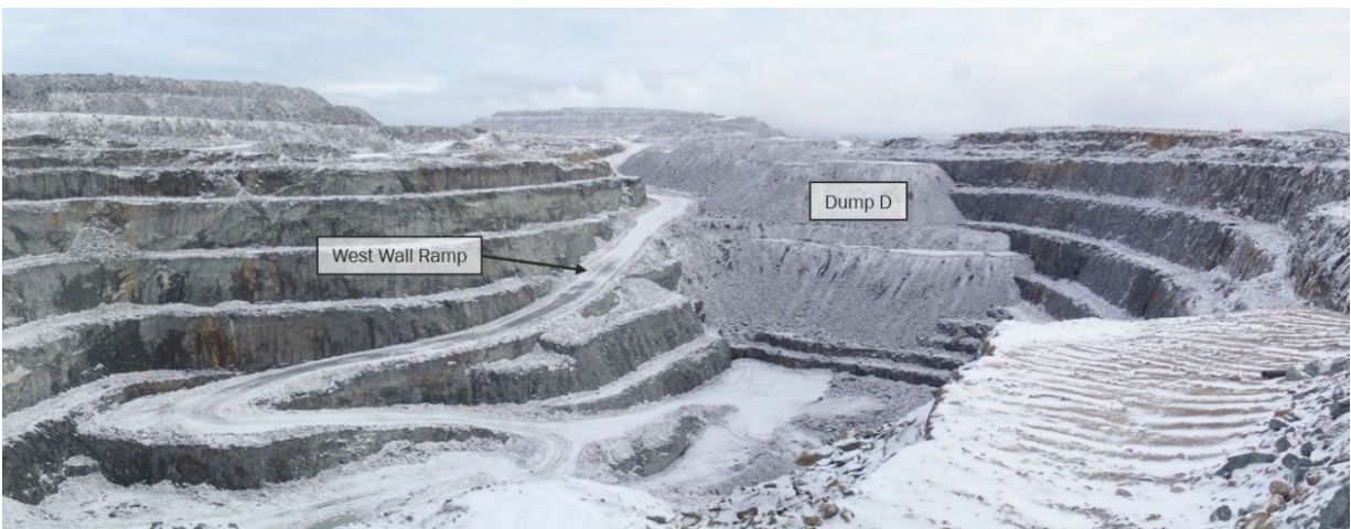
Photograph 6-1: Pit E viewing north (2018)
