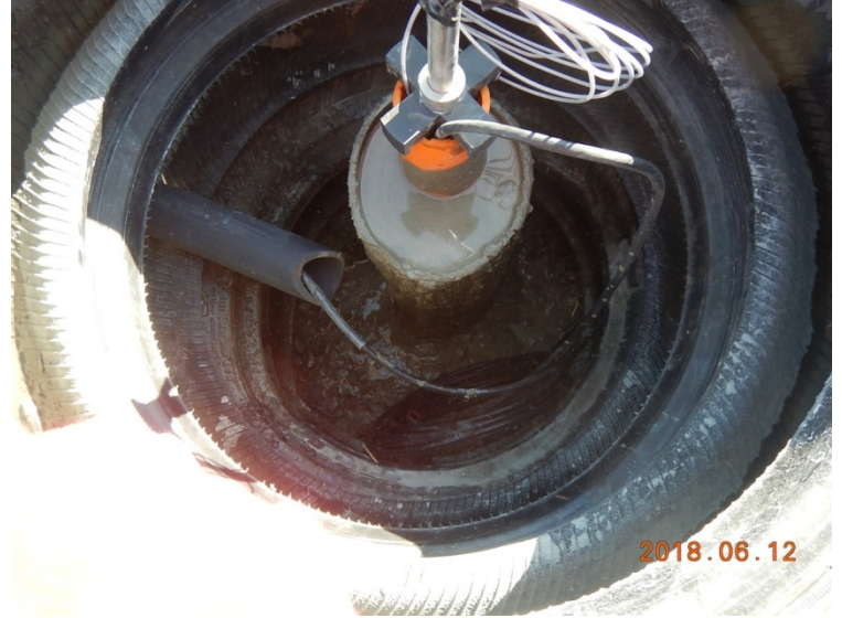
Photo 3.9: Grout added around the top of the casing to stabilize it
