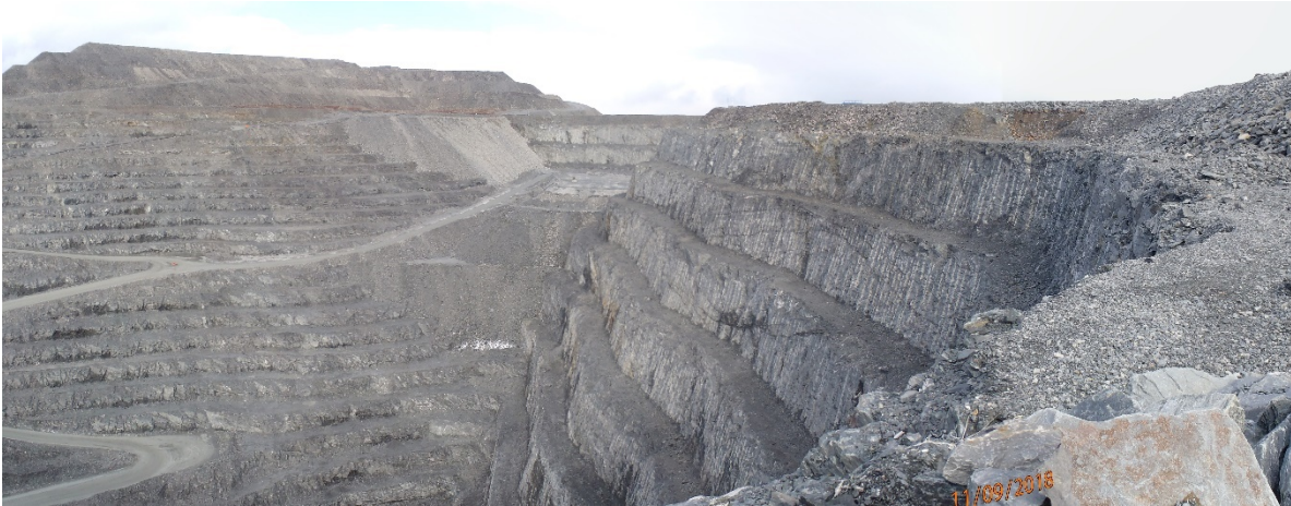
Photograph 8-7: Vault Pit east highwall bench performance, southeast end looking north (2018)
