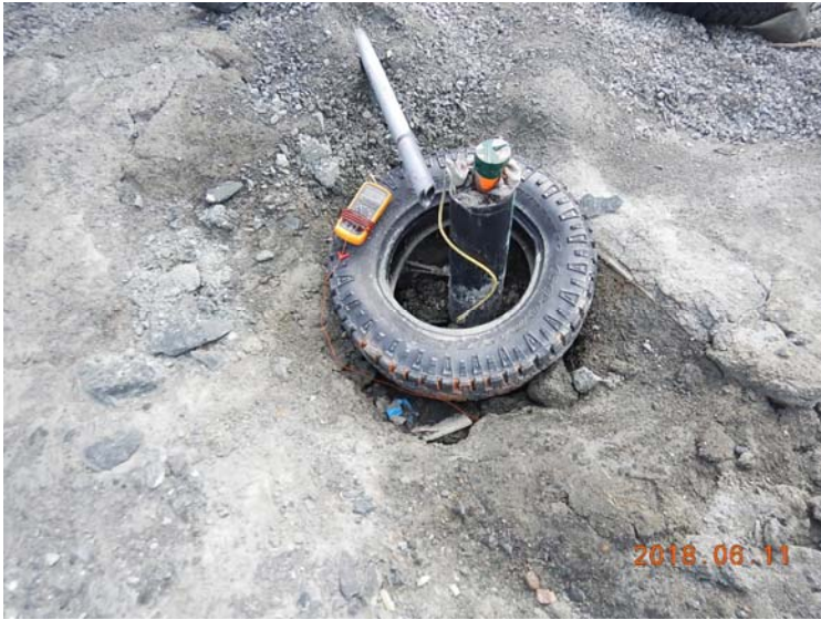
Photo 3.1 : Casing and PVC pipe before the re-installation of the IPI
