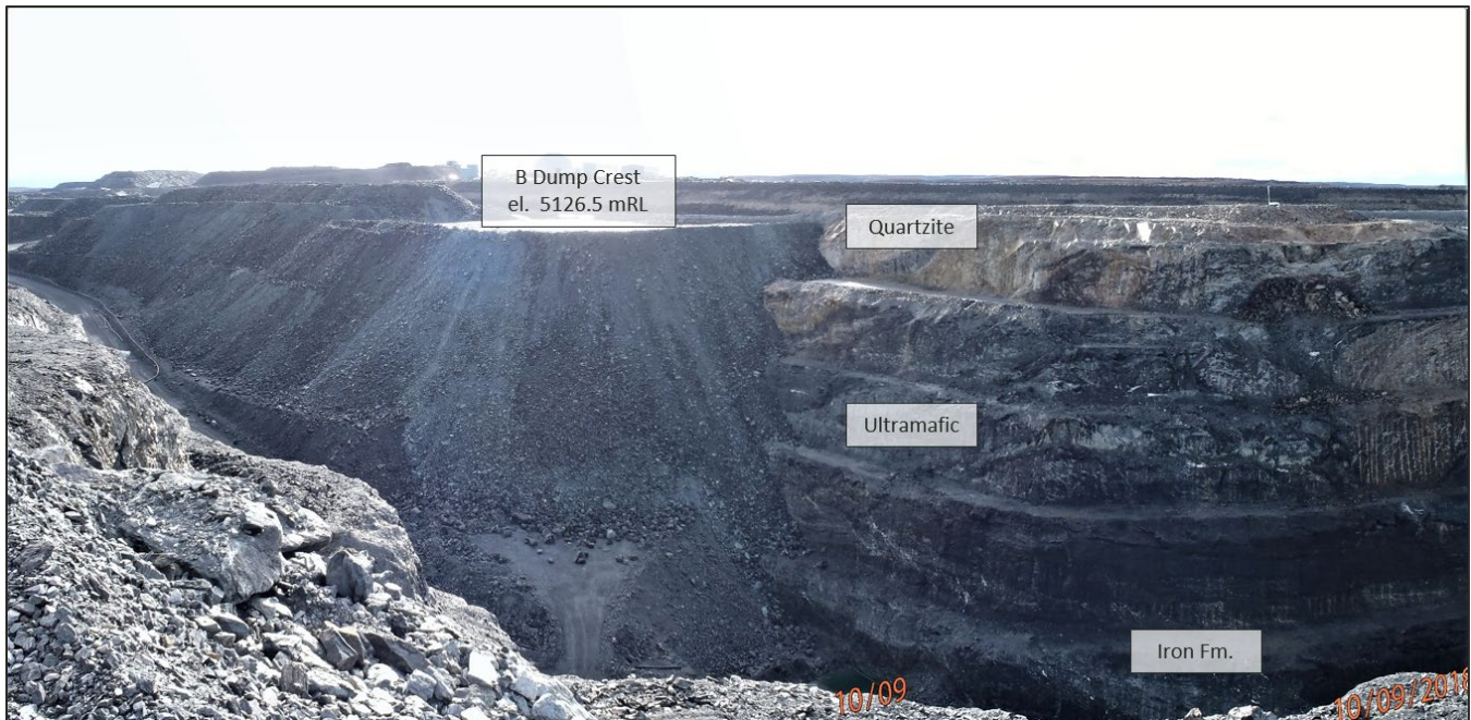
Photograph 4-11: Pit B west wall
