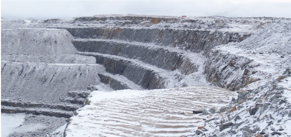
Photograph 6-3: Pit E east wall performance (2018)
