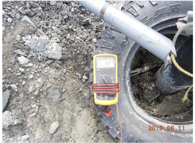
Photo 3.2 : Temperature monitored during installation
