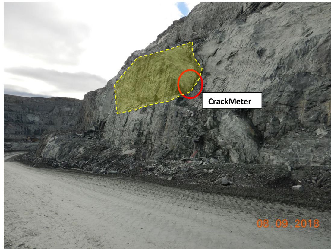
Zone E31: E3 Ramp, West Wall: Perform monitoring with crack meter.
