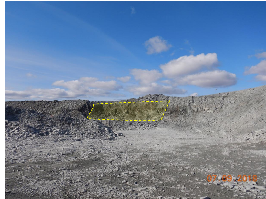
Zone BB05: BB Phaser, West Wall: Thermal capping is required on the section.
