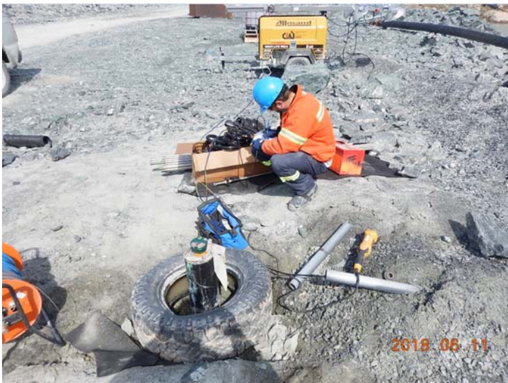
Photo 3.3: Preparation for the installation of the instrument and equipment
