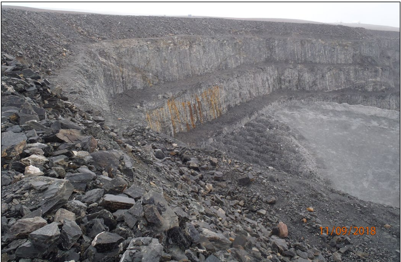
Photograph 8-11: Vault Pit northeast wall bench performance (2018) and dump platform
