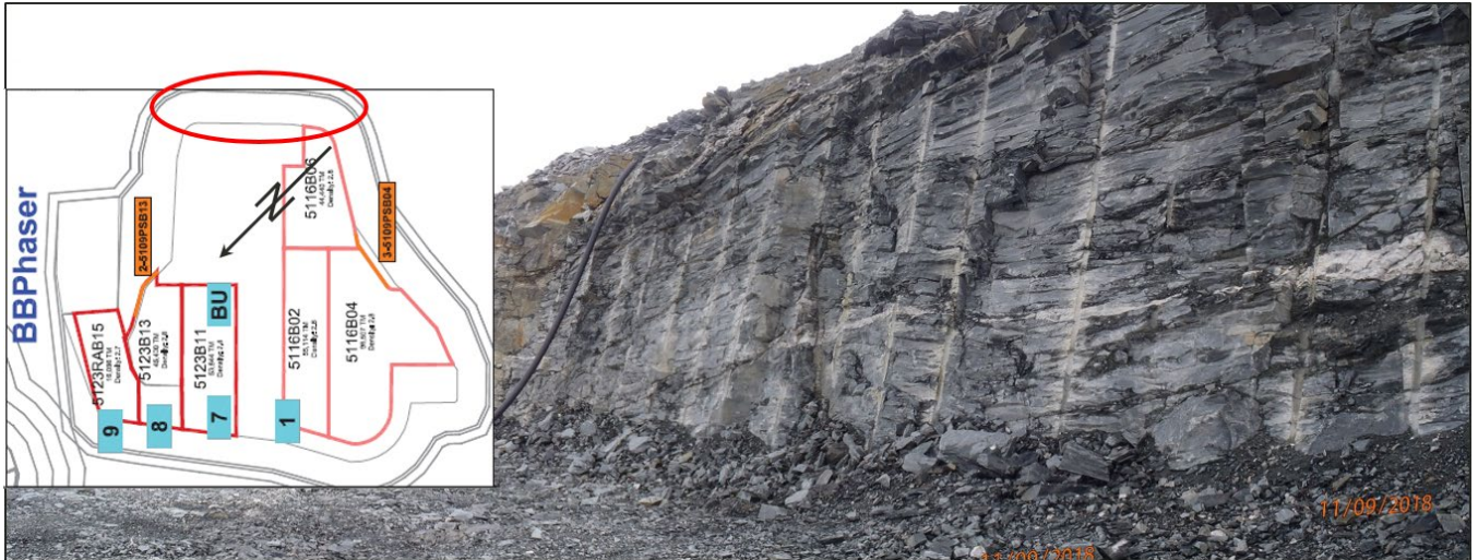
Photograph 8-20: BB Phaser Pit south through east highwall showing good performance
