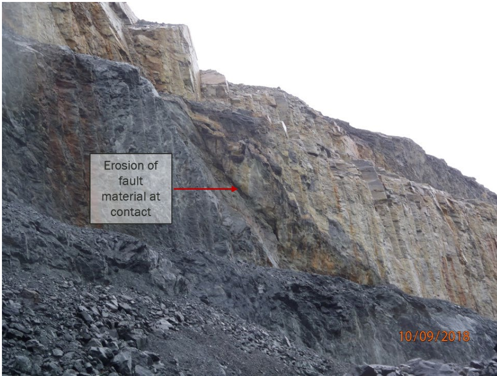
Photograph 7-3: Erosion of faulted contact Goose Pit south wall (2018)
