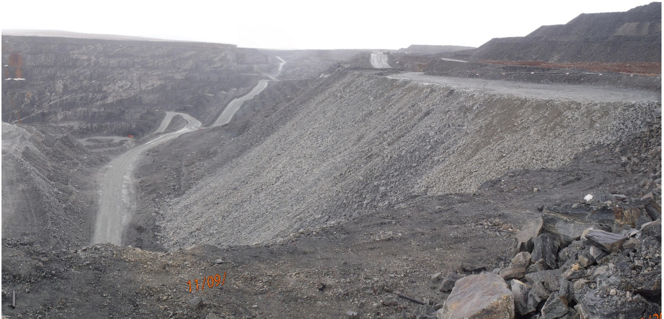
Photograph 8-2: Vault Pit west wall looking south (2018) showing dump advance
