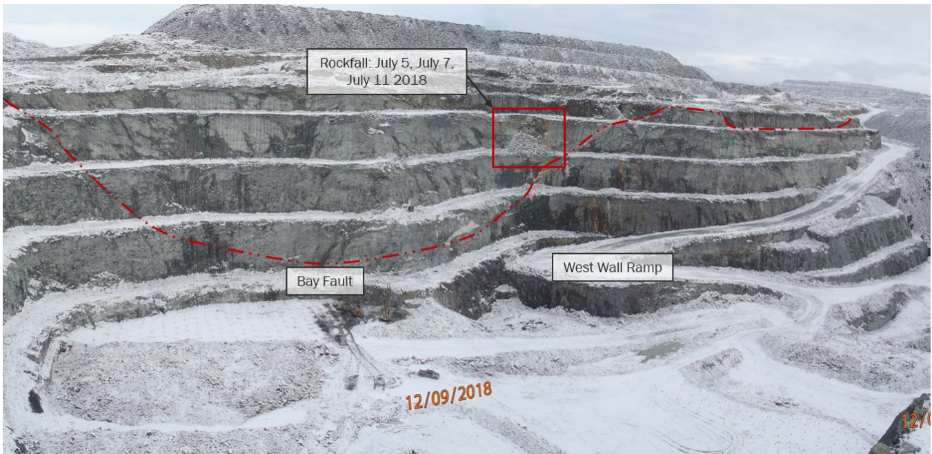
Photograph 6-11: Pit E west wall showing seepage and Bay Fault (2018)
