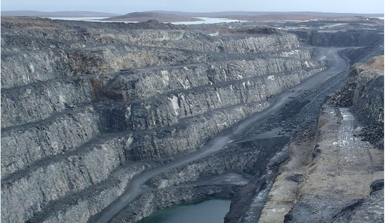
Photograph 4-12: Pit B east wall, looking south (2018)
