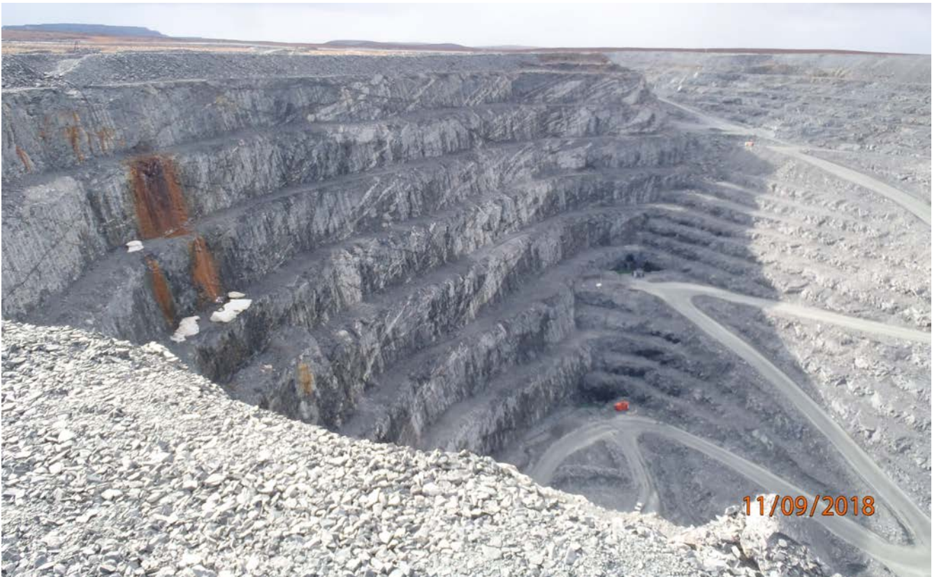
Photograph 8-8: Vault Pit east wall northeast end looking south (2018)
