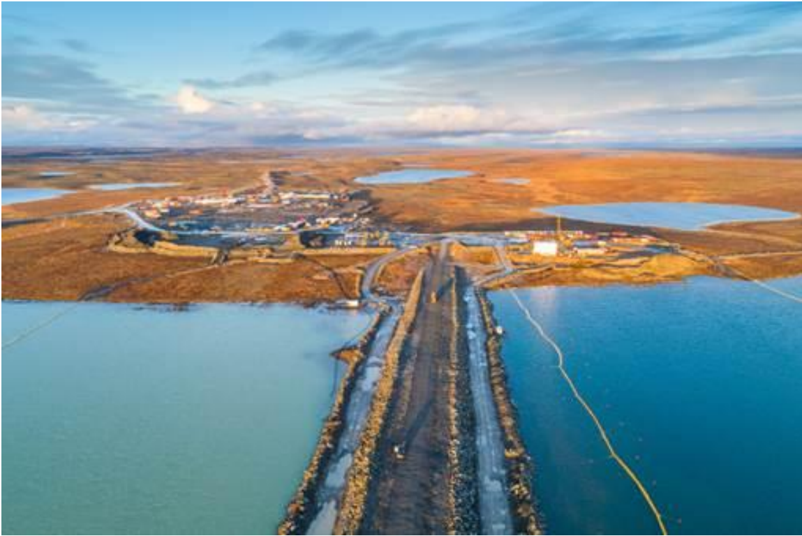
Figure A- 4. Whale Tail dike construction, 2018 (looking east).
