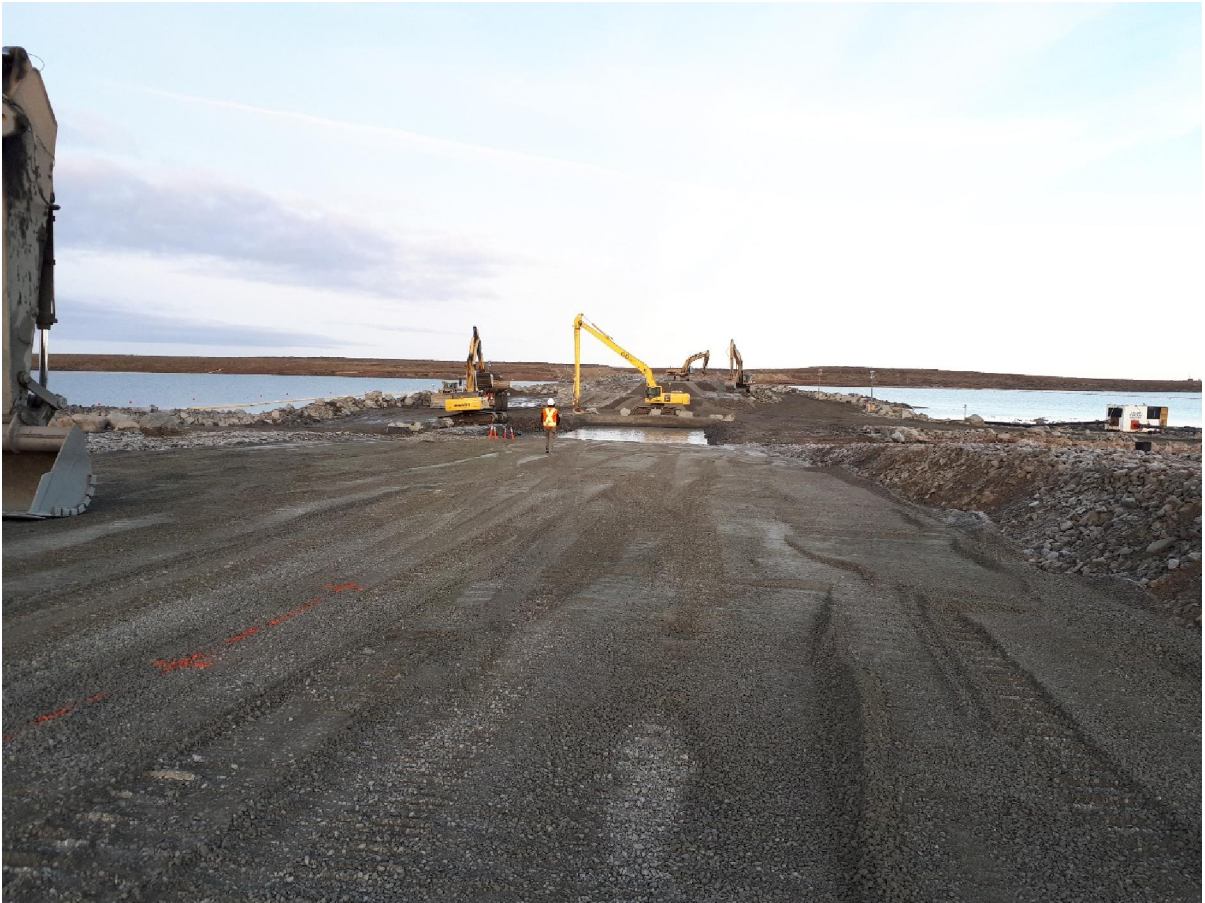
Figure A- 3. Whale Tail dike construction, August 26, 2018.
