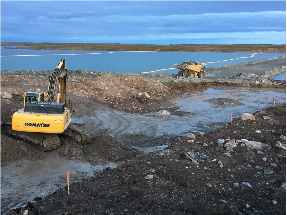
Figure A- 2. Whale Tail dike construction, July 31, 2018 (looking west).
