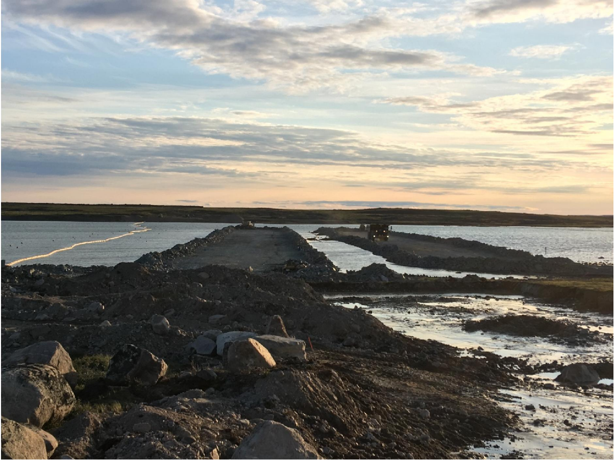
Figure A- 1. Whale Tail dike construction, July 30, 2018.
