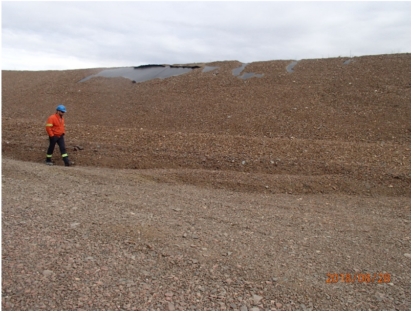
Photograph G1-21 Baker Lake Tank Farm
