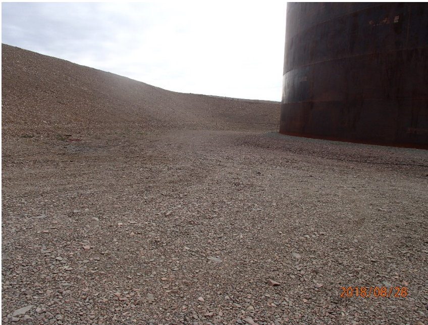
Photograph G1-19 Baker Lake Tank Farm
