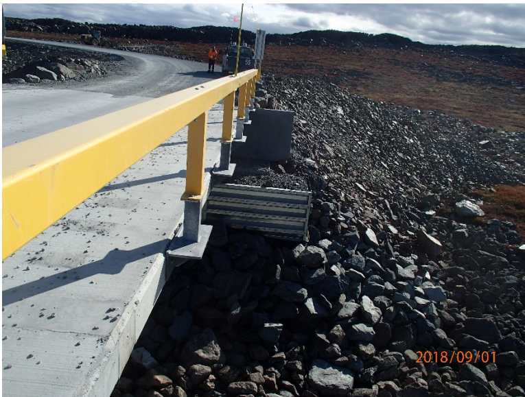
Photograph E2-8 Bridges 2 – km 10+700
