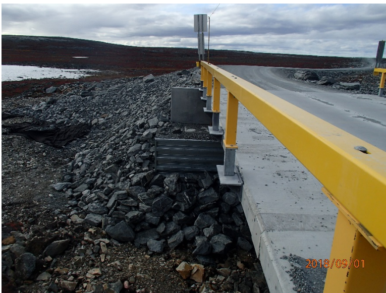
Photograph E2-2 Bridges 1 – km 3+400
