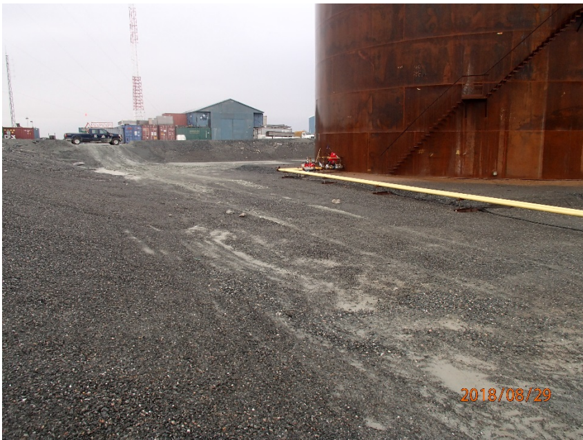
Photograph G2-6 Meadowbank Tank Farm
