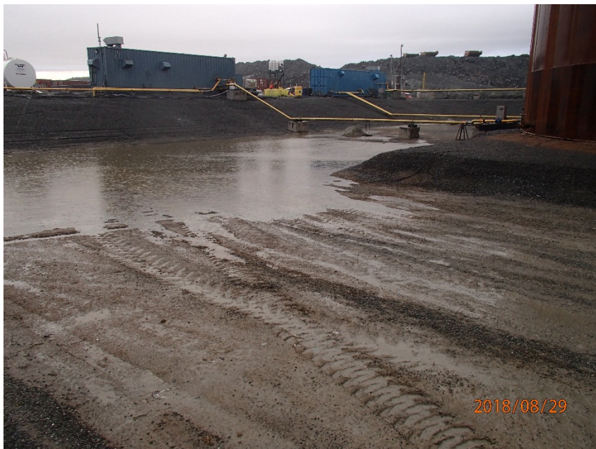
Photograph G2-4 Meadowbank Tank Farm
