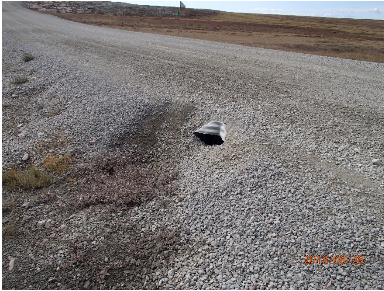
Photograph D1-1: unnamed km 5+700
