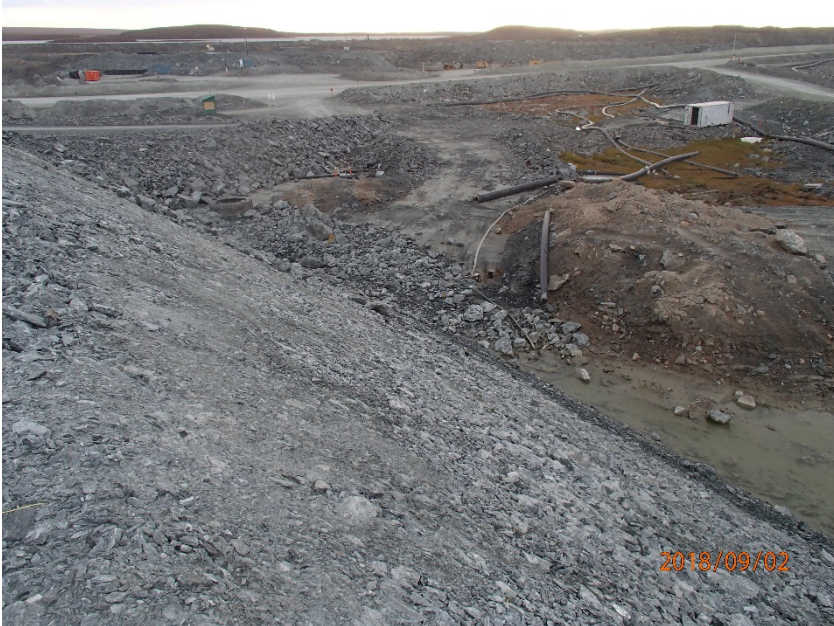
Photograph B7-15 Central Dike and Saddle Dam 5
