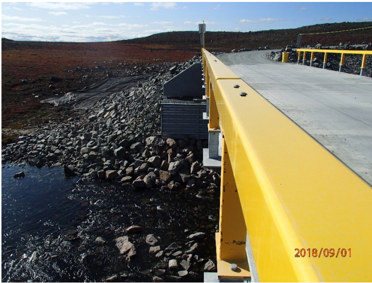
Photograph E2-25 Bridges 7 – km 32+300
