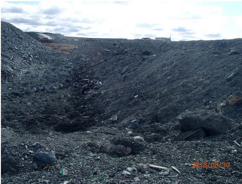
Photograph A2-5 South Camp Dike
