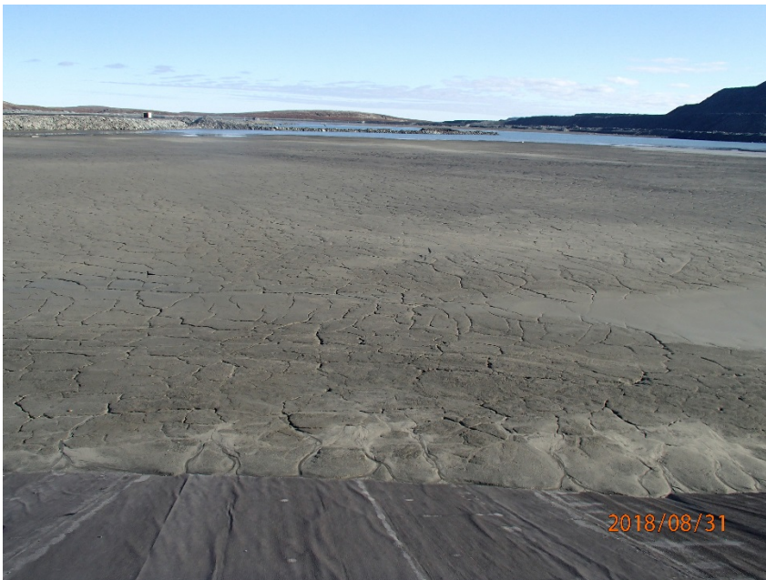
Photograph B4-12 Stormwater Dike
