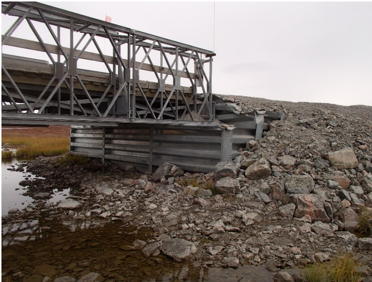
Photograph D2-3 Bridges 2 – R05 km 17+600
