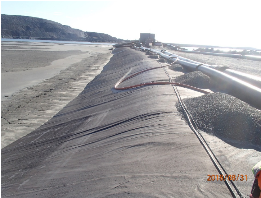
Photograph B4-11 Stormwater Dike
