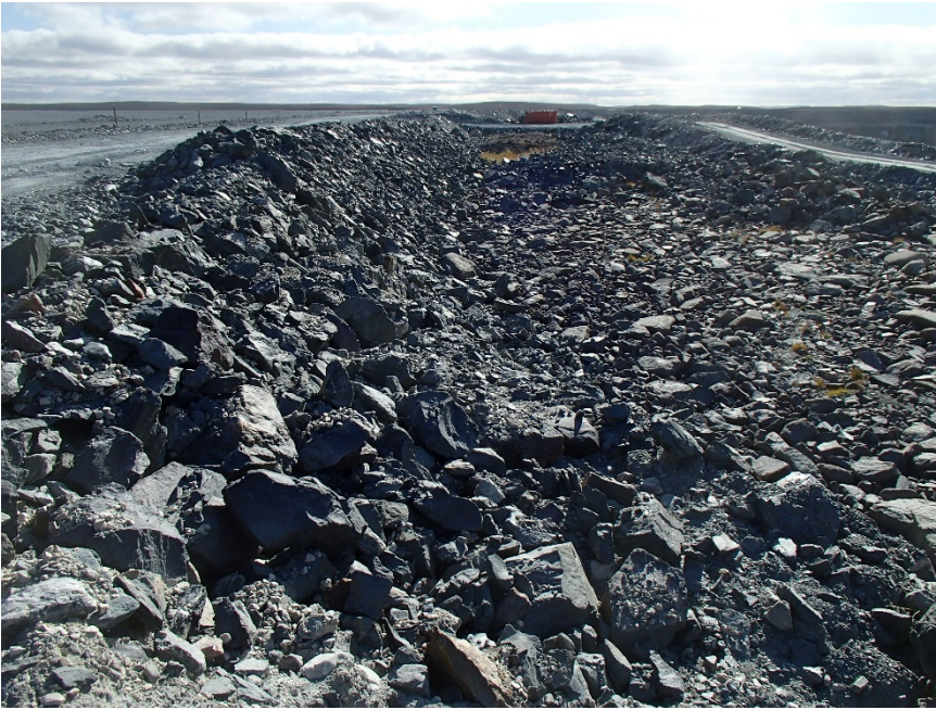
Photograph A3-15 Bay Goose Dike
