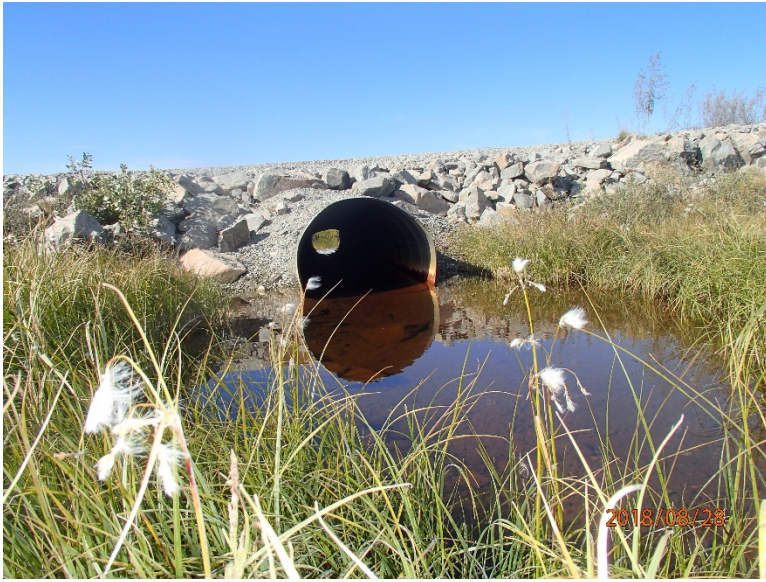
Photograph D1-9: R-05A km 15+745
