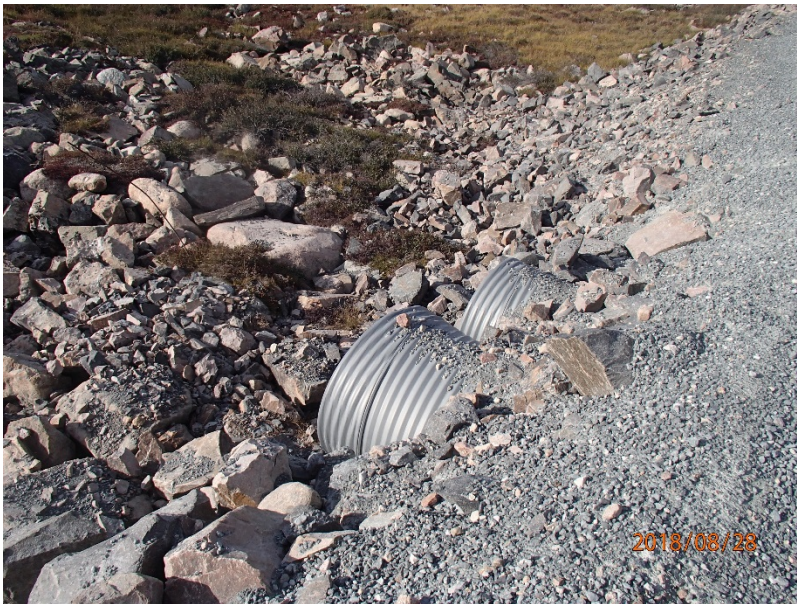
Photograph D1-24: R-24 km 98+100
