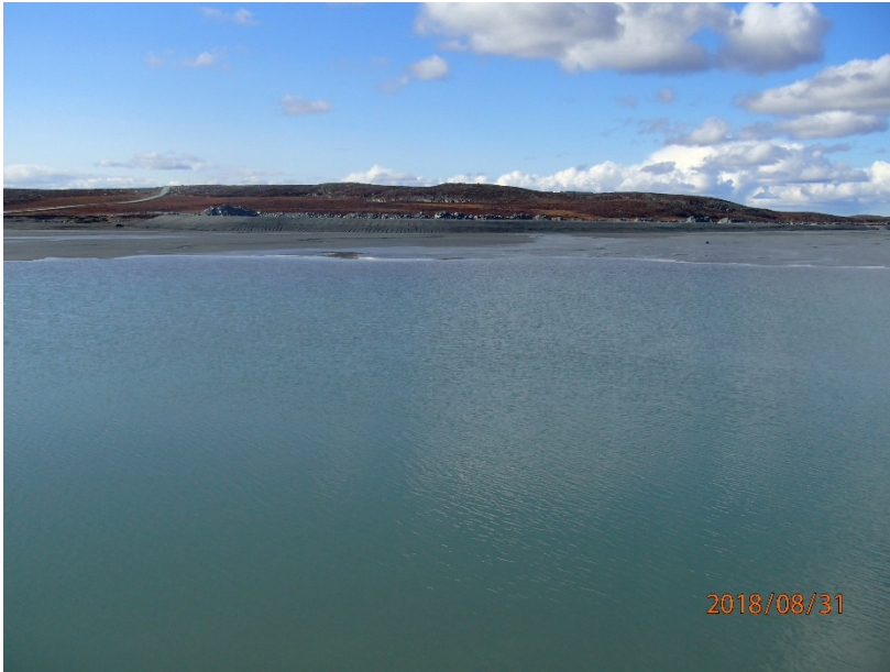
Photograph B1-9 Tailings Storage Facility
