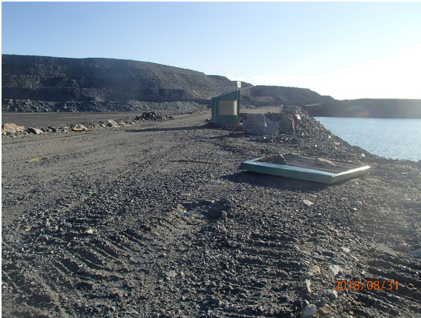
Photograph B4-3 Stormwater Dike
