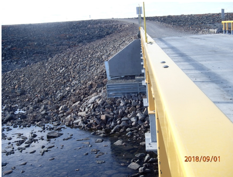
Photograph E2-17 Bridges 5 – km 23+900
