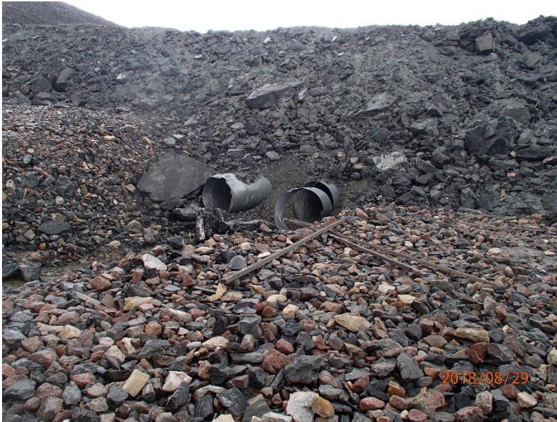
Photograph H1-5 Vault Road Culverts
