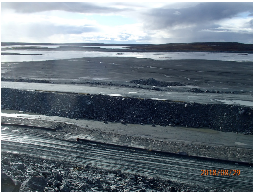
Photograph B1-19 Tailings Storage Facility
