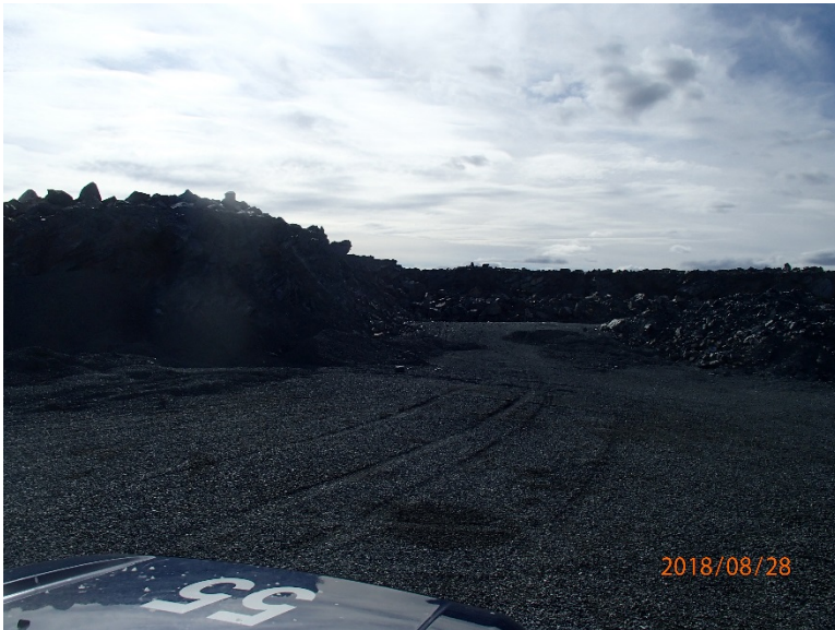
Photograph F1-11: Quarry 8 – km 42+950
