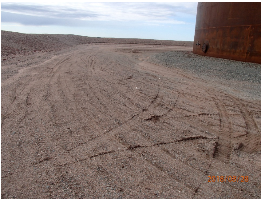
Photograph G1-12 Baker Lake Tank Farm
