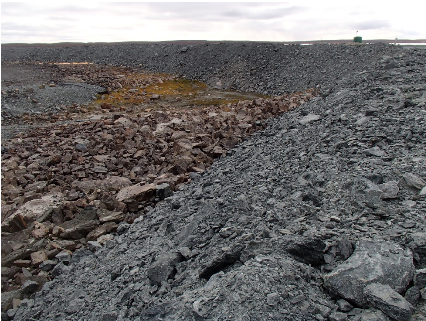
Photograph A3-34 Bay Goose Dike
