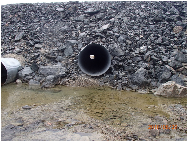
Photograph H1-4 Vault Road Culverts
