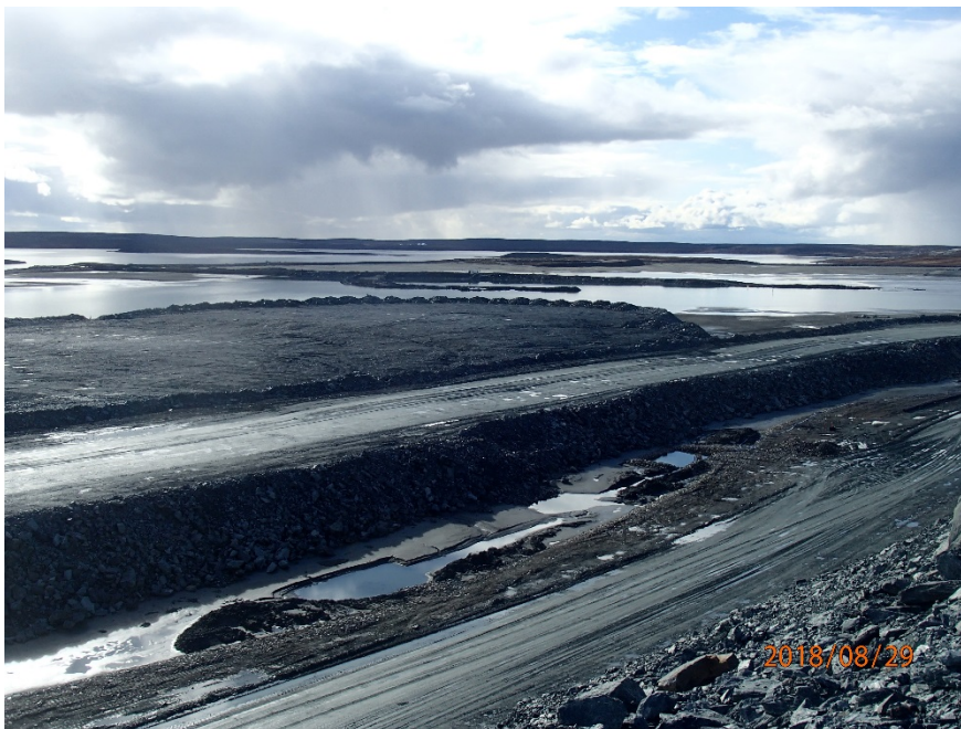
Photograph B1-12 Tailings Storage Facility
