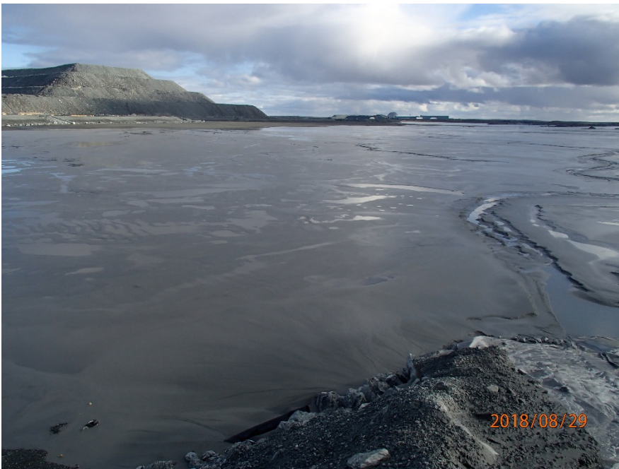
Photograph B1-17 Tailings Storage Facility
