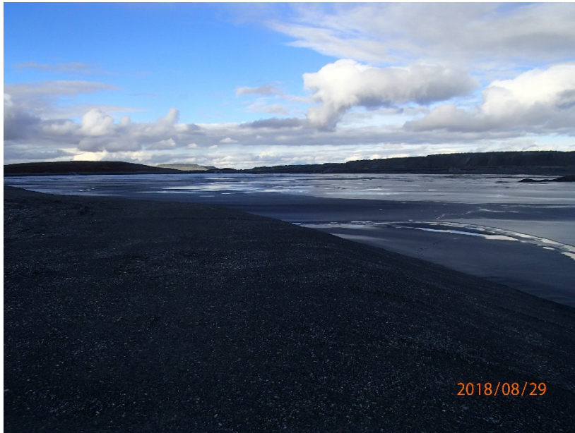
Photograph B1-5 Tailings Storage Facility
