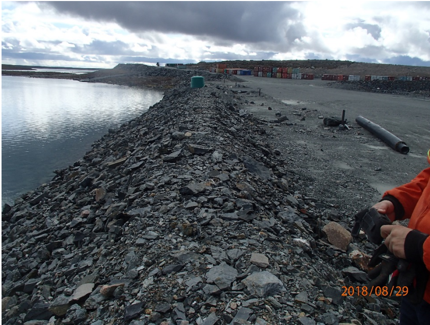
Photograph A1-9 East Dike
