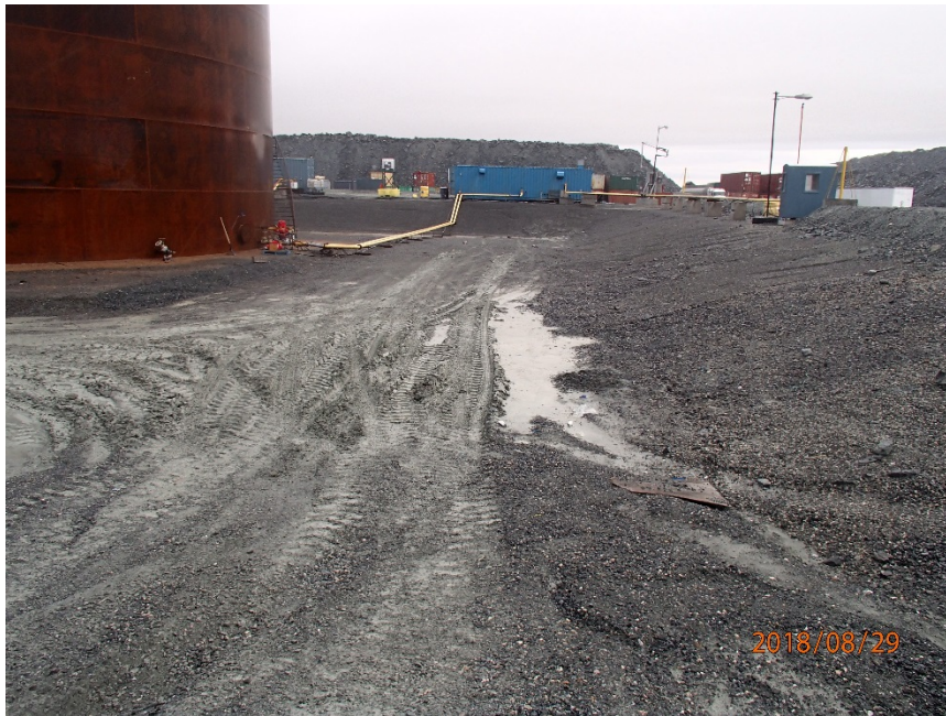
Photograph G2-1 Meadowbank Tank Farm
