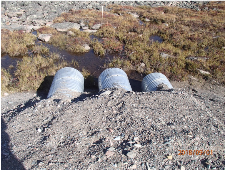
Photograph E1-3: Culverts #208, #209 and #210, km 49+431 to 49+435
