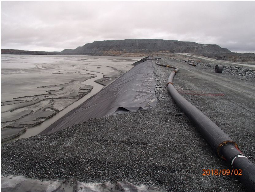
Photograph B7-9 Central Dike and Saddle Dam 5
