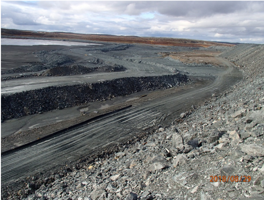
Photograph B1-20 Tailings Storage Facility
