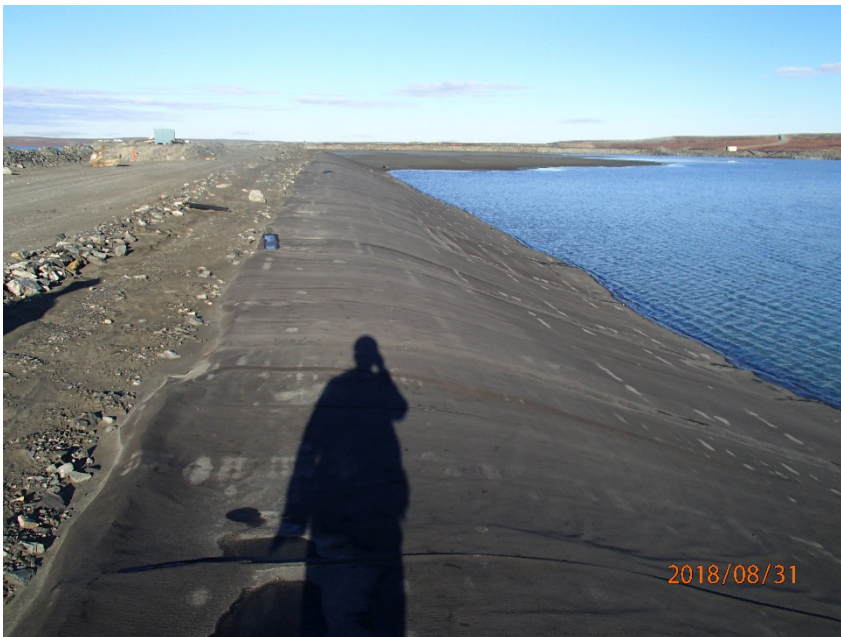
Photograph B4-16 Stormwater Dike
