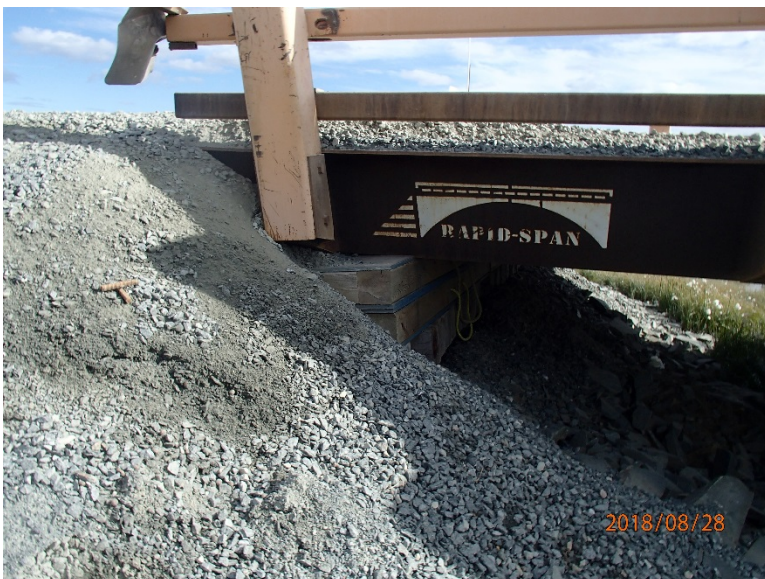
Photograph D2-8 Bridges 5 – R13 km 62+060
