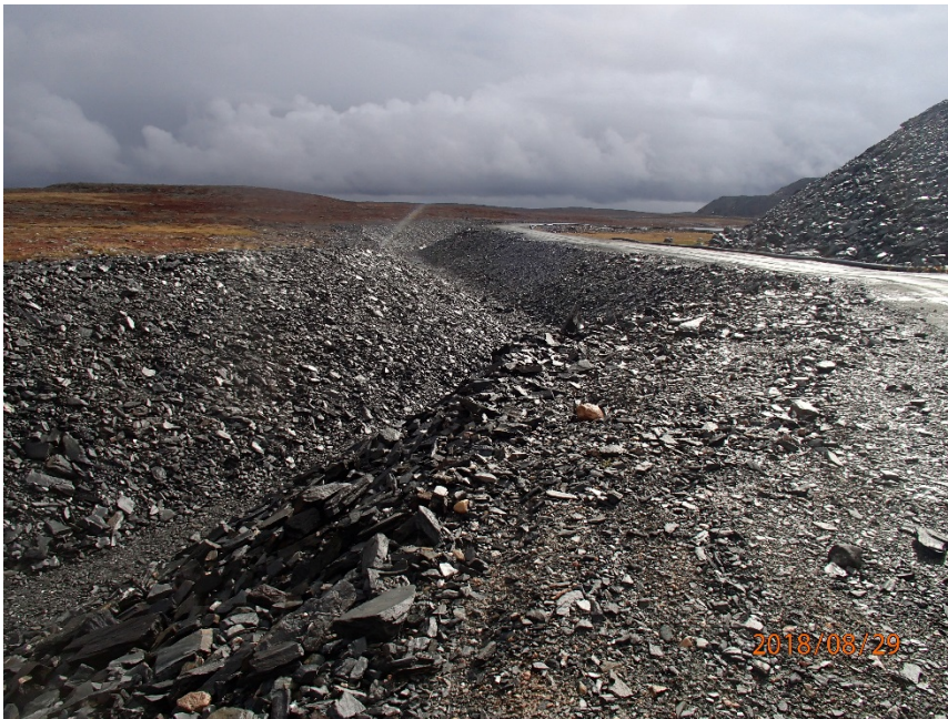
Photograph H2-5 Diversion Ditch and its Sediment and Erosion Protection Structure
