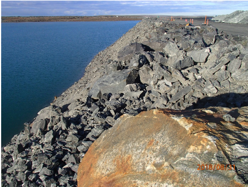
Photograph B4-7 Stormwater Dike
