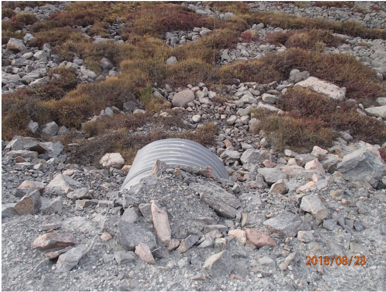
Photograph D1-15: R-17 km 77+440
