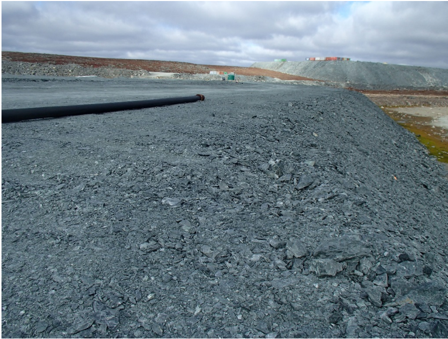
Photograph A3-39 Bay Goose Dike
