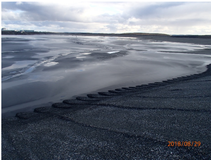
Photograph B1-6 Tailings Storage Facility
