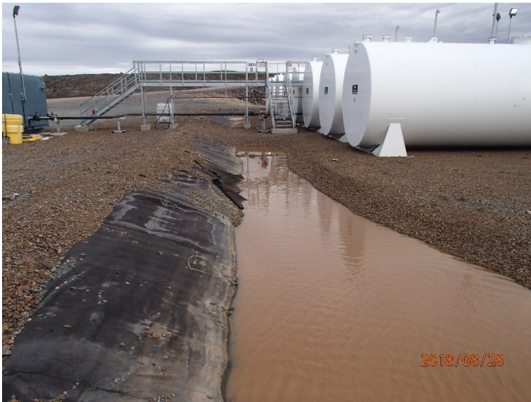
Photograph G1-25 Baker Lake Tank Farm
