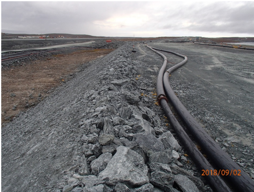
Photograph B7-16 Central Dike and Saddle Dam 5
