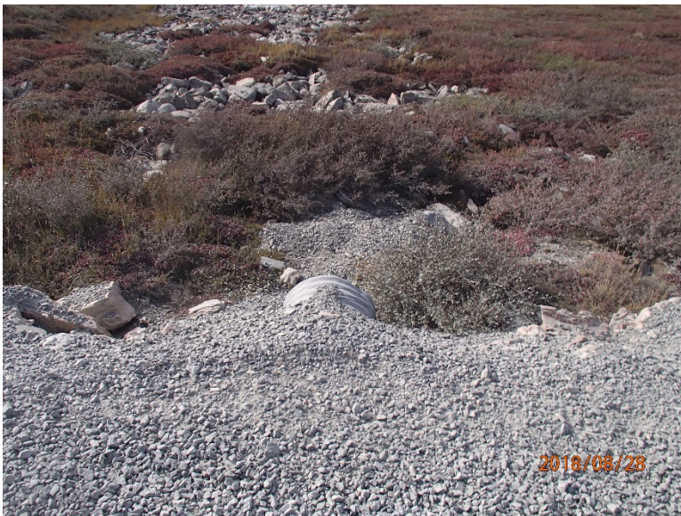
Photograph D1-12: PC-11 km 39+552
