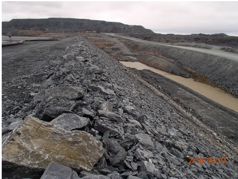
Photograph B7-6 Central Dike and Saddle Dam 5
