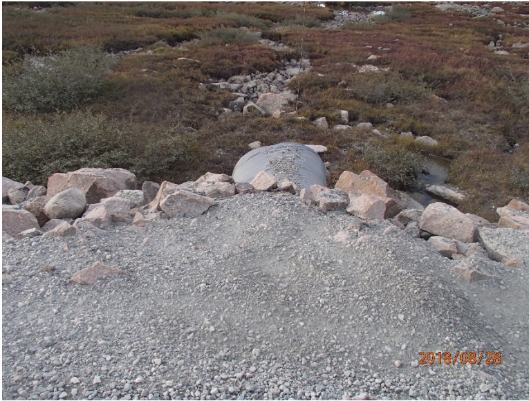
Photograph D1-23: R-23 km 93+600
