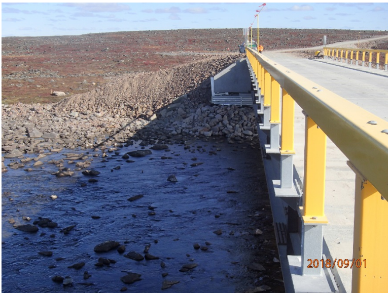
Photograph E2-20 Bridges 5 – km 23+900
