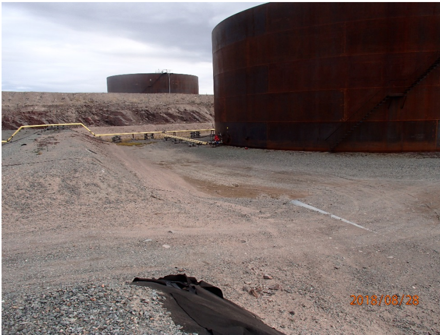
Photograph G1-7 Baker Lake Tank Farm
