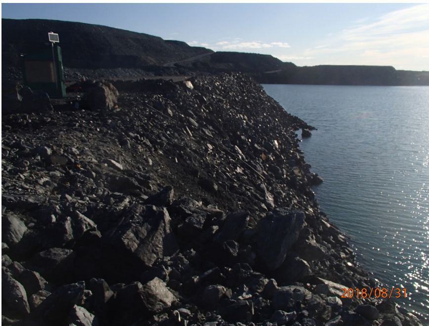
Photograph B4-6 Stormwater Dike
