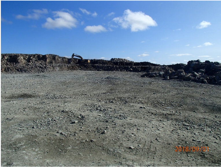
Photograph F2-5 Eskers and Quarries 3 – km 30+180
