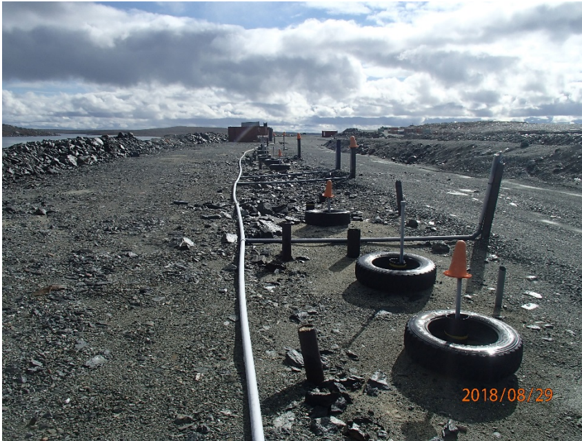
Photograph A1-5 East Dike
