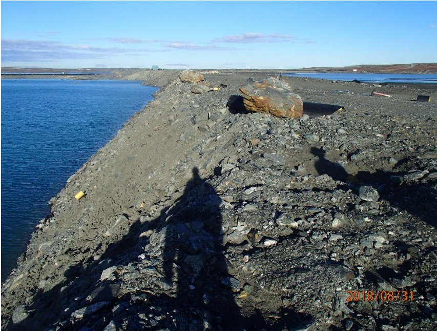
Photograph B4-5 Stormwater Dike
