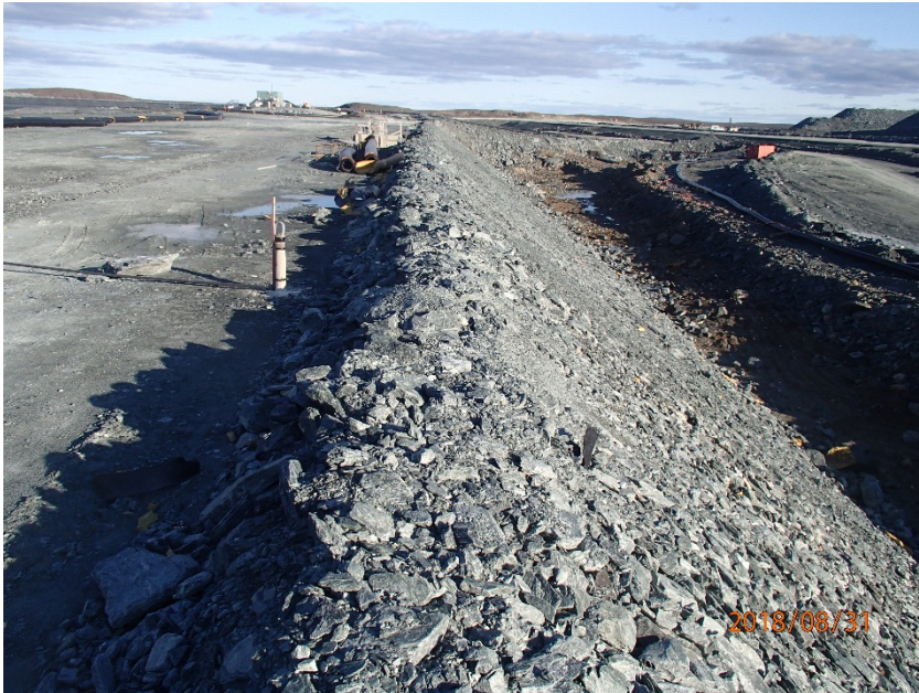
Photograph B7-17 Central Dike and Saddle Dam 5
