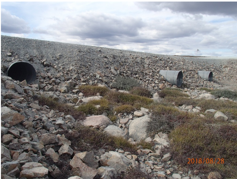
Photograph D1-14: R-14 km 67+840
