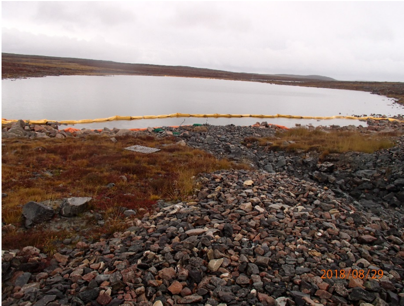
Photograph H2-1 Diversion Ditch and its Sediment and Erosion Protection Structure
