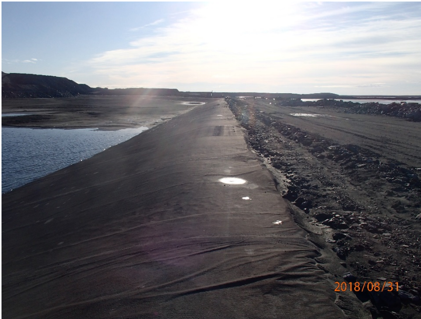
Photograph B4-15 Stormwater Dike
