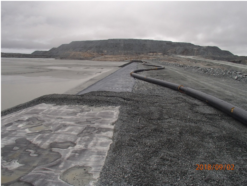
Photograph B7-2 Central Dike and Saddle Dam 5
