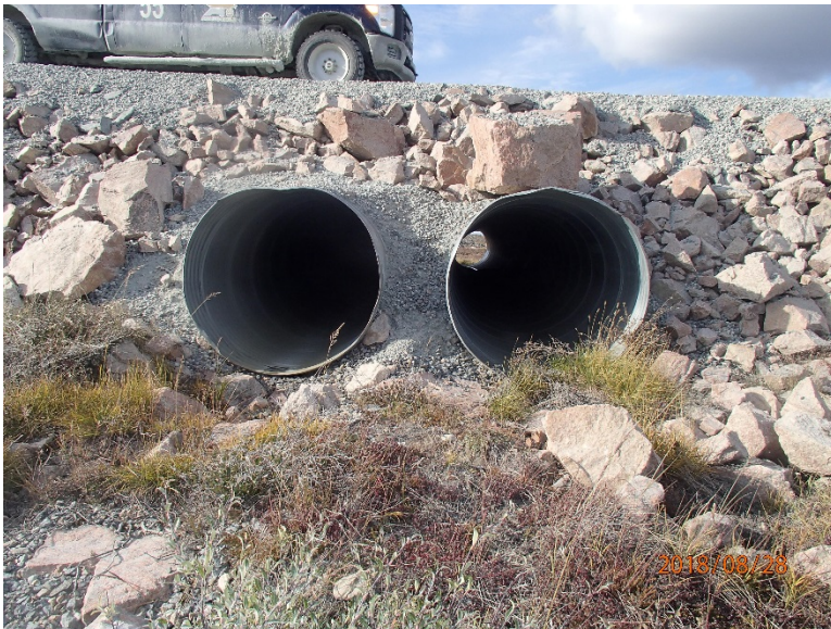
Photograph D1-20: R-21 km 87+300
