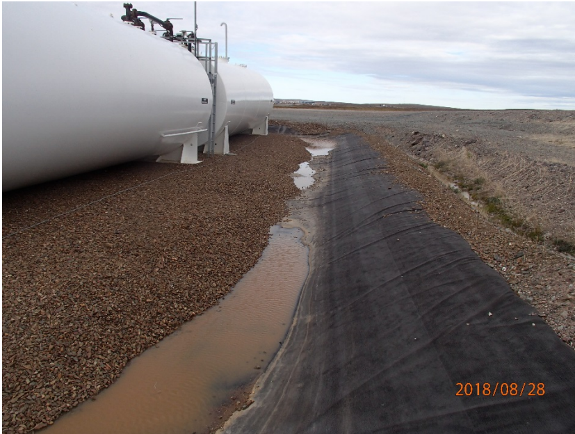
Photograph G1-23 Baker Lake Tank Farm
