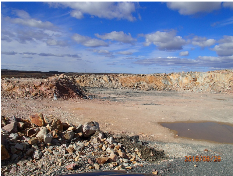
Photograph F1-8: Quarry 5 – km 34+650
