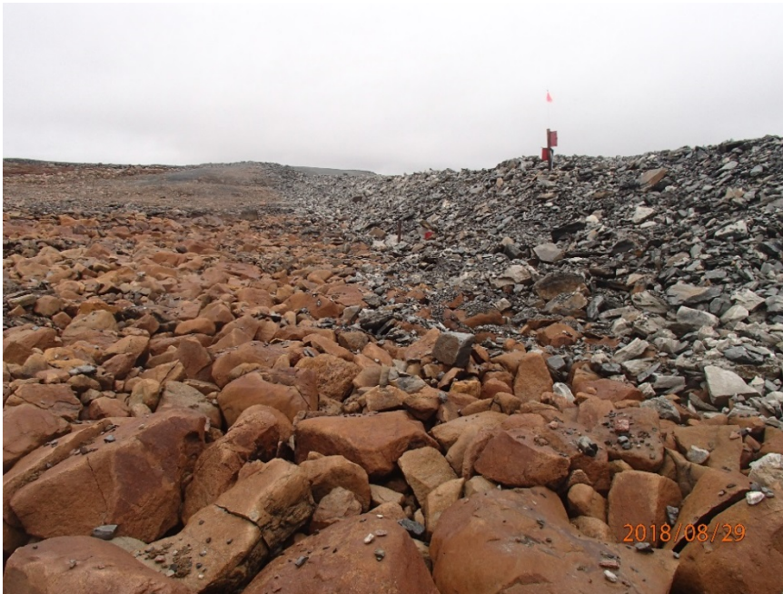
Photograph A4-3 Vault Dike
