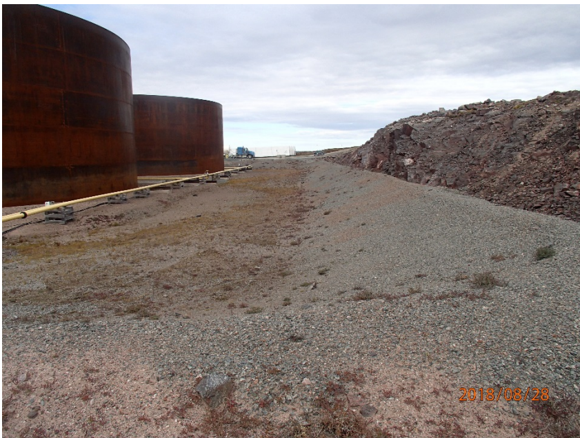
Photograph G1-14 Baker Lake Tank Farm
