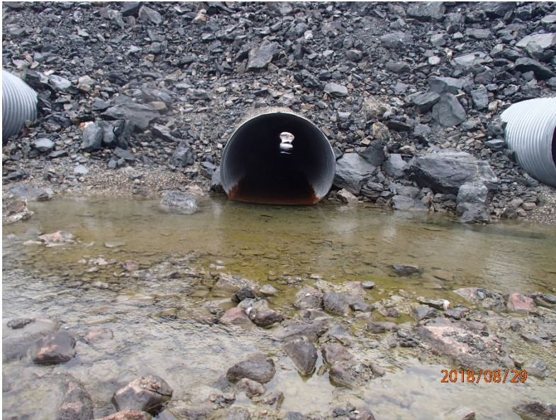
Photograph H1-3 Vault Road Culverts
