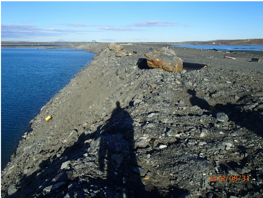
Photograph B4-10 Stormwater Dike
