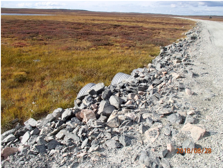
Photograph D1-18: R-18A km 80+950
