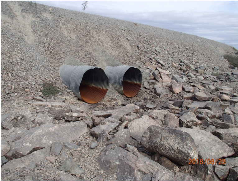
Photograph D1-5: PC-17 km 8+850
