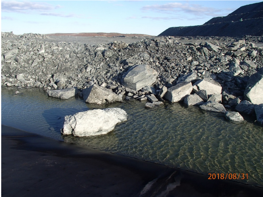
Photograph B1-16 Tailings Storage Facility
