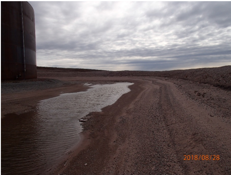
Photograph G1-11 Baker Lake Tank Farm
