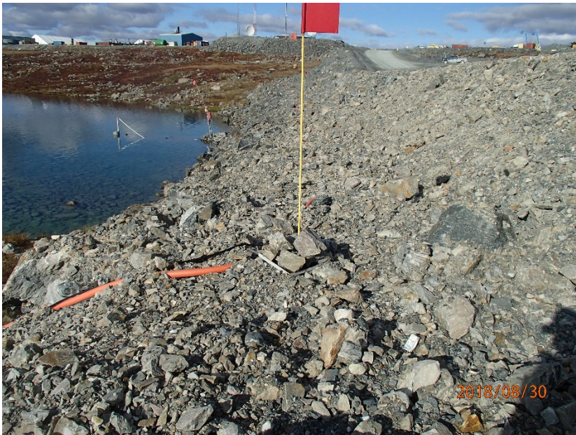
Photograph A2-1 South Camp Dike
