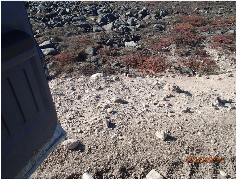
Photograph E1-5: Culvert #283 km 62+965
