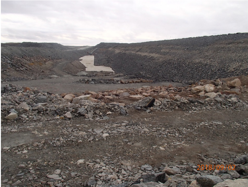
Photograph B7-1 Central Dike and Saddle Dam 5
