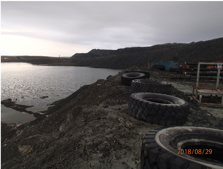
Photograph H7-1 Stormwater Pond
