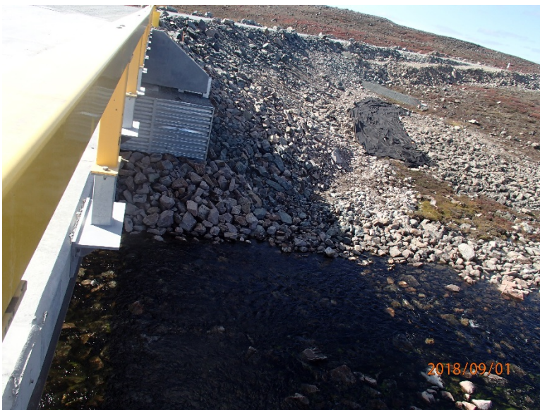
Photograph E2-26 Bridges 7 – km 32+300
