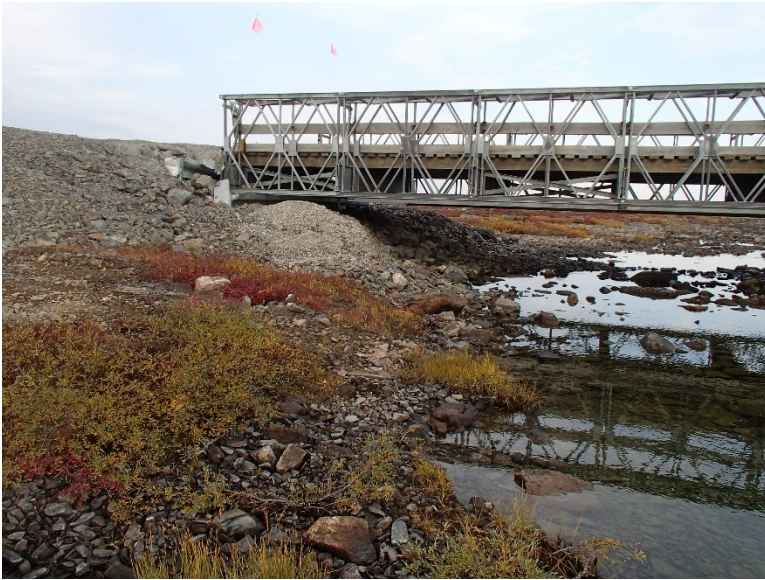
Photograph D2-9 Bridges 6 – R15 km 69+200
