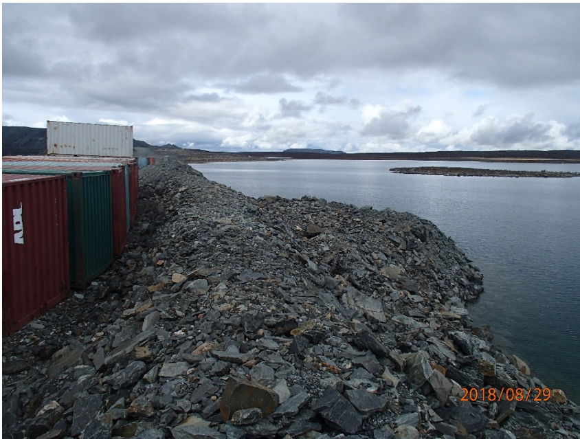
Photograph A1-8 East Dike
