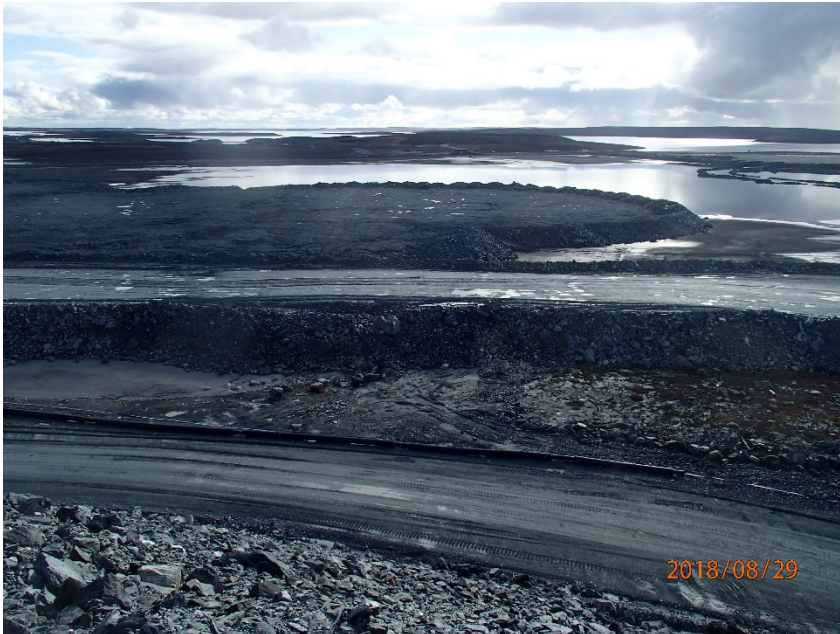
Photograph B1-13 Tailings Storage Facility
