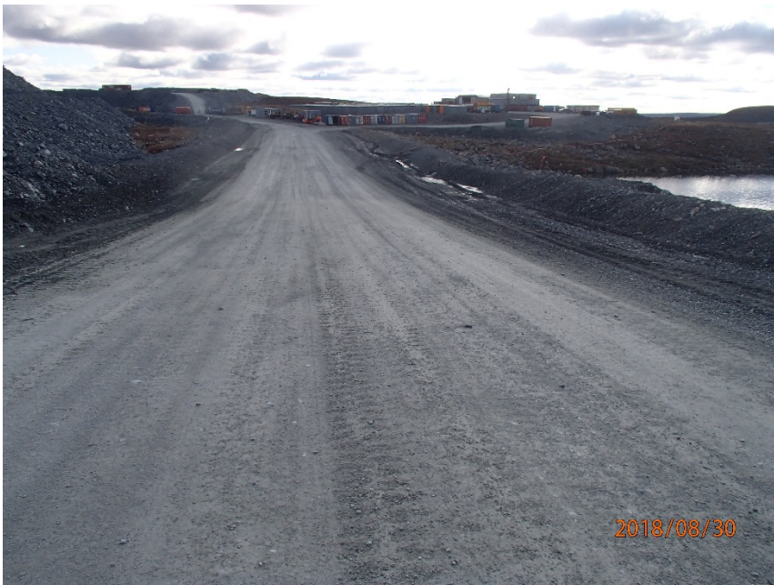
Photograph A2-4 South Camp Dike
