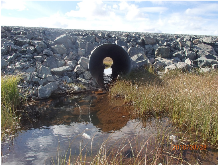
Photograph D1-11: R-07 km 25+900
