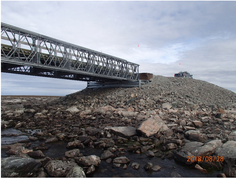
Photograph D2-1 Bridges 1 – R02 km 8+750
