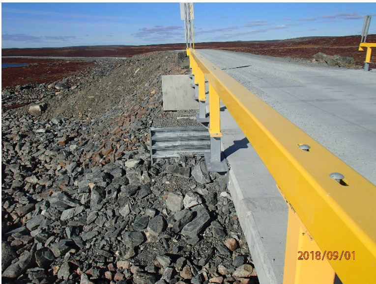
Photograph E2-6 Bridges 2 – km 10+700
