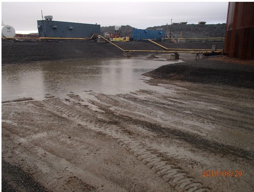
Photograph G2-4 Meadowbank Tank Farm
