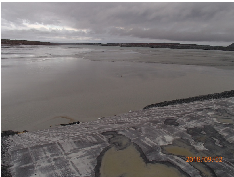
Photograph B1-21 Tailings Storage Facility
