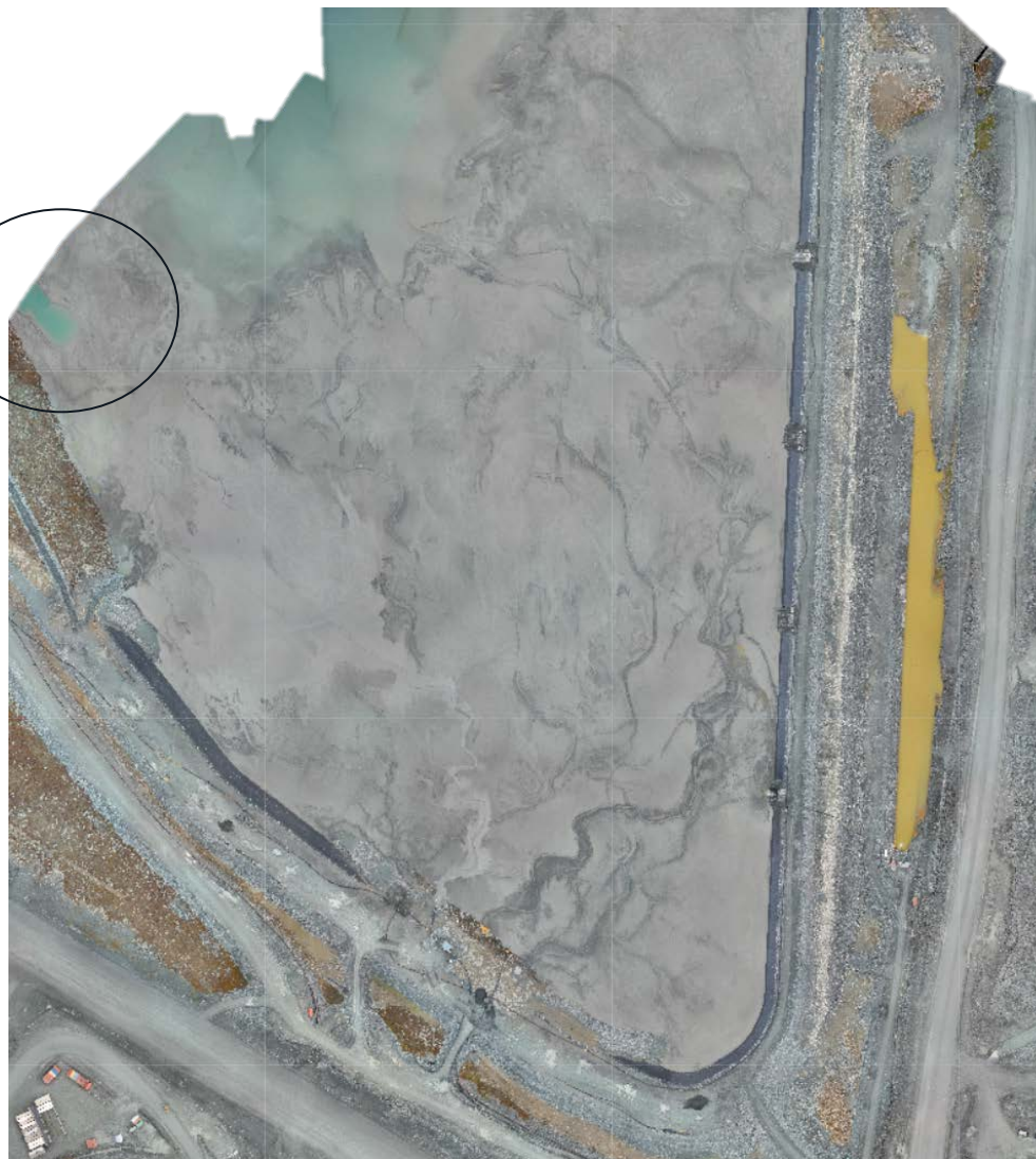
Drone survey September 7 th 2018
