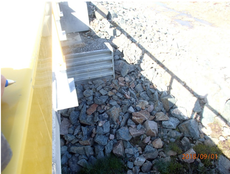
Photograph E2-30 Bridges 8 – km 43+500
