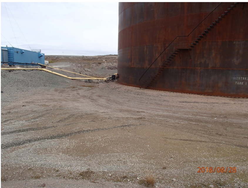
Photograph G1-2 Baker Lake Tank Farm
