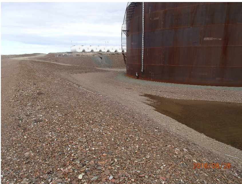
Photograph G1-16 Baker Lake Tank Farm
