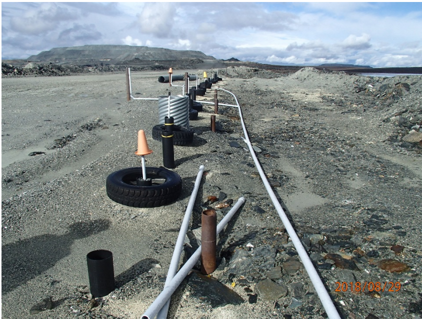
Photograph A1-6 East Dike
