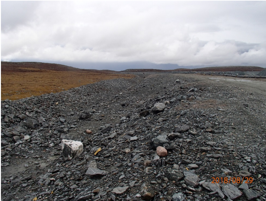
Photograph H2-15 Diversion Ditch and its Sediment and Erosion Protection Structure
