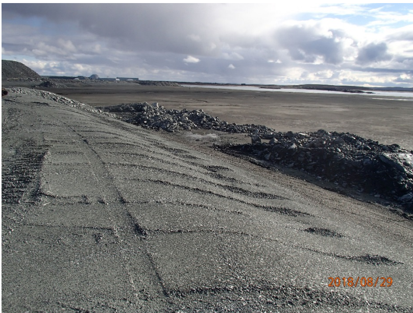
Photograph B1-8 Tailings Storage Facility
