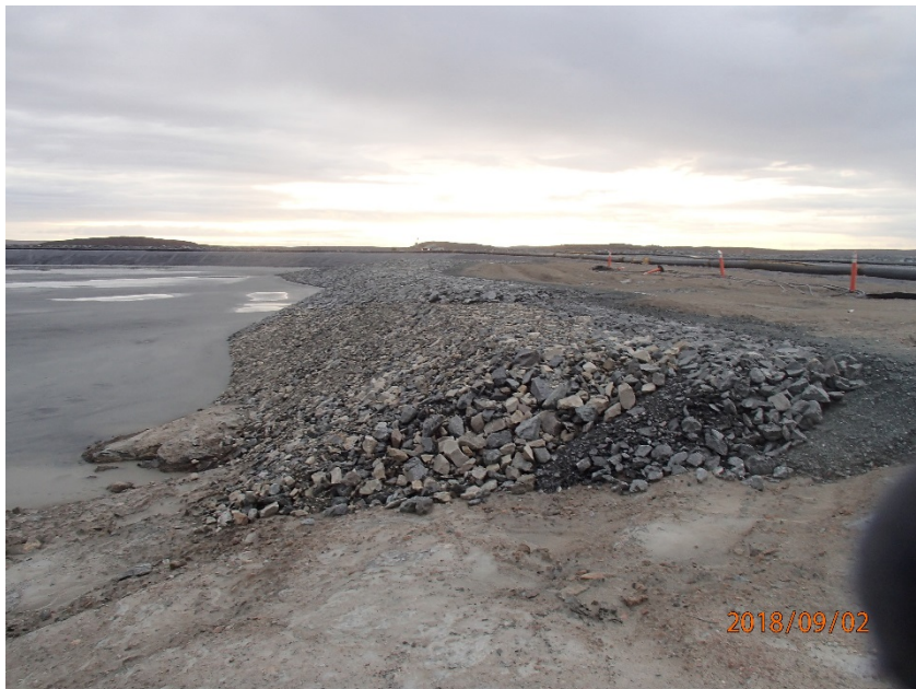
Photograph B7-18 Central Dike and Saddle Dam 5
