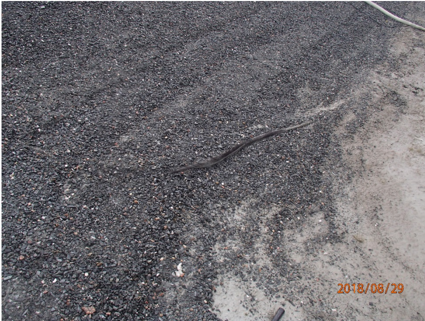
Photograph G2-7 Meadowbank Tank Farm
