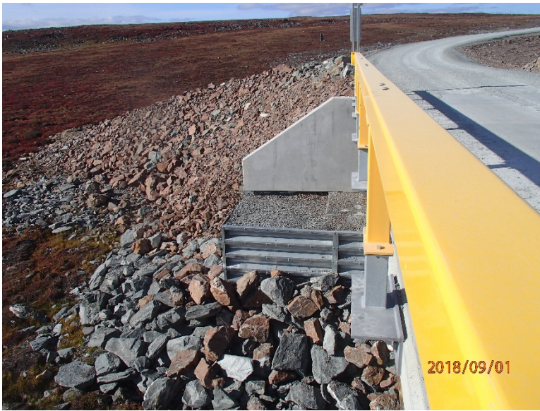
Photograph E2-9 Bridges 3 – km 16+000
