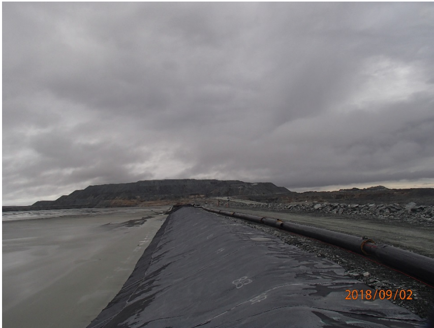
Photograph B7-13 Central Dike and Saddle Dam 5
