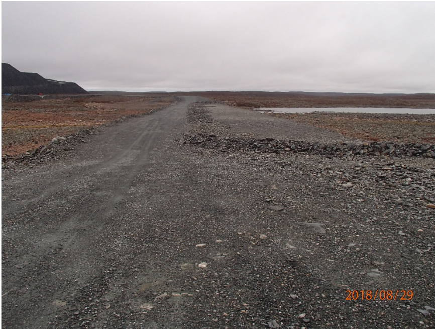
Photograph A4-1 Vault Dike
