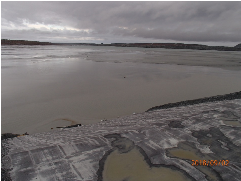
Photograph B7-4 Central Dike and Saddle Dam 5
