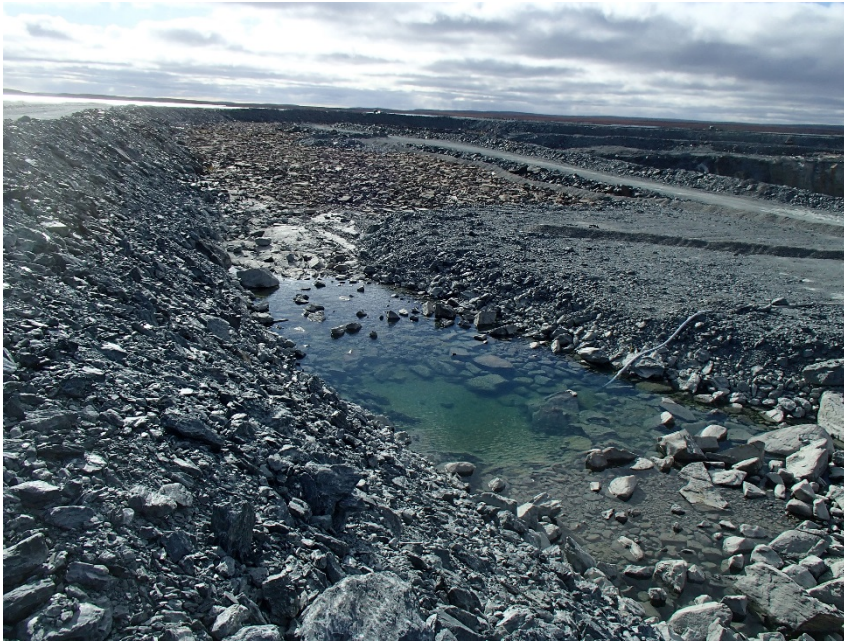
Photograph A3-19 Bay Goose Dike
