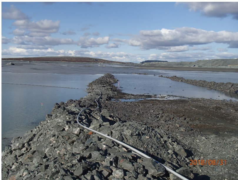
Photograph B1-10 Tailings Storage Facility
