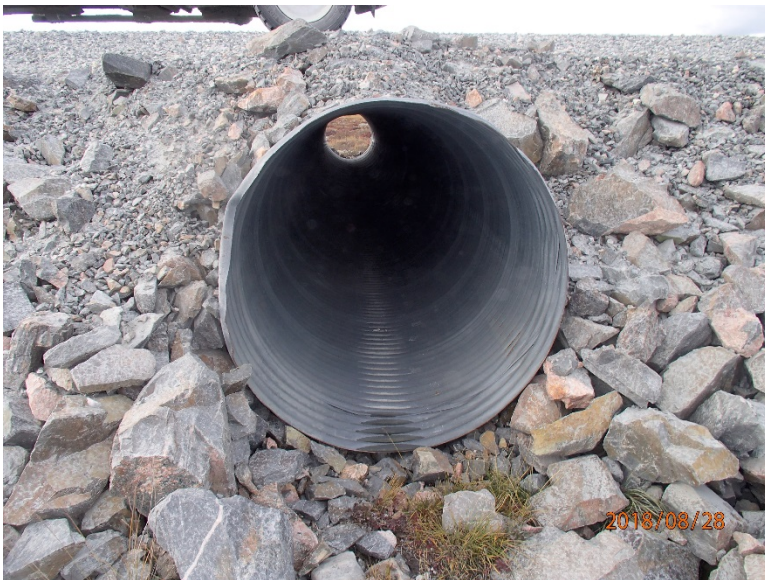
Photograph D1-16: R-17 km 77+440
