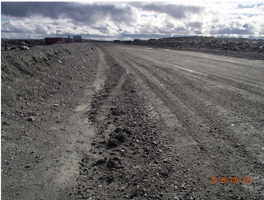
Photograph A1-4 East Dike
