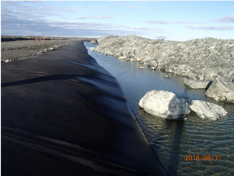
Photograph B4-1 Stormwater Dike
