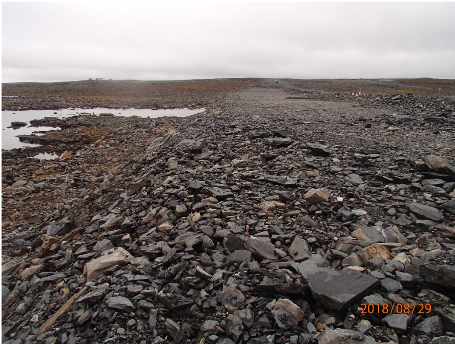
Photograph A4-5 Vault Dike
