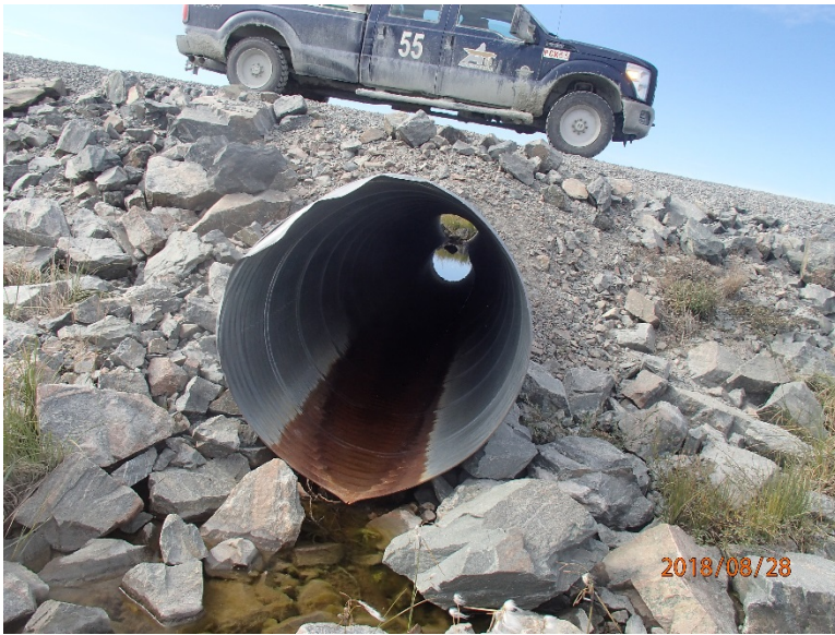
Photograph D1-7: R-04 km 12+050
