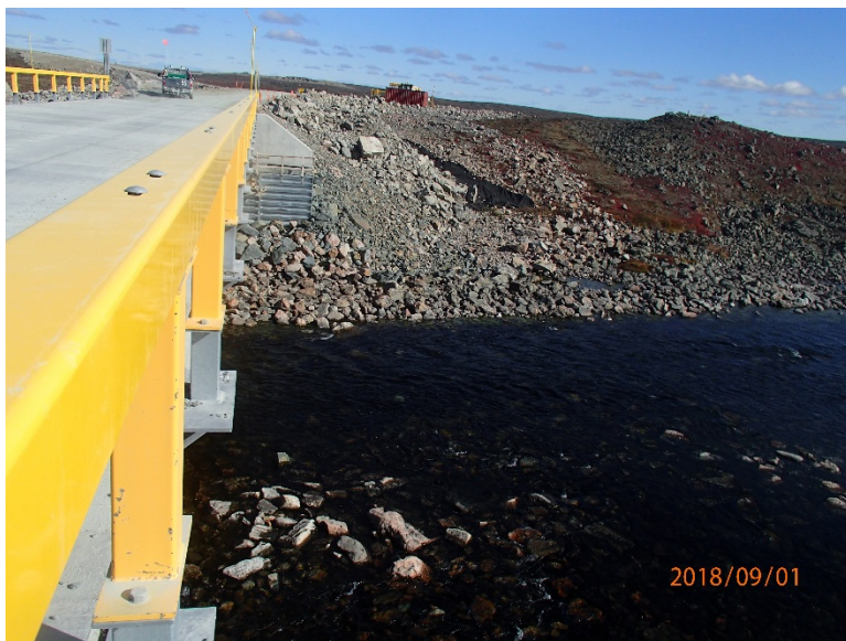
Photograph E2-28 Bridges 7 – km 32+300
