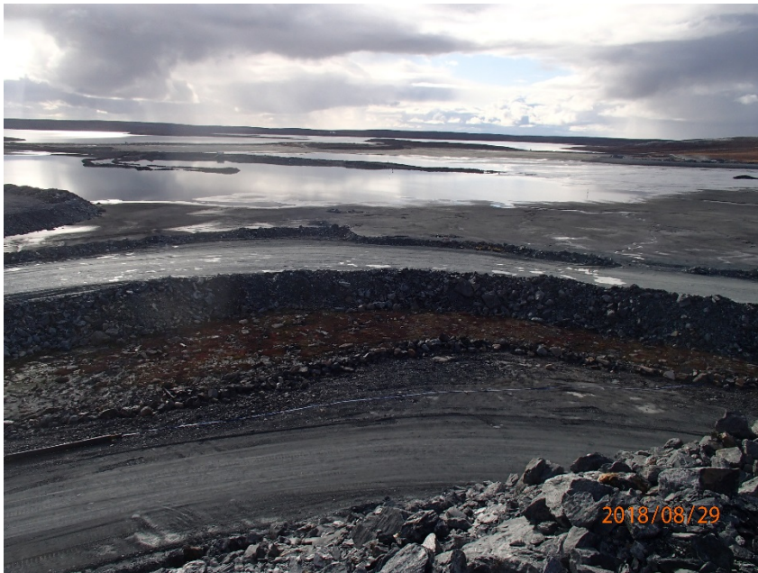
Photograph B1-14 Tailings Storage Facility
