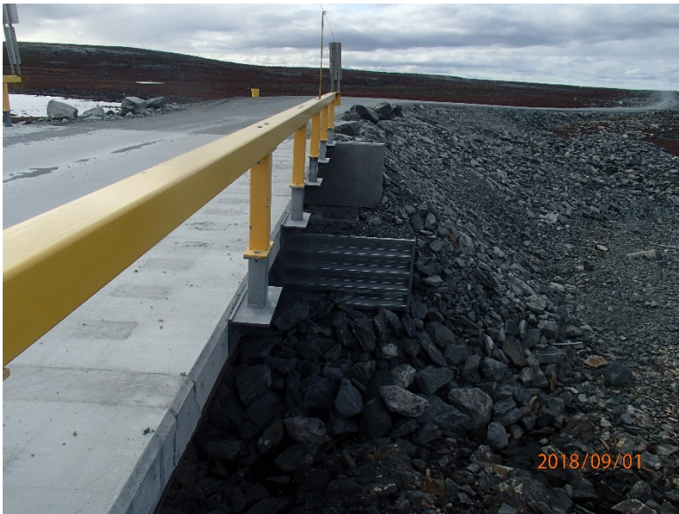
Photograph E2-1 Bridges 1 – km 3+400
