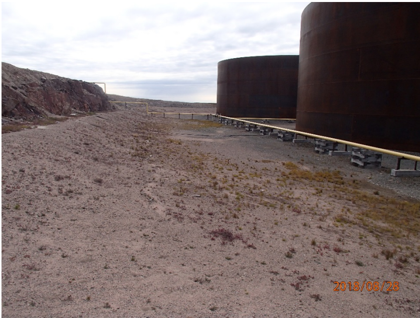
Photograph G1-15 Baker Lake Tank Farm
