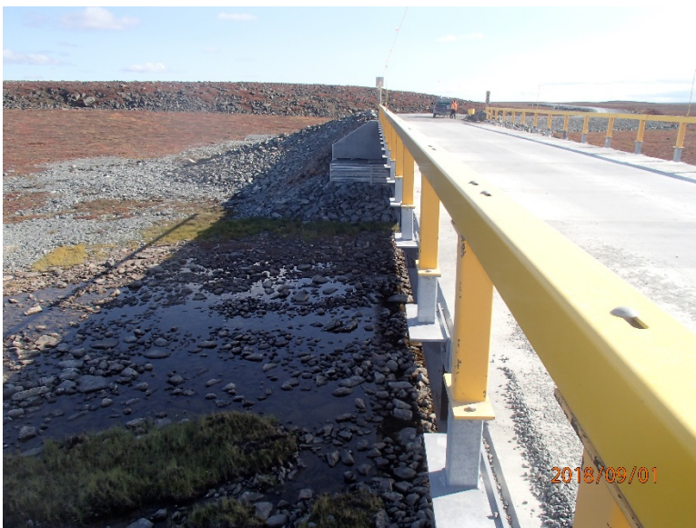
Photograph E2-12 Bridges 3 – km 16+000
