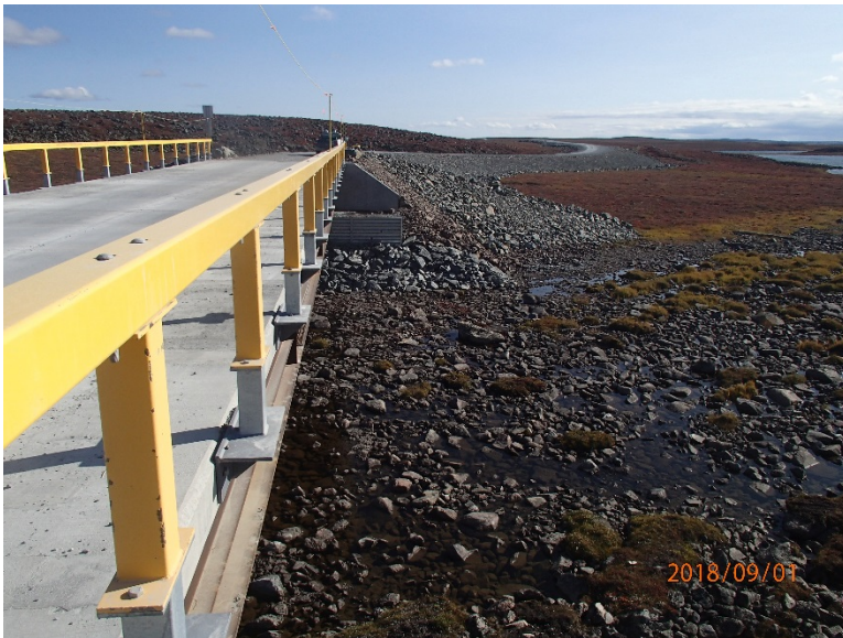
Photograph E2-11 Bridges 3 – km 16+000
