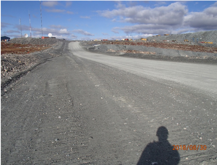
Photograph A2-3 South Camp Dike
