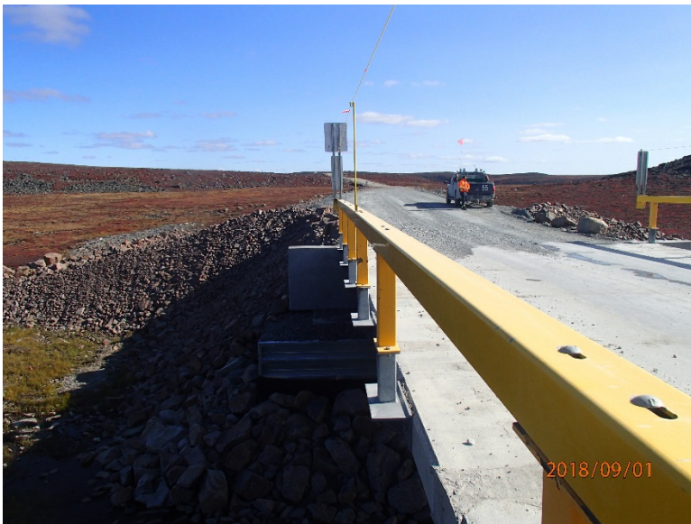
Photograph E2-16 Bridges 4 – km 20+000
