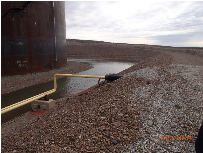
Photograph G1-18 Baker Lake Tank Farm
