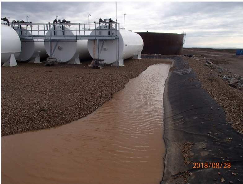
Photograph G1-24 Baker Lake Tank Farm
