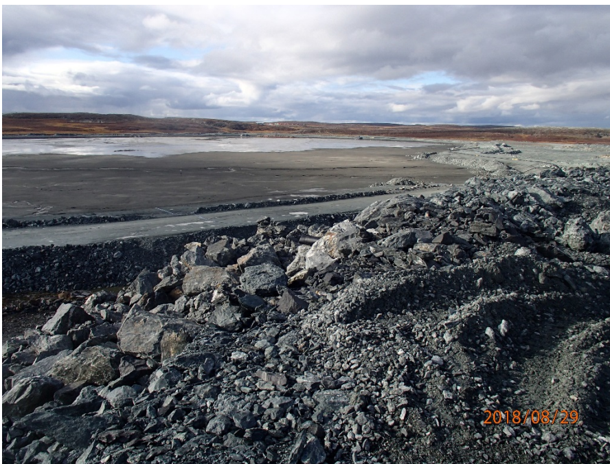
Photograph B1-15 Tailings Storage Facility
