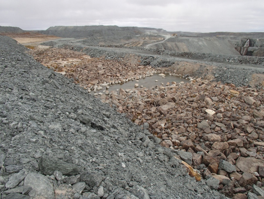
Photograph A3-35 Bay Goose Dike
