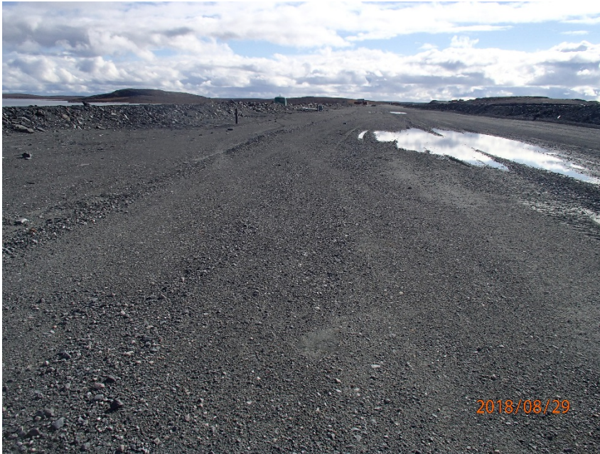
Photograph A1-7 East Dike
