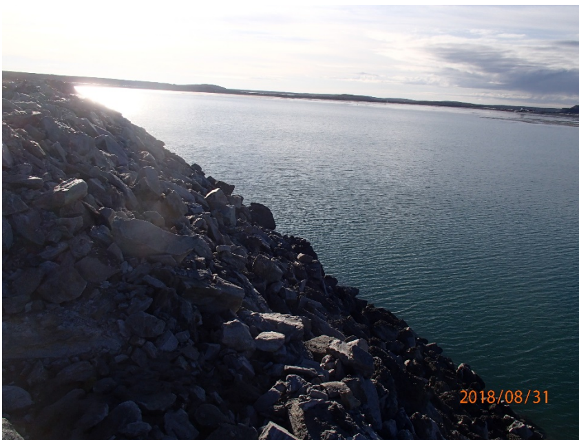
Photograph B4-14 Stormwater Dike
