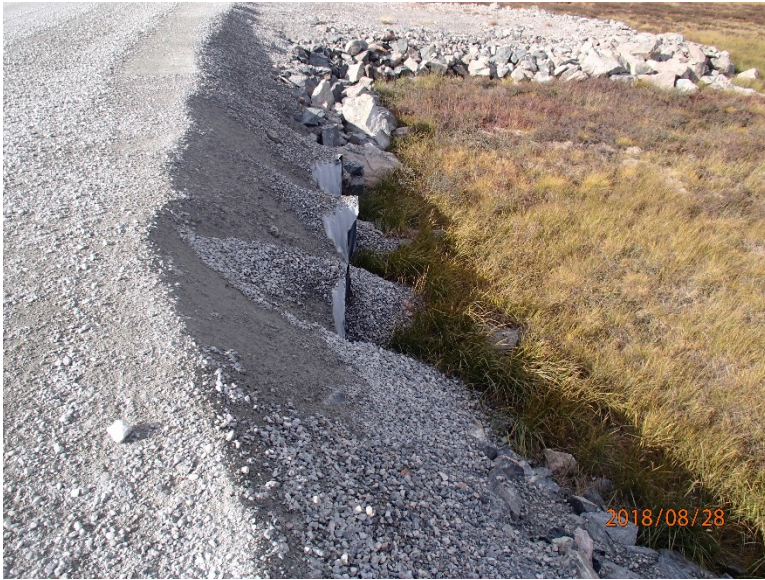
Photograph D1-17: R-18A km 80+950
