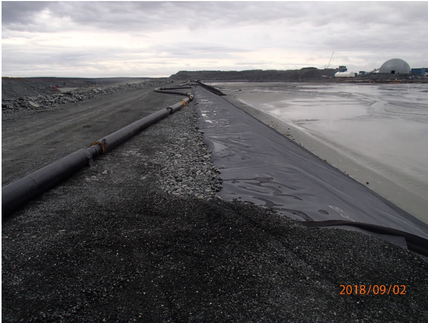
Photograph B7-3 Central Dike and Saddle Dam 5
