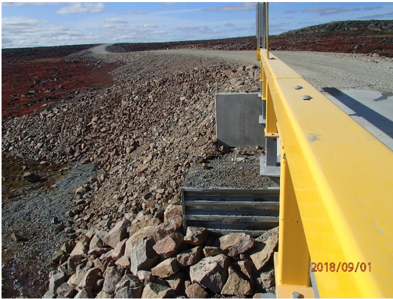
Photograph E2-13 Bridges 4 – km 20+000
