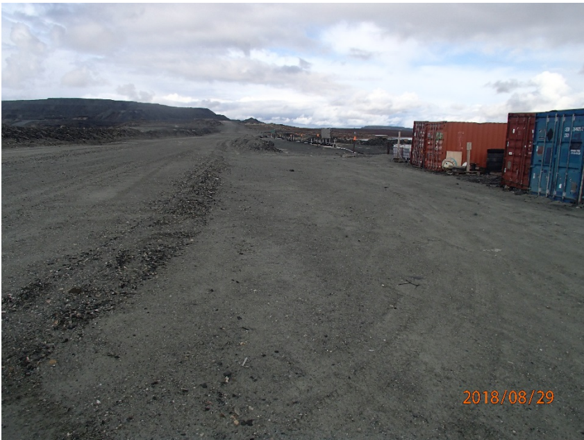
Photograph A1-2 East Dike
