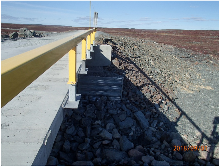
Photograph E2-5 Bridges 2 – km 10+700
