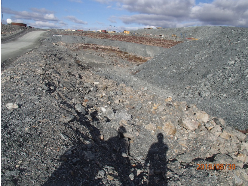
Photograph A2-6 South Camp Dike
