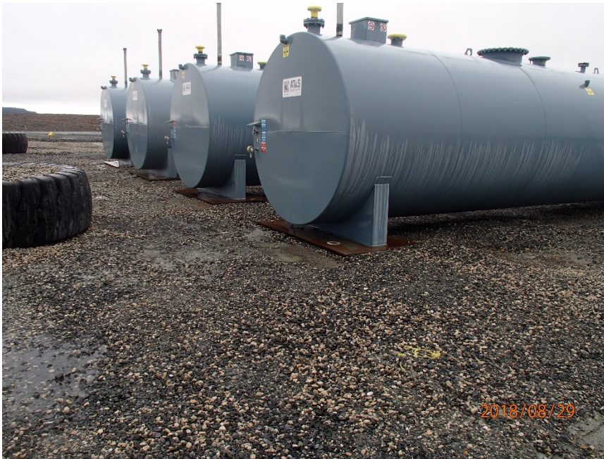
Photograph G3-1 Vault Tank Farm
