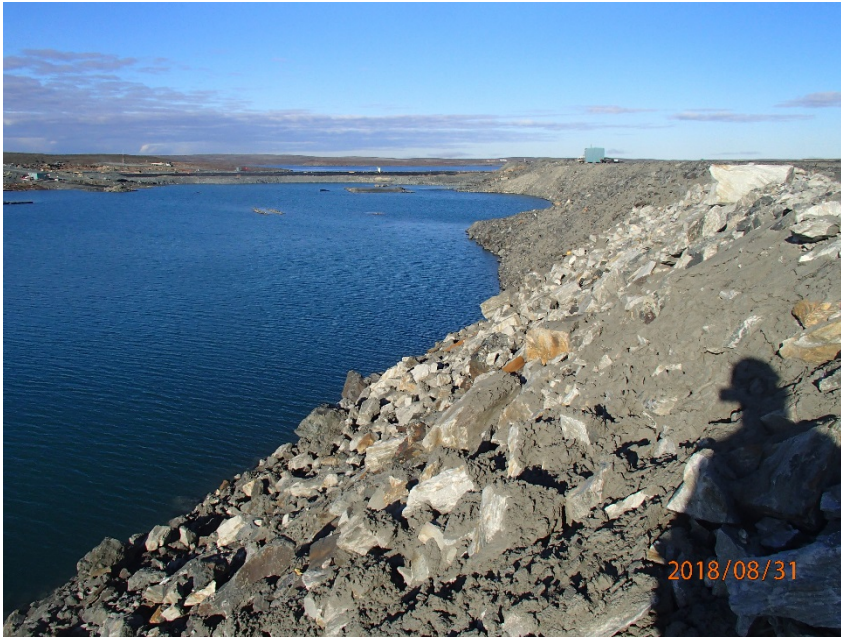
Photograph B4-13 Stormwater Dike
