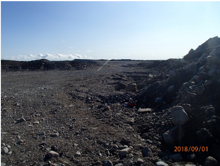
Photograph F2-9 Eskers and Quarries 6 – km 62+500
