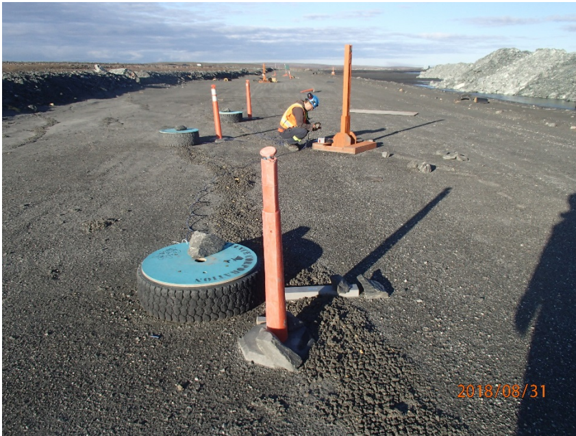
Photograph B4-17 Stormwater Dike
