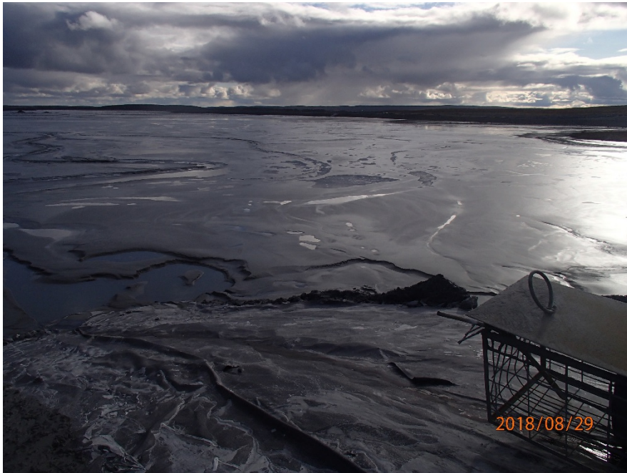
Photograph B1-18 Tailings Storage Facility
