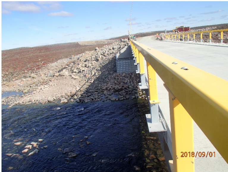
Photograph E2-27 Bridges 7 – km 32+300
