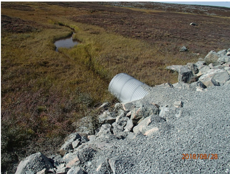
Photograph D1-10: R-07 km 25+900
