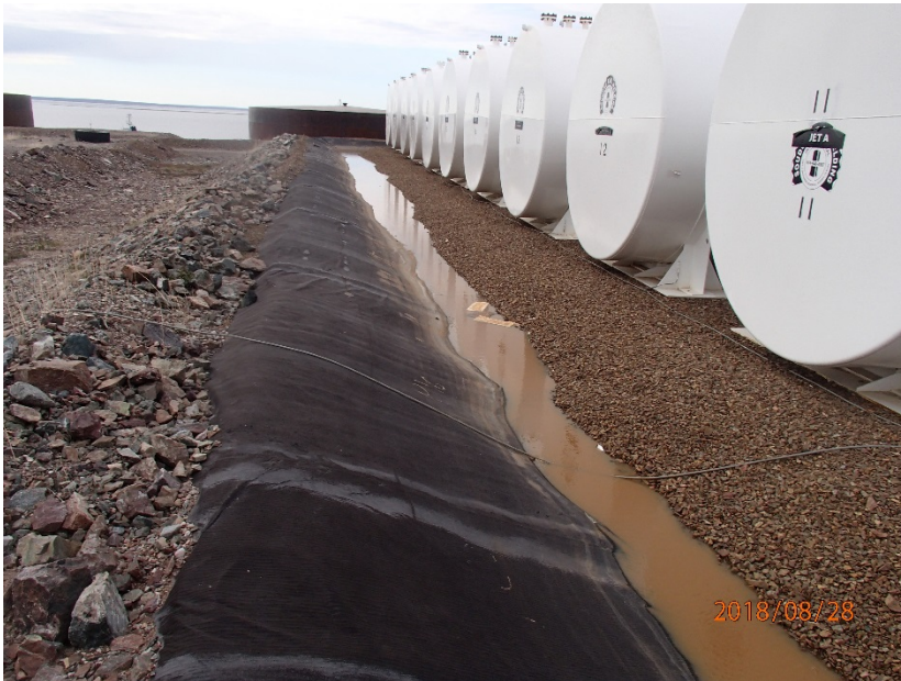
Photograph G1-22 Baker Lake Tank Farm
