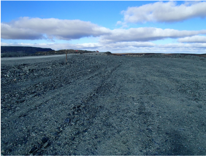
Photograph A3-3 Bay Goose Dike
