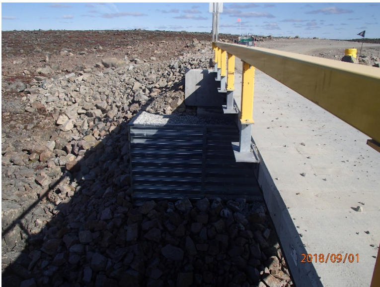
Photograph E2-24 Bridges 6 – km 26+100
