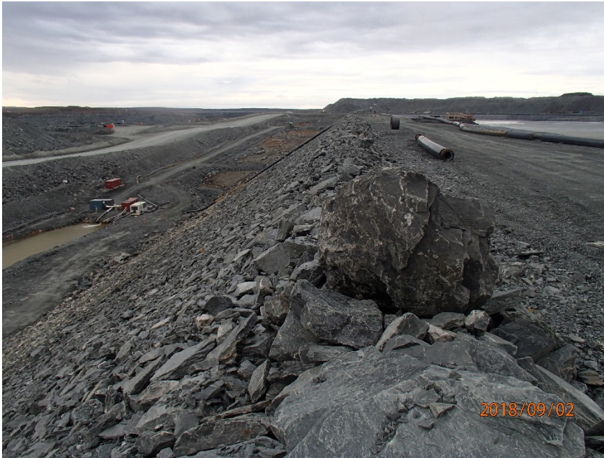
Photograph B7-5 Central Dike and Saddle Dam 5
