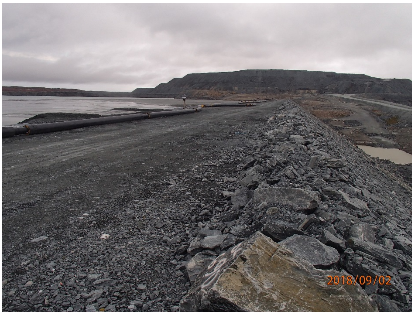
Photograph B7-8 Central Dike and Saddle Dam 5
