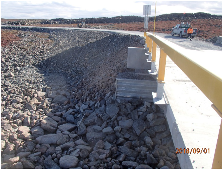
Photograph E2-7 Bridges 2 – km 10+700
