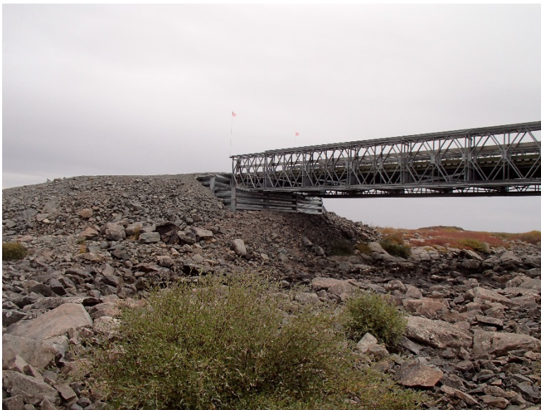
Photograph D2-2 Bridges 1 – R02 km 8+750
