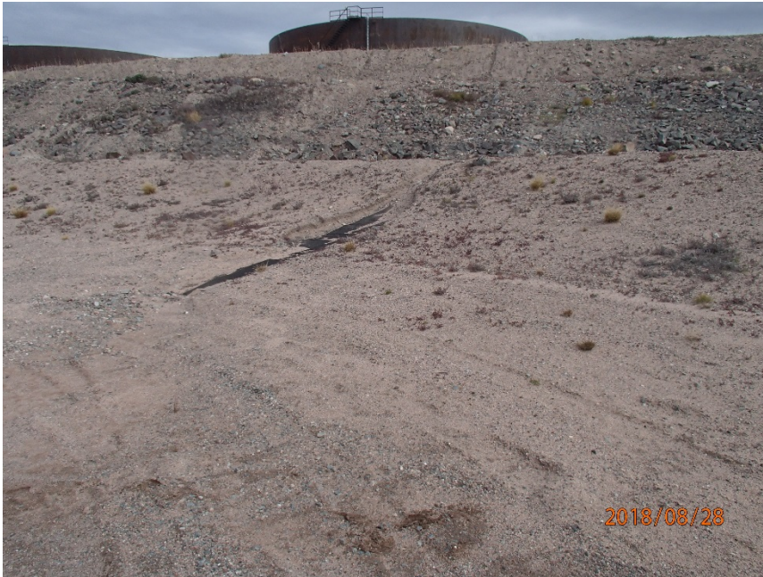
Photograph G1-13 Baker Lake Tank Farm
