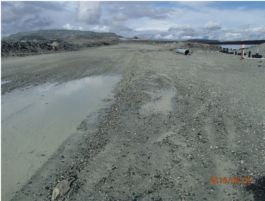
Photograph A1-3 East Dike
