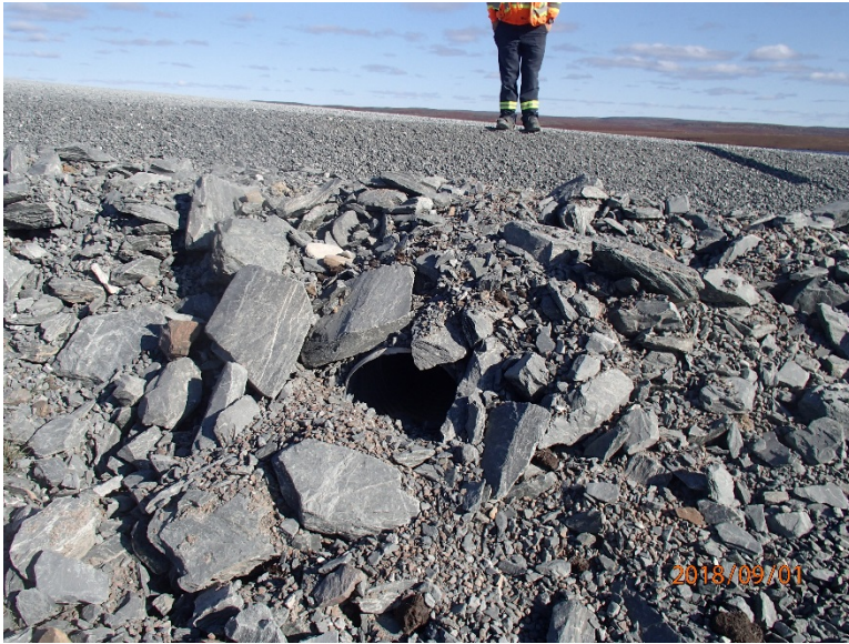
Photograph E1-1: Culvert #66 km 16+324
