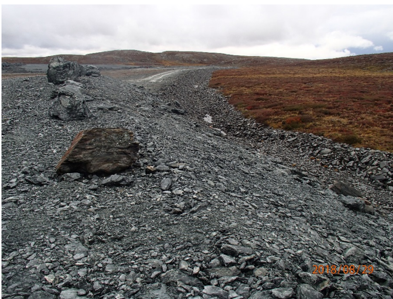
Photograph H2-10 Diversion Ditch and its Sediment and Erosion Protection Structure
