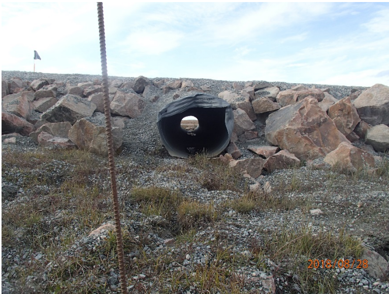
Photograph D1-22: R-23 km 93+600
