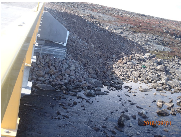
Photograph E2-18 Bridges 5 – km 23+900
