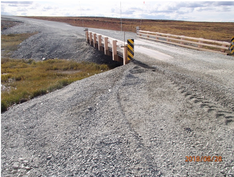
Photograph D2-7 Bridges 5 – R13 km 62+060
