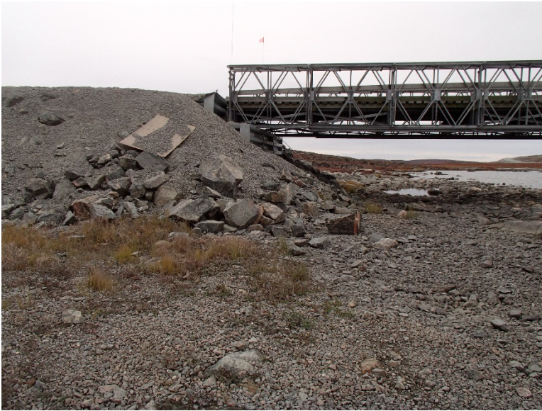
Photograph D2-5 Bridges 3 – R06 km 23+100
