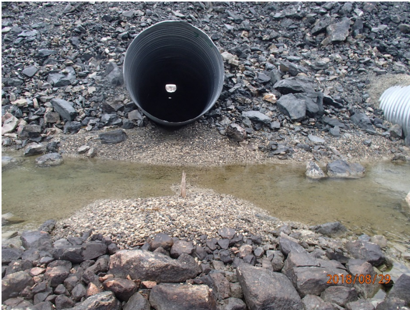
Photograph H1-2 Vault Road Culverts
