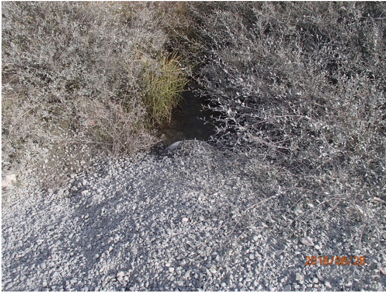
Photograph D1-13: PC-11 km 39+552
