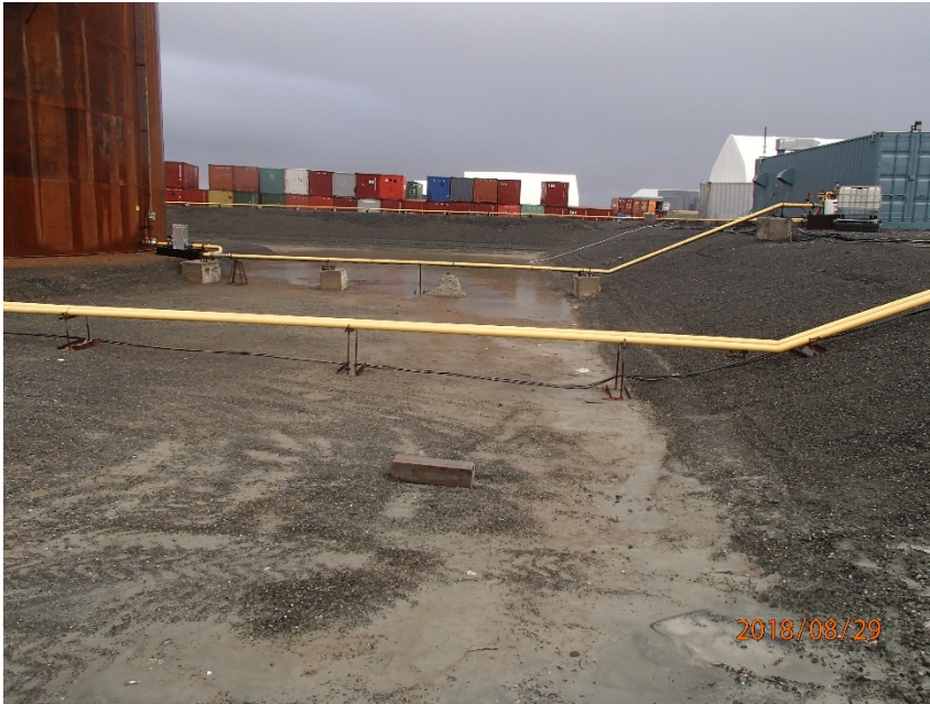
Photograph G2-5 Meadowbank Tank Farm
