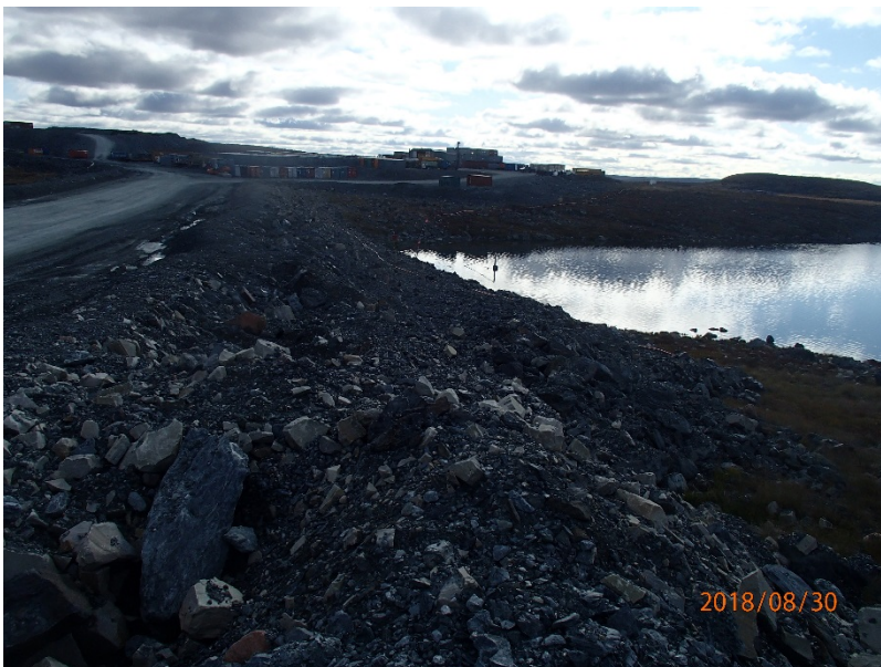
Photograph A2-2 South Camp Dike
