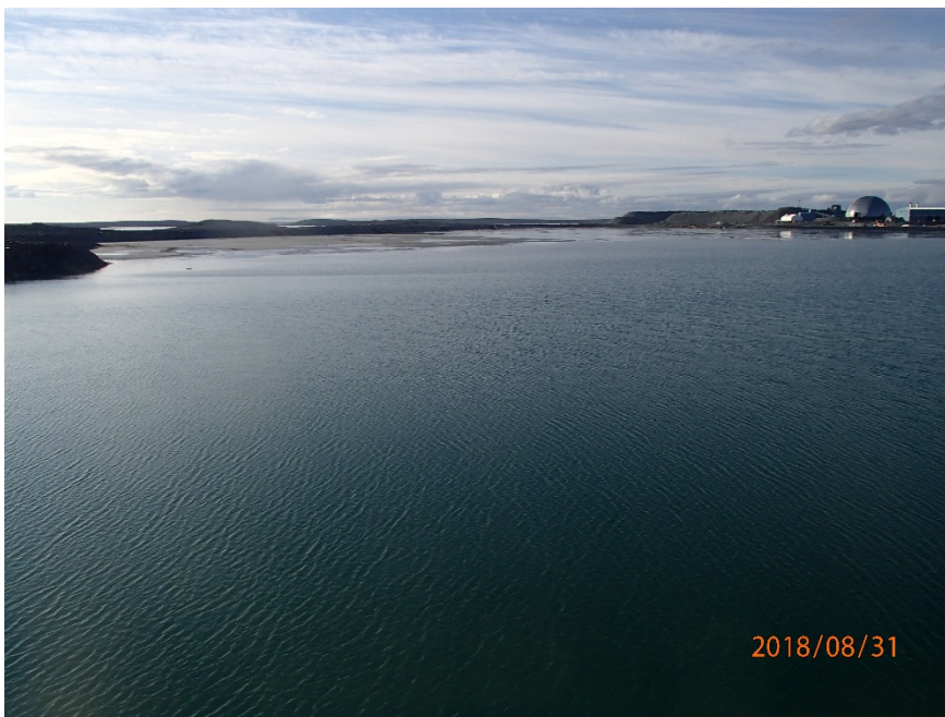
Photograph B4-8 Stormwater Dike
