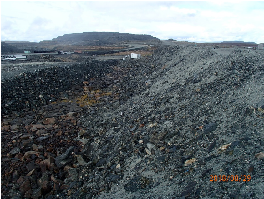
Photograph A1-11 East Dike
