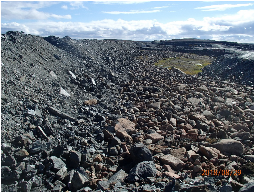
Photograph A1-12 East Dike
