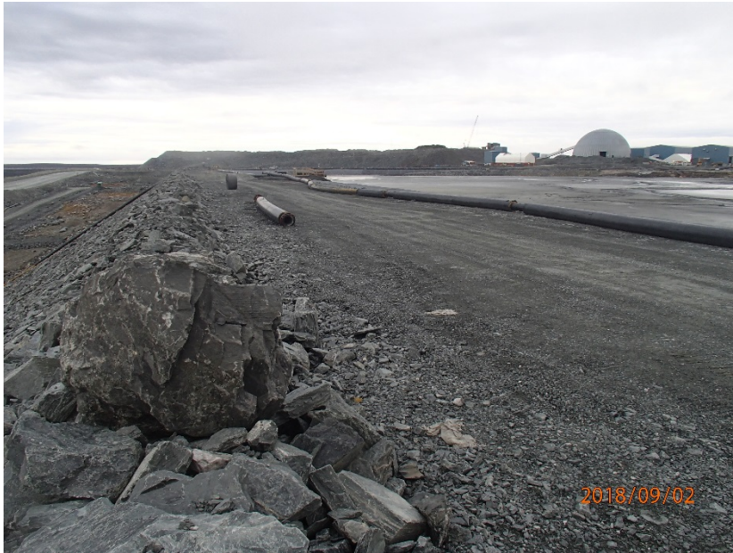
Photograph B7-7 Central Dike and Saddle Dam 5
