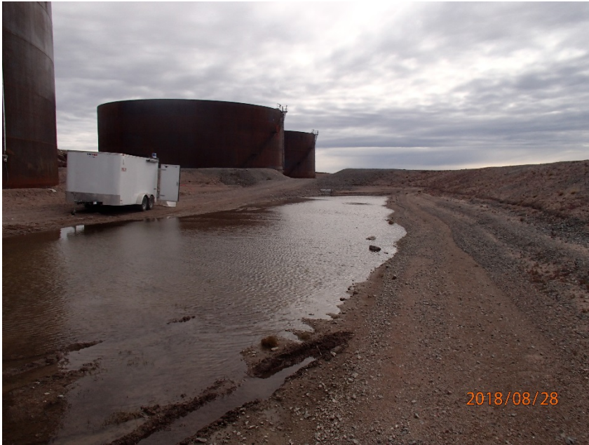
Photograph G1-5 Baker Lake Tank Farm
