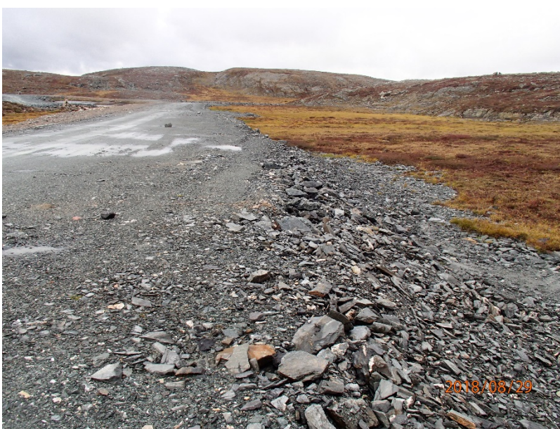
Photograph H2-12 Diversion Ditch and its Sediment and Erosion Protection Structure
