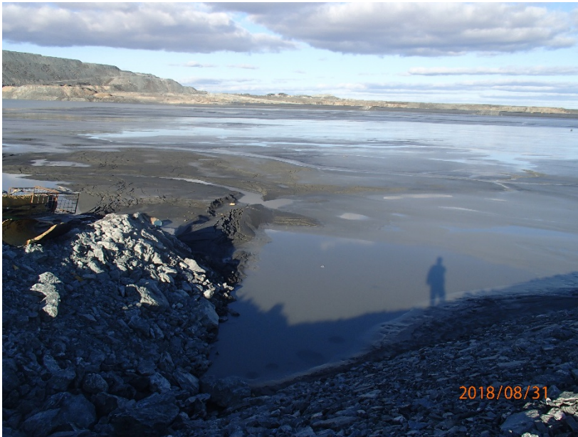
Photograph B1-22 Tailings Storage Facility
