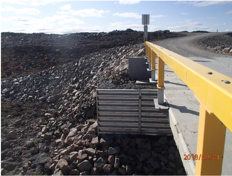
Photograph E2-21 Bridges 6 – km 26+100
