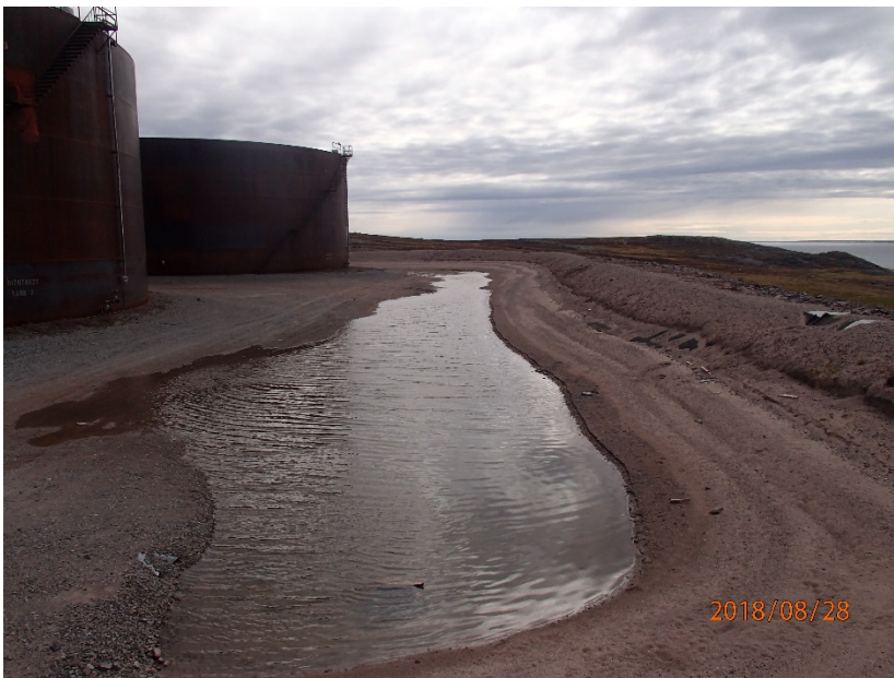
Photograph G1-8 Baker Lake Tank Farm
