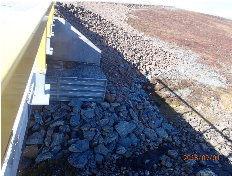
Photograph E2-10 Bridges 3 – km 16+000
