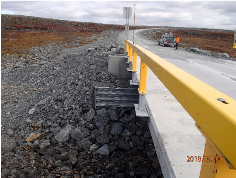
Photograph E2-3 Bridges 1 – km 3+400
