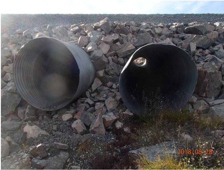
Photograph D1-25: R-24 km 98+100
