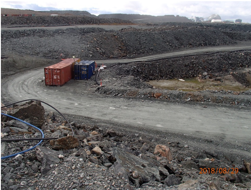
Photograph A1-10 East Dike
