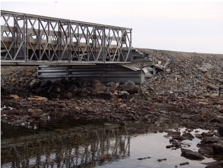
Photograph D2-10 Bridges 6 – R15 km 69+200
