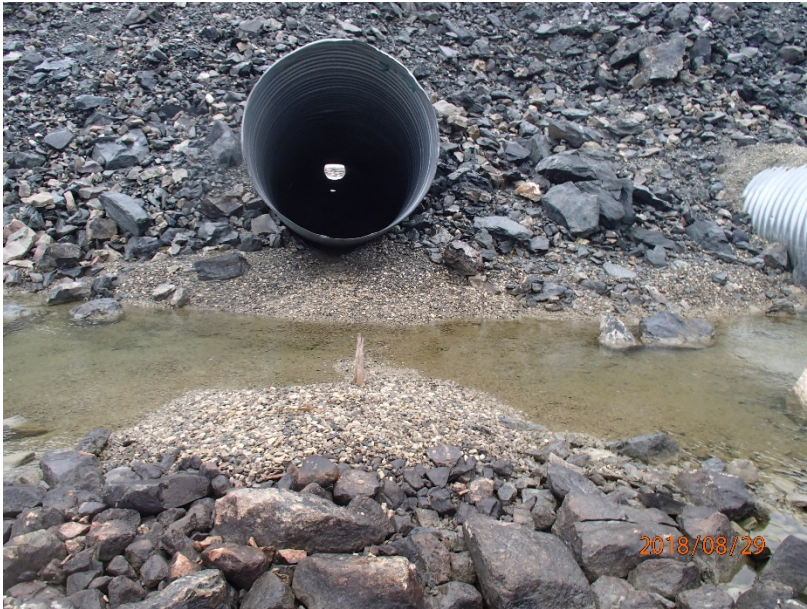
Photograph H1-1 Vault Road Culverts
