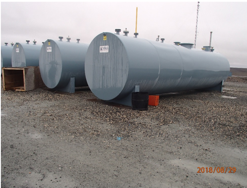
Photograph G3-2 Vault Tank Farm
