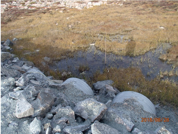
Photograph D1-27: R-26 km 104+400
