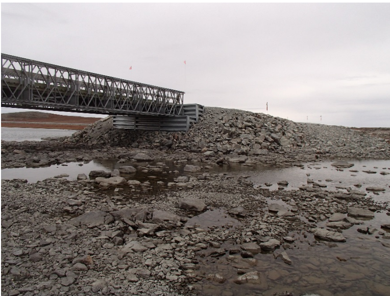
Photograph D2-6 Bridges 3 – R06 km 23+100
