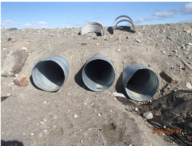
Photograph E1-4: Culverts #208, #209 and #210, km 49+431 to 49+435
