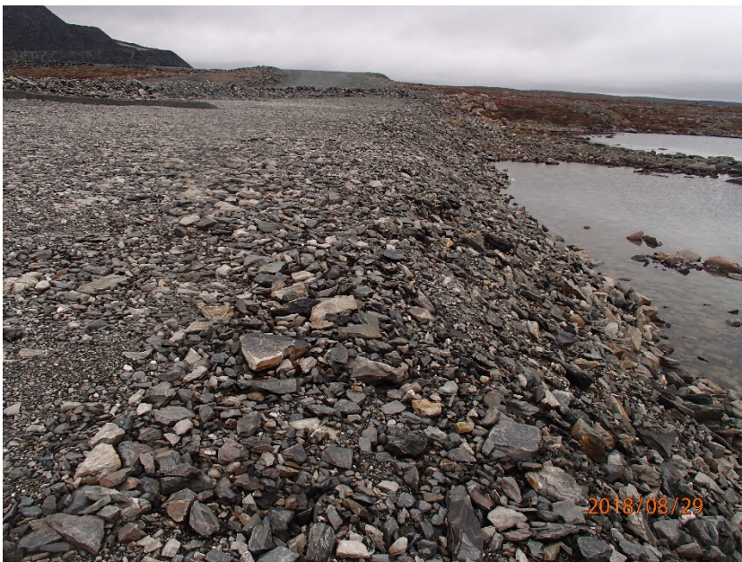
Photograph A4-6 Vault Dike
