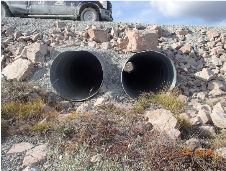
Photograph D1-21: R-21 km 87+300
