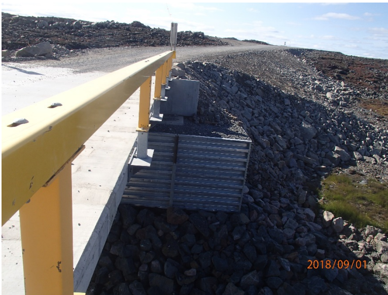
Photograph E2-22 Bridges 6 – km 26+100
