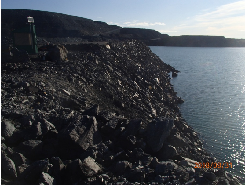
Photograph B4-9 Stormwater Dike
