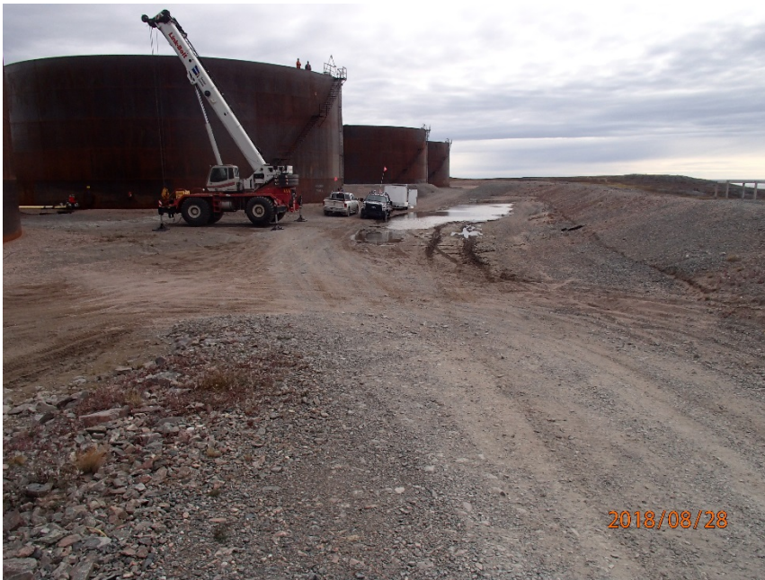
Photograph G1-1 Baker Lake Tank Farm
