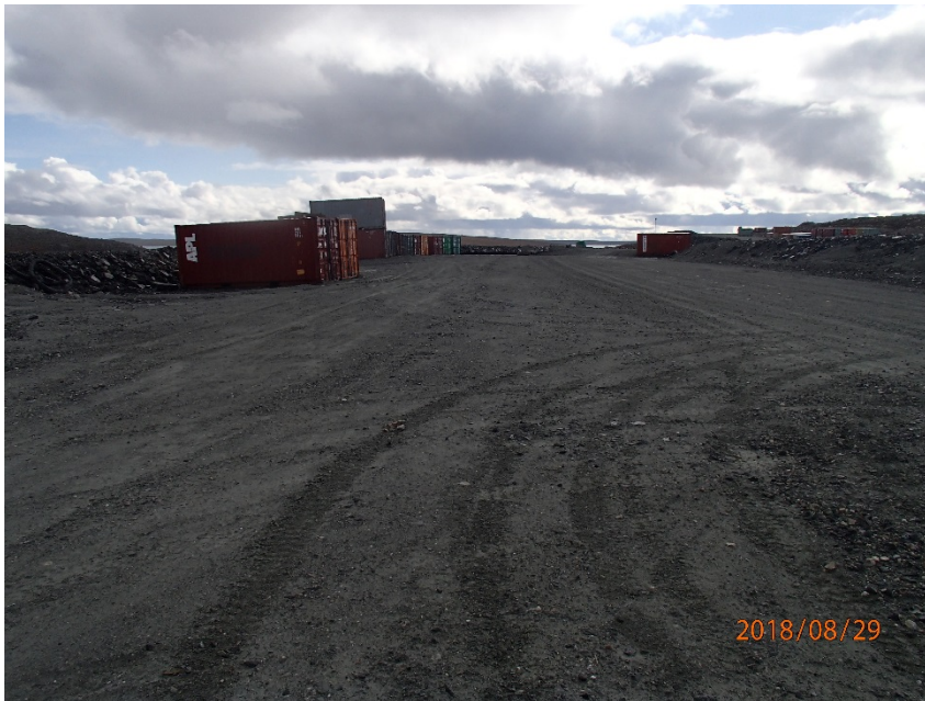
Photograph A1-1 East Dike
