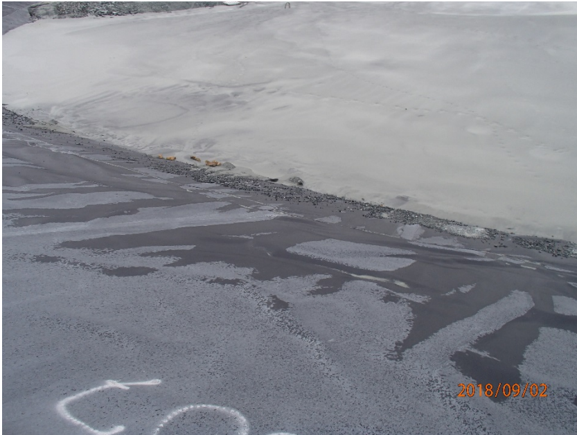
Photograph B7-11 Central Dike and Saddle Dam 5
