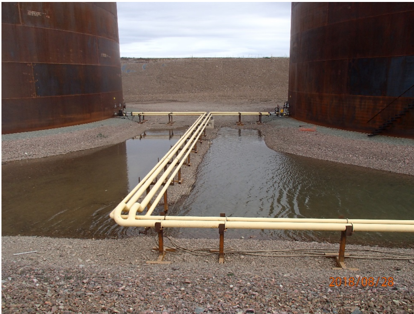
Photograph G1-17 Baker Lake Tank Farm
