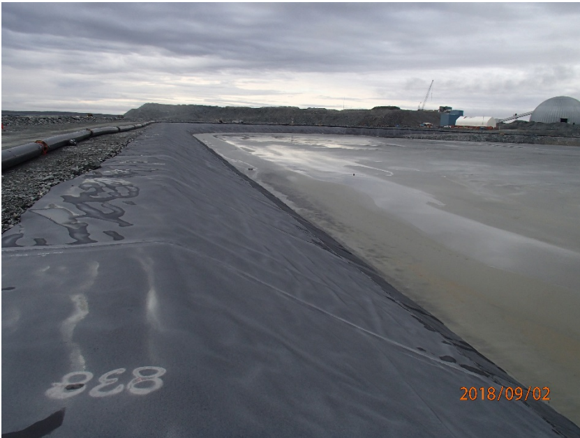
Photograph B7-10 Central Dike and Saddle Dam 5
