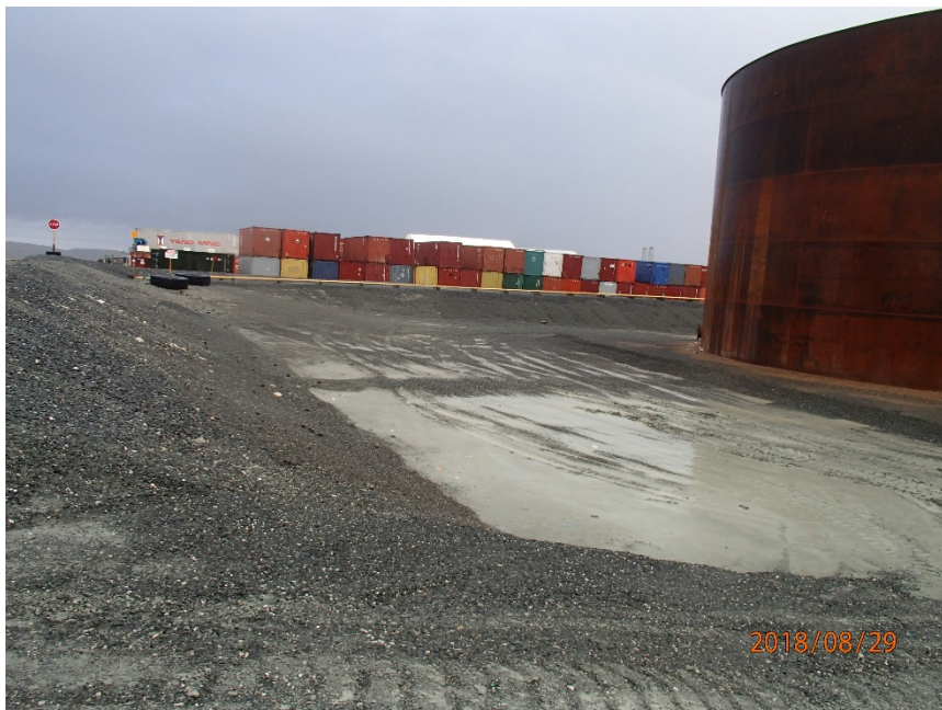
Photograph G2-2 Meadowbank Tank Farm
