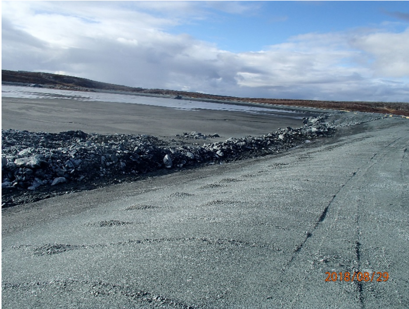
Photograph B1-7 Tailings Storage Facility
