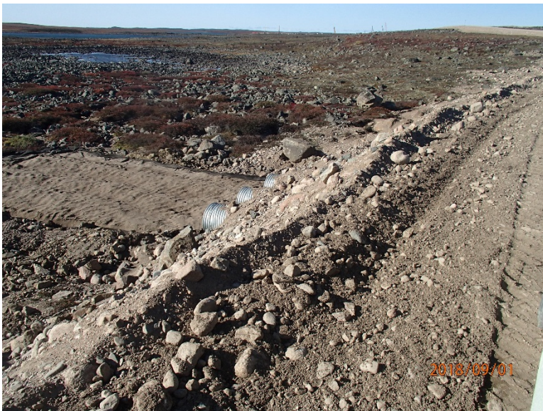
Photograph E1-6: Culverts #284, #284-2 and #284-3, km 63+070 to 63+074
