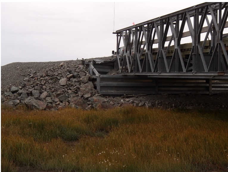
Photograph D2-4 Bridges 2 – R05 km 17+600
