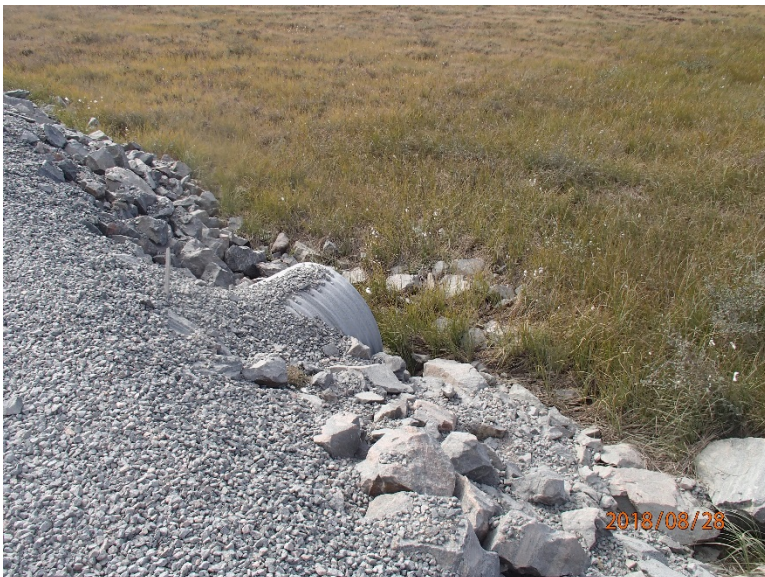
Photograph D1-6: R-04 km 12+050
