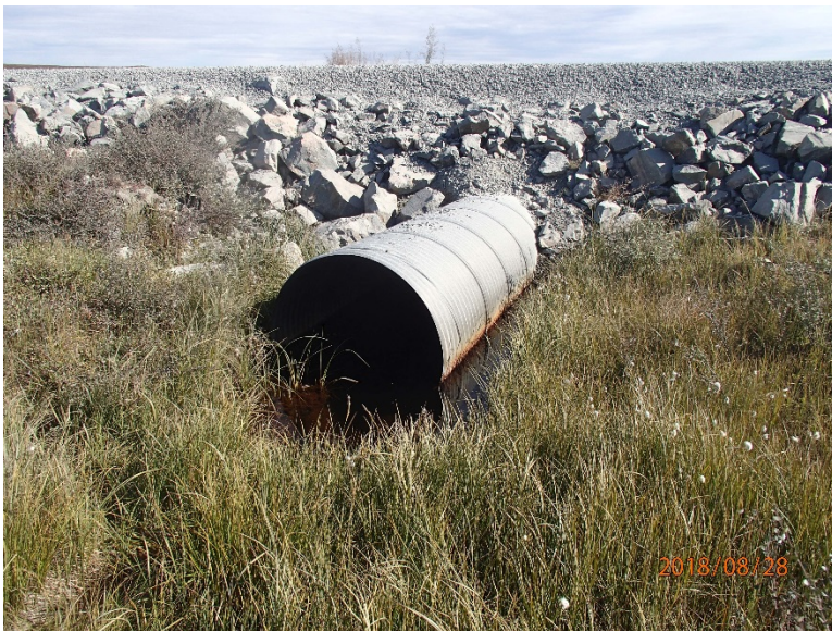
Photograph D1-8: R-05A km 15+745
