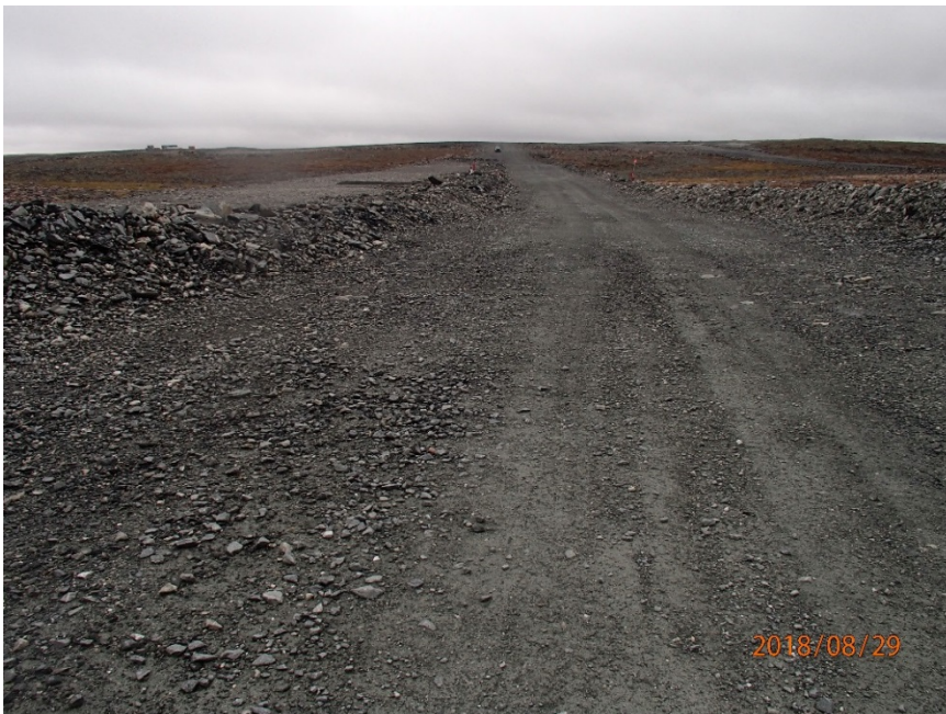
Photograph A4-4 Vault Dike
