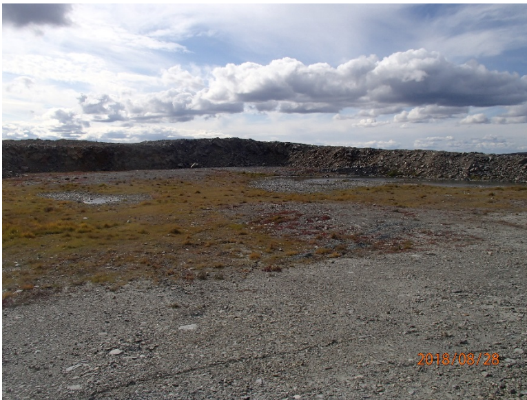
Photograph F1-26: Quarry 15 – km 67+600
