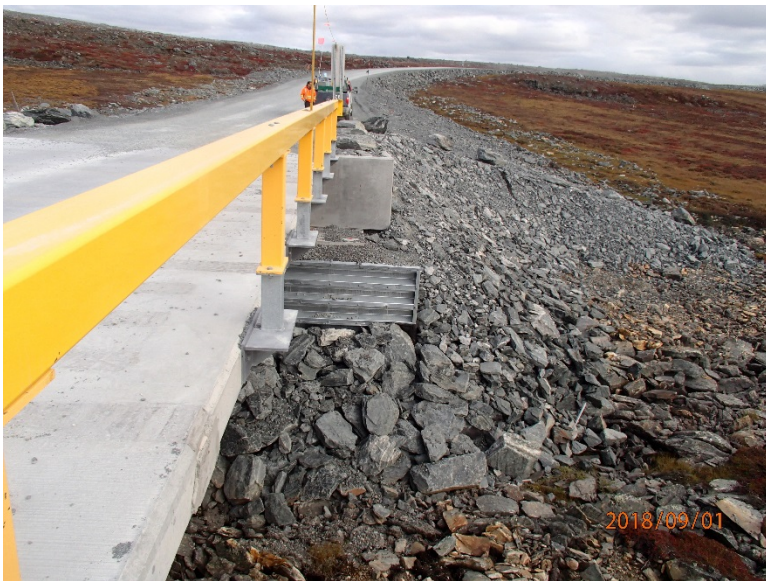
Photograph E2-4 Bridges 1 – km 3+400
