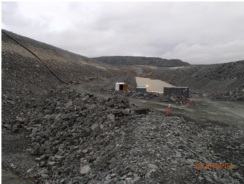
Photograph B7-12 Central Dike and Saddle Dam 5
