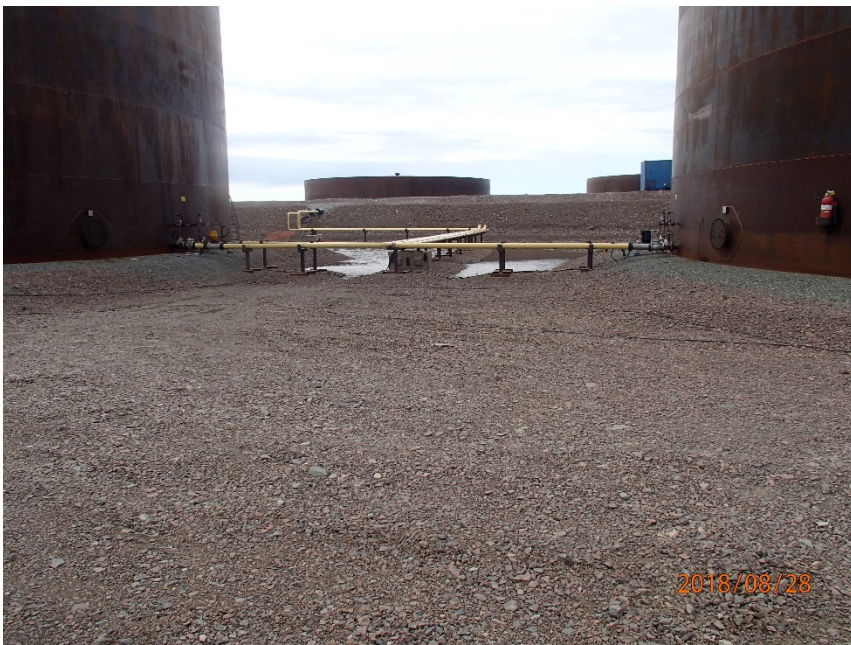
Photograph G1-20 Baker Lake Tank Farm
