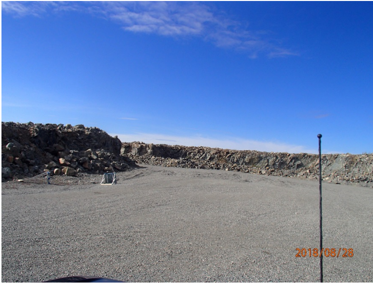
Photograph F1-3: Quarry 2 – km 13+250
