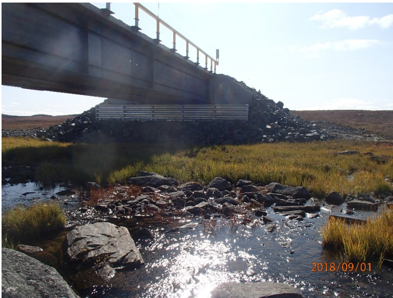
Photograph E2-32 Bridges 9 – km 44+800
