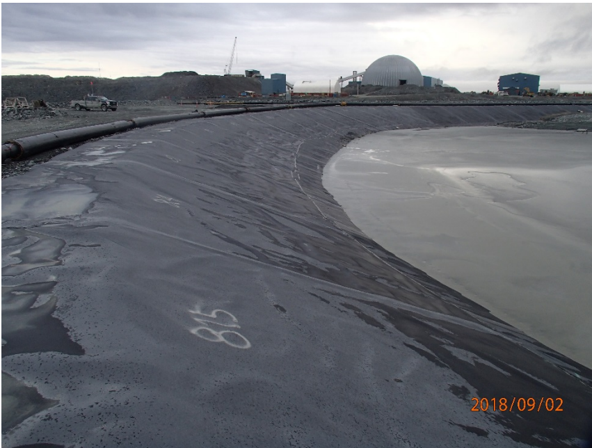
Photograph B7-14 Central Dike and Saddle Dam 5
