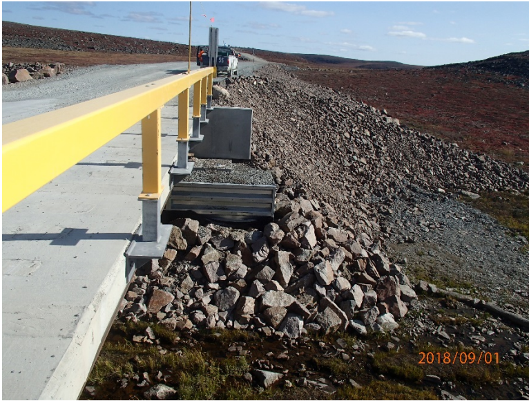
Photograph E2-15 Bridges 4 – km 20+000
