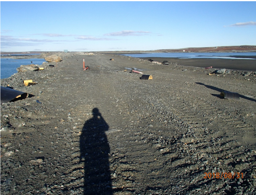
Photograph B4-4 Stormwater Dike
