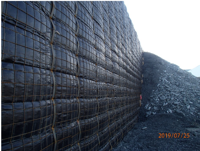
Photograph H6-5 Crusher Retaining Wall
