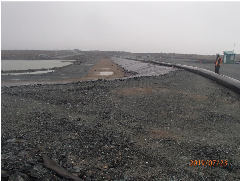
Photograph B5-4 Saddle Dam 3
