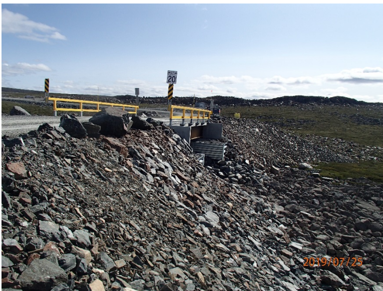
Photograph E3-4 Bridges 2 – km 10+700
