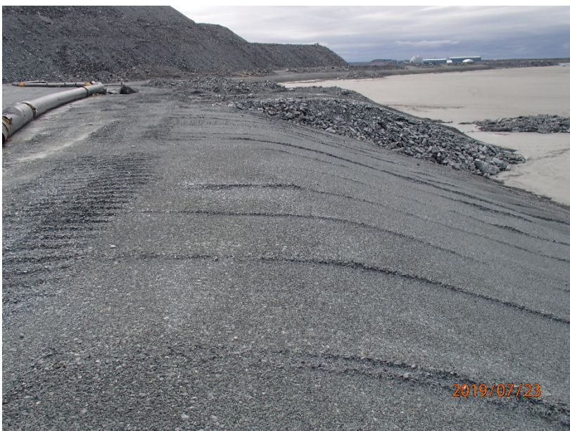
Photograph B1-4 Tailings Storage Facility
