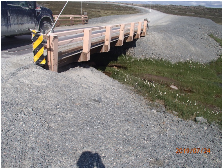
Photograph D3-7 Bridges 4 – R13 km 62+060
