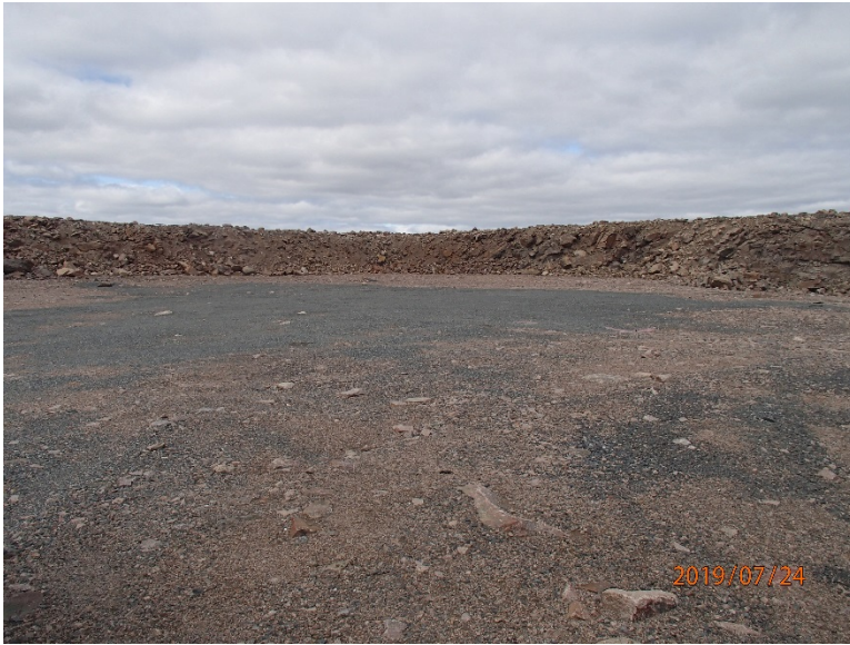
Photograph F-27: Quarry 20 – km 89+550
