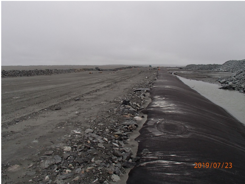
Photograph B4-1 Stormwater Dike
