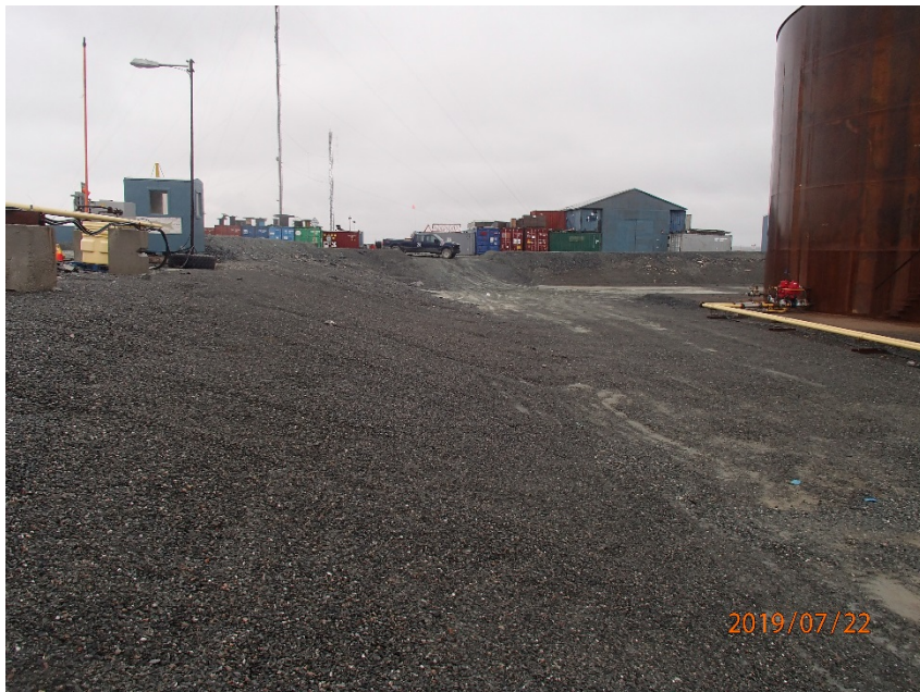
Photograph G2-6 Meadowbank Tank Farm
