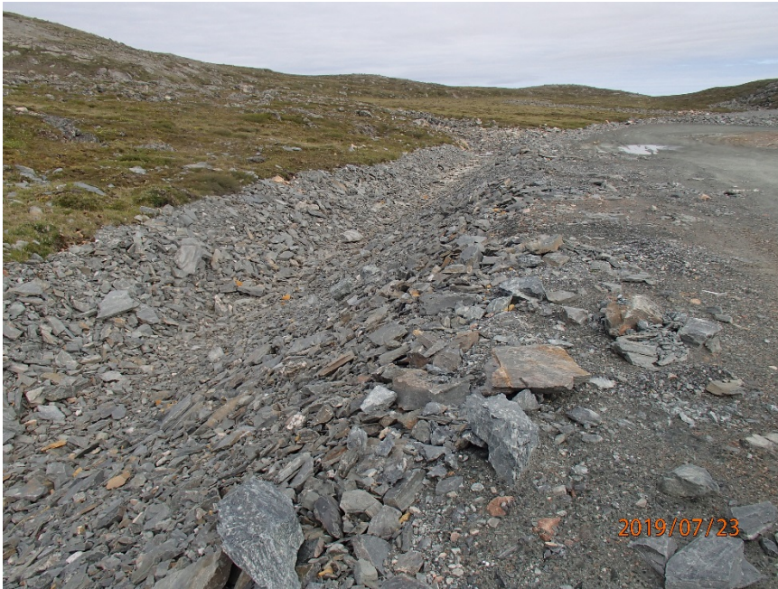
Photograph H2-13 Diversion Ditch and its Sediment and Erosion Protection Structure
