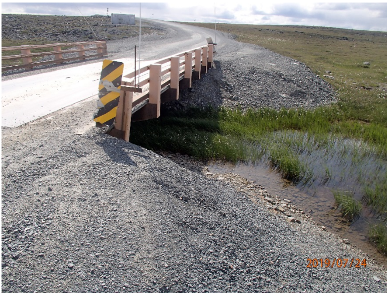
Photograph D3-8 Bridges 4 – R13 km 62+060
