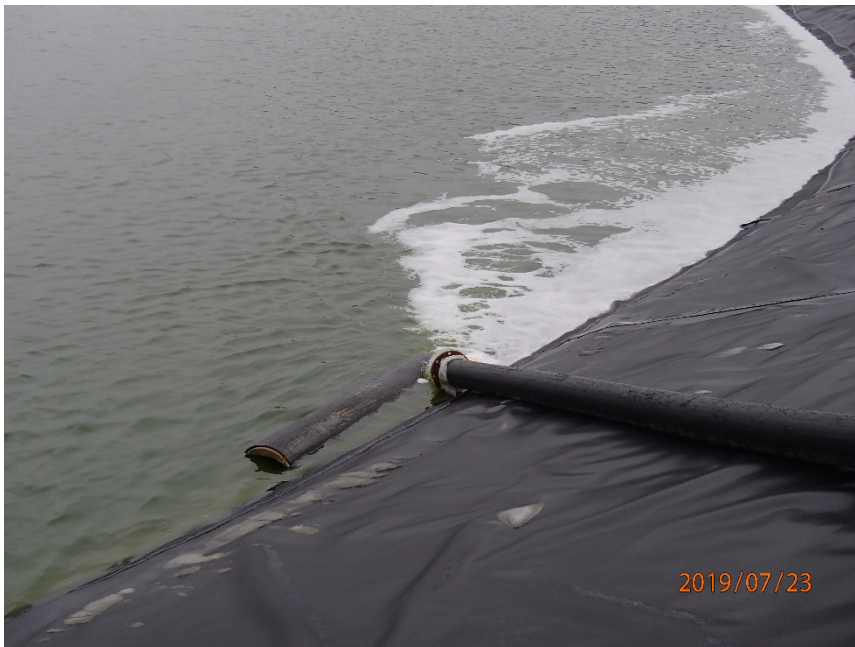
Photograph B7-10 Central Dike and Saddle Dam 5
