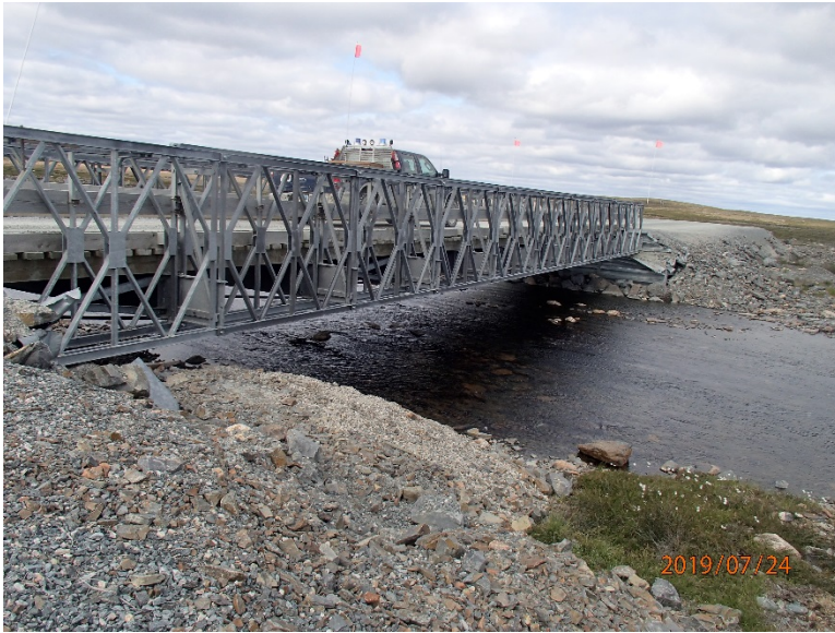
Photograph D3-9 Bridges 5 – R15 km 69+200
