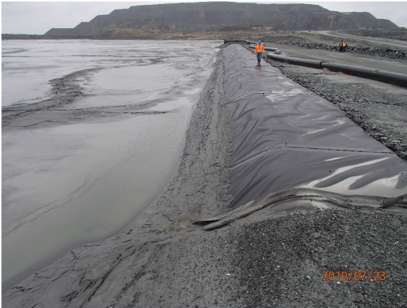
Photograph B7-1 Central Dike and Saddle Dam 5
