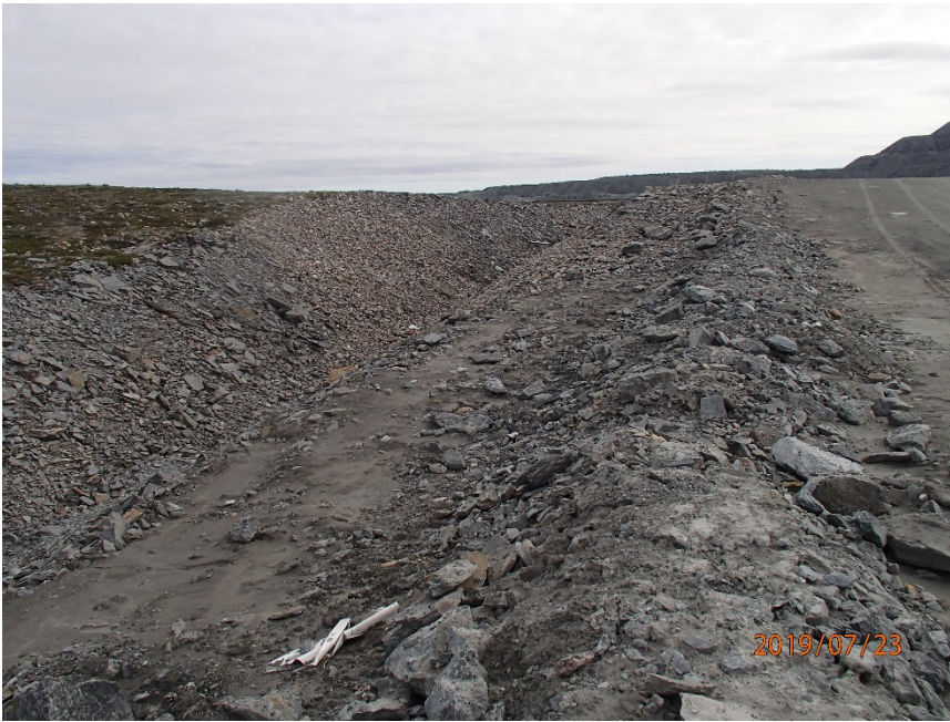
Photograph H2-17 Diversion Ditch and its Sediment and Erosion Protection Structure
