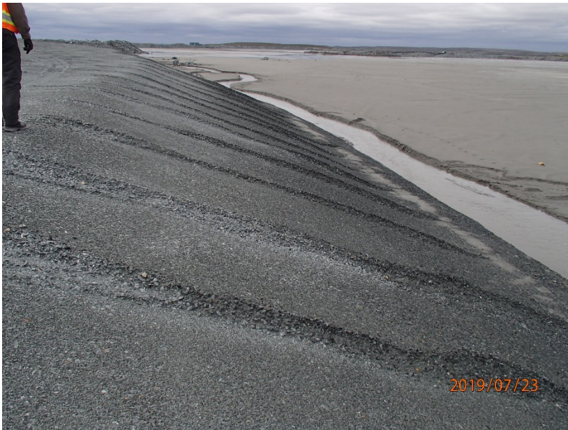
Photograph B1-9 Tailings Storage Facility
