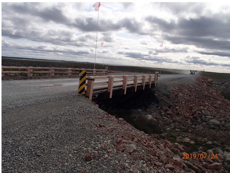
Photograph D3-14 Bridges 7 – R18 km 79+500
