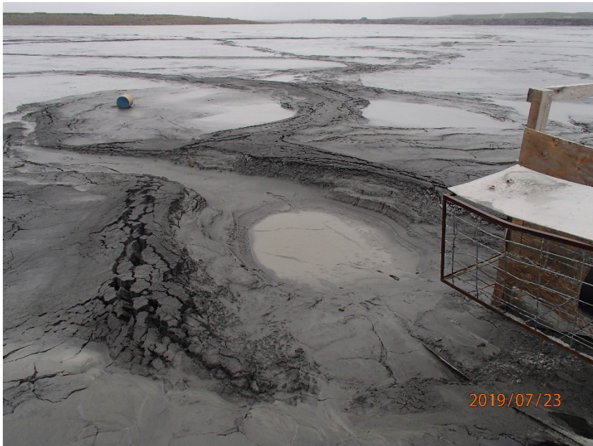
Photograph B7-3 Central Dike and Saddle Dam 5
