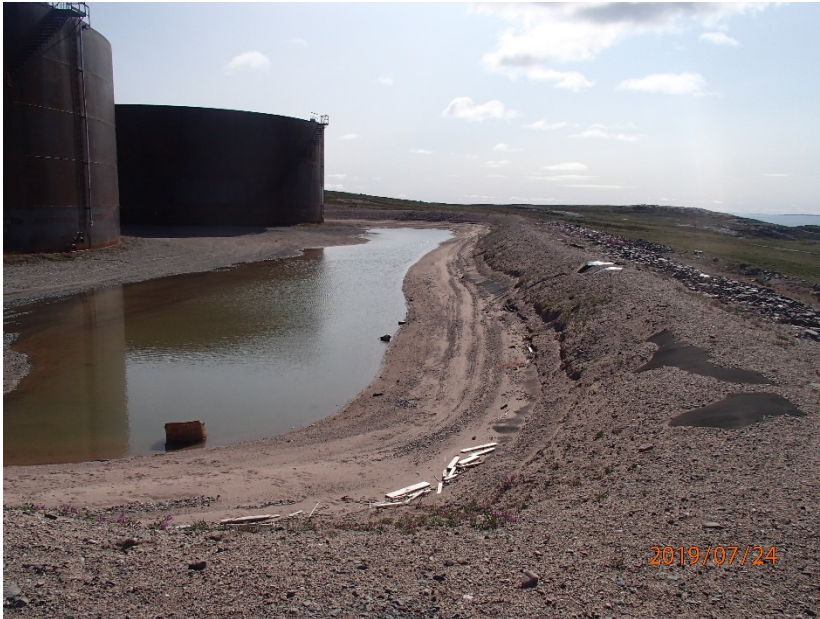
Photograph G1-7 Baker Lake Tank Farm
