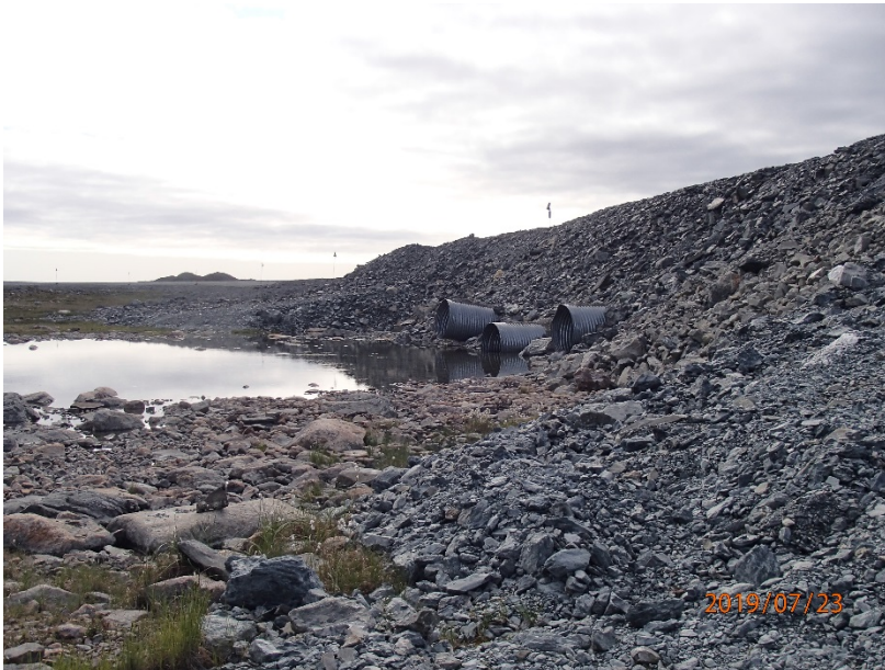
Photograph H1-2 Vault Road Culverts
