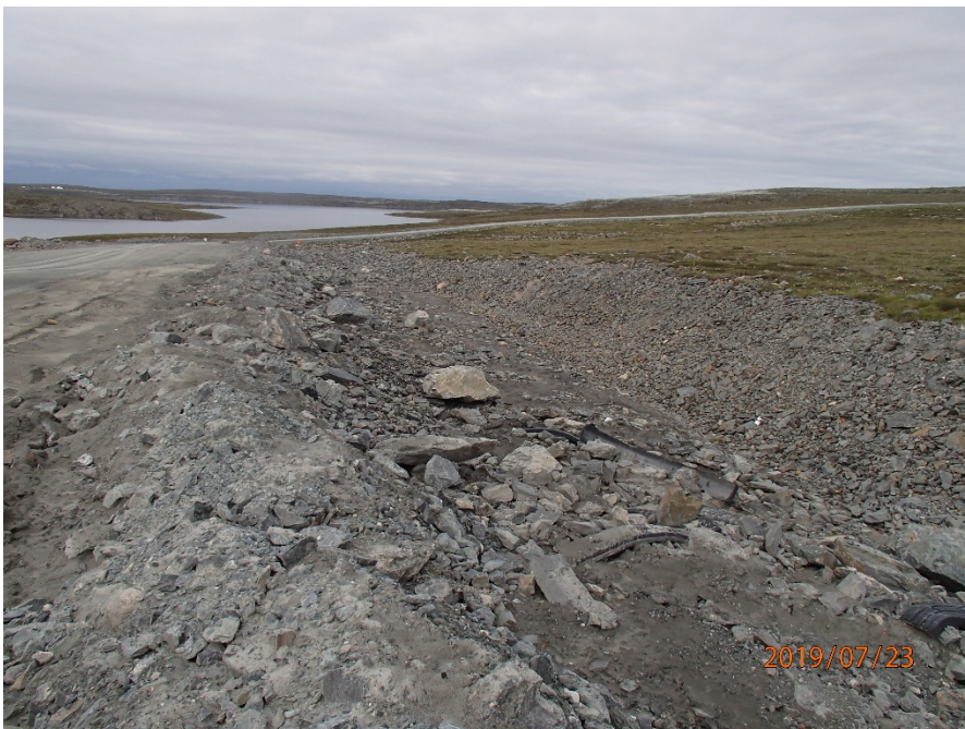
Photograph H2-18 Diversion Ditch and its Sediment and Erosion Protection Structure
