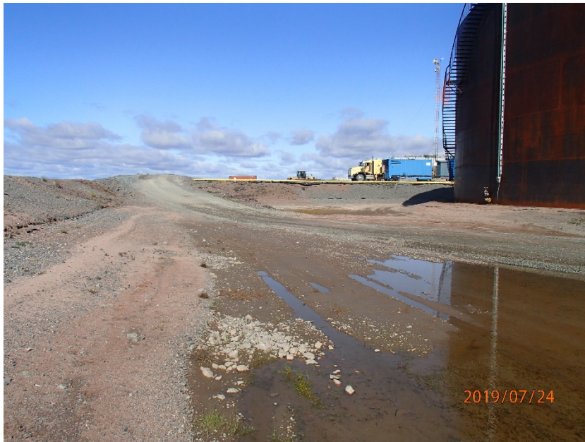
Photograph G1-3 Baker Lake Tank Farm
