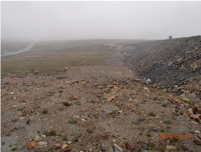
Photograph B2-1 Saddle Dam 1
