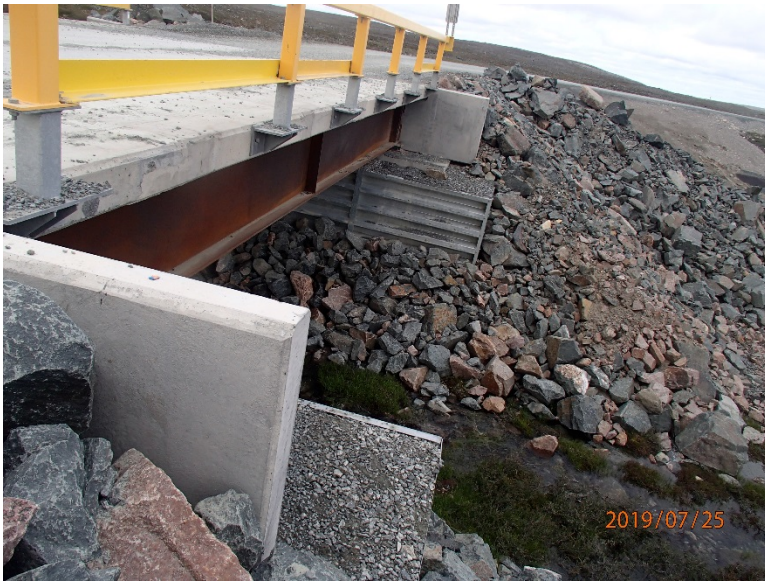
Photograph E3-15 Bridges 8 – km 43+500
