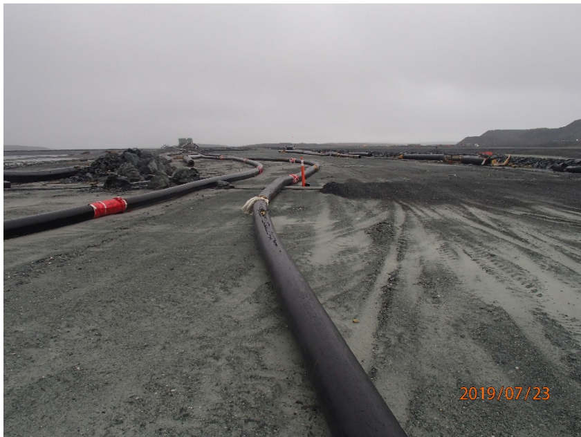
Photograph B6-6 Saddle Dam 4
