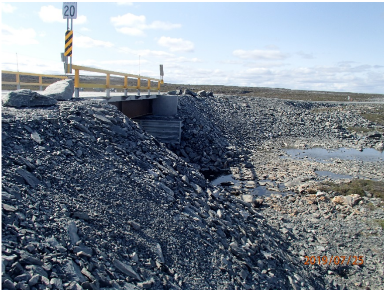
Photograph E3-1 Bridges 1 – km 3+400
