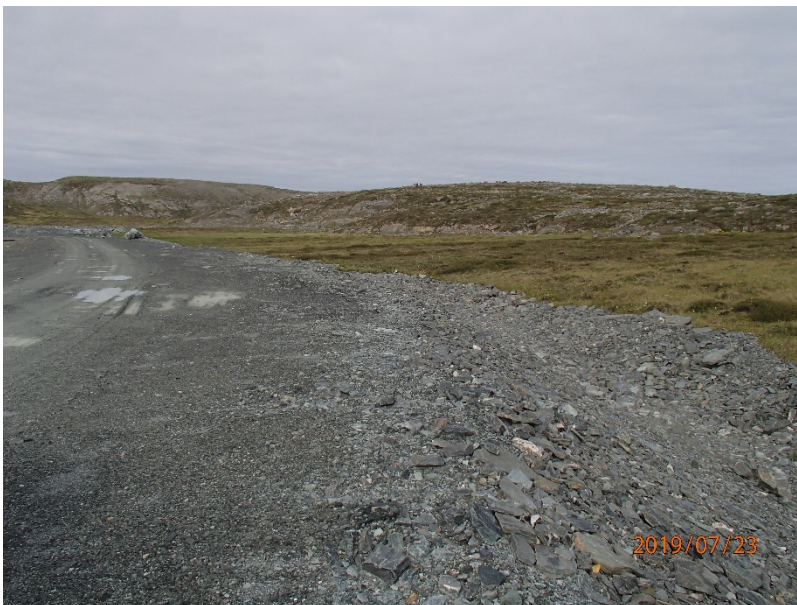
Photograph H2-12 Diversion Ditch and its Sediment and Erosion Protection Structure
