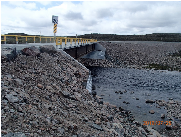
Photograph E3-13 Bridges 7 – km 32+300
