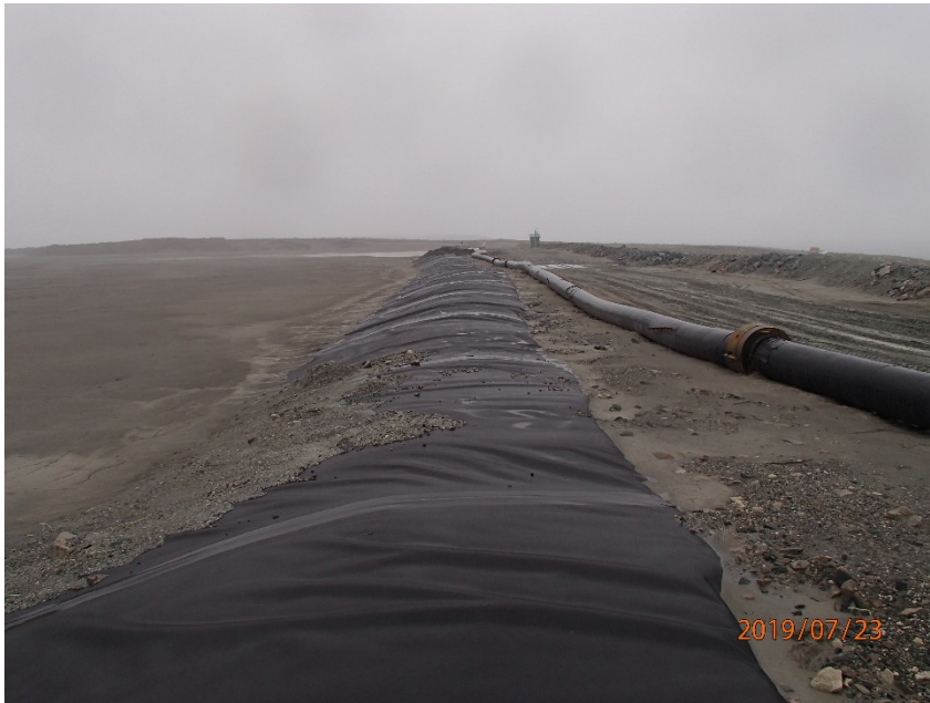
Photograph B2-5 Saddle Dam 1
