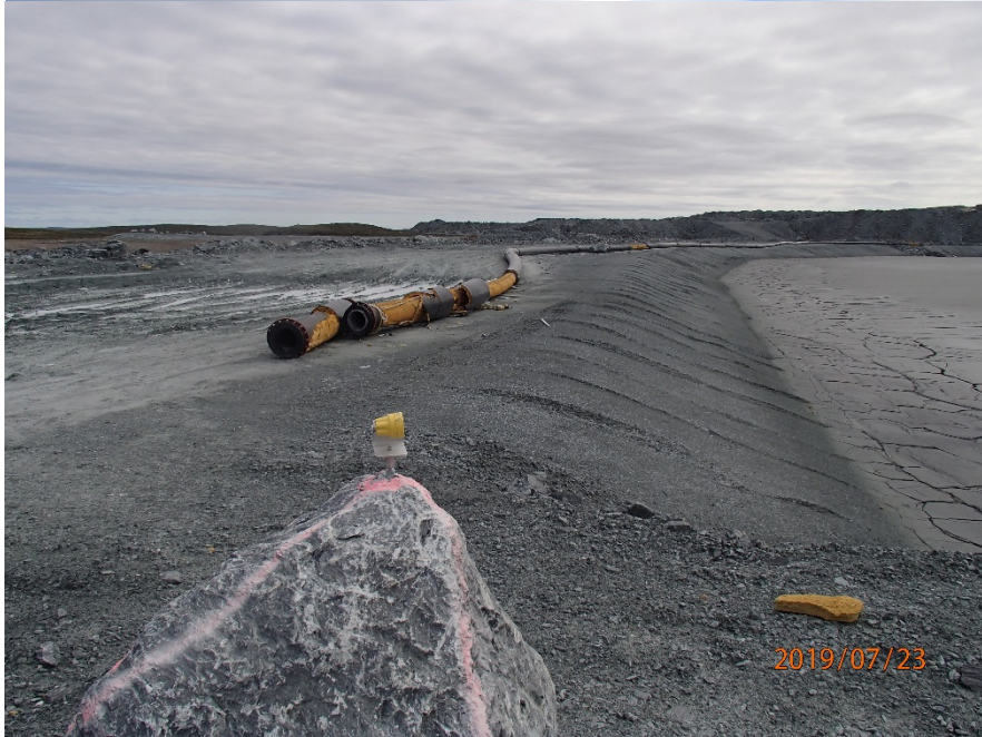
Photograph B1-5 Tailings Storage Facility
