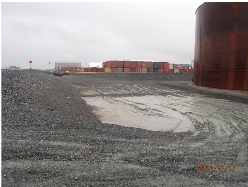
Photograph G2-2 Meadowbank Tank Farm
