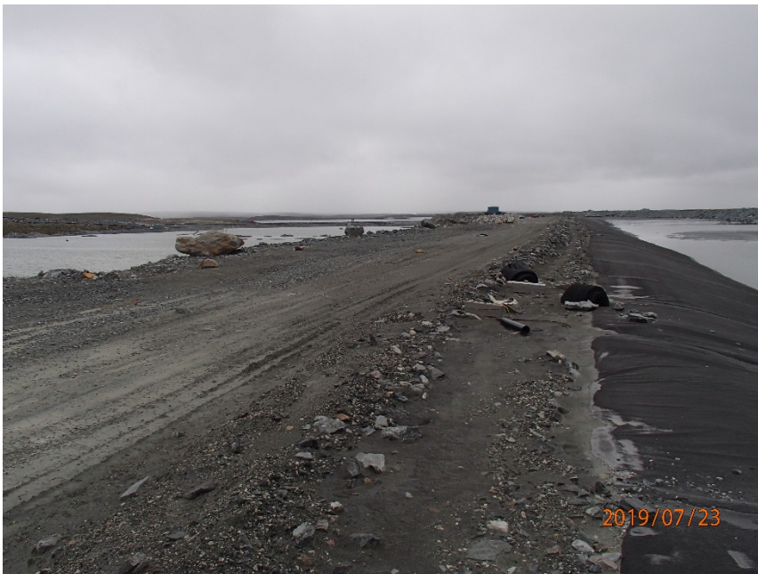
Photograph B4-4 Stormwater Dike
