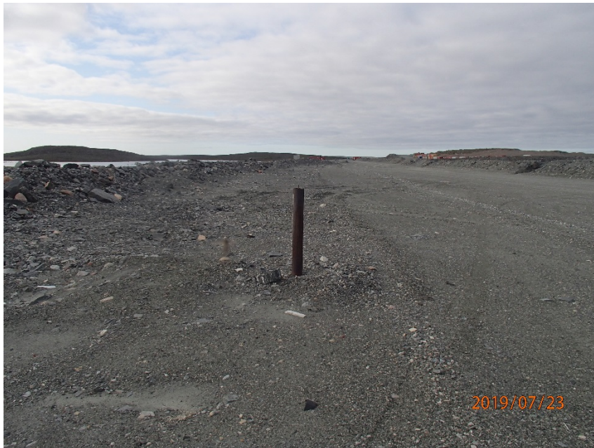
Photograph A1-5 East Dike
