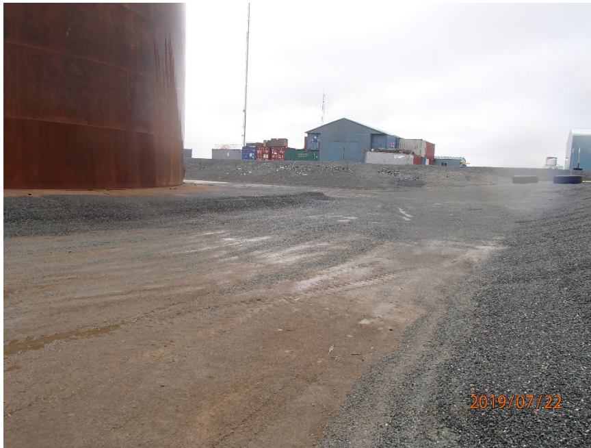
Photograph G2-3 Meadowbank Tank Farm
