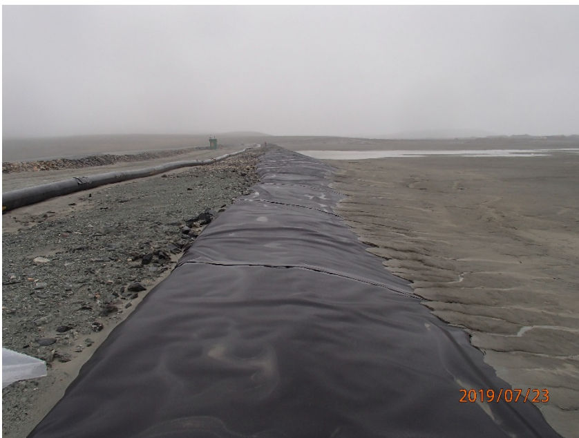
Photograph B2-8 Saddle Dam 1
