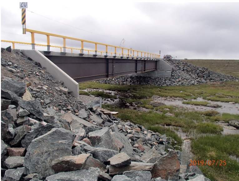
Photograph E3-18 Bridges 9 – km 44+800
