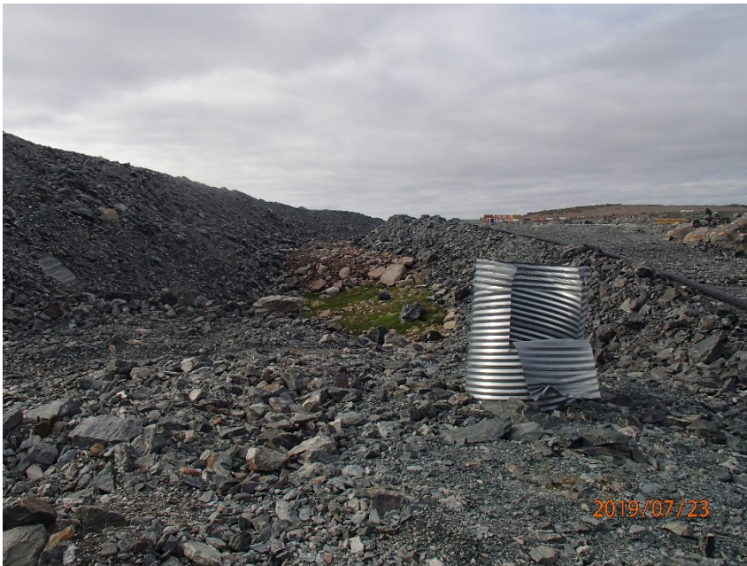
Photograph A1-10 East Dike
