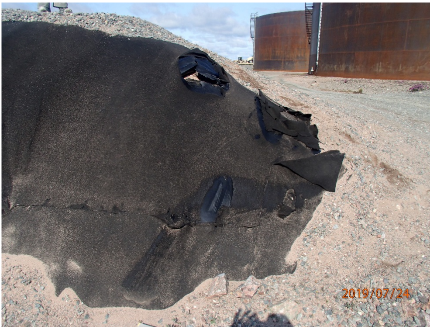
Photograph G1-6 Baker Lake Tank Farm
