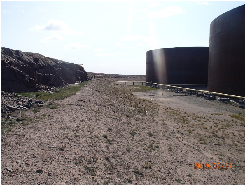
Photograph G1-13 Baker Lake Tank Farm
