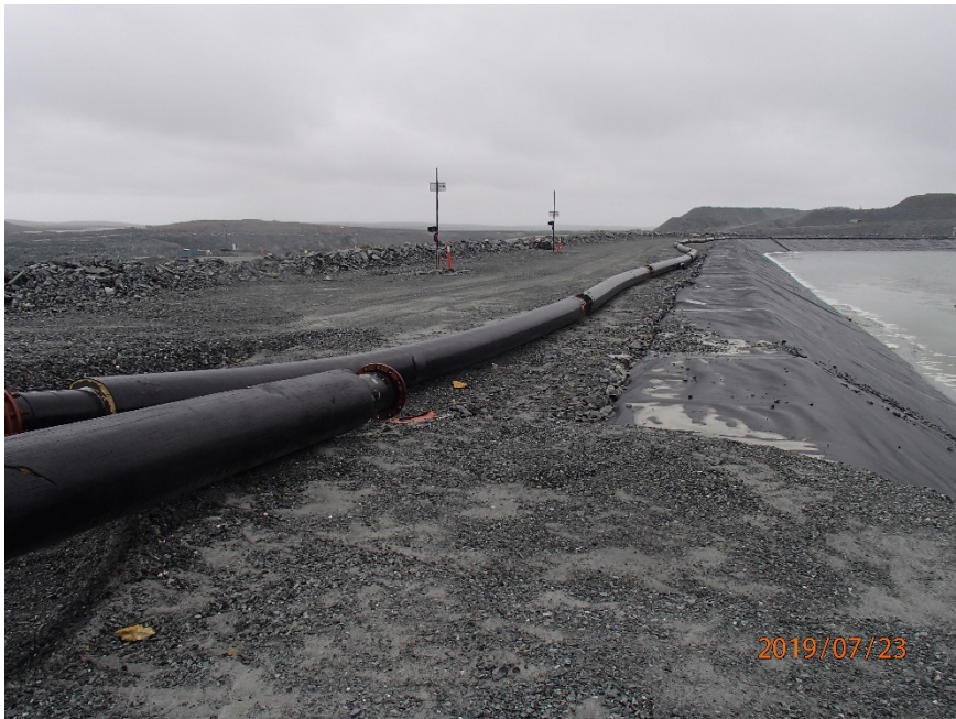
Photograph B7-4 Central Dike and Saddle Dam 5
