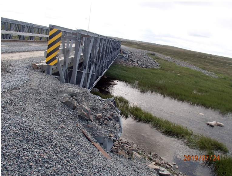
Photograph D3-4 Bridges 2 – R05 km 17+600
