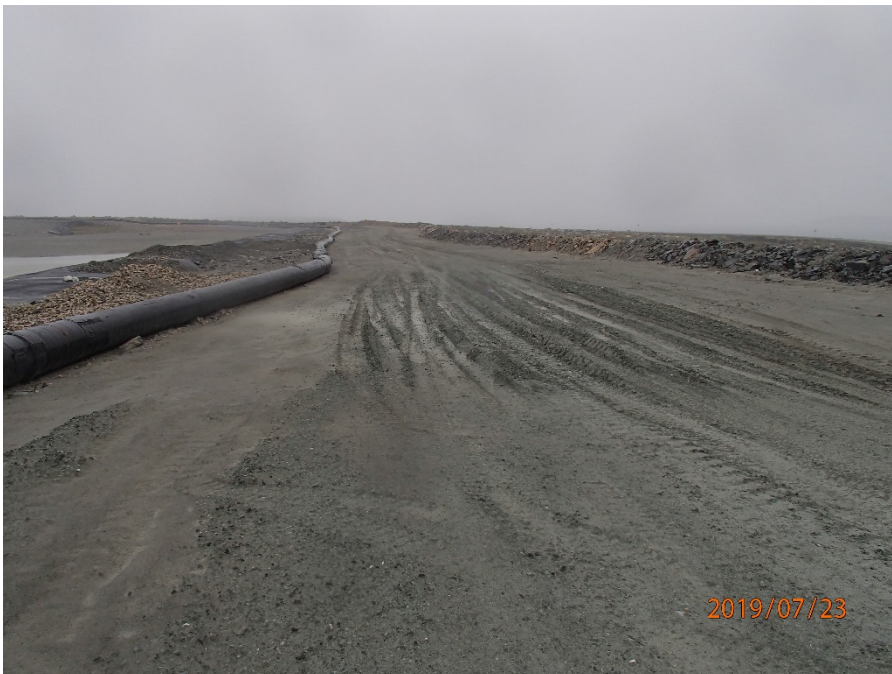
Photograph B2-4 Saddle Dam 1
