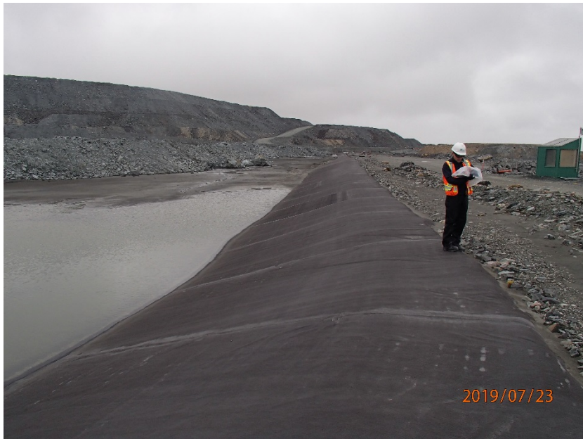
Photograph B4-2 Stormwater Dike
