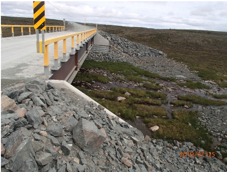
Photograph E3-17 Bridges 9 – km 44+800
