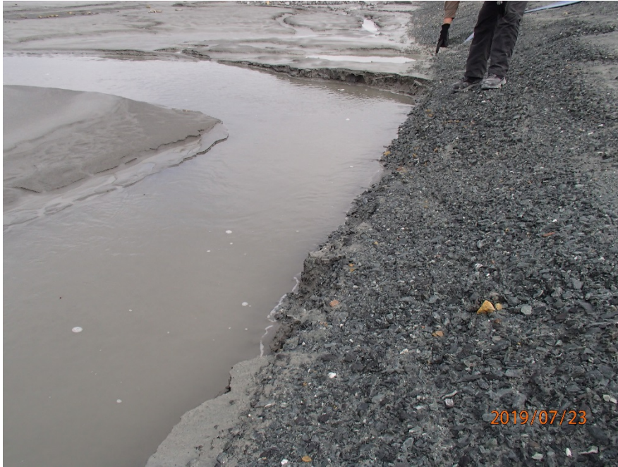
Photograph B1-7 Tailings Storage Facility
