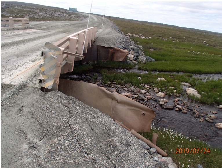
Photograph D3-16 Bridges 8 – R19 km 83+150
