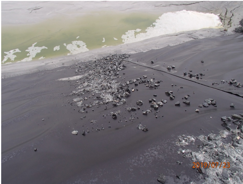
Photograph B7-8 Central Dike and Saddle Dam 5
