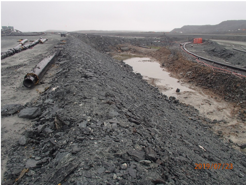
Photograph B6-7 Saddle Dam 4
