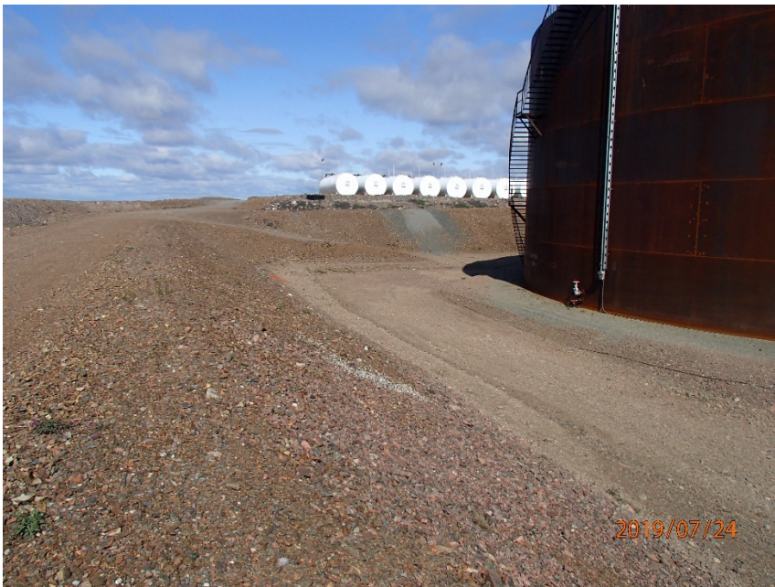
Photograph G1-14 Baker Lake Tank Farm
