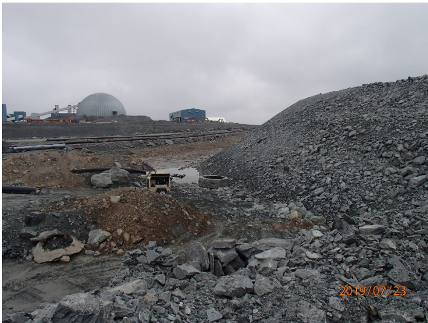
Photograph B7-12 Central Dike and Saddle Dam 5
