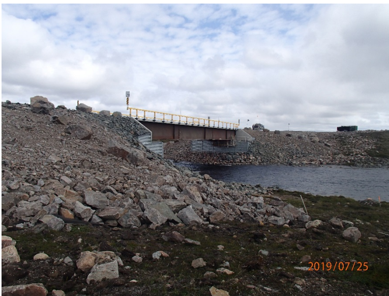
Photograph E3-14 Bridges 7 – km 32+300
