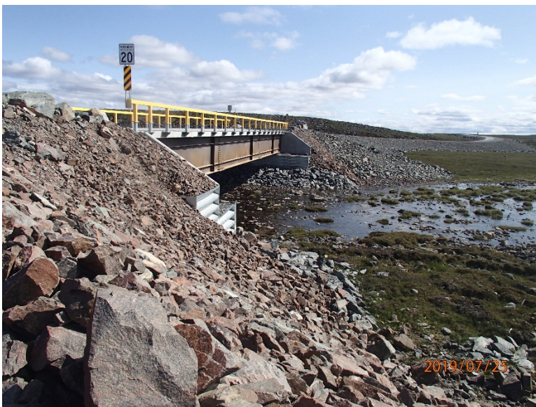
Photograph E3-6 Bridges 3 – km 16+000
