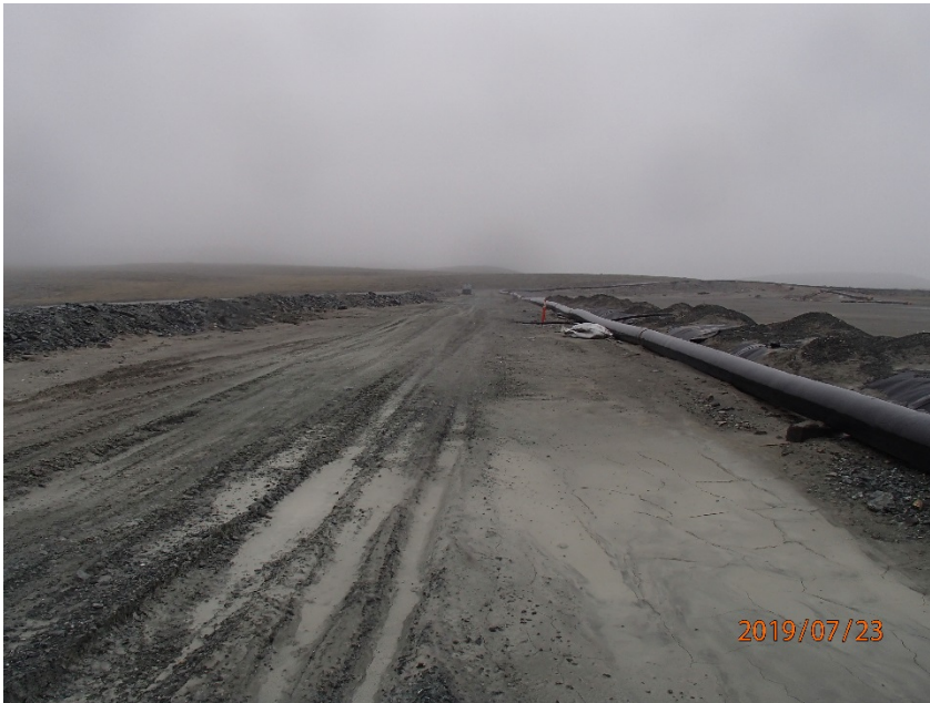
Photograph B2-3 Saddle Dam 1
