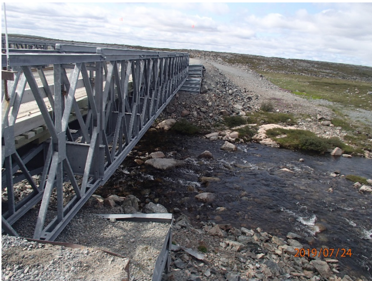
Photograph D3-2 Bridges 1 – R02 km 8+750
