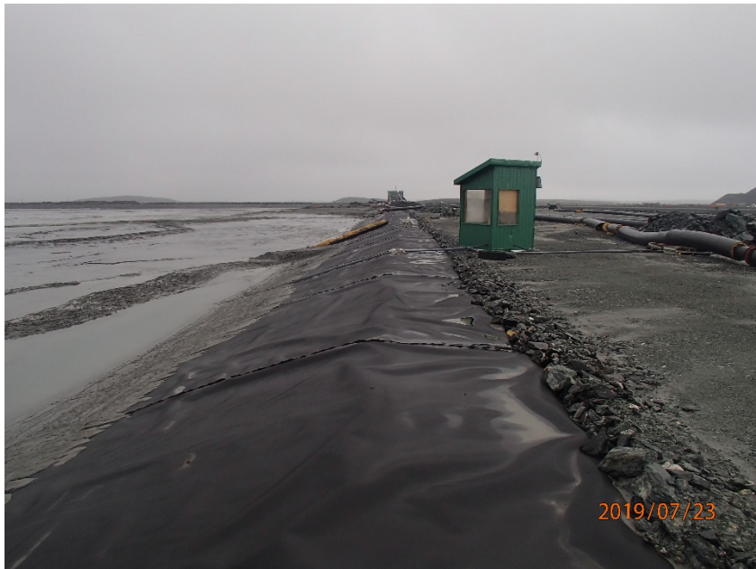
Photograph B6-5 Saddle Dam 4
