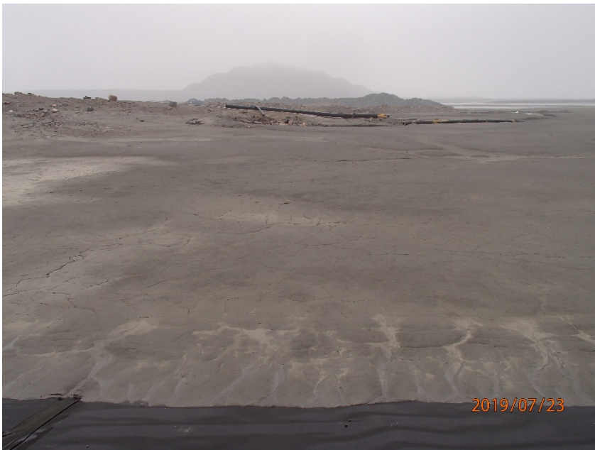
Photograph B2-10 Saddle Dam 1
