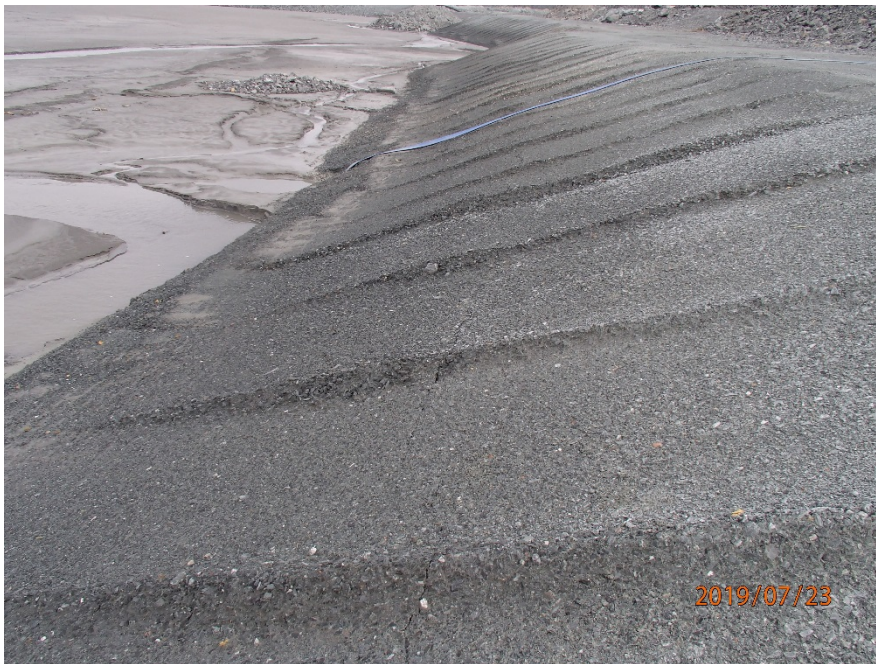
Photograph B1-8 Tailings Storage Facility
