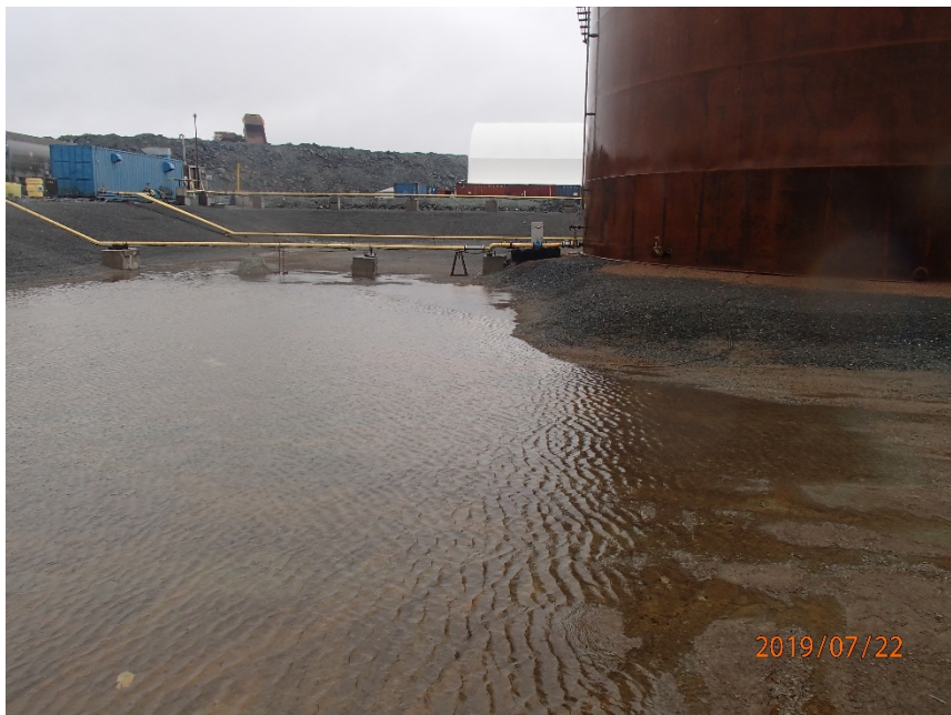
Photograph G2-4 Meadowbank Tank Farm
