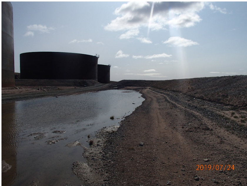
Photograph G1-4 Baker Lake Tank Farm
