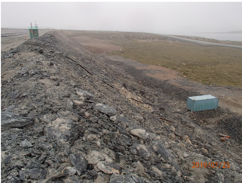
Photograph B2-2 Saddle Dam 1
