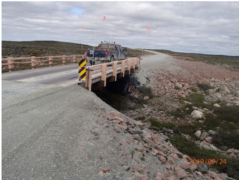
Photograph D3-13 Bridges 7 – R18 km 79+500
