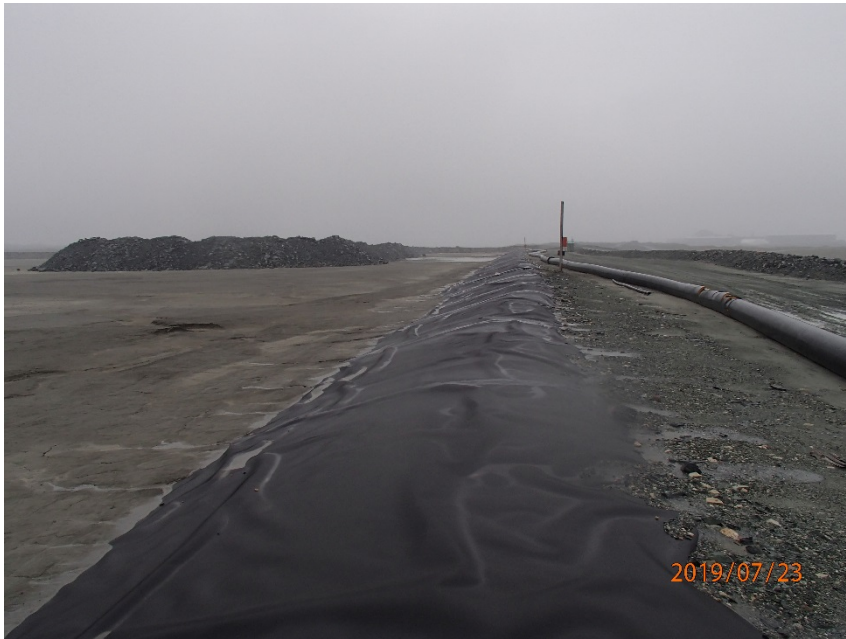
Photograph B3-1 Saddle Dam 2
