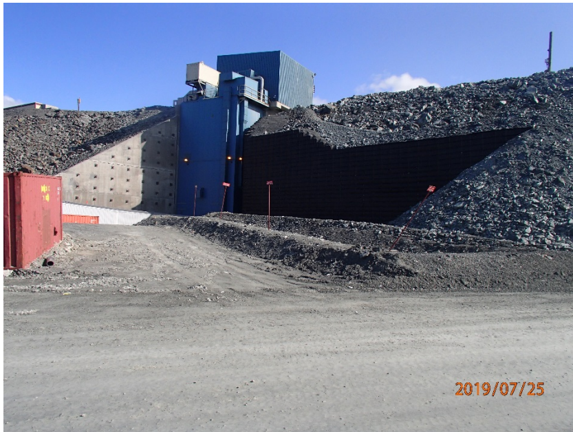
Photograph H6-1 Crusher Retaining Wall
