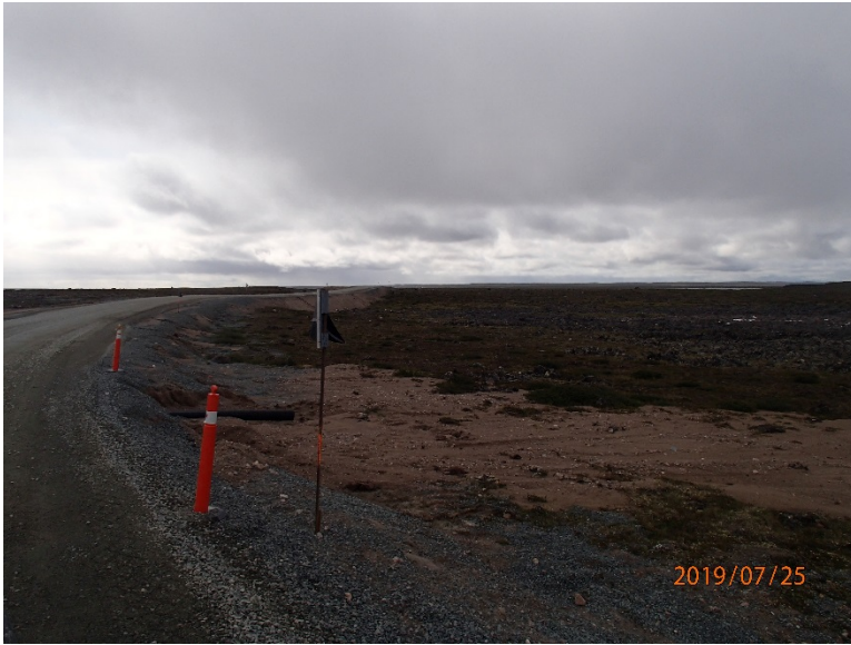
Photograph E2-1: Unnamed pipe, km 61+170
