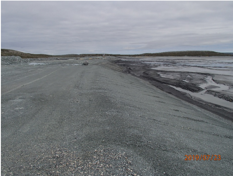
Photograph B1-1 Tailings Storage Facility
