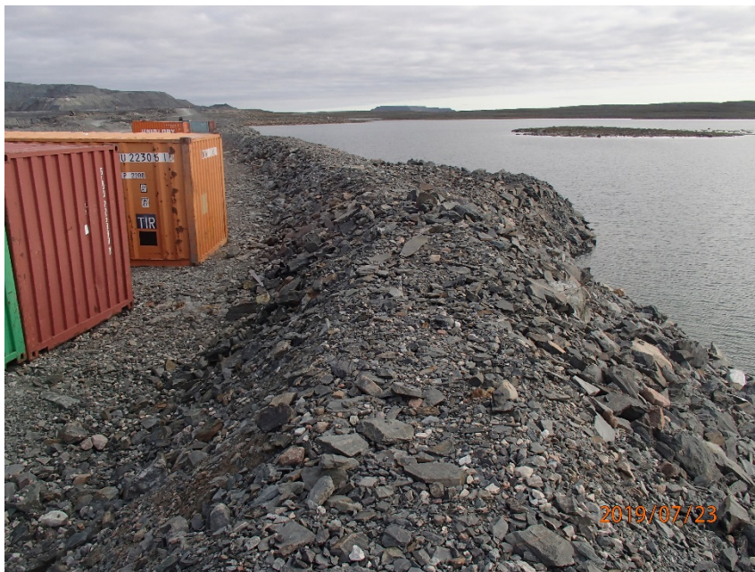
Photograph A1-6 East Dike
