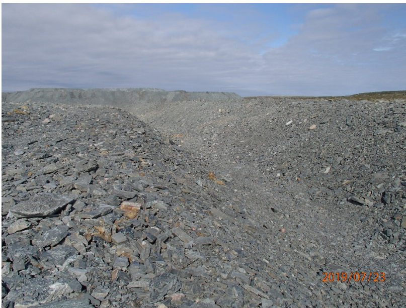
Photograph H2-2 Diversion Ditch and its Sediment and Erosion Protection Structure
