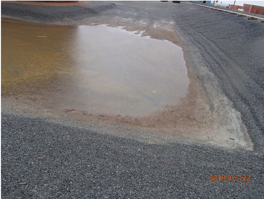
Photograph G2-7 Meadowbank Tank Farm
