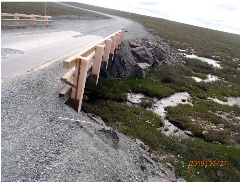
Photograph D3-12 Bridges 6 – R16 km 73+800
