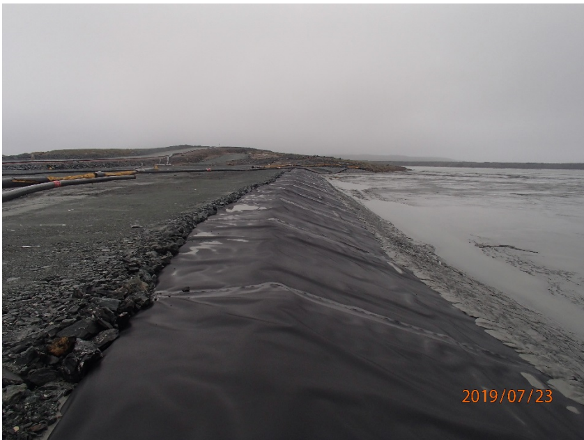
Photograph B6-4 Saddle Dam 4
