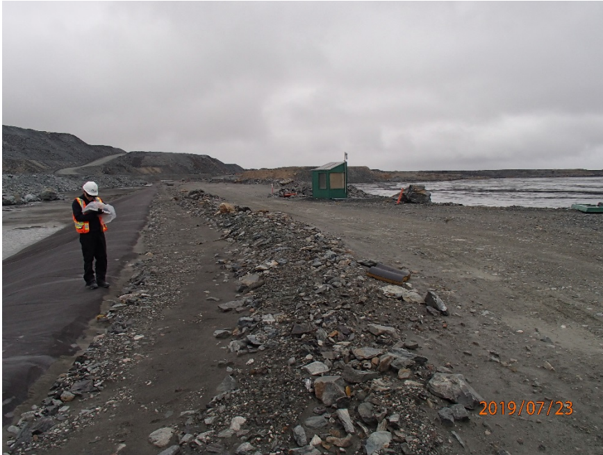
Photograph B4-5 Stormwater Dike
