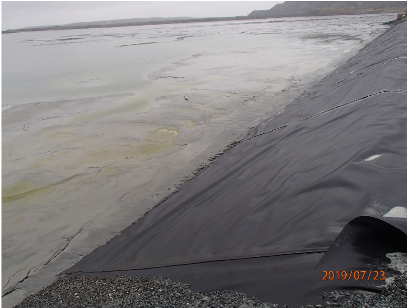
Photograph B7-7 Central Dike and Saddle Dam 5
