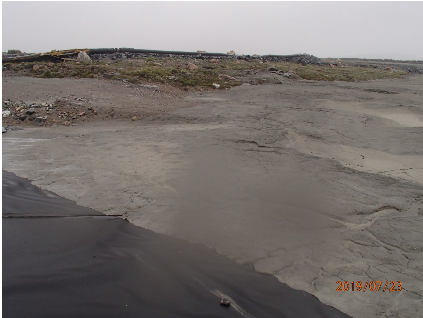
Photograph B3-2 Saddle Dam 2
