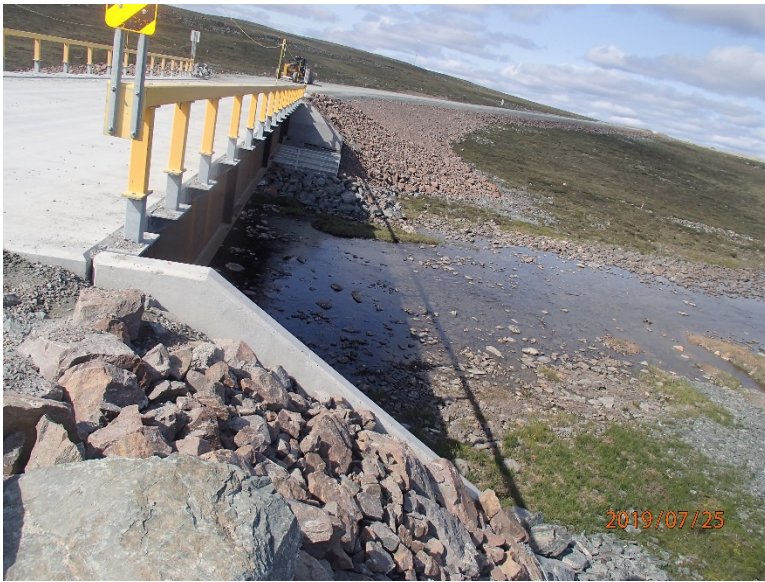
Photograph E3-5 Bridges 3 – km 16+000
