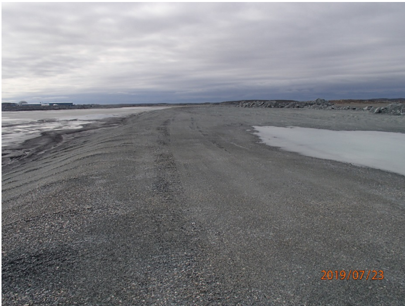
Photograph B1-2 Tailings Storage Facility
