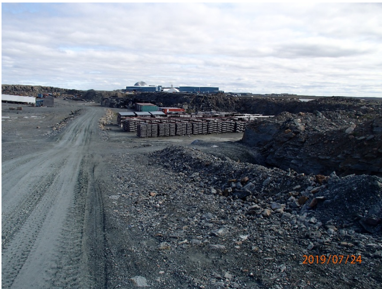
Photograph F-28: Quarry 23 (Airstrip Quarry)
