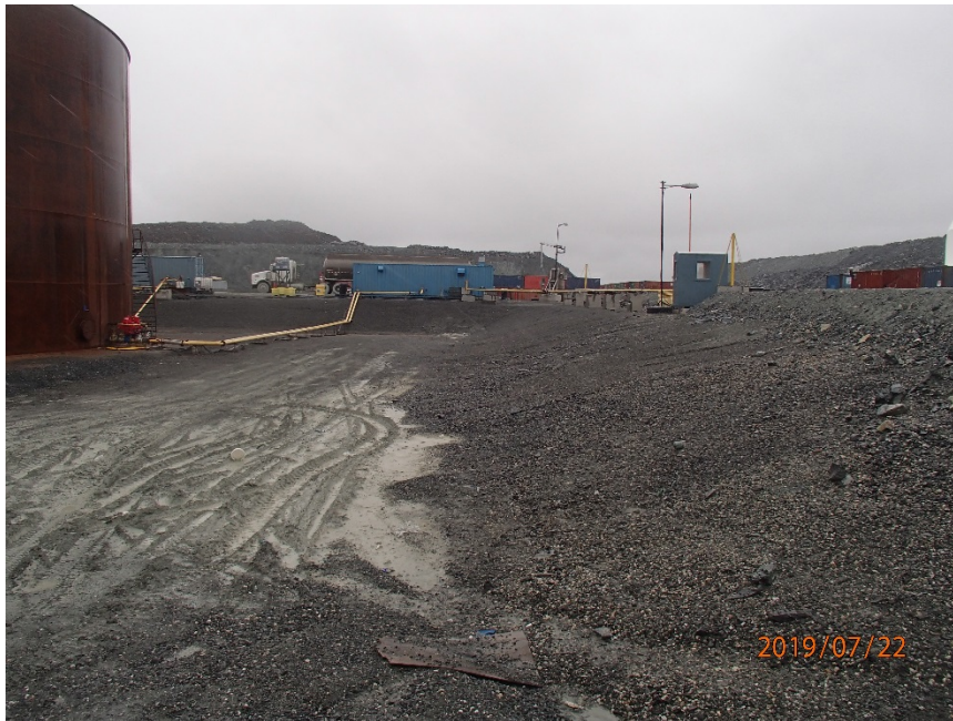
Photograph G2-1 Meadowbank Tank Farm
