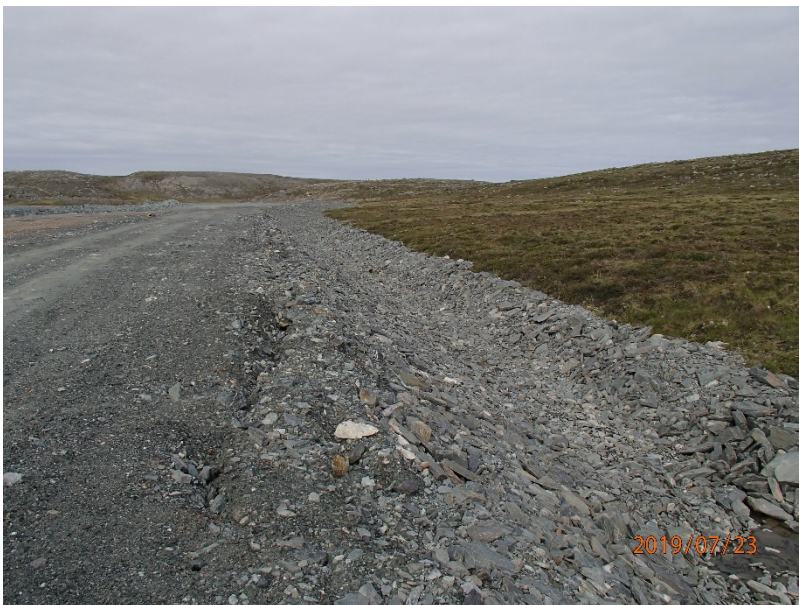
Photograph H2-10 Diversion Ditch and its Sediment and Erosion Protection Structure
