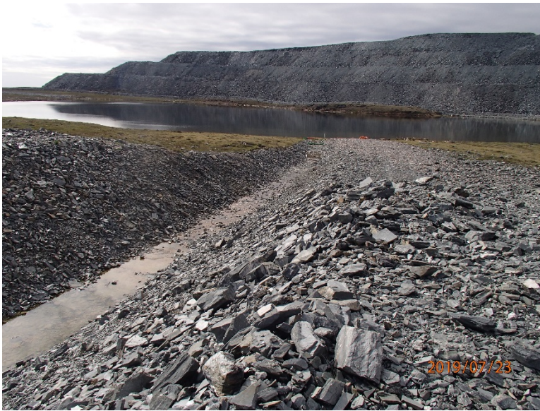
Photograph H2-3 Diversion Ditch and its Sediment and Erosion Protection Structure
