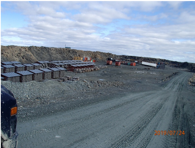
Photograph F-29: Quarry 23 (Airstrip Quarry)
