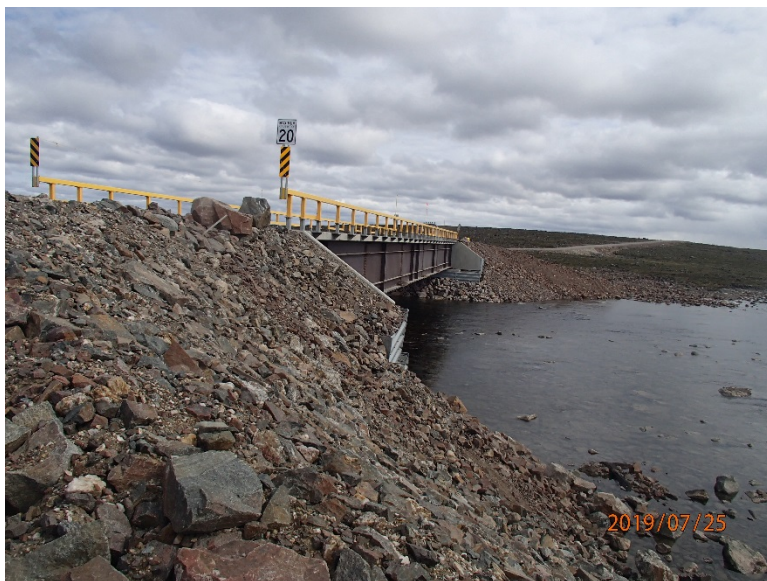
Photograph E3-10 Bridges 5 – km 23+900
