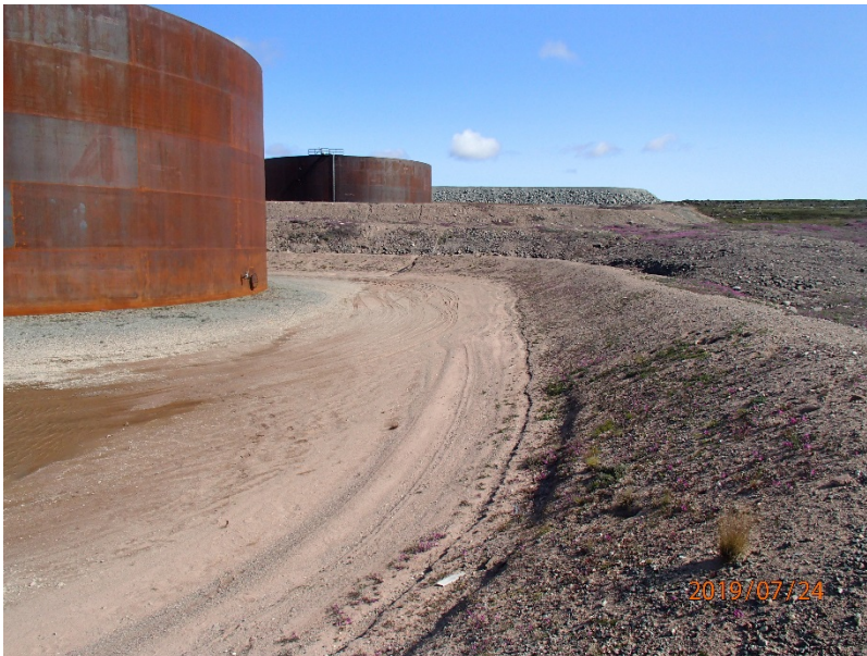
Photograph G1-9 Baker Lake Tank Farm
