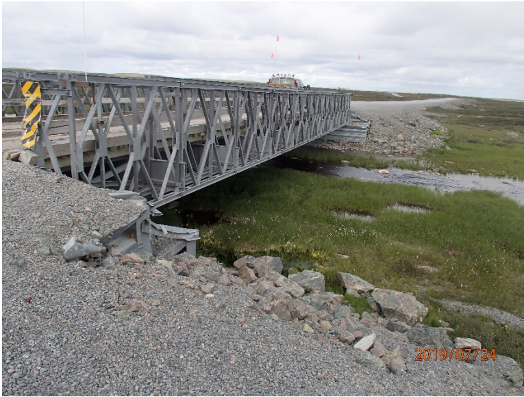
Photograph D3-3 Bridges 2 – R05 km 17+600
