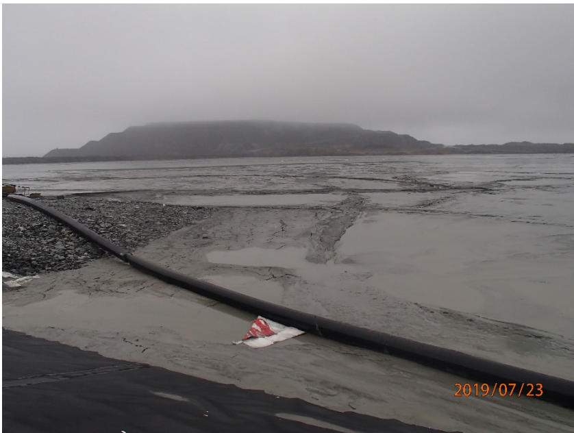
Photograph B6-2 Saddle Dam 4
