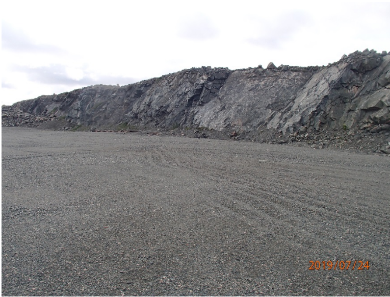
Photograph F-3: Quarry 3 – km 23+700
