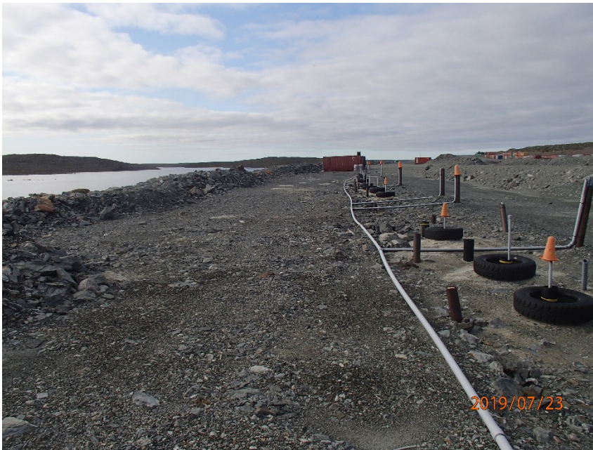
Photograph A1-3 East Dike
