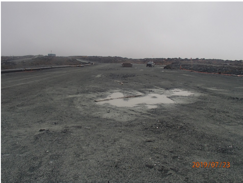
Photograph B5-2 Saddle Dam 3
