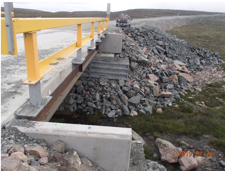
Photograph E3-16 Bridges 8 – km 43+500
