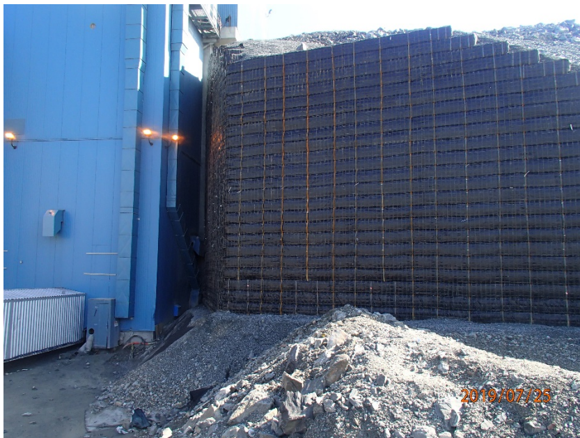
Photograph H6-2 Crusher Retaining Wall
