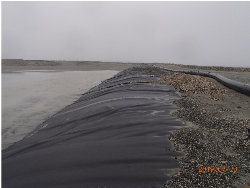
Photograph B2-6 Saddle Dam 1
