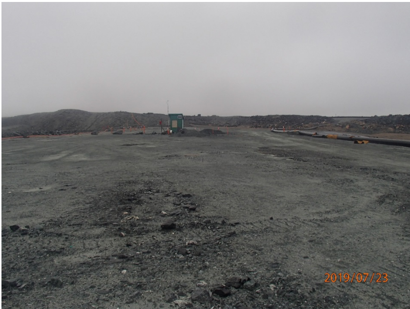
Photograph B5-3 Saddle Dam 3
