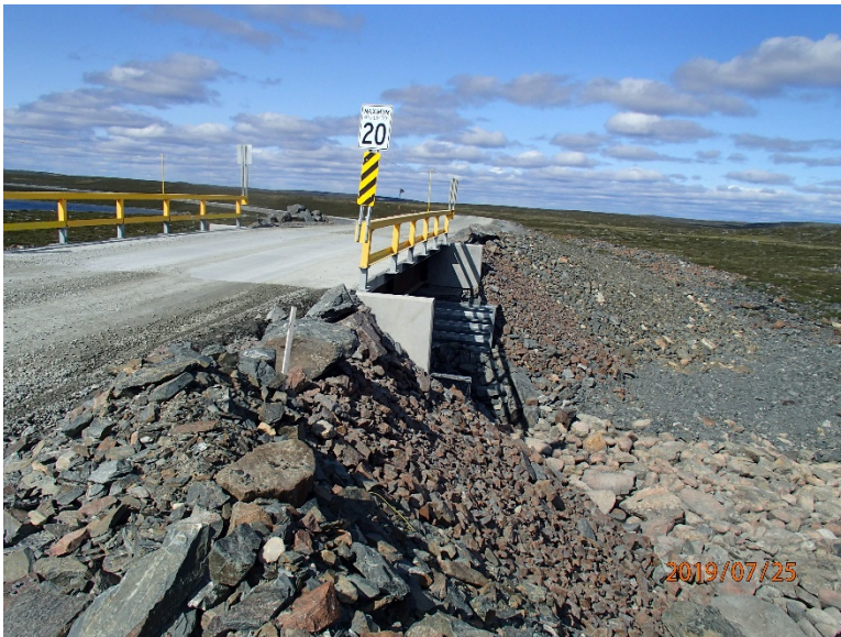
Photograph E3-3 Bridges 2 – km 10+700
