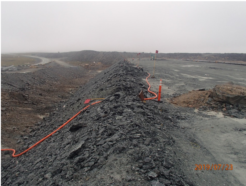
Photograph B5-1 Saddle Dam 3
