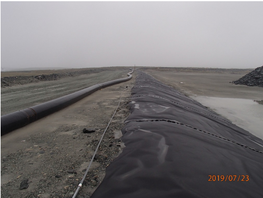
Photograph B3-4 Saddle Dam 2
