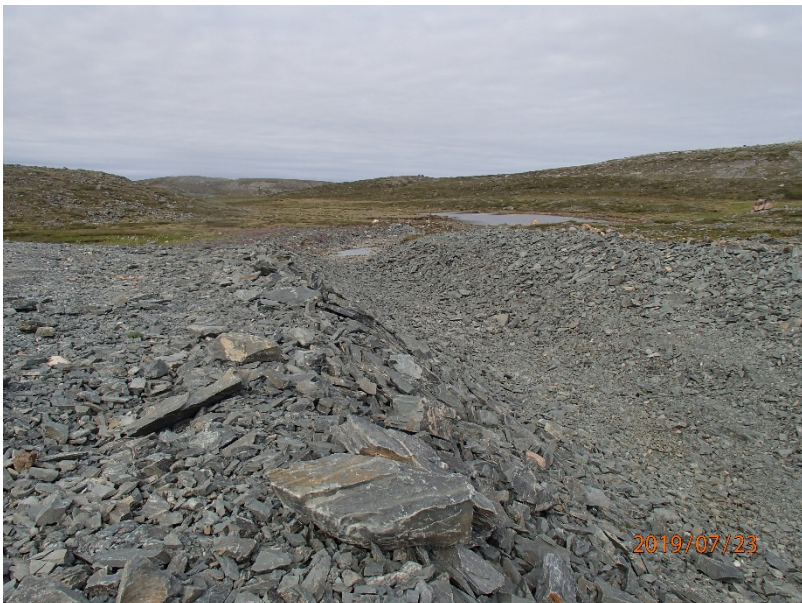
Photograph H2-8 Diversion Ditch and its Sediment and Erosion Protection Structure
