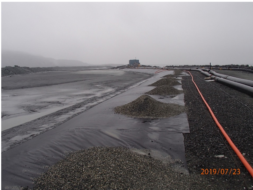
Photograph B4-6 Stormwater Dike
