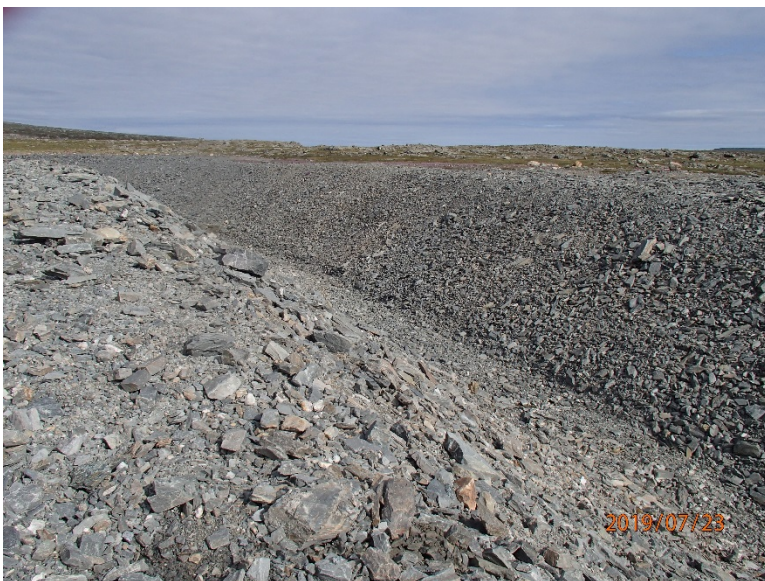
Photograph H2-4 Diversion Ditch and its Sediment and Erosion Protection Structure
