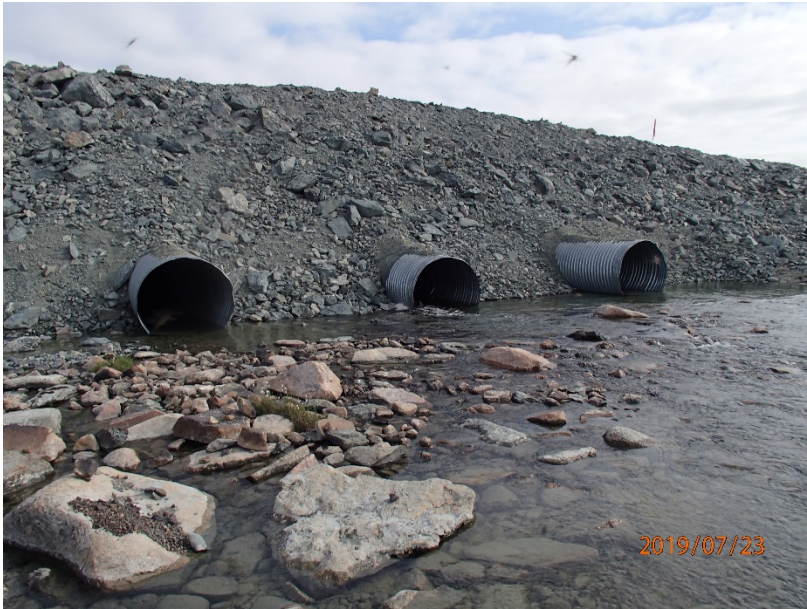
Photograph H1-1 Vault Road Culverts
