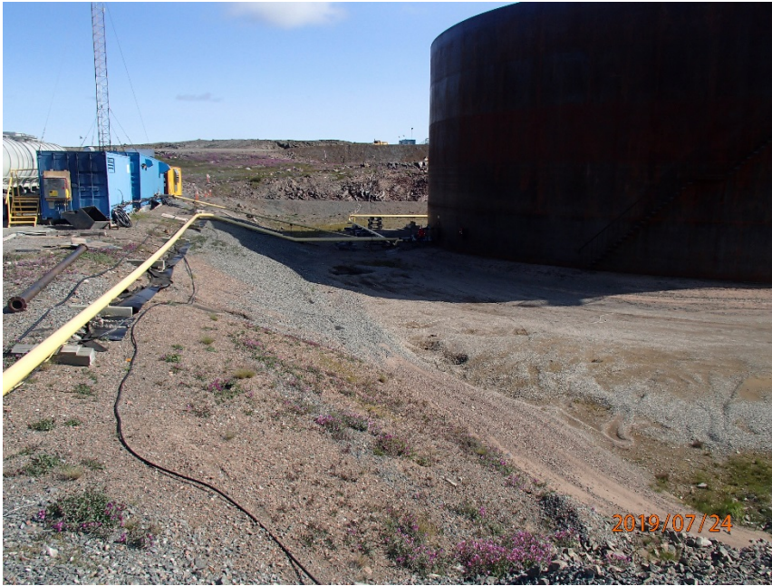
Photograph G1-1 Baker Lake Tank Farm
