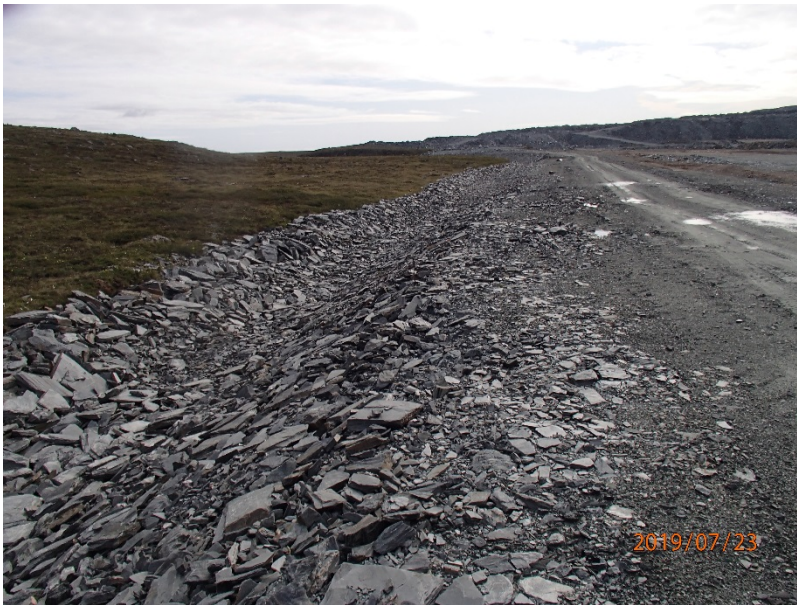
Photograph H2-11 Diversion Ditch and its Sediment and Erosion Protection Structure
