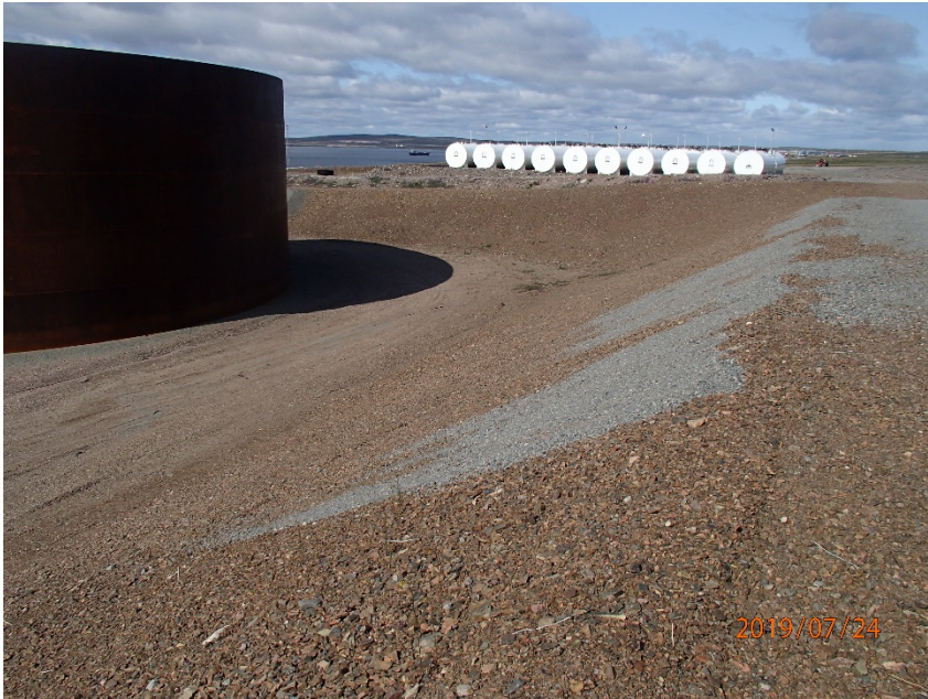
Photograph G1-19 Baker Lake Tank Farm
