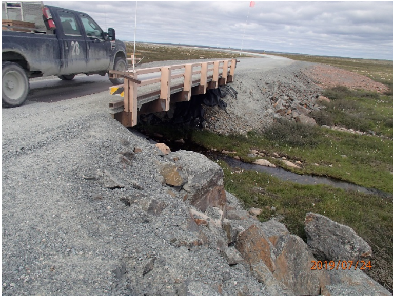
Photograph D3-11 Bridges 6 – R16 km 73+800
