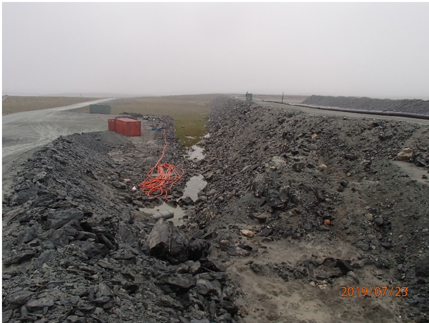
Photograph B3-6 Saddle Dam 2
