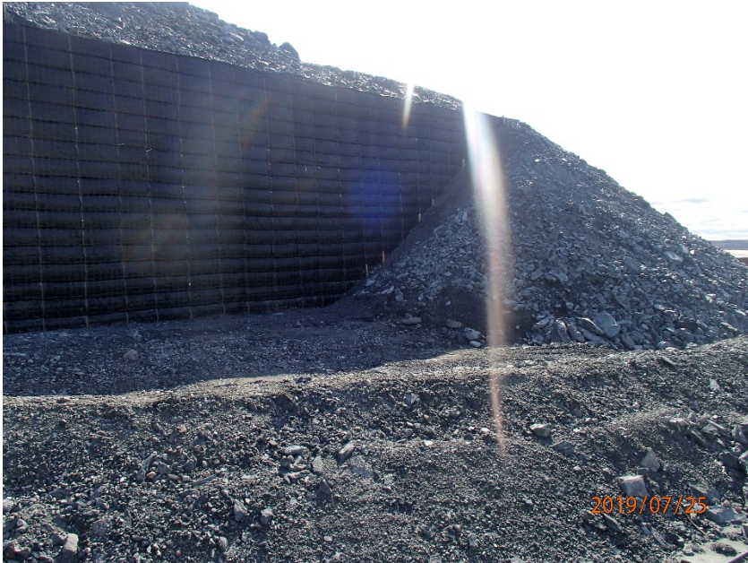
Photograph H6-3 Crusher Retaining Wall
