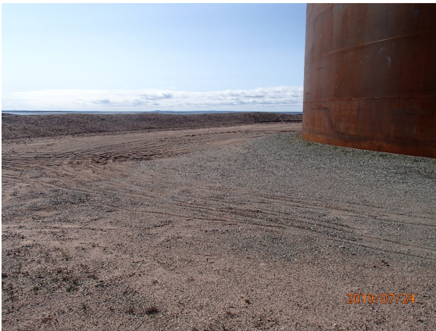
Photograph G1-10 Baker Lake Tank Farm
