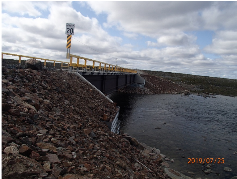
Photograph E3-9 Bridges 5 – km 23+900
