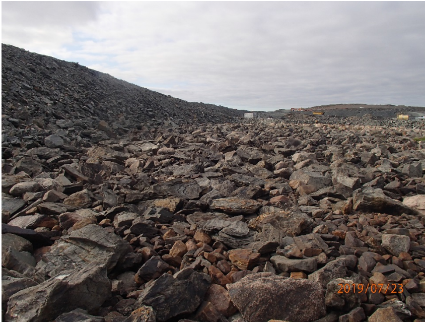
Photograph A1-9 East Dike
