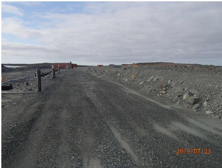
Photograph A1-2 East Dike
