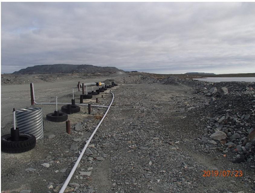
Photograph A1-4 East Dike
