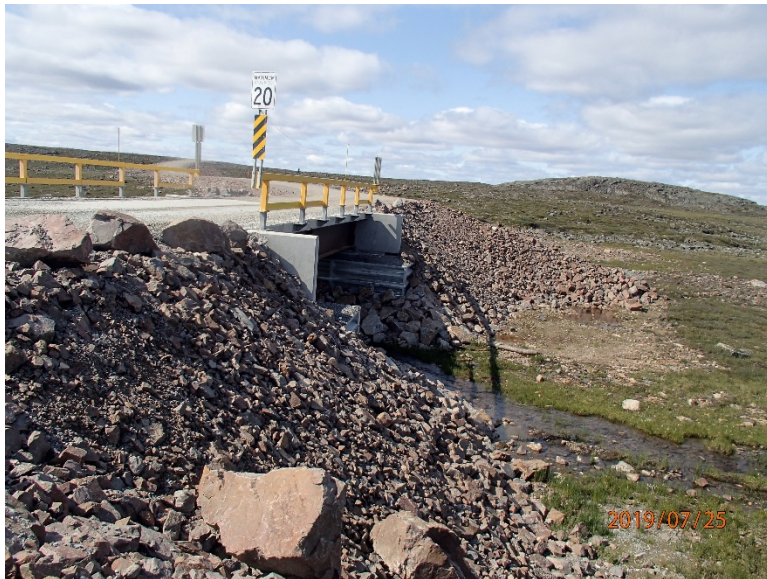
Photograph E3-7 Bridges 4 – km 20+000
