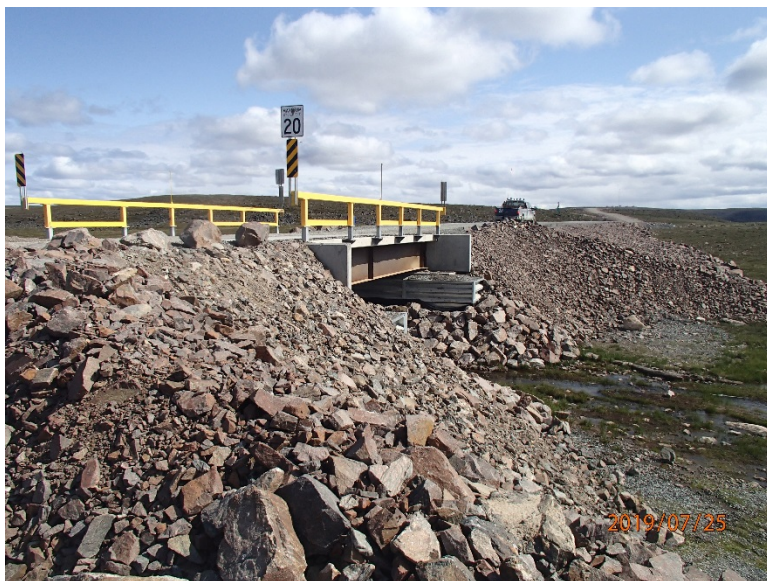
Photograph E3-8 Bridges 4 – km 20+000
