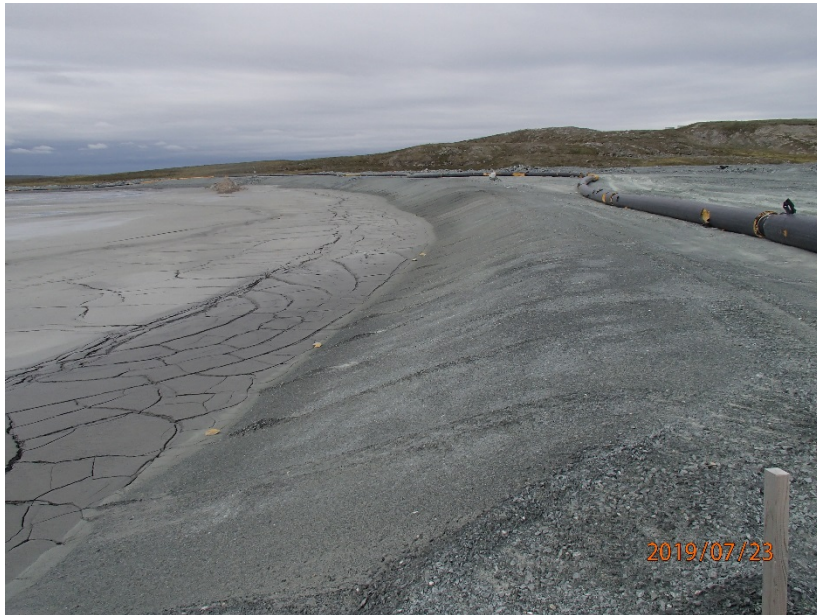
Photograph B1-6 Tailings Storage Facility
