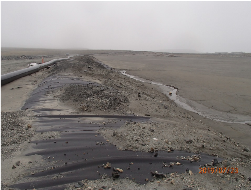
Photograph B2-7 Saddle Dam 1
