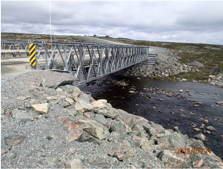
Photograph D3-5 Bridges 3 – R06 km 23+100
