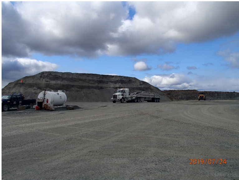
Photograph F-17: Quarry 11 – km 53+500
