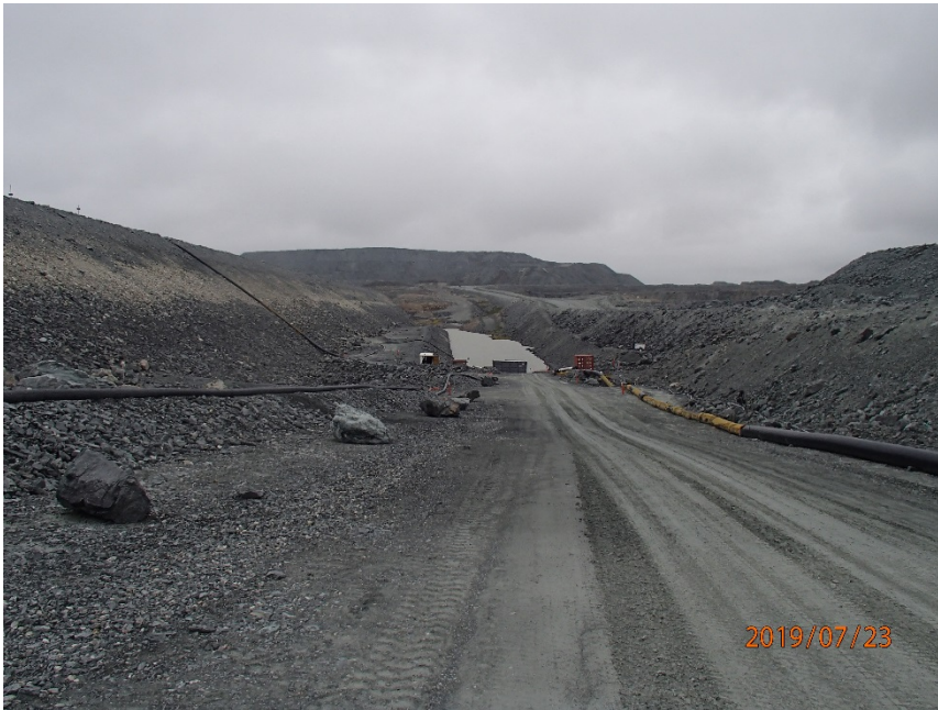
Photograph B7-9 Central Dike and Saddle Dam 5
