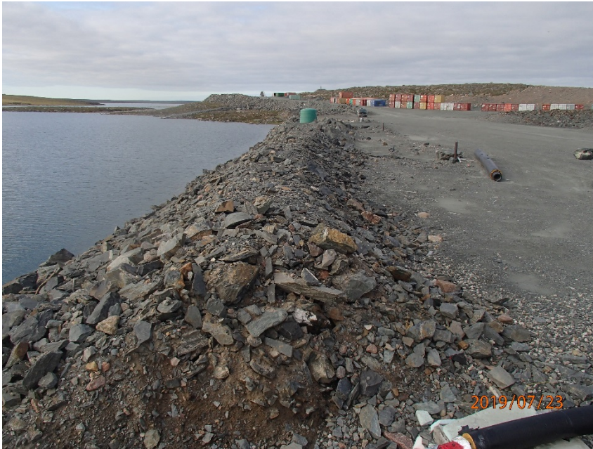
Photograph A1-7 East Dike
