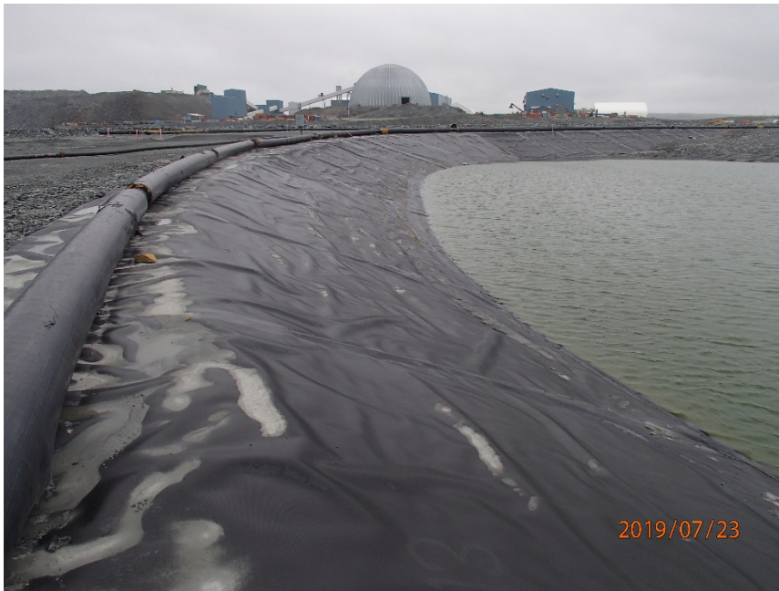
Photograph B7-11 Central Dike and Saddle Dam 5
