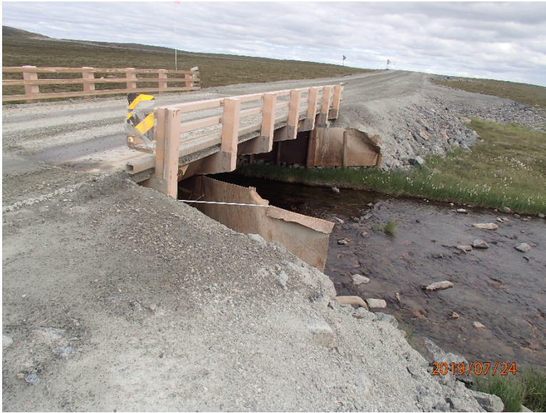
Photograph D3-15 Bridges 8 – R19 km 83+150
