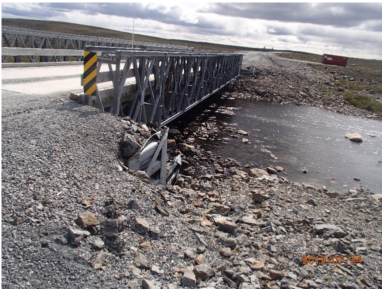
Photograph D3-10 Bridges 5 – R15 km 69+200
