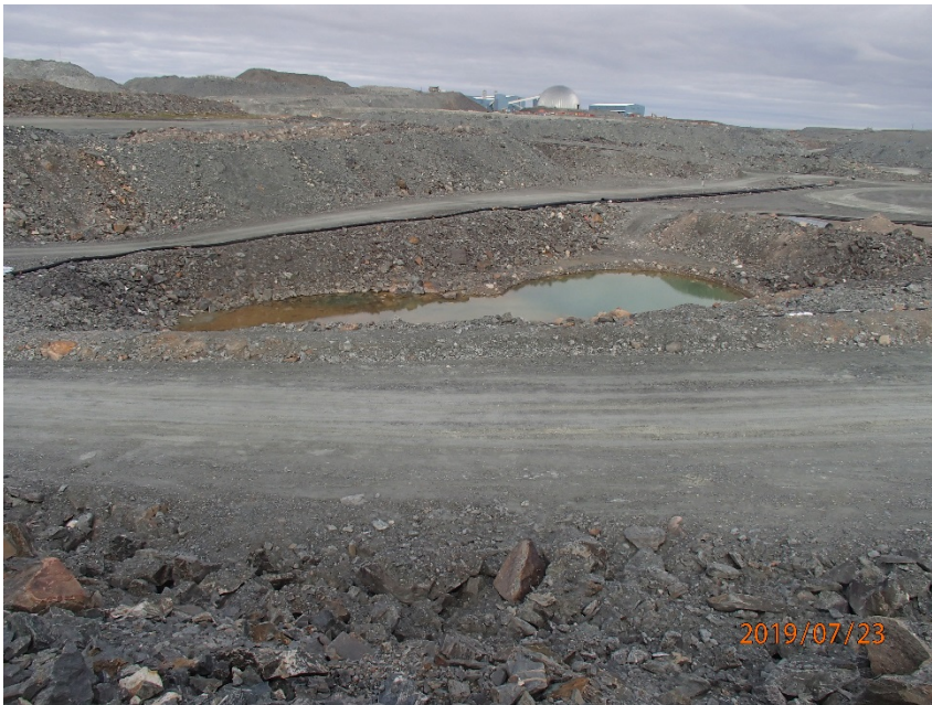
Photograph A1-8 East Dike
