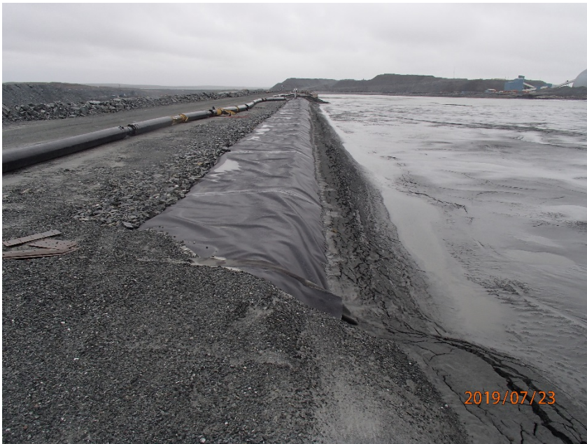
Photograph B7-2 Central Dike and Saddle Dam 5
