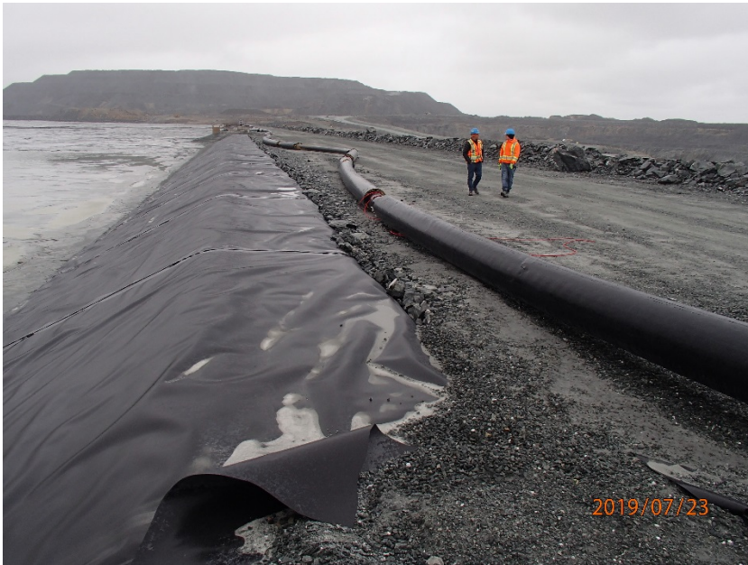
Photograph B7-5 Central Dike and Saddle Dam 5
