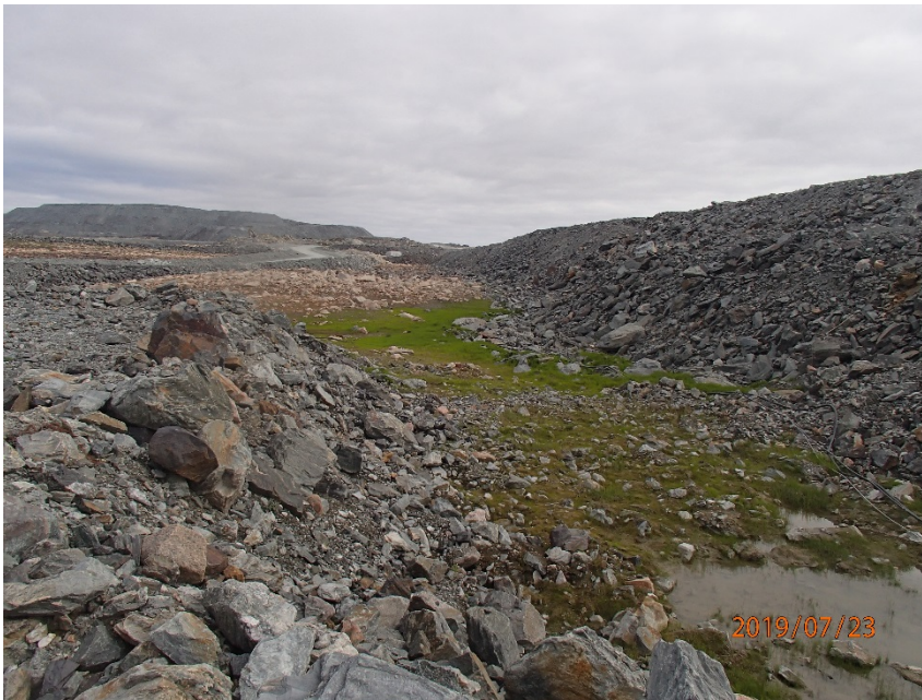
Photograph A1-11 East Dike
