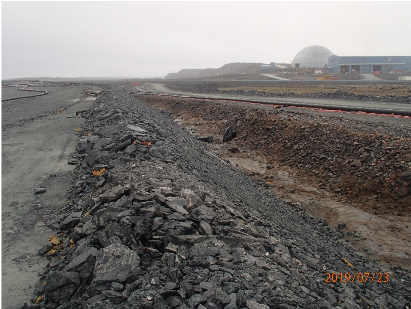
Photograph B6-1 Saddle Dam 4
