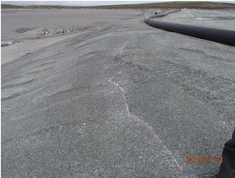
Photograph B1-3 Tailings Storage Facility
