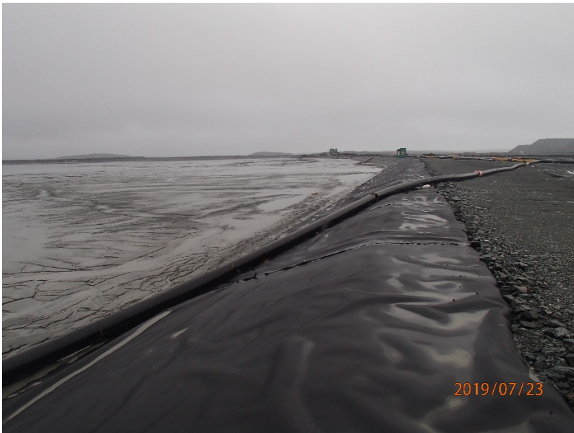
Photograph B6-3 Saddle Dam 4
