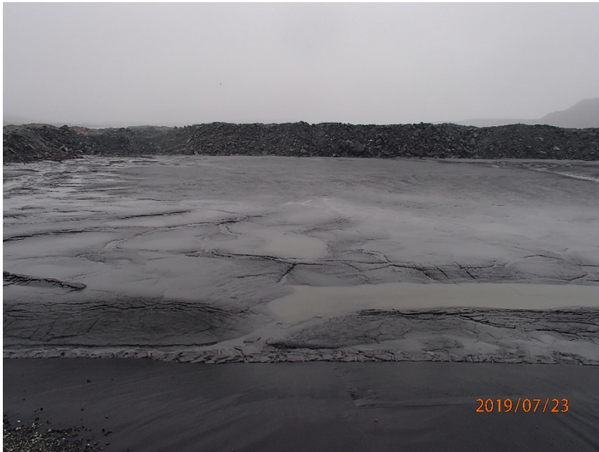
Photograph B4-7 Stormwater Dike
