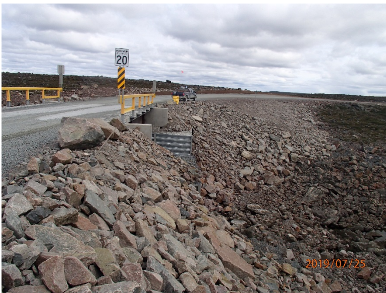
Photograph E3-12 Bridges 6 – km 26+100
