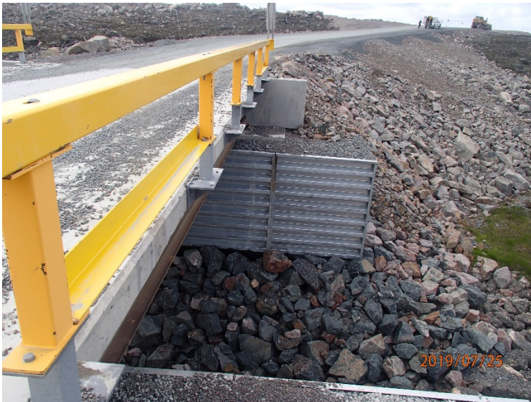
Photograph E3-11 Bridges 6 – km 26+100
