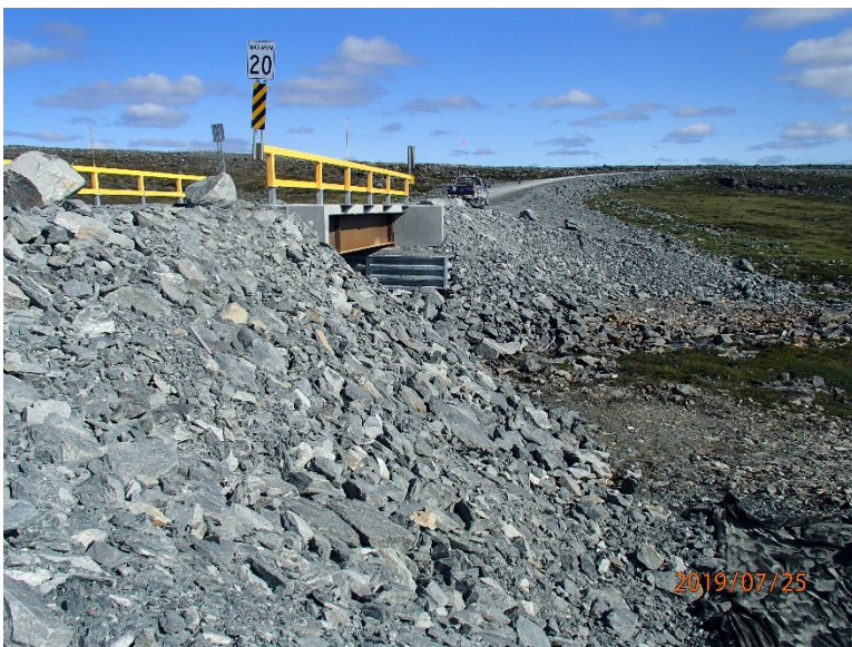
Photograph E3-2 Bridges 1 – km 3+400
