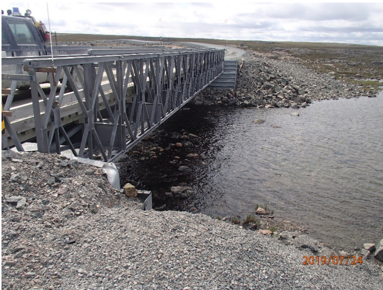
Photograph D3-6 Bridges 3 – R06 km 23+100
