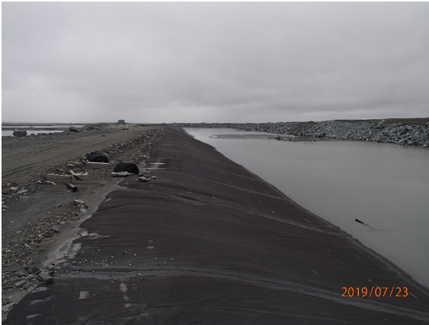
Photograph B4-3 Stormwater Dike
