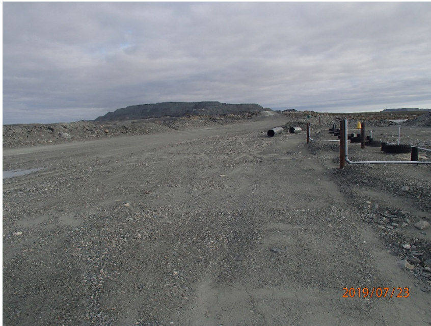
Photograph A1-1 East Dike
