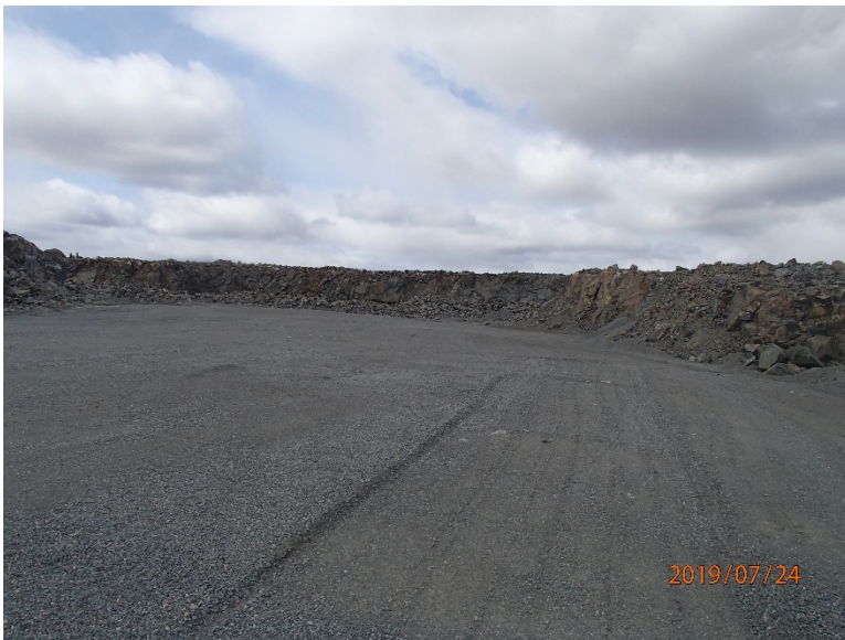
Photograph F-2: Quarry 2 – km 13+250
