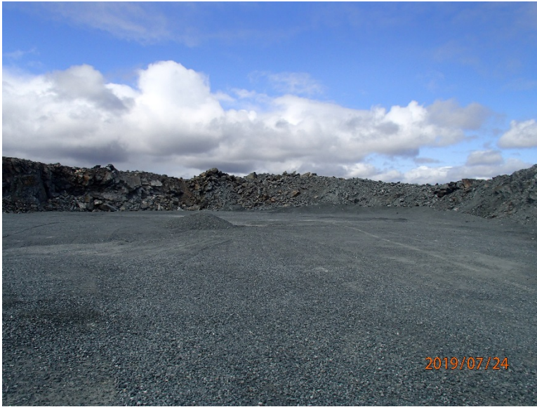
Photograph F-15: Quarry 9 – km 44+600
