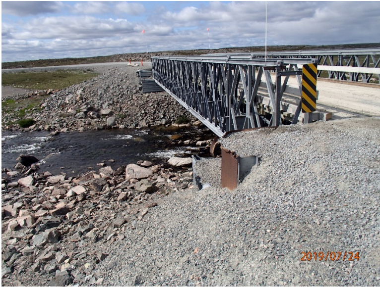
Photograph D3-1 Bridges 1 – R02 km 8+750
