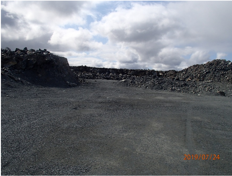
Photograph F-13: Quarry 8 – km 42+950
