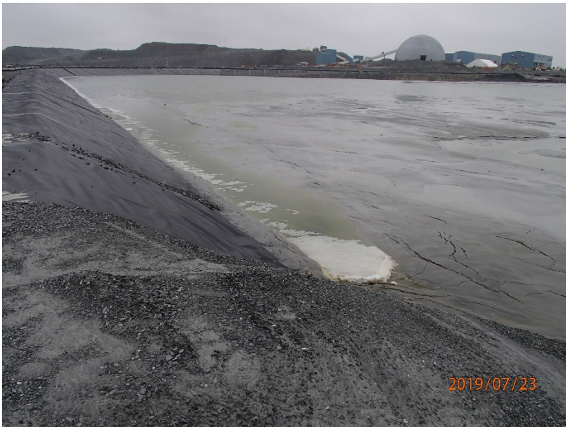
Photograph B7-6 Central Dike and Saddle Dam 5
